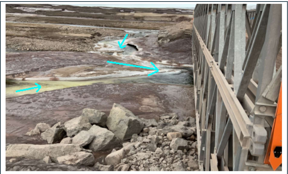
Figure 98: View of the two stable abutments with riprap scour protection at the east side of bridge KM97.
