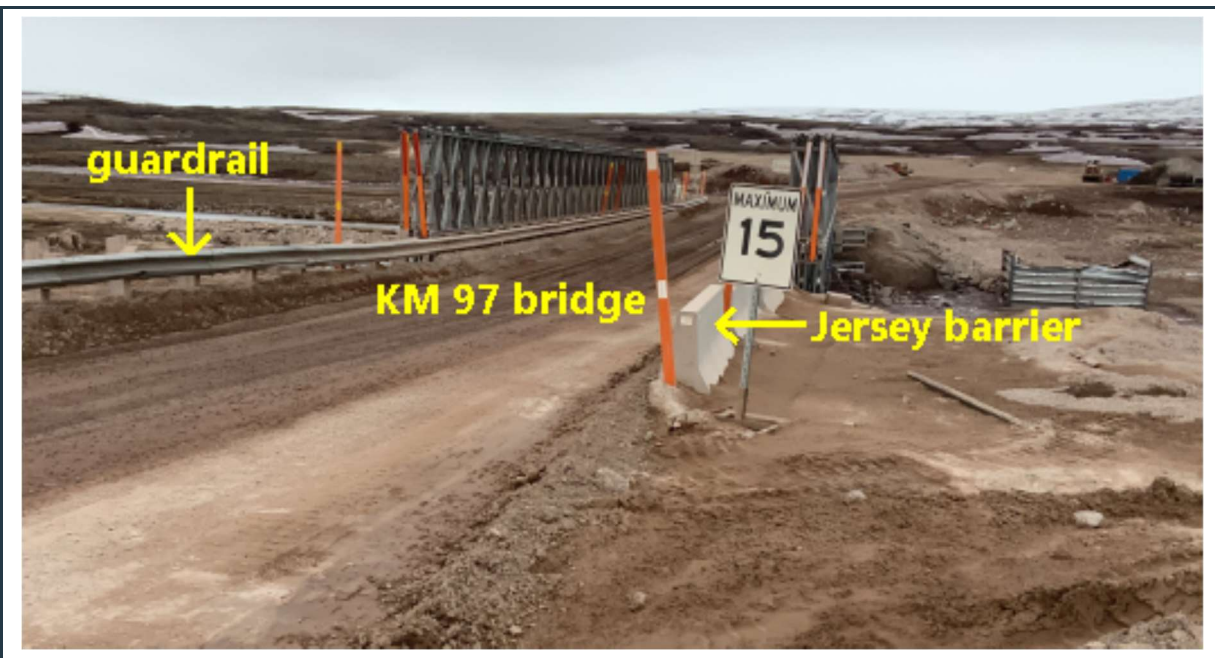
Figure 96: View of the approach embankment and abutment at bridge KM 97.
