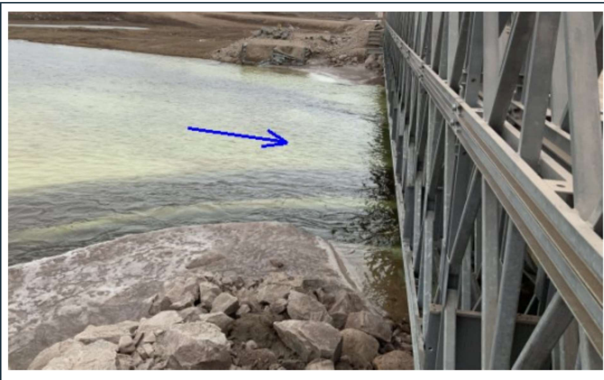
Figure 88: View of the stable abutments with riprap scour protection at the south side of bridge KM-17.
