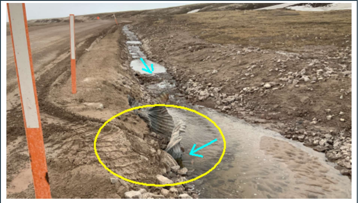
Figure 103: View of the damaged culvert at its inlet at KM 33+000. The culvert should be replaced as soon as practically possible. More rockfill should also be placed around the culvert's inlet.
