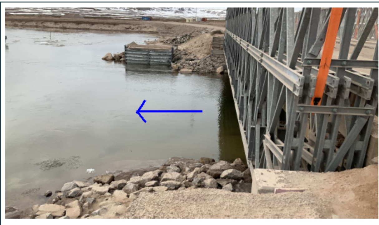
Figure 92: View of the west side of bridge 80, with riprap scour protection around the abutments.
