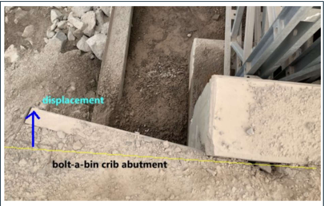
Figure 94: View of some displacement of the bolt-a-bin crib at one of the abutments at bridge 80.
