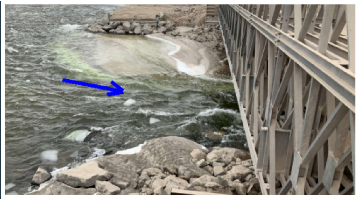
Figure 90: View of the stable abutments at the east side of bridge 63. Also note one of the two “old” abutments with riprap protection. Snow and ice still present around the abutments.
