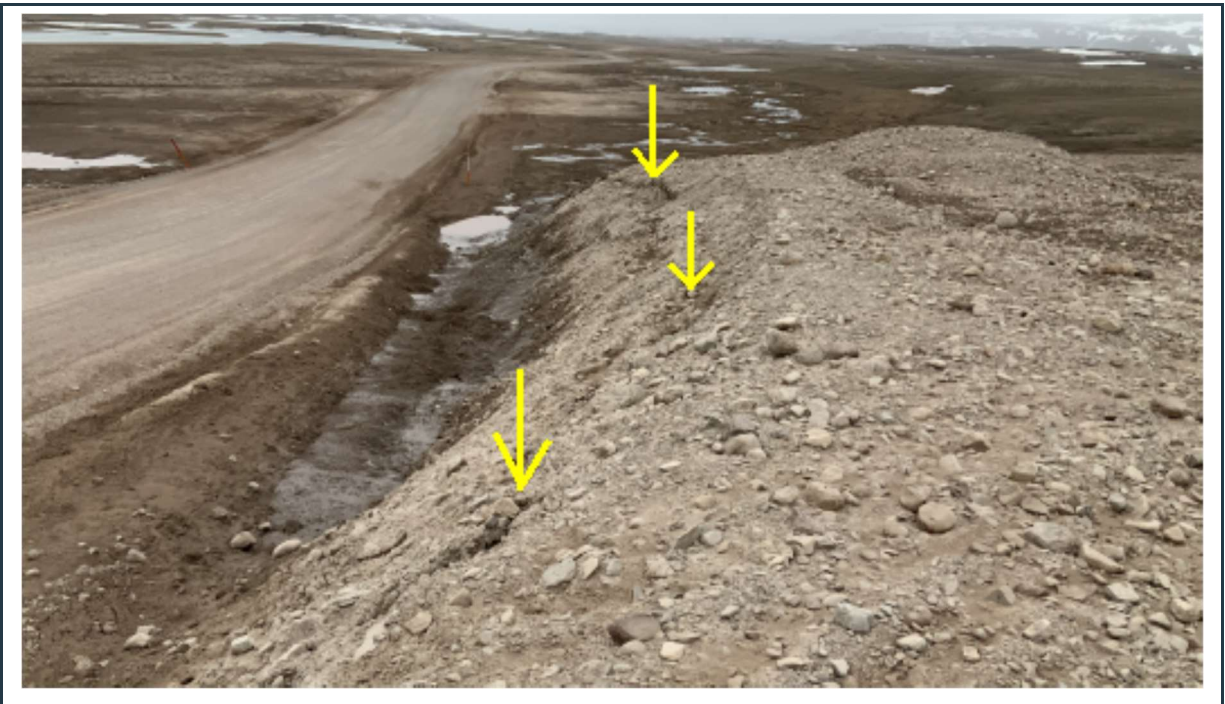
Figure 102: View of the slope at a cut section of the road at KM 28+900. Note the tension cracks on the crest of the slope (yellow arrows) due to freezing and thawing action. The slope should be monitored and reshaped to shallower inclination if necessary.
