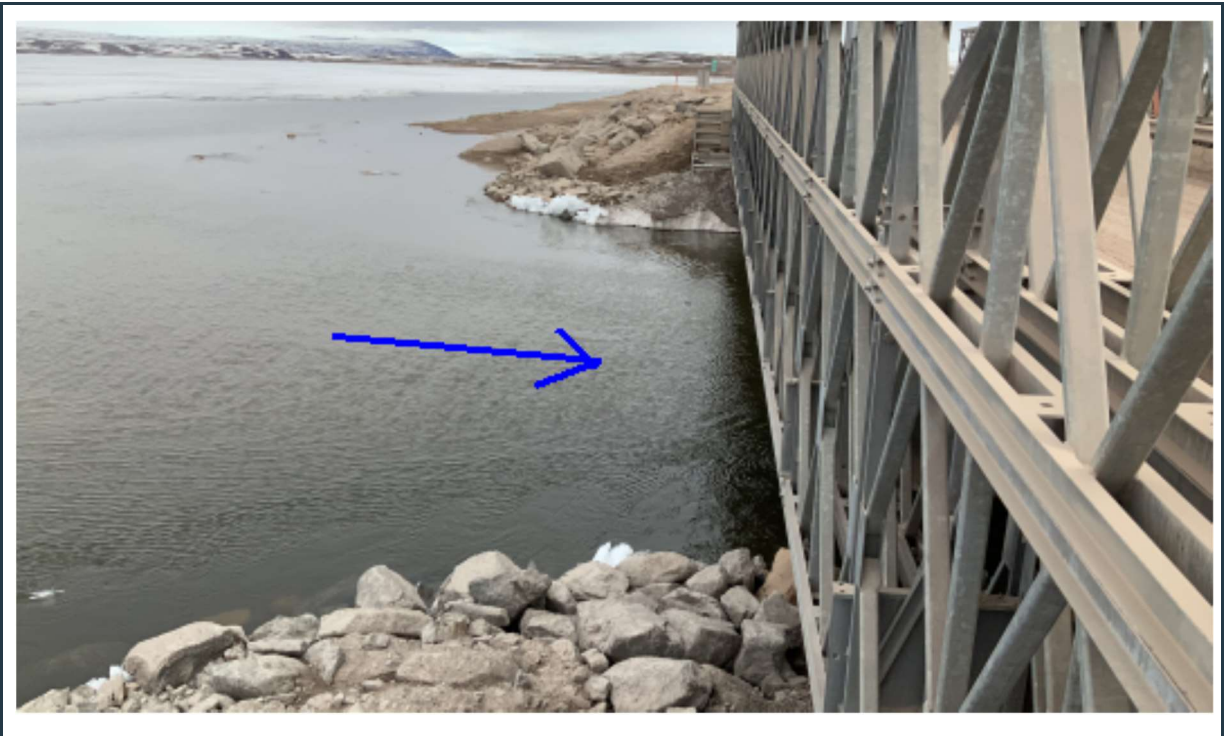
Figure 93: View of abutments with riprap scour protection at the east side of bridge 80.
