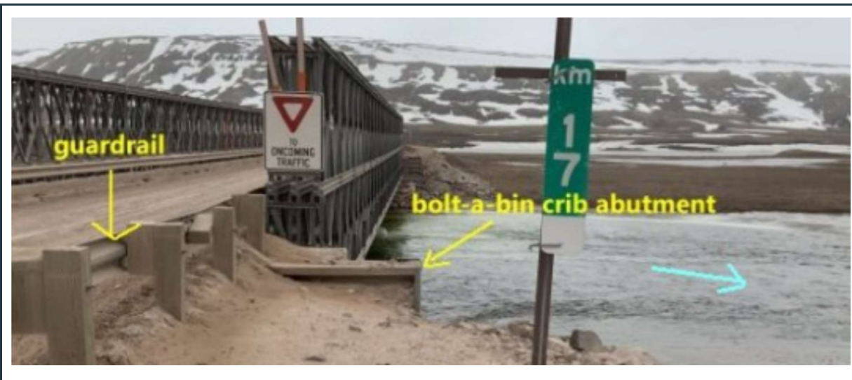
Figure 85: View of the north side of "bridge 17", with the bolt-a-bin crib abutment and guardrail.
