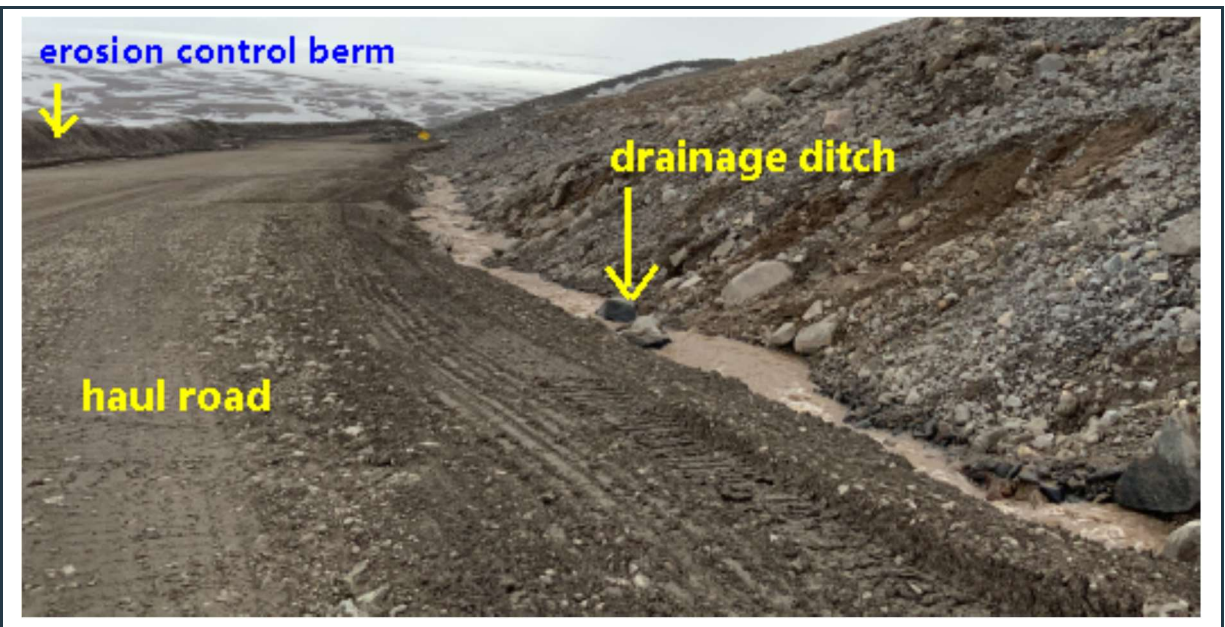
Figure 106: View of the well-maintained haul road between the crusher pad and the open pit around KM-107. Note the standard road components in the image, the safety berm along the fill (left) side of the road and the upgraded drainage ditch along the cut side (right) of the road.
