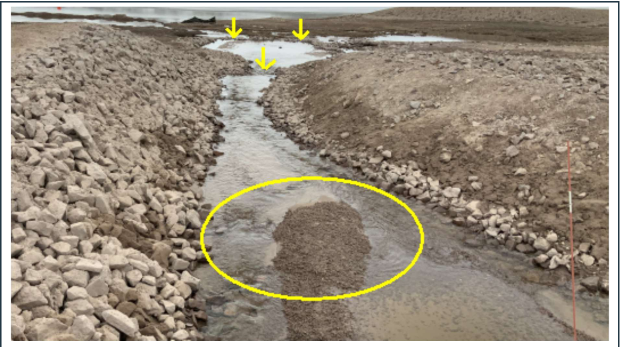
Figure 105: View of the ditch and check dams at KM 33+000. The ditch should be cleaned (yellow circle) and the crest of the check dams repaired/raised (yellow arrows) during culvert replacement.
