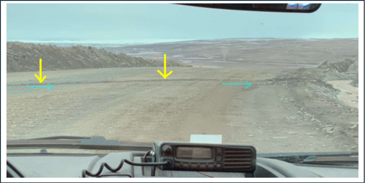
Figure 107: View of a cross drain (combination of a whoa-boy and shallow ditch) intercepting run-off flowing down the haul road and direct the collected water to the side-ditch. Many of such drains have been formed recently to improve erosion control along the haul road.
