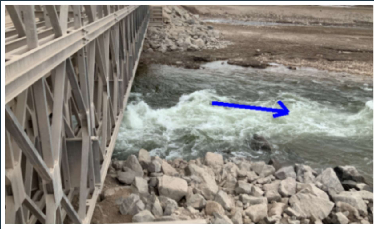
Figure 89: View of the west side of bridge 63, with stable abutments protected against scour.
