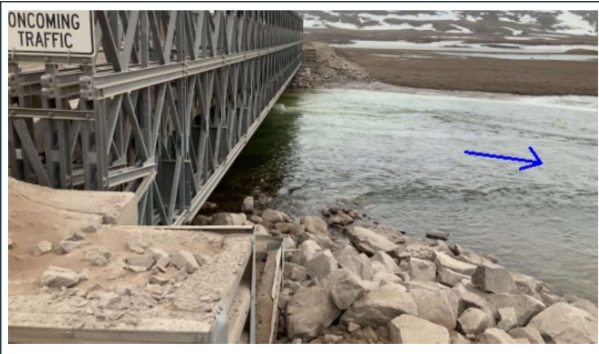
Figure 87: View of the stable abutments with riprap erosion protection at the north side of bridge KM17.
