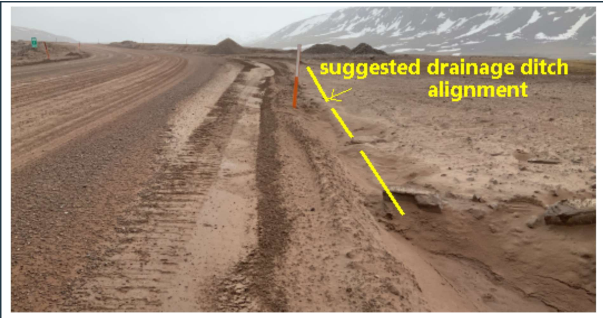
Figure 99: View of a section of the tote road around KM 06+900. Excavation of a drainage ditch is suggested to improve drainage of surface water from the road's surface.
