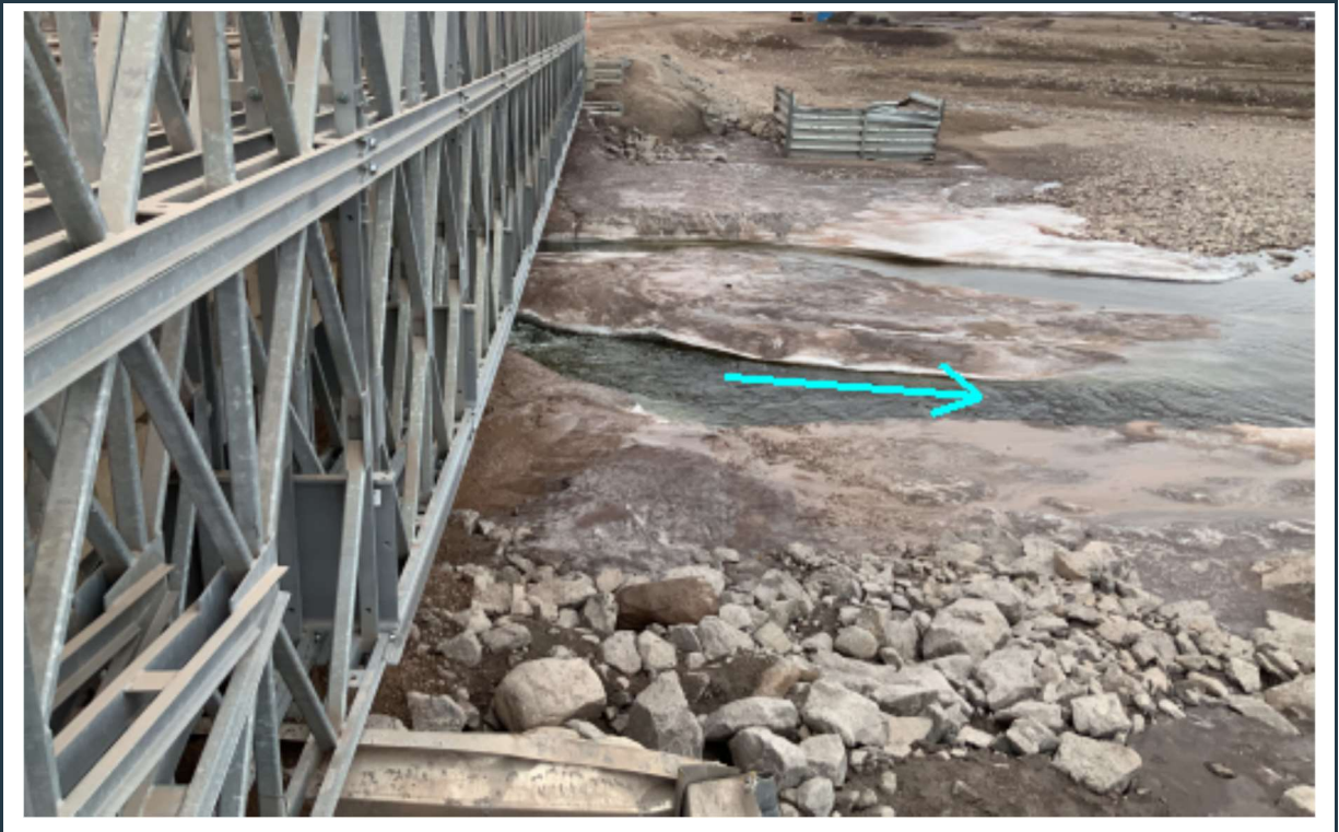
Figure 97: View of the stable abutments with riprap scour protection at the west side of bridge KM 97.
