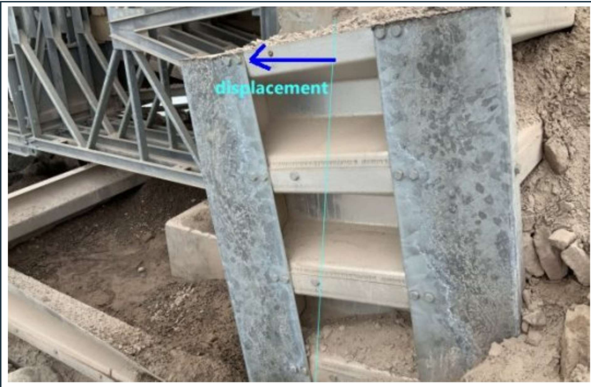
Figure 95: View of displacement/tilt of the bolt-a-bin crib at one of the abutments at bridge 80.
