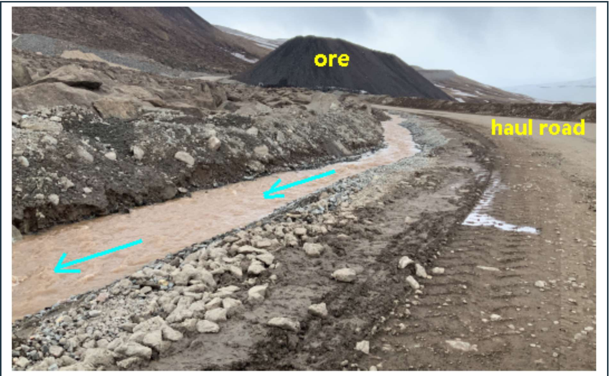
Figure 108: View of a section of the haul road near the ore stockpile (KM106) with improved side drainage ditch.
