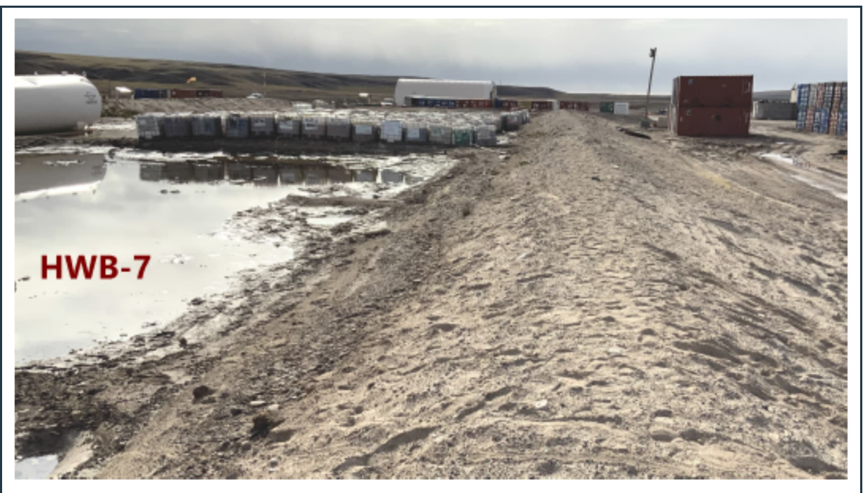
Figure 23: View of the stable berm around the HWB-7 cell, with an old fuel tank and oil filled plastic containers stored in the cell. The ponding water indicates good liner performance.
