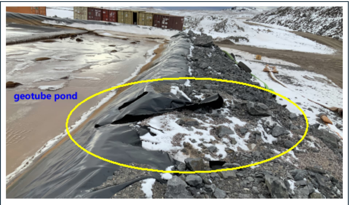
Figure 31: View of the perimeter berm around the geotube pond. A small section of the liner at the south-west section of the berm (yellow circle) is still damaged and will require repair.
