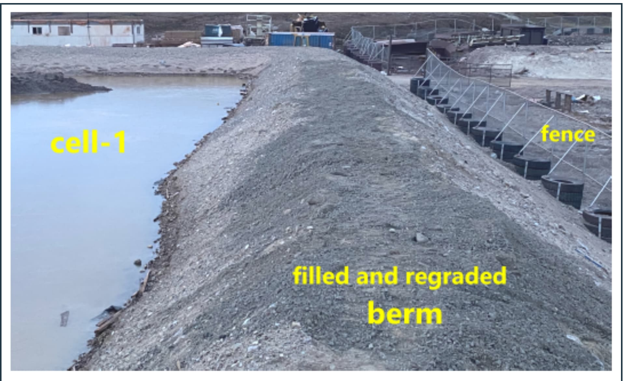
Figure 41: View of a section of the stable berm at the landfarm's Cell 1. Note that the settled anchor trench on the crest of the berm has been regraded and the exposed liner covered by Site Services, as specified in our earlier report (June 2023).
