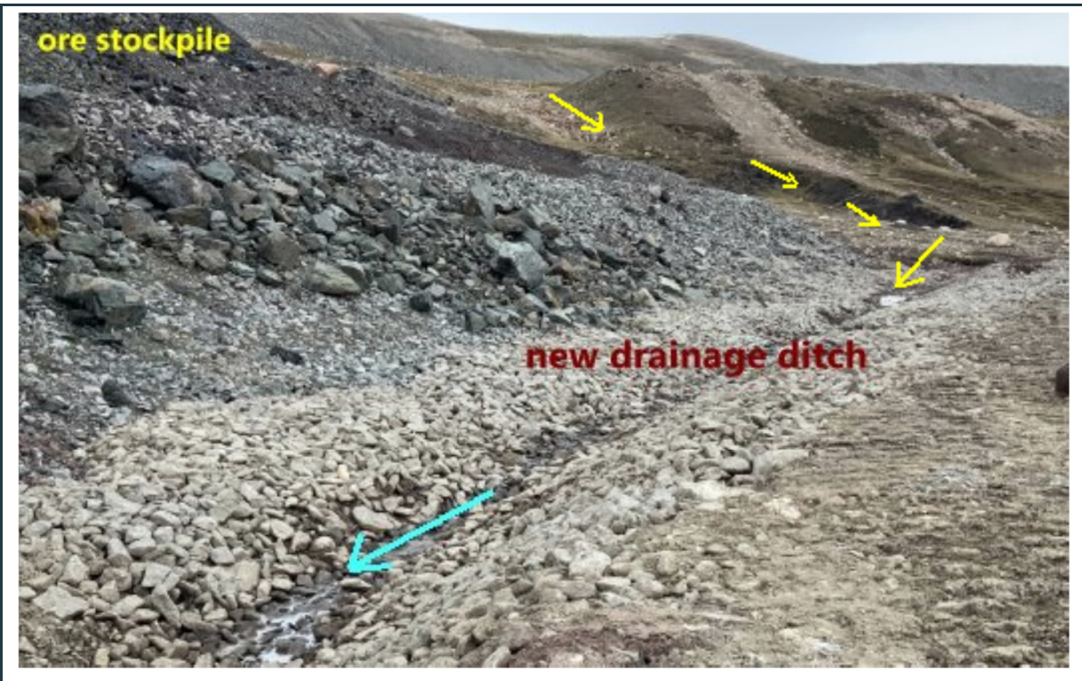
Figure 50: View of the new drainage ditch south of the KM-106 ore stockpile area, collecting local run-off (yellow arrows).
