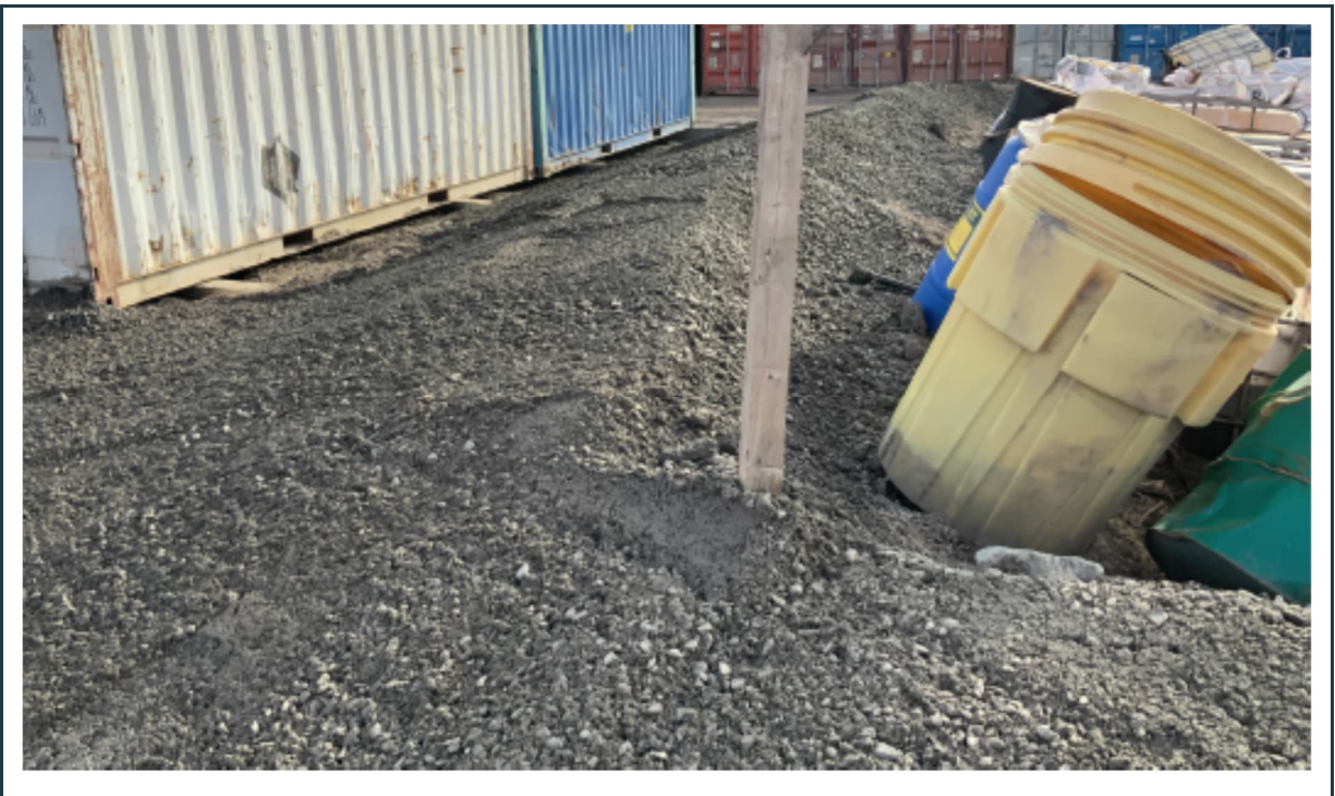
Figure 22: View of the north-east corner cell HWB-6 one day after the initial inspection. Note that the problem with the berm had been rectified by site services (all boulders have been removed).
