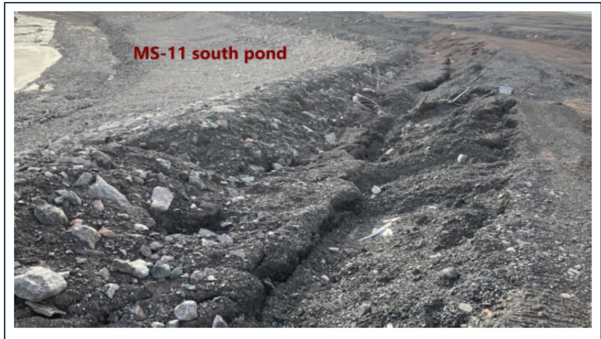
Figure 34: View of the loosely filled liner anchor trench along the road next to the south MS-11 pond's slope. The open gaps do not appear to be related to slope movements, but they should be backfilled and regraded to minimize water infiltration into the ground next to the slope.
