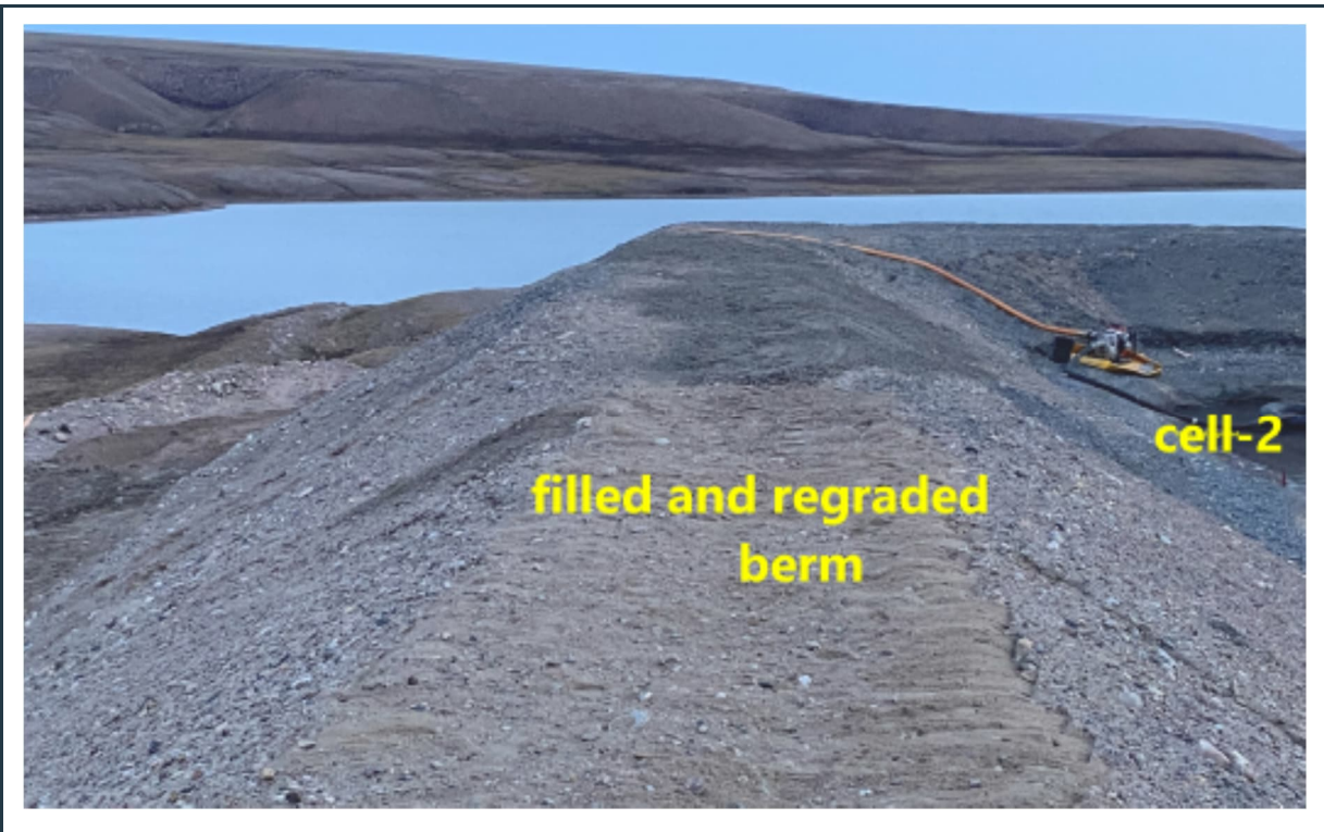
Figure 42: View of the currently empty cell-2 at the new landfarm. Note that the previously exposed liner has been covered and the anchor trench filled as specified in our earlier report.
