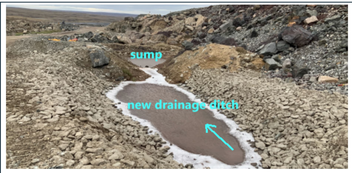
Figure 51: View of the new drainage ditch and sump (under construction) south of the ore stockpile area. Placement of riprap is required on the slopes of the sump as well.
