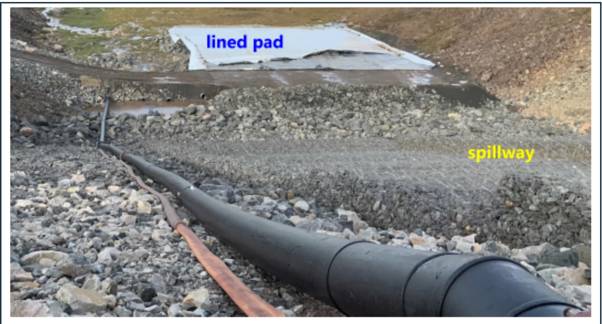
Figure 33: View of the robust and stable emergency spillway (gabion baskets and blankets filled with crushed rock) at KM105. Note the lined, compacted pad that will support geotubes at that location.
