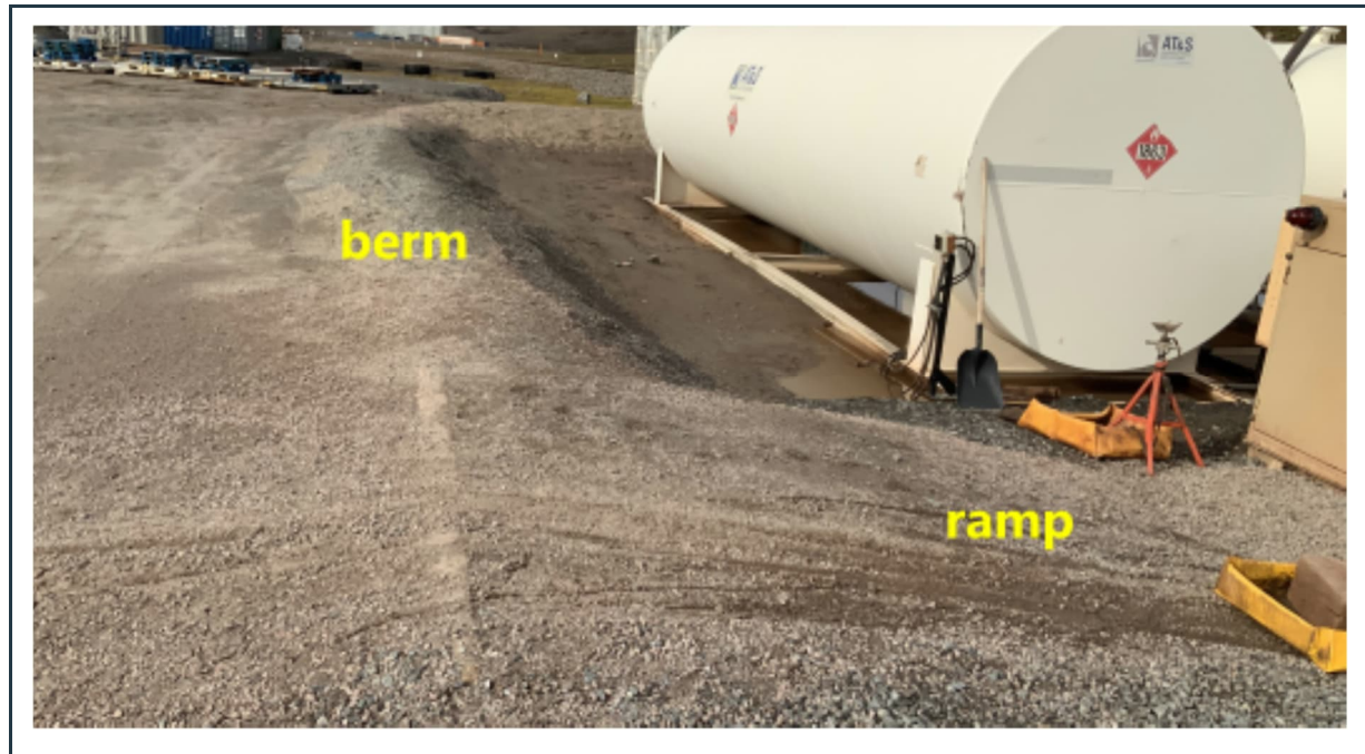
Figure 36: View of the well-maintained sand and gravel berm and access ramp at the lined jet-fuel storage facility. Ponding water in the cell indicates good liner performance.
