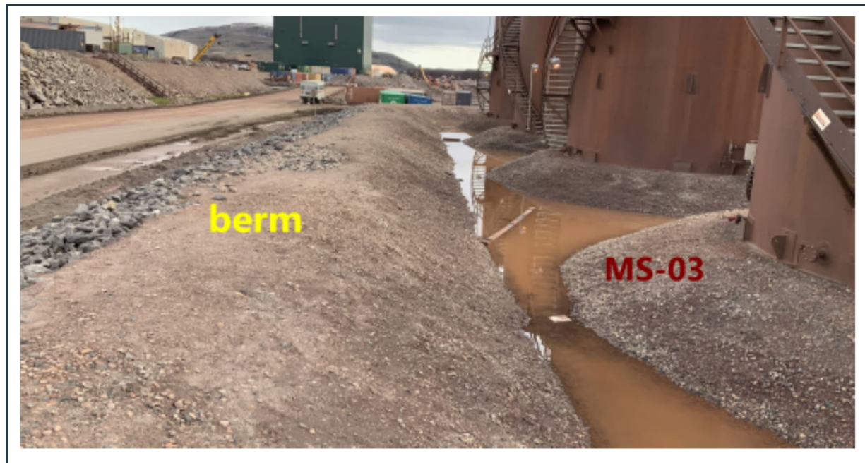
Figure 37: Well-maintained, stable berm around the MS-03 diesel fuel farm, with some ponding water, which is indication of good liner performance. Note the rock fill on the downstream slope.
