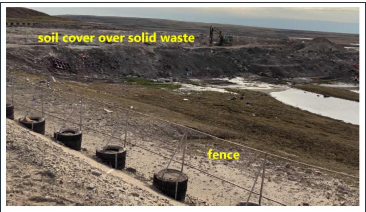
Figure 40: View of soil cover over non-hazardous solid waste in the fenced-in, gated landfill facility.
