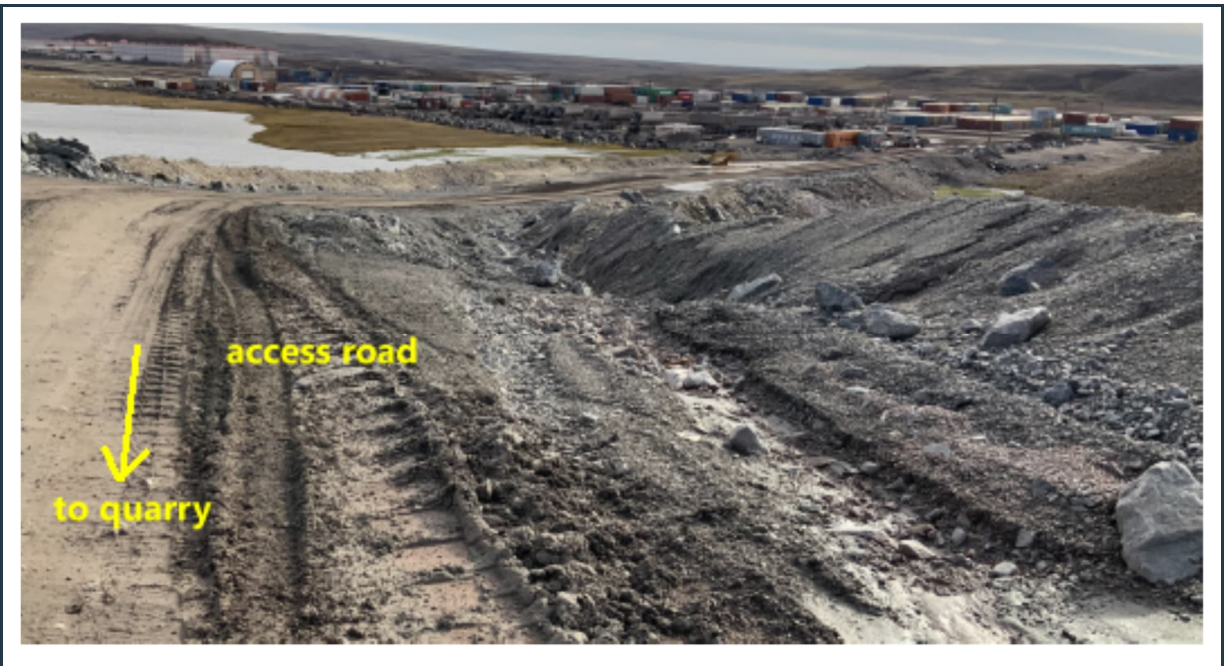
Figure 48: Erosion problem still exists along the edge of the access road to the quarry.
