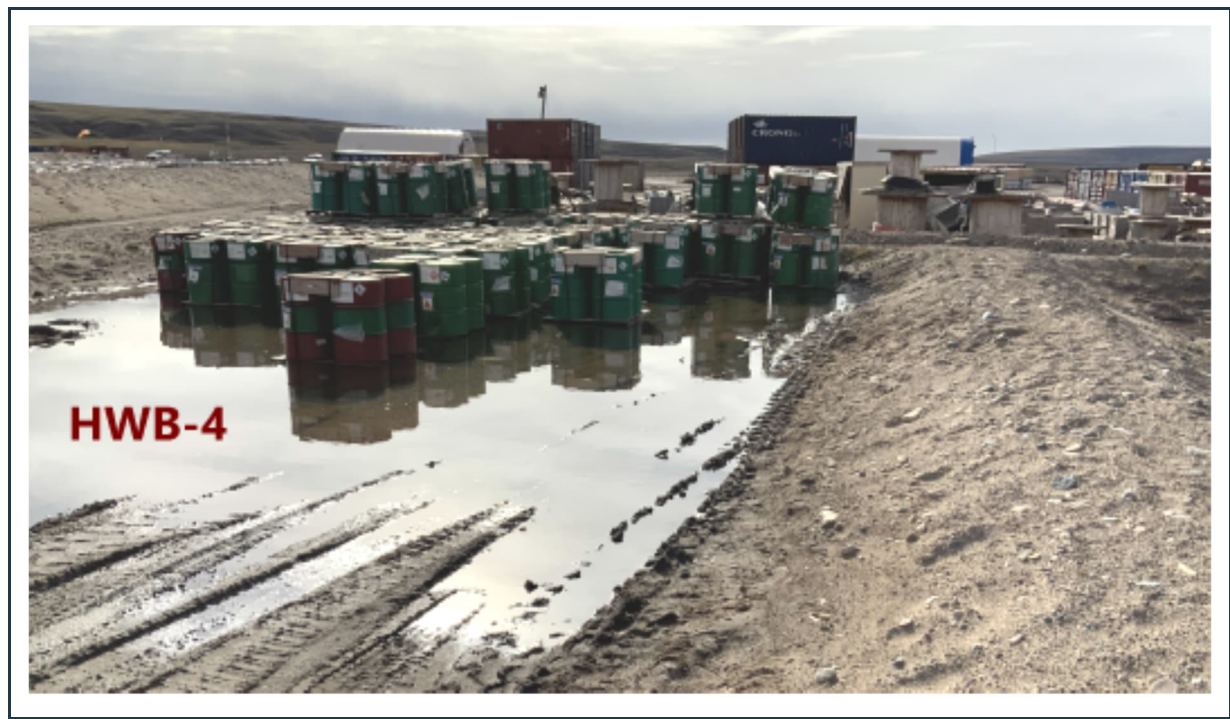
Figure 19: View of stable berms around the HWB-4 cell, with fuel barrels on wooden pallets stored in the cell. The shipping container and debris that were visible in June in this cell, have been removed.
