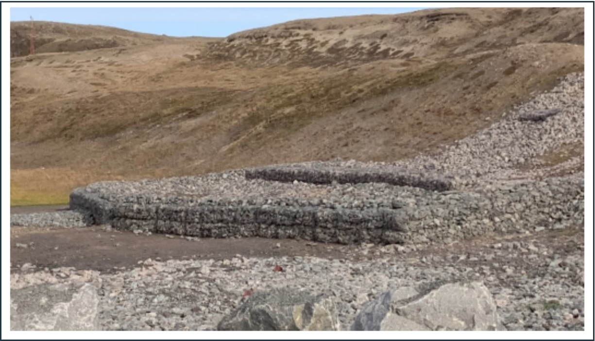
Figure 44: View of the new check-dam and riprap cover adjacent to Camp Lake to capture suspended solids potentially eroding from the airfield area and to prevent siltation in the lake.
