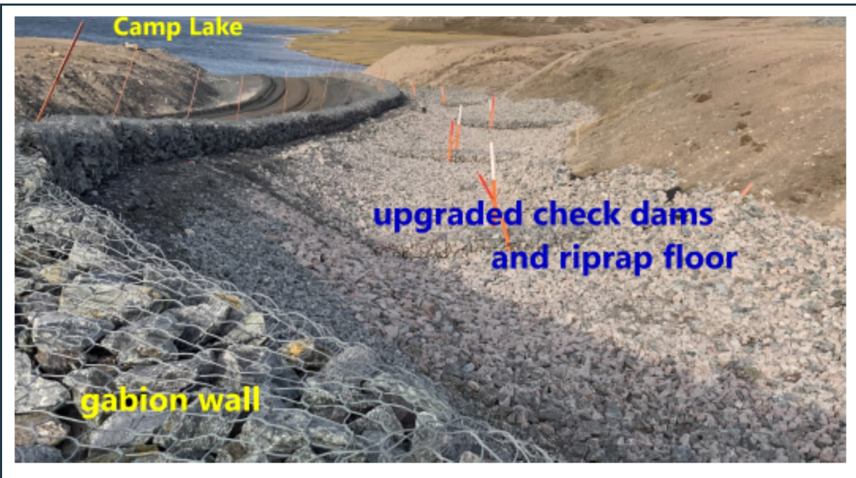
Figure 43: View of the upgraded Camp Lake check dams and new gabion wall along the road to the lake.
