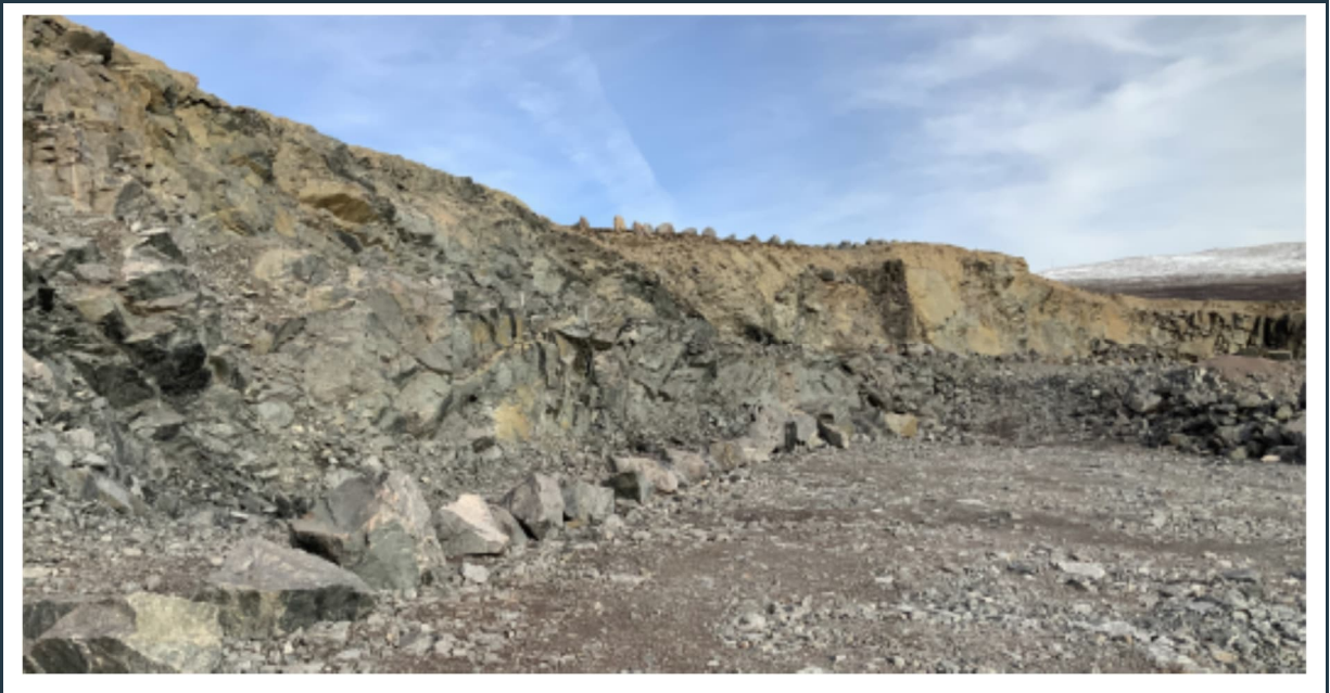
Figure 46: View of the stable rock face at the upper quarry level with protective boulders placed along the toe and crest of the rock cut. No activity is currently carried out in this quarry.
