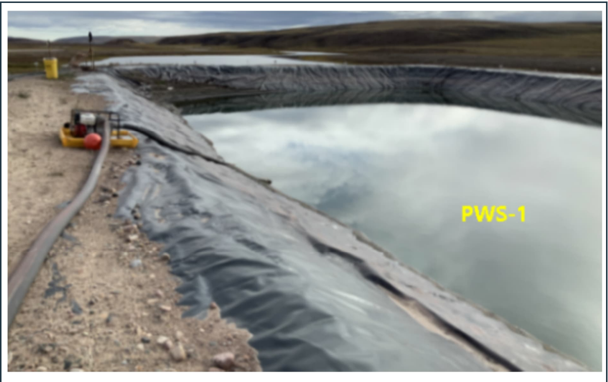
Figure 13: PWS pond #1. Well-maintained, stable perimeter berm and intact liner at the pond.
