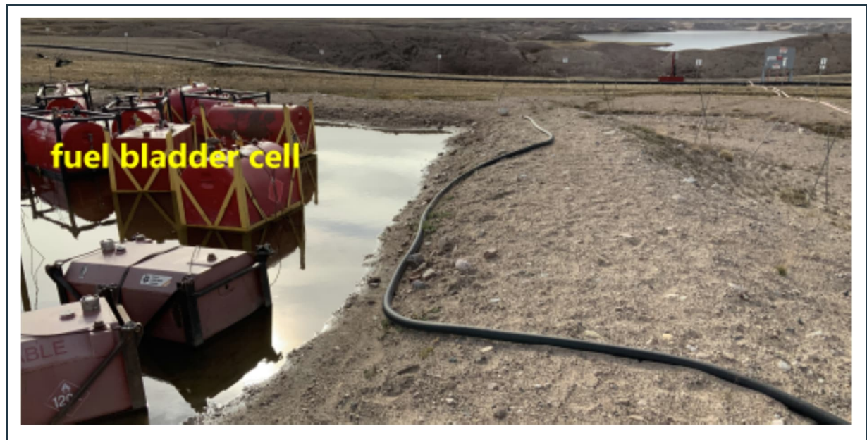
Figure 35: View of the stable berm around the "fuel bladder" cell. The ponding water in the cell indicates good liner performance.
