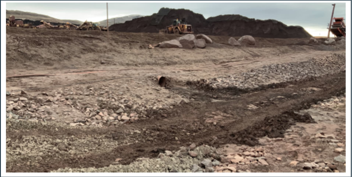
Figure 24: View of the discharge end of the recently cleaned culvert, draining the collected surface water from the crusher area to the MS-06 pond.
