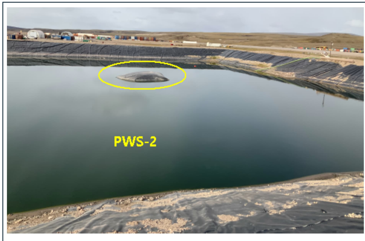
Figure 14: PWS pond #2 with stable, well-maintained berms and liner. – A section of the liner is visible in the pond above the water (yellow circle), which does not pose a risk to the integrity of the liner.
