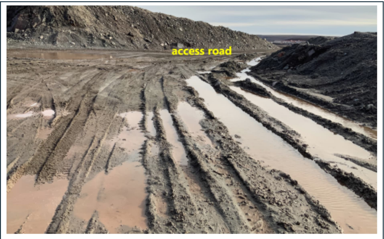
Figure 47: Drainage problems still exist at the first quarry level. Surface drainage shall be rectified.
