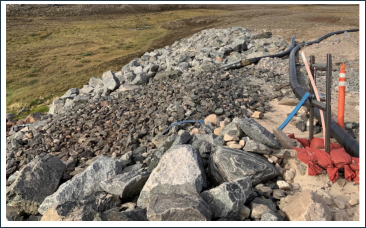
Figure 45: View of the stable rockfill riprap slope at the water discharge area.
