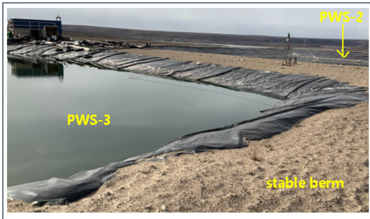
Figure 15: Robust, stable perimeter berms around PWS pond #3
