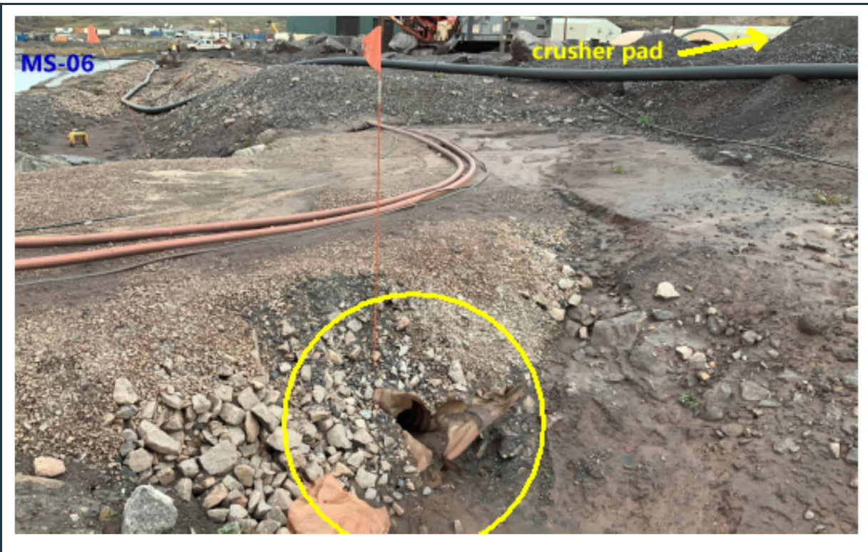
Figure 26: View of the side-ditch and culvert leading to the MS-06 pond. Based on field observation, the culvert requires cleaning (removal of trapped silt and sand from the pipe).
