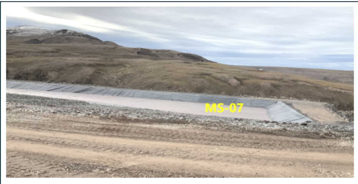
Figure 27: View of the robust, stable berms and intact liner at the MS-07 surface-water management pond.
