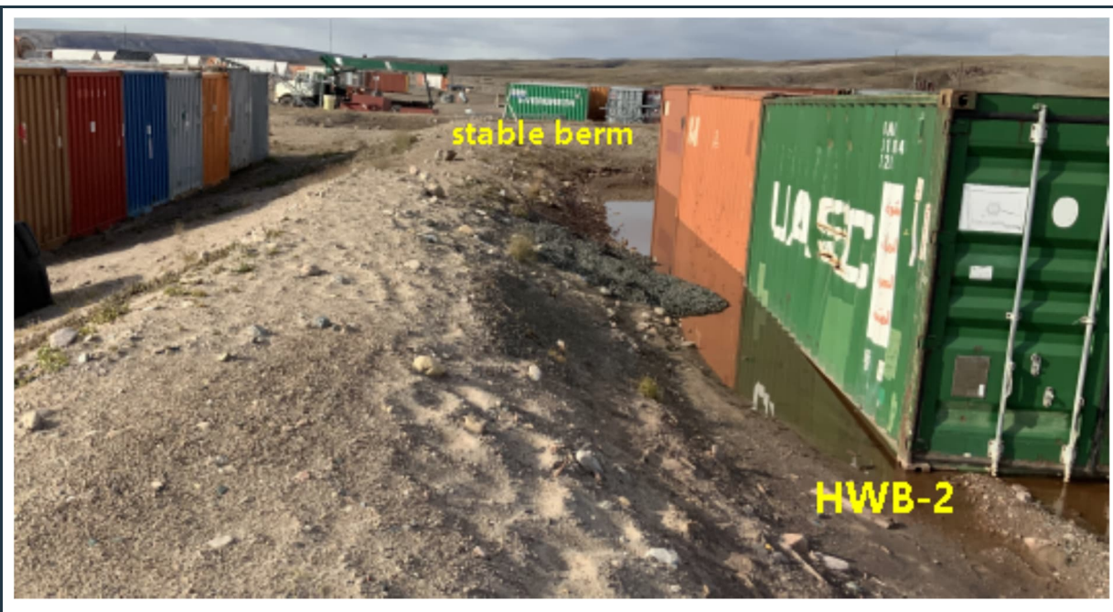
Figure 17: View of the robust, stable berms around HWB-2. The presence of water in the cell indicates good liner performance.
