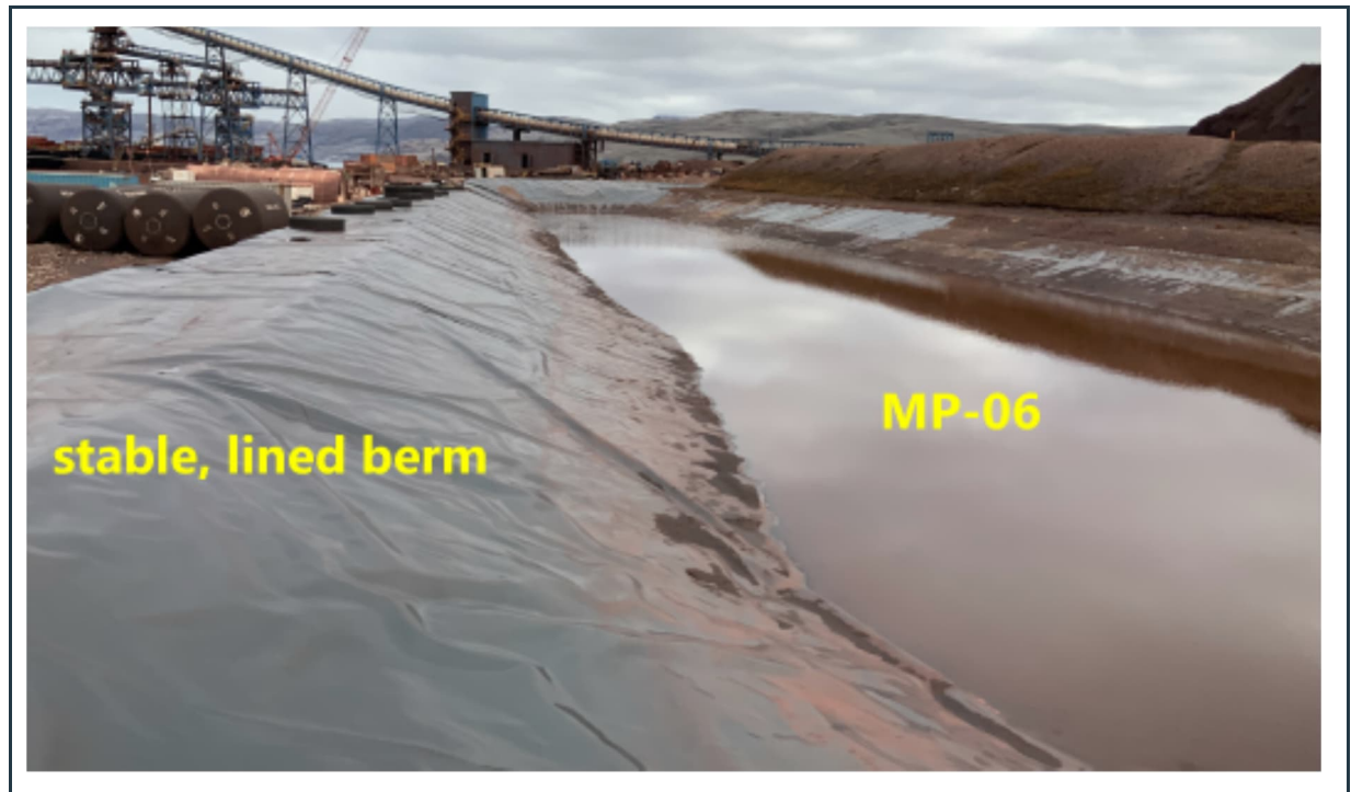
Figure 66: View of the lined MP-06 pond with robust, stable berms.
