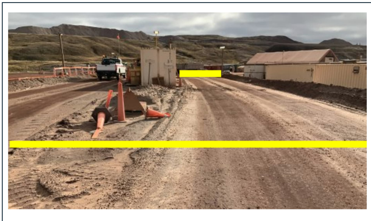
Figure 91: The yellow lines indicate where the drainage control humps should be provided.
