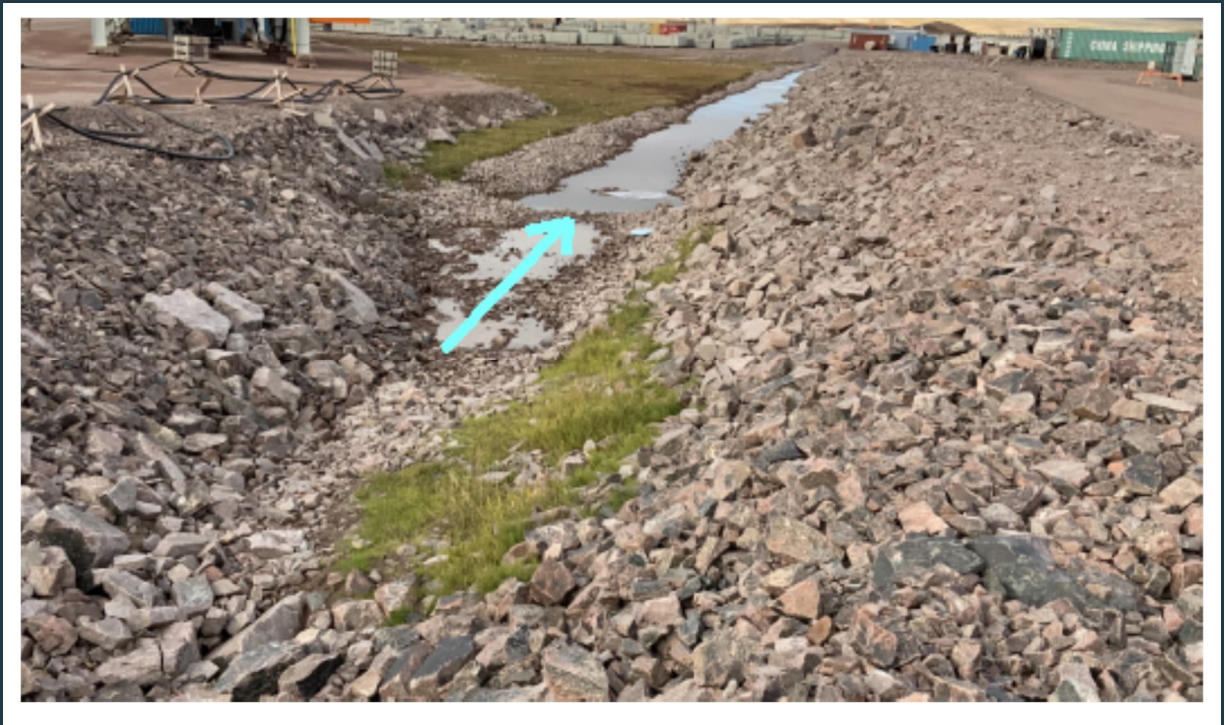
Figure 80: View of the south section of the 380-Person Camp surface water collection ditch.
