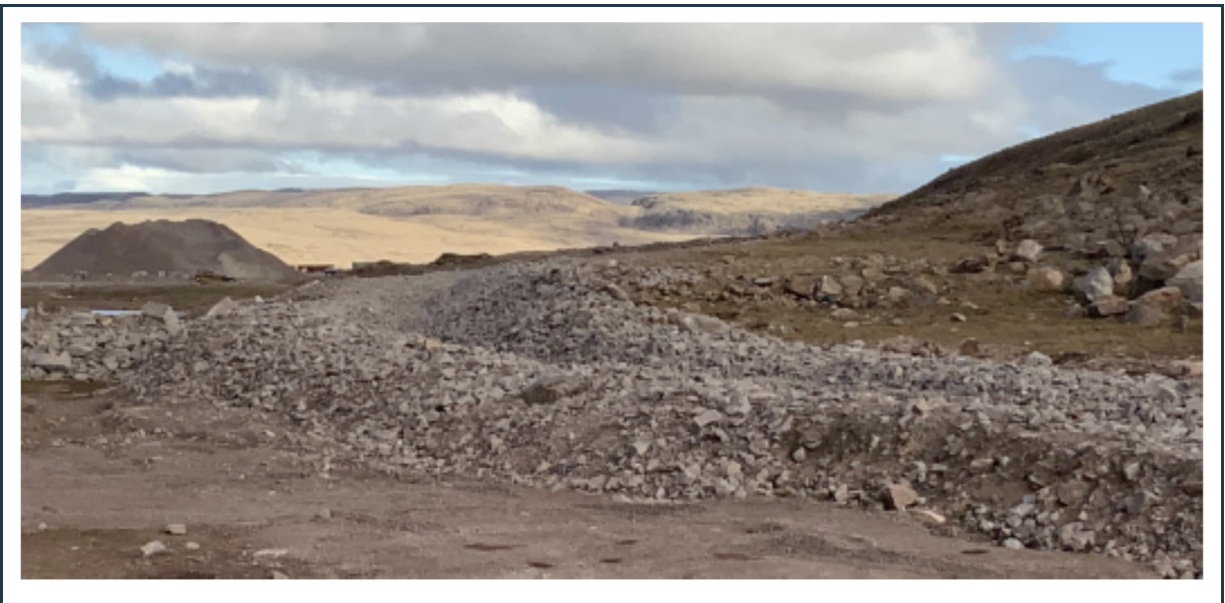
Figure 75: View of the P-SWD-6 surface water collection ditch. No water is drained from the quarry in this ditch with its invert level constructed above the lower level of the quarry.
