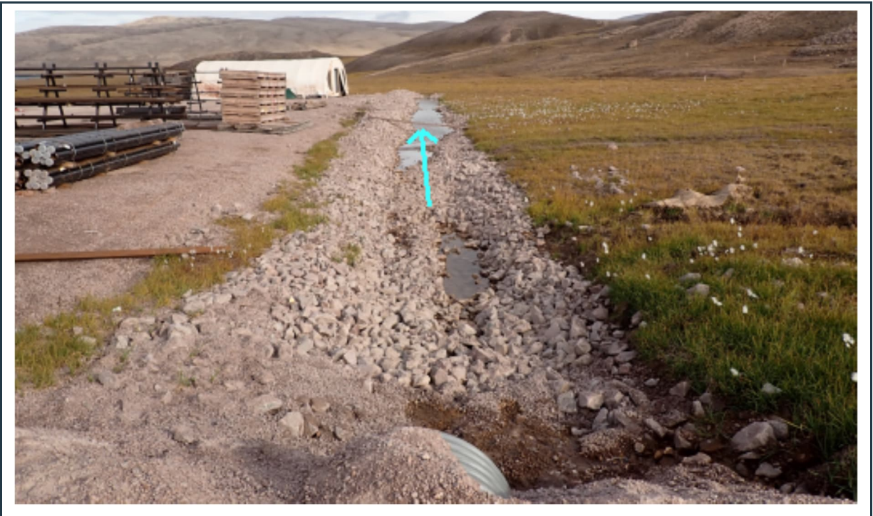
Figure 72: View of the northern section of the P-SWD-3 surface water collection ditch with failed slopes and ponding water. The ditch should be reconstructed with flow direction shown in the image.
