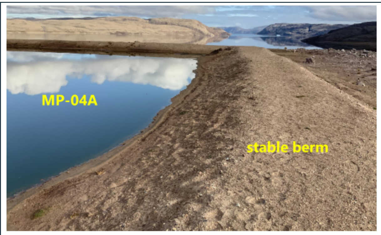
Figure 61: View of the lined MP-04A contaminated snow disposal cell with stable berms. The ponding water (melted snow) indicates good liner performance.
