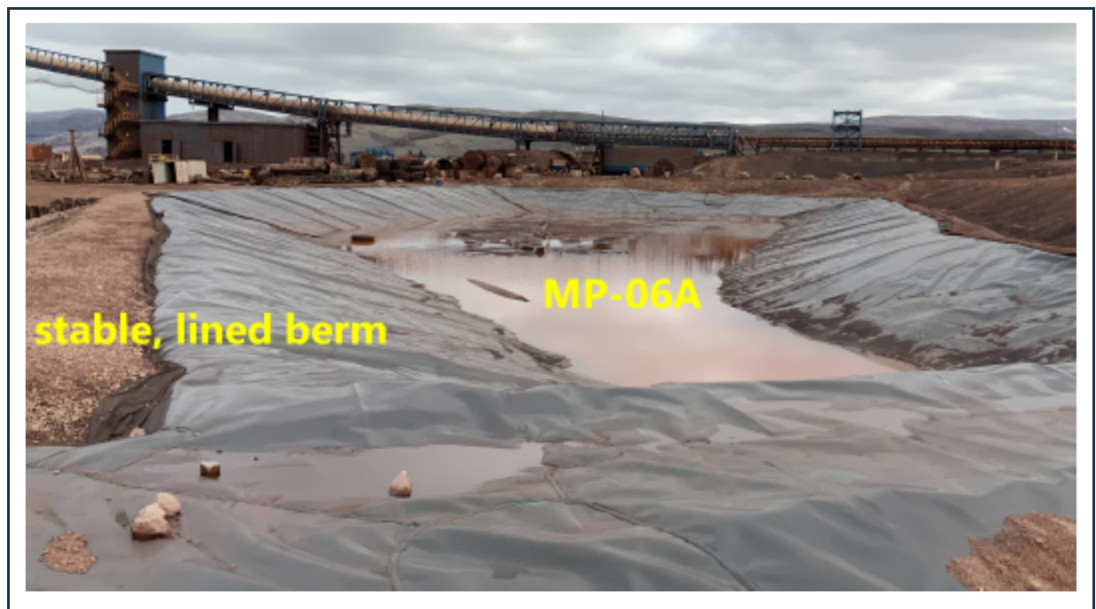
Figure 67: View of the lined MP-06A overflow pond with robust stable berms.
