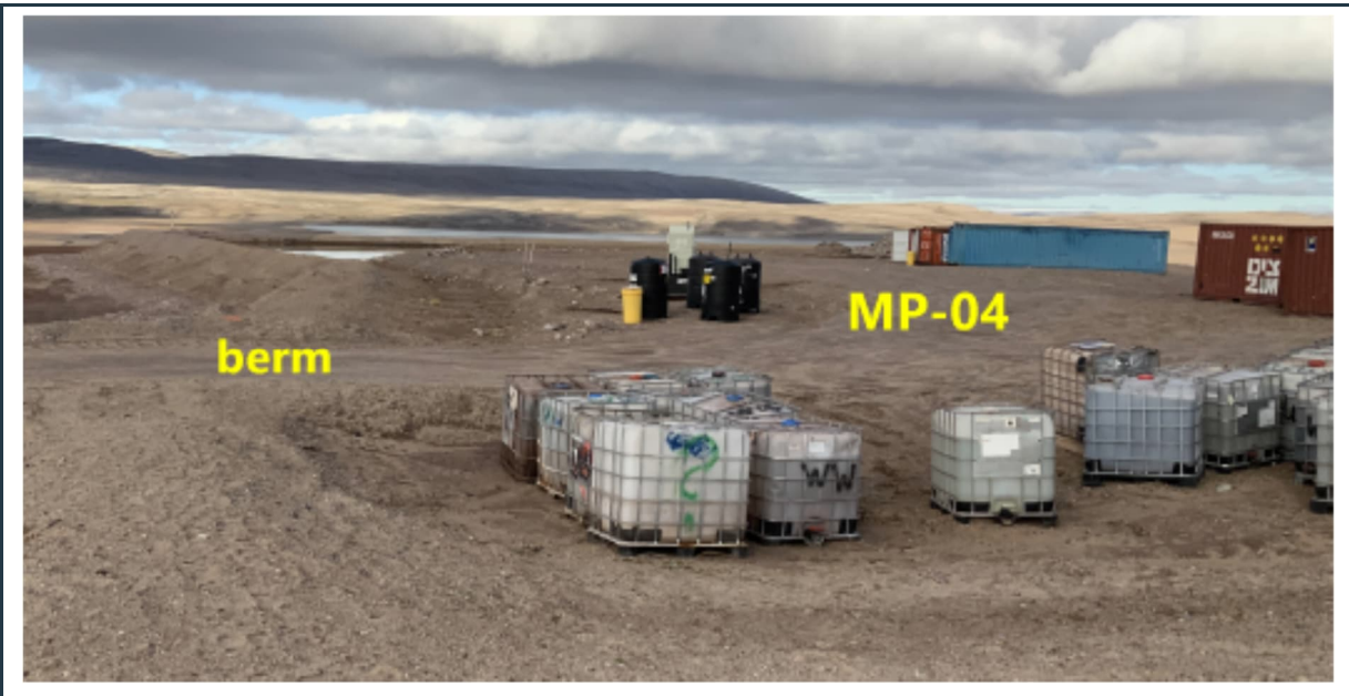
Figure 60: View of stable berm around the MP-04 land-farm, with ponding water in one corner of the cell. In addition to the buried waste, shipping and plastic containers are stored in the cell.
