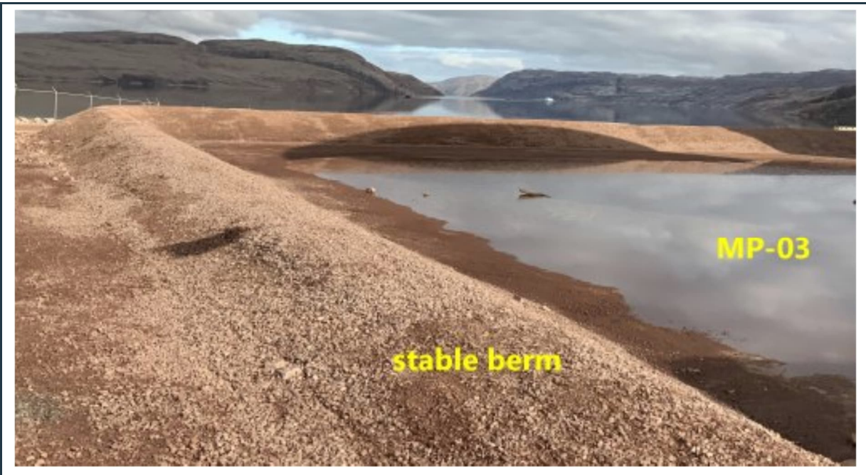
Figure 58: View of the well-maintained stable berms around the lined MP-03 fuel tank farm. The ponding water indicates good liner performance.
