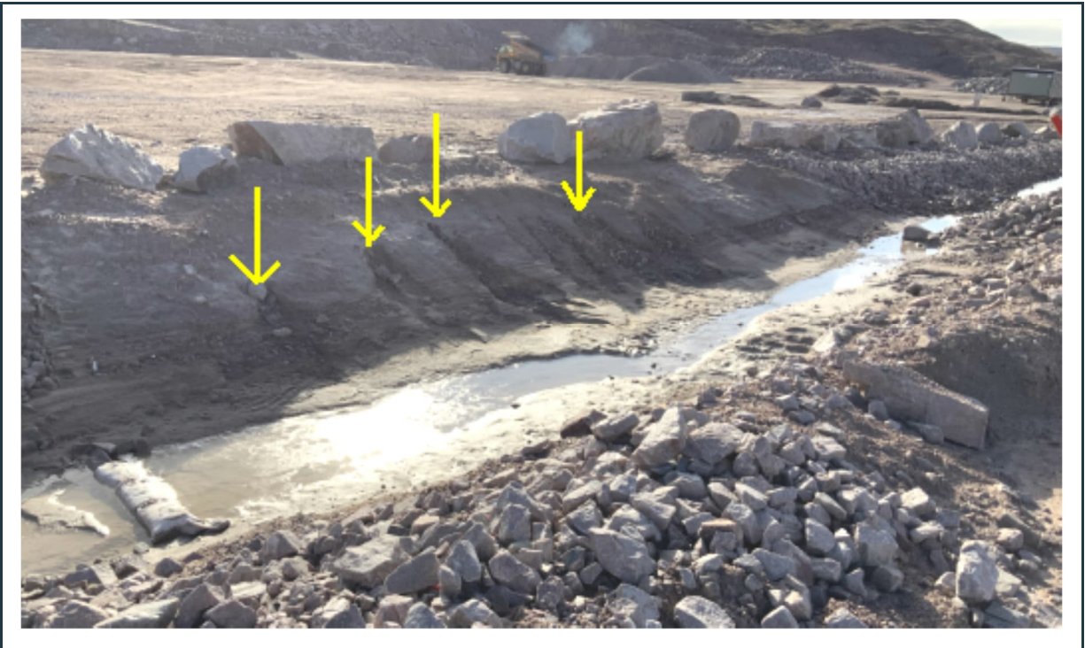
Figure 74: P-SWD-5 – “Q01-North” surface water collection ditch with missing riprap at one section of the ditch. Note the continuous seepage from the granular fill of the quarry’s lower level.
