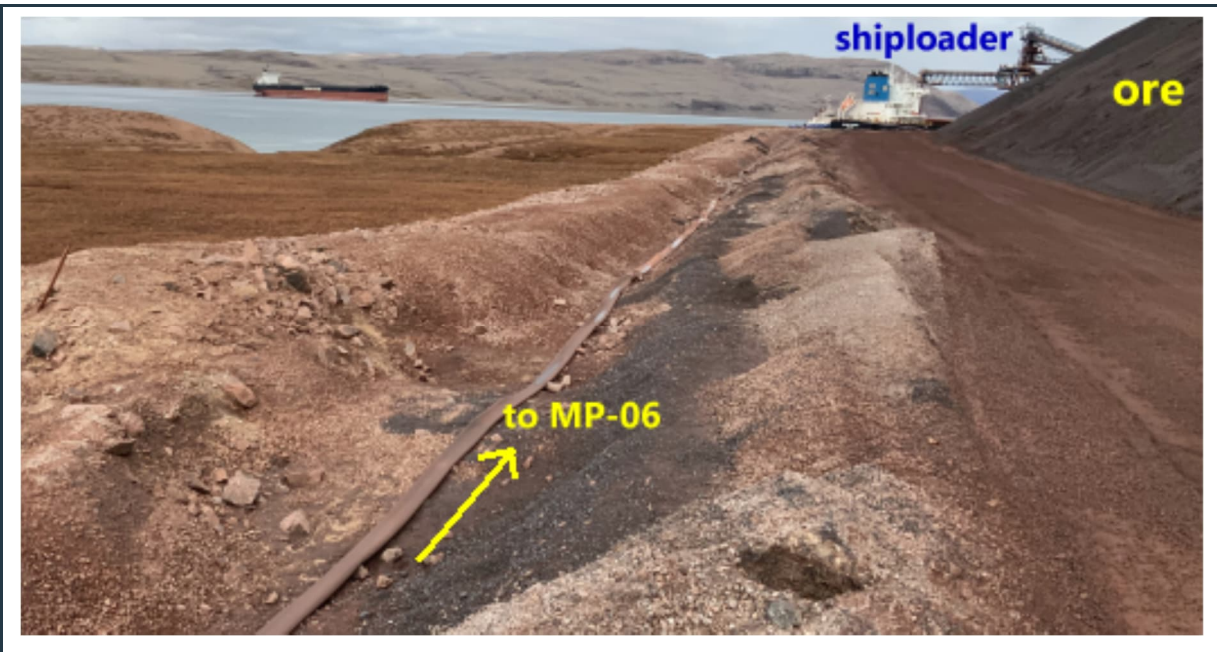
Figure 68: View of the “west” surface water collection ditch adjacent to the ore storage, draining from pond #3 to the MP-06 pond.
