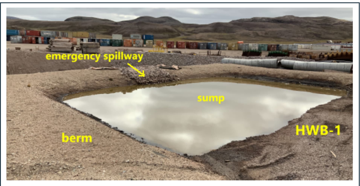
Figure 53: View of the sump and emergency spillway at the back of the HWB-1 cell with stable berms.
