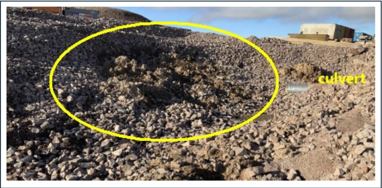
Figure 82: View of the “west end” of the PSC surface water collection ditch (red circle in Figure 7). Note the localized slope degradation due to frequent water seepage from the granular fill of the LP-2 laydown pad (yellow circle here). The culvert shown in the image can be removed.
