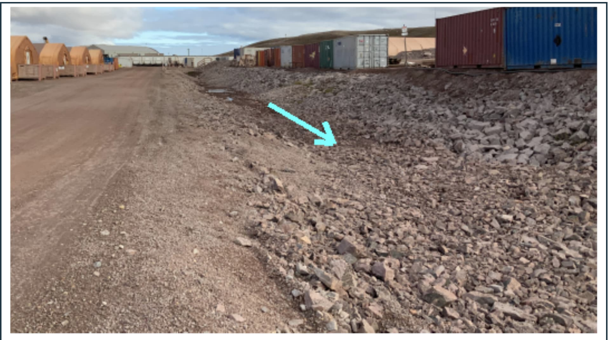
Figure 81: View of the east section of the 380-Person Camp surface water collection ditch. The clogged culvert in the ditch has been cleaned.
