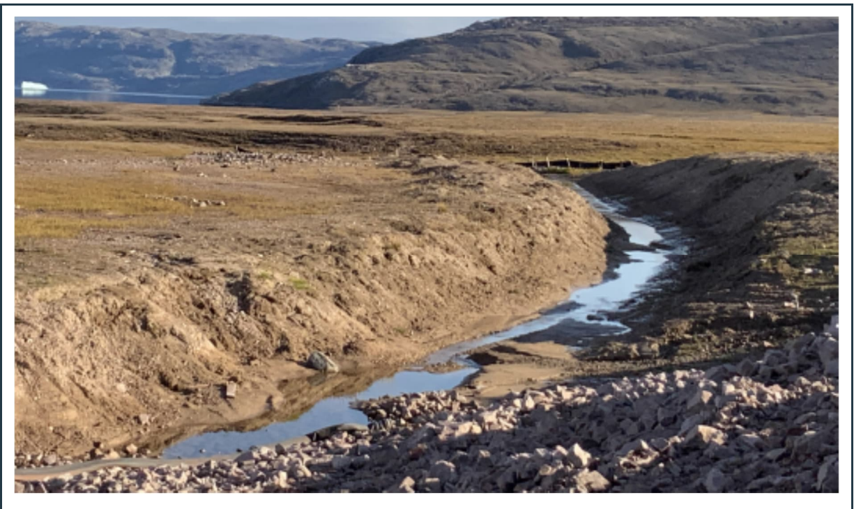
Figure 83: View of the unfinished “east end” of the PSC surface water collection ditch (also shown by the green circle in Figure 7). Riprap and a check dam should be installed at this section if the ditch.
