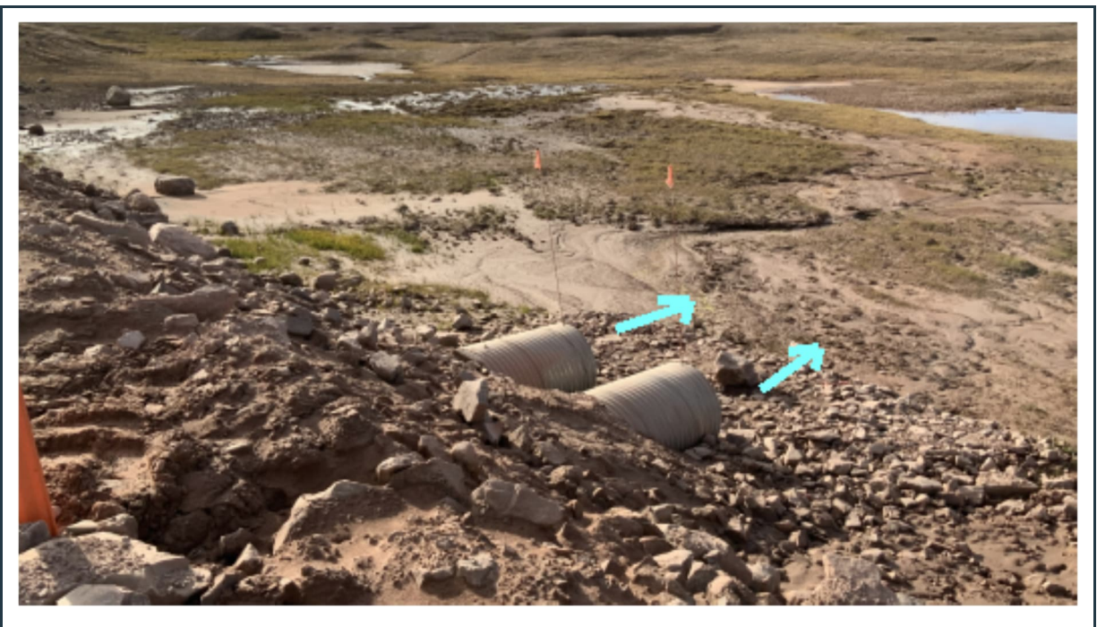
Figure 85: View of twin culverts, draining surface water from the P-SWD-6 ditch under the road (outlet).
