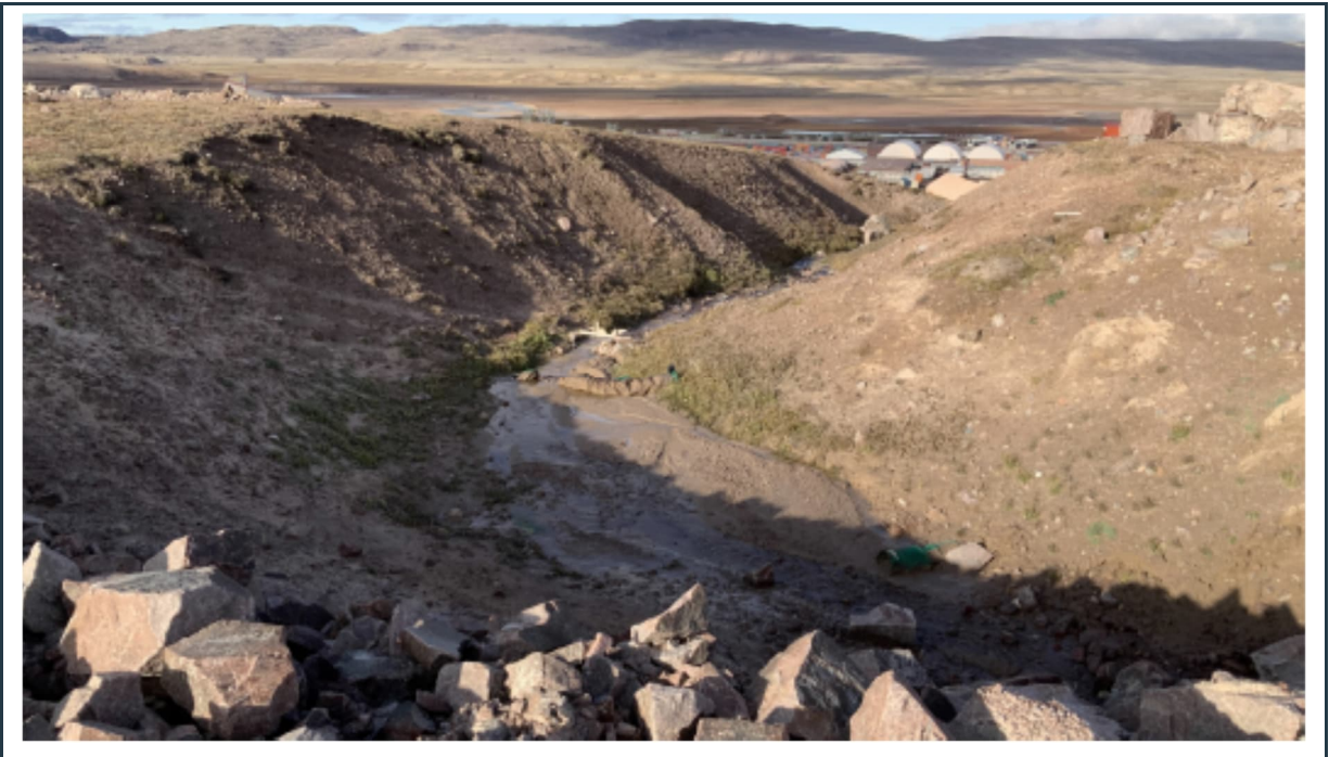
Figure 76: View of a side-valley near the south-west corner of the quarry (see also the red rectangle in Figure 10 of the report). This valley should be “upgraded” to drain the collected surface water from the quarry to the side ditch of the tote road and then to the W3/W14 ditch.
