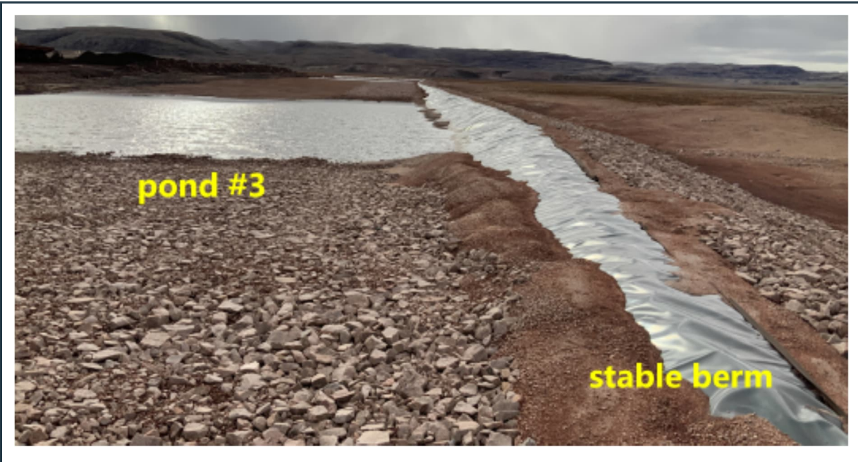
Figure 62: View of surface water management pond #3, with lined, stable berms.
