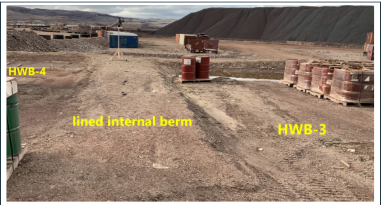
Figure 55: View of the well-maintained HWB-3 cell (right) with stable berms, containing fuel barrels. The interior subgrade of the cells has been regraded recently using clean sand and gravel fill.
