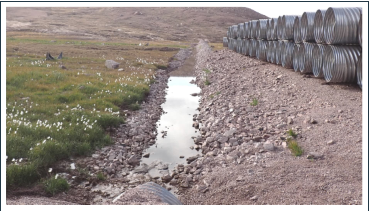
Figure 71: View of the southern section of the P-SWD-3 surface water collection ditch with failed slope sections, and ponding water due to inadequate longitudinal channel slope.
