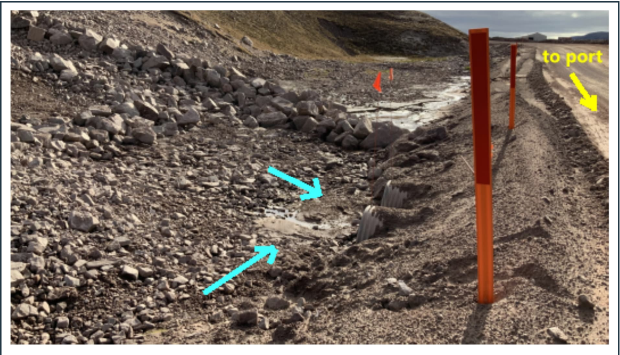
Figure 84: View the inlet of twin culverts draining surface water from the P-SWD-6 ditch under the road.
