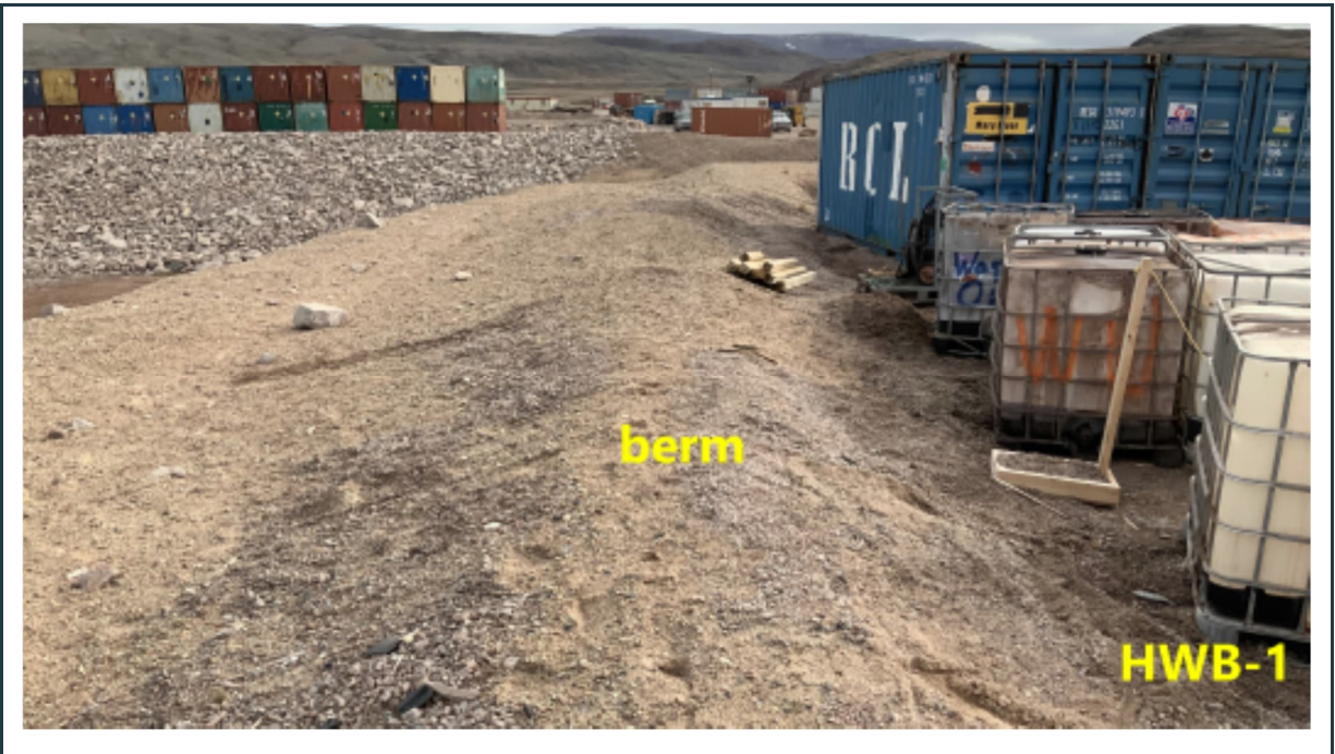
Figure 52: View of the stable berm around the lined HWB-1 cell.
