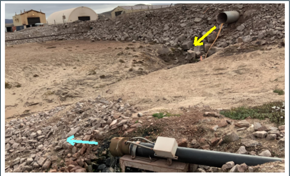
Figure 86: View of the end of the water discharge pipe (blue arrow) and a nearby culvert (yellow arrow) draining water to the same valley (see the next image below).
