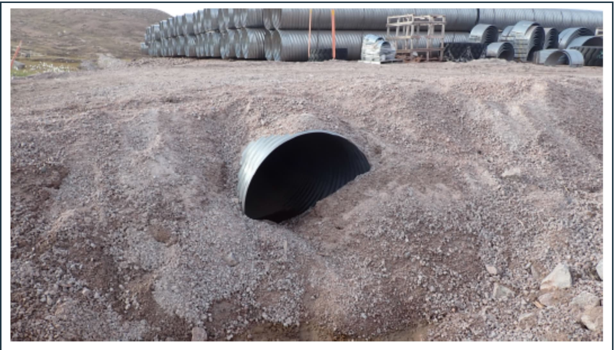
Figure 73: View of the culvert in the P-SWD-3 ditch with its invert above the invert level of the ditch. The culvert should be removed and then reinstalled during the rehabilitation of the ditch.
