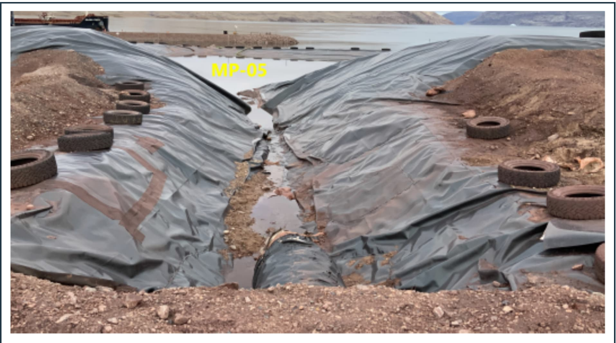
Figure 64: View of the inlet channel to the MP-05 pond. The previously damaged liner has been repaired.
