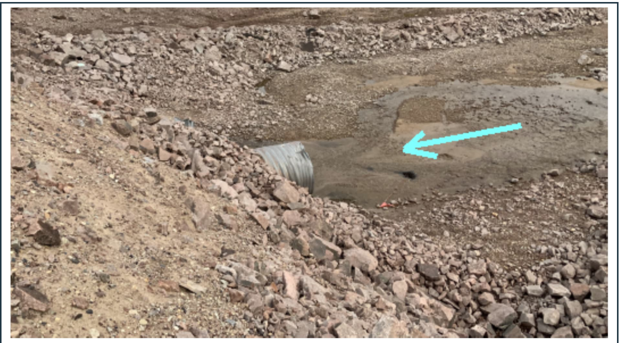
Figure 77: View of the P-SWD-7 surface water collection ditch and culverts (inlet).
