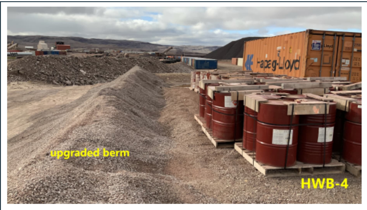
Figure 56: Recently improved (raised) berm at the HWB-4 cell, storing jet fuel and shipping containers. Note the improved granular base within the cell, protecting the liner.
