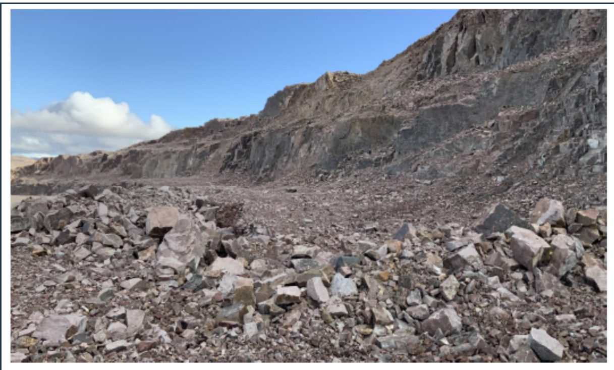
Figure 69: View of the stable rock face with some weathering and bench erosion in the Q01 rock quarry. Currently there is no activity in this quarry.
