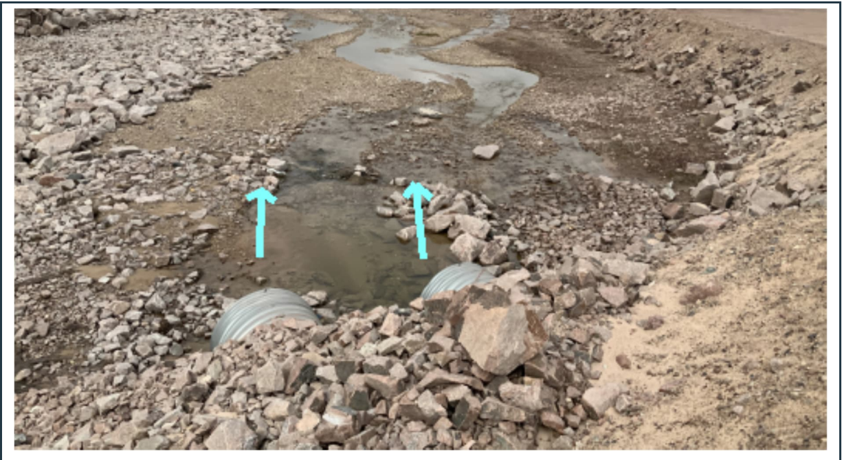
Figure 78: View of the well-maintained P-SWD-7 surface water collection ditch and culverts (outlet).
