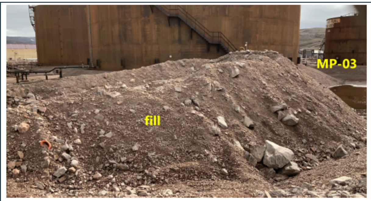
Figure 59: View of a pile of fill in the western part of the MP-03 fuel farm. Based on site information, this material was part of the granular base within the cell and potentially contaminated. Hence, it should be left in place at its current location within the lined facility.
