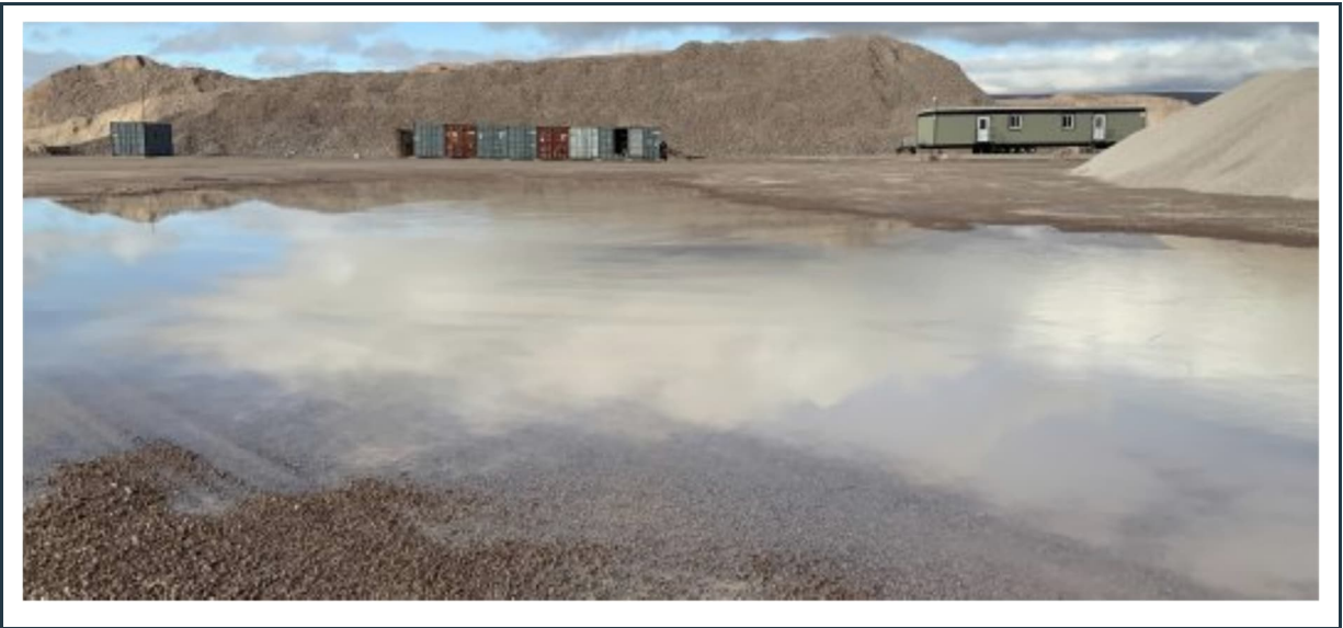
Figure 70: View of ponding water across the lower level of the Q01 rock quarry. The drainage problem should be rectified prior to restarting the operation in the quarry.
