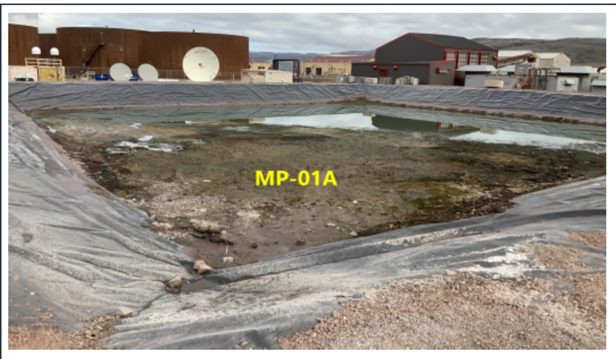
Figure 57: View of the robust, stable berms and intact liner at the practically empty MP-01A pond.
