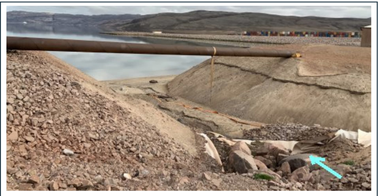
Figure 87: View of the "valley" at the front of the water discharge area (blue arrow) and deteriorating (eroding) slopes. This section of the valley should be filled with rock fill, placed over geotextile.
