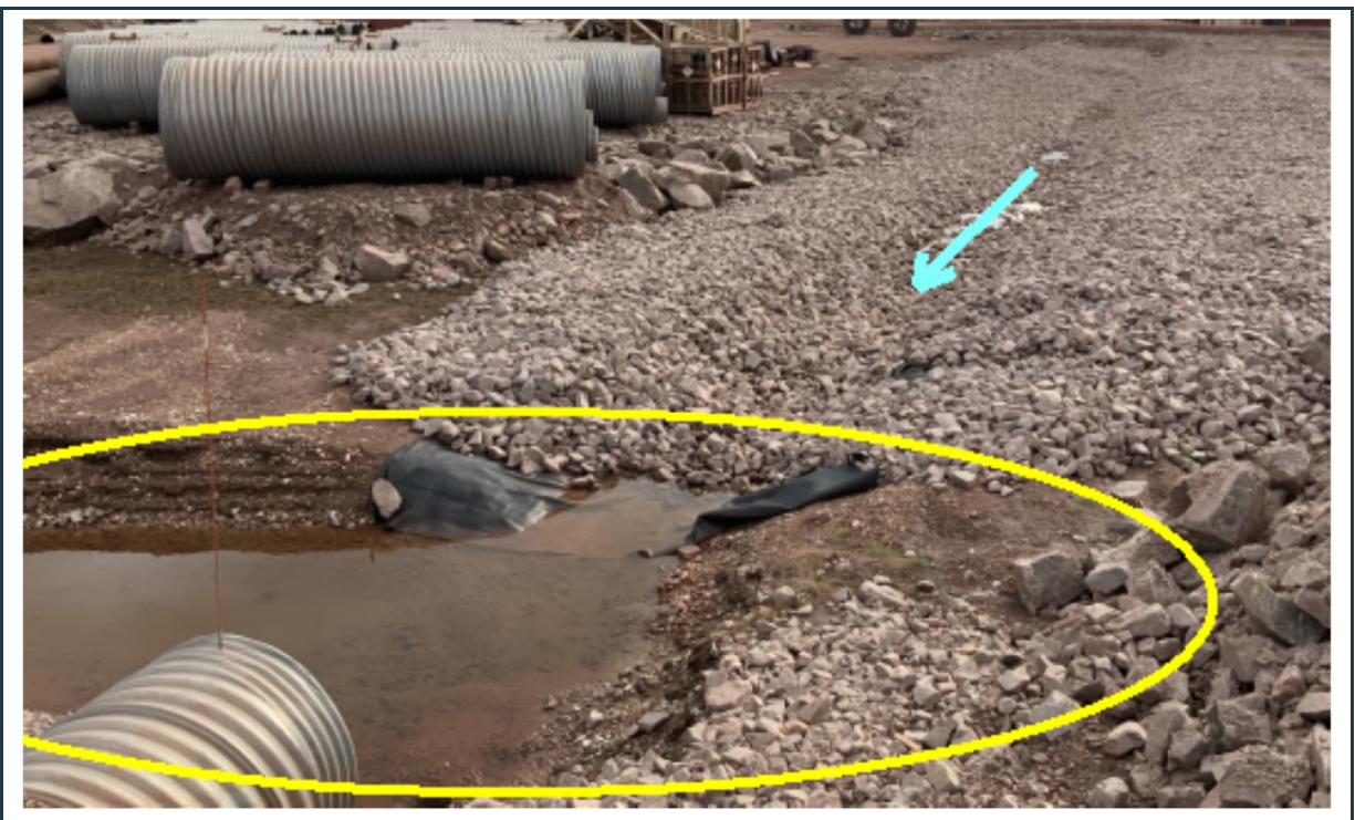
Figure 79: View of the W3/W14 surface water collection ditch with crushed rock riprap slope protection. The area around the culvert's inlet still requires the placement of geotextile and riprap.
