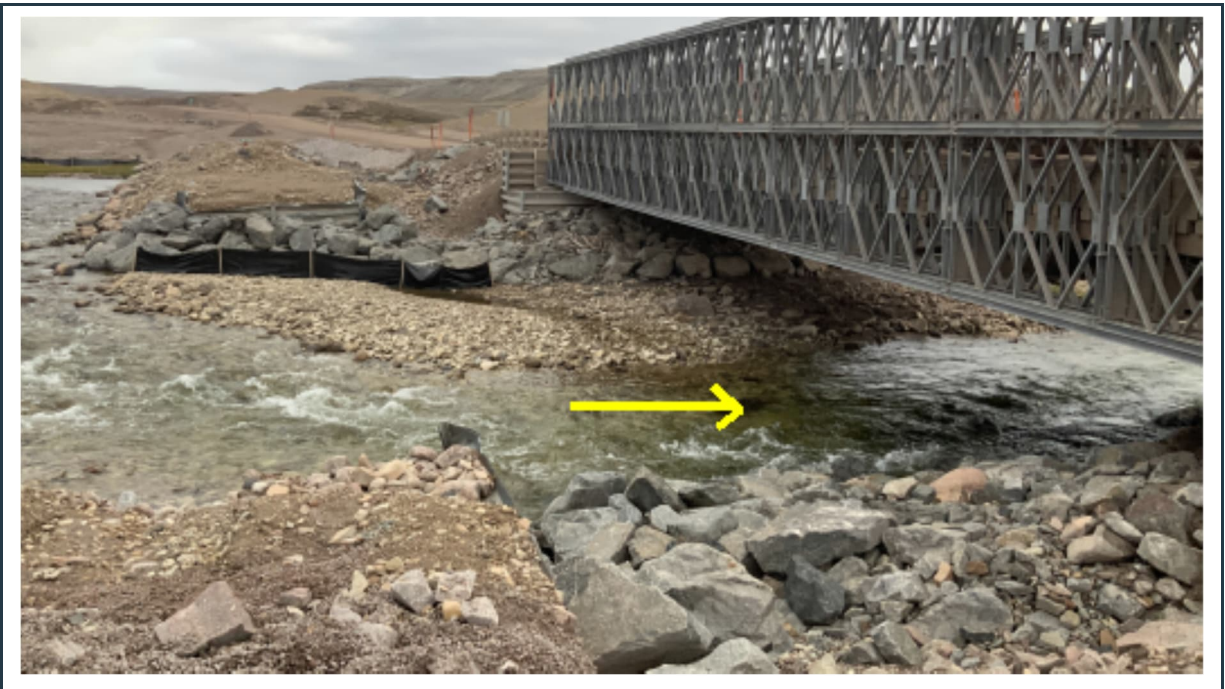
Figure 97: View of the stable abutments at the east side of bridge 63. Also note one (south) of the two “old” crib abutments with riprap protection and a silt-curtain.
