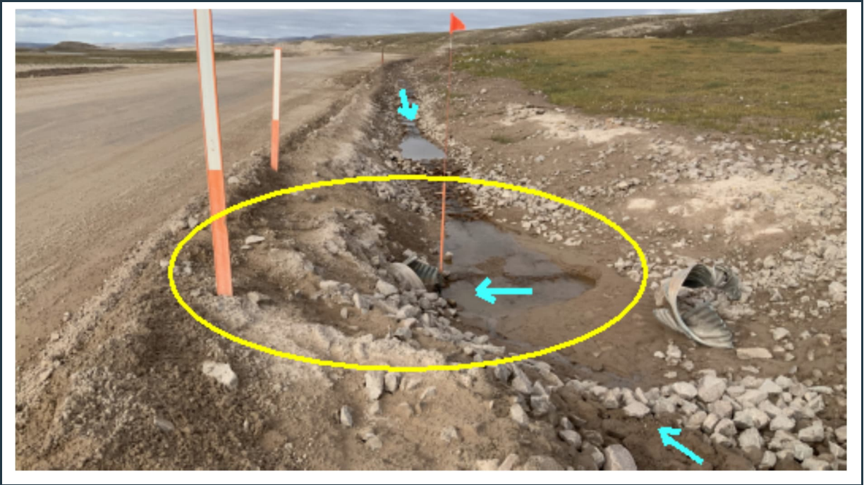
Figure 102: View of the damaged culvert at its inlet at KM 33+000. The culvert should be replaced as soon as practically possible. More rockfill should also be placed around the culvert's inlet.
