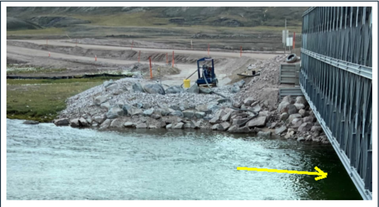
Figure 94: View of the west abutment, where the old metal crib has been removed and replaced with new riprap erosion protection at the south side of bridge KM17 (yellow circle in Figure 93).
