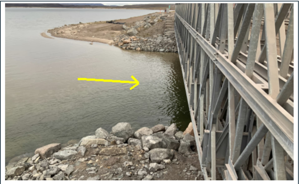
Figure 99: View of the abutments with riprap scour protection at the east side of bridge 80.
