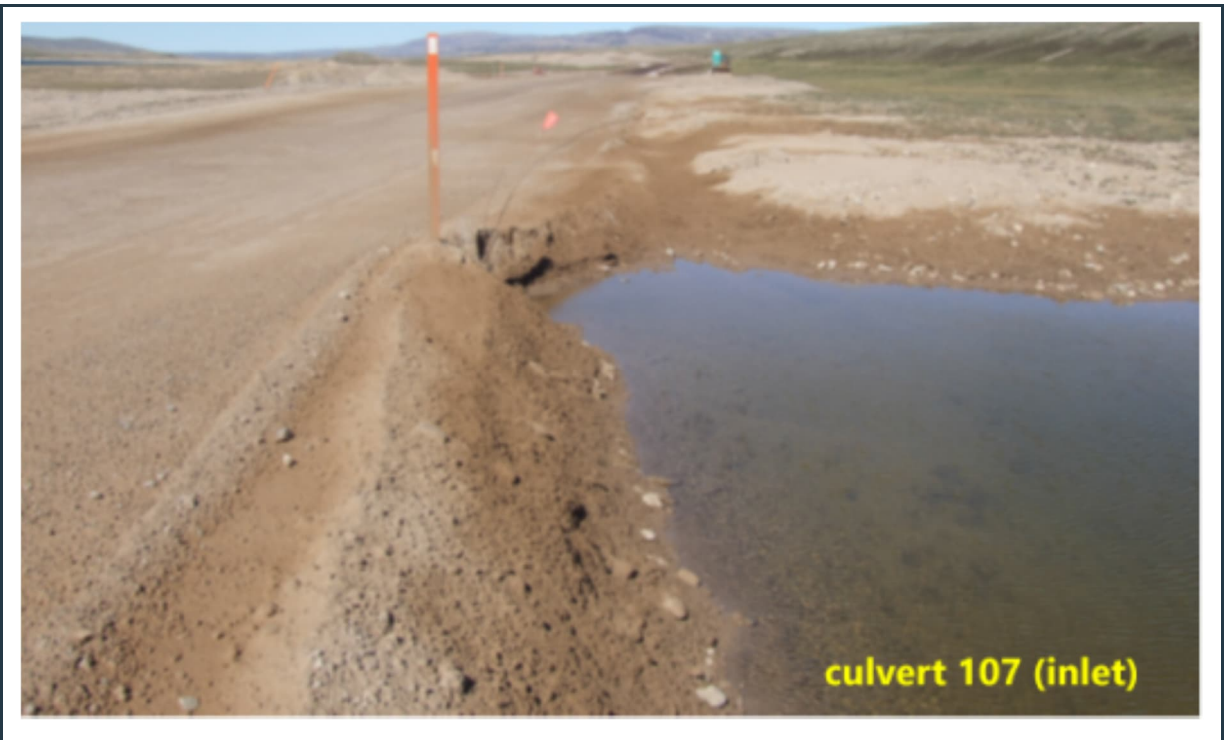
Figure 113: View of typical problems at one section of the Tote Road. (a) Ponding water adjacent to shallow road embankment and (b) unacceptably short culvert in a historic image from 2019.
