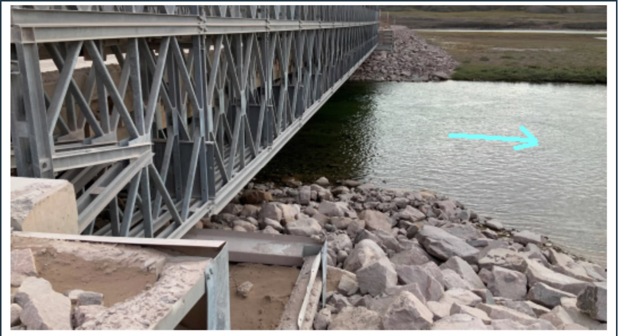
Figure 92: View of the stable abutments with riprap erosion protection at the north side of bridge KM17.
