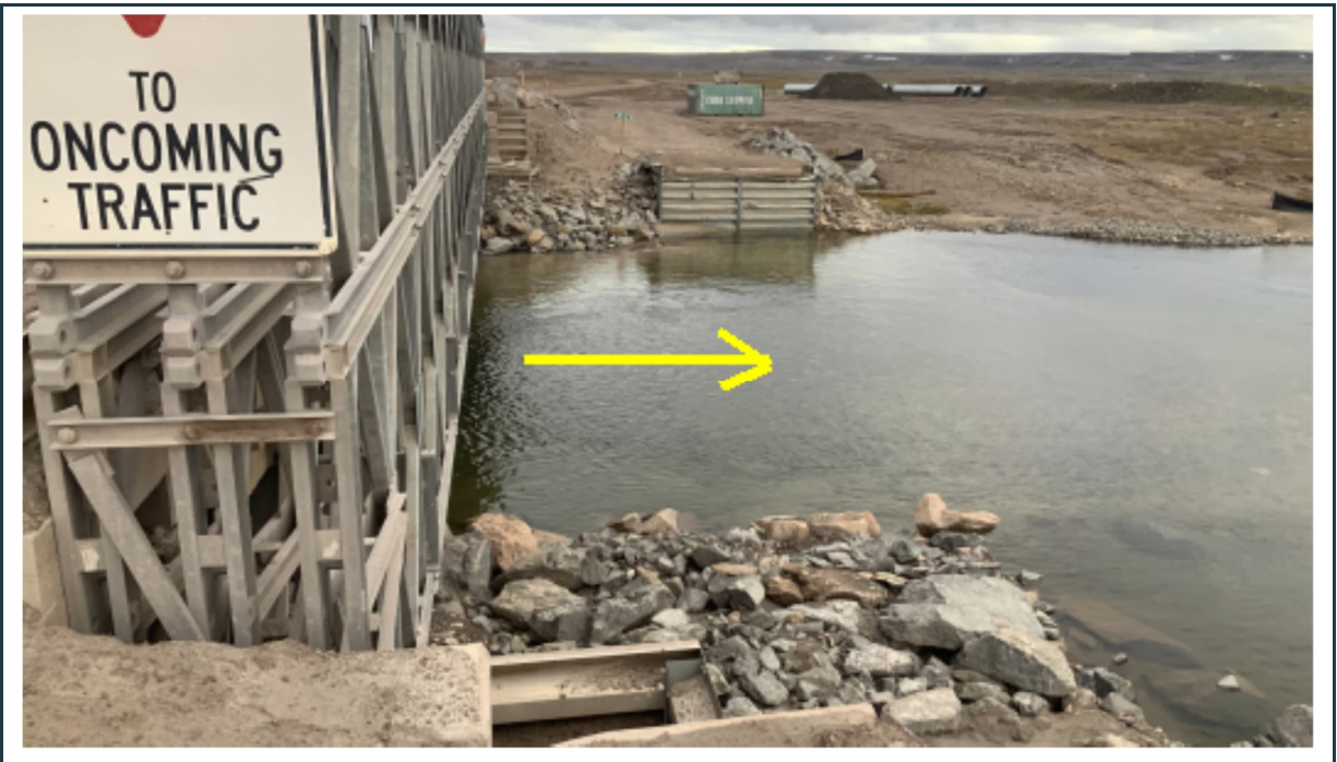
Figure 98: View of the west side of bridge 80, with riprap scour protection around the abutments.
