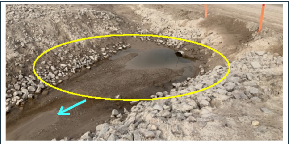
Figure 103: View of the outlet of the culvert at KM 33+000. The ditch at the front of the culvert should be cleaned during culvert replacement and more ripraps should be placed.
