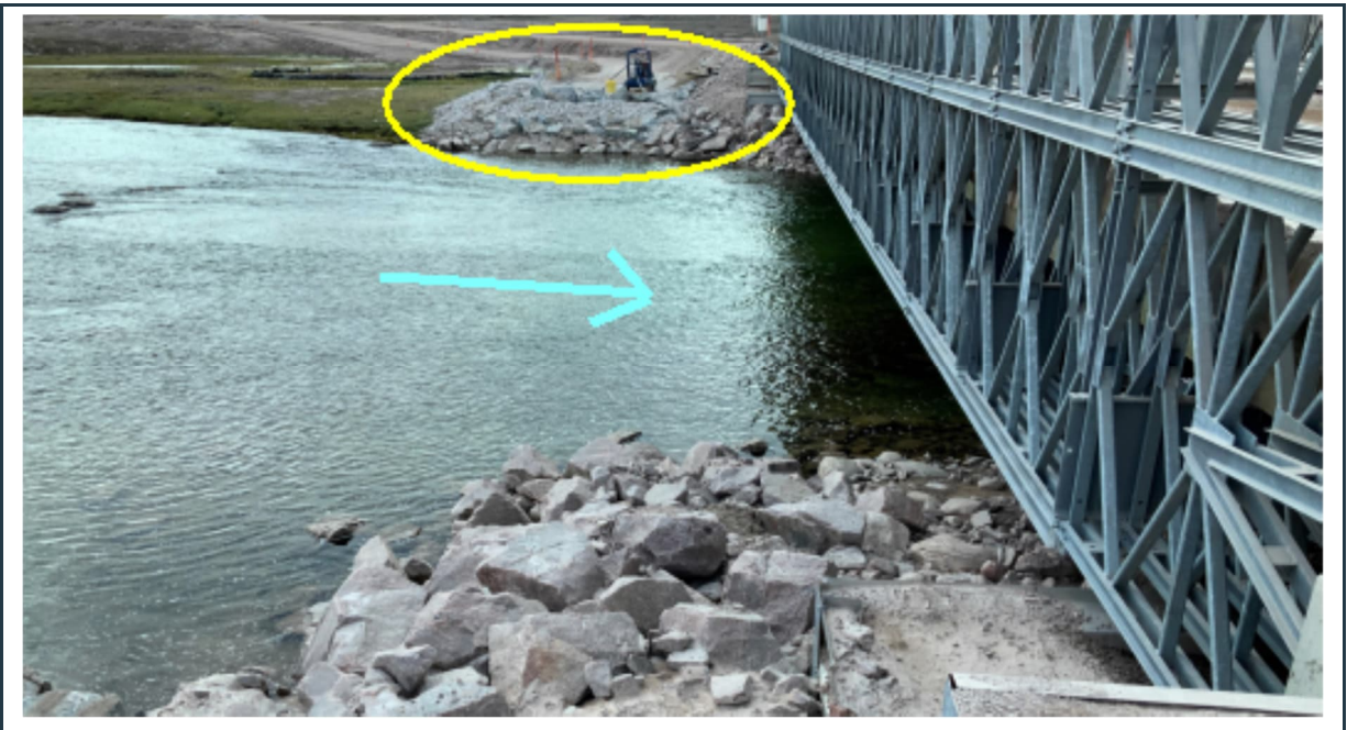
Figure 93: View of the stable abutments with riprap scour protection at the south side of bridge KM-17.
