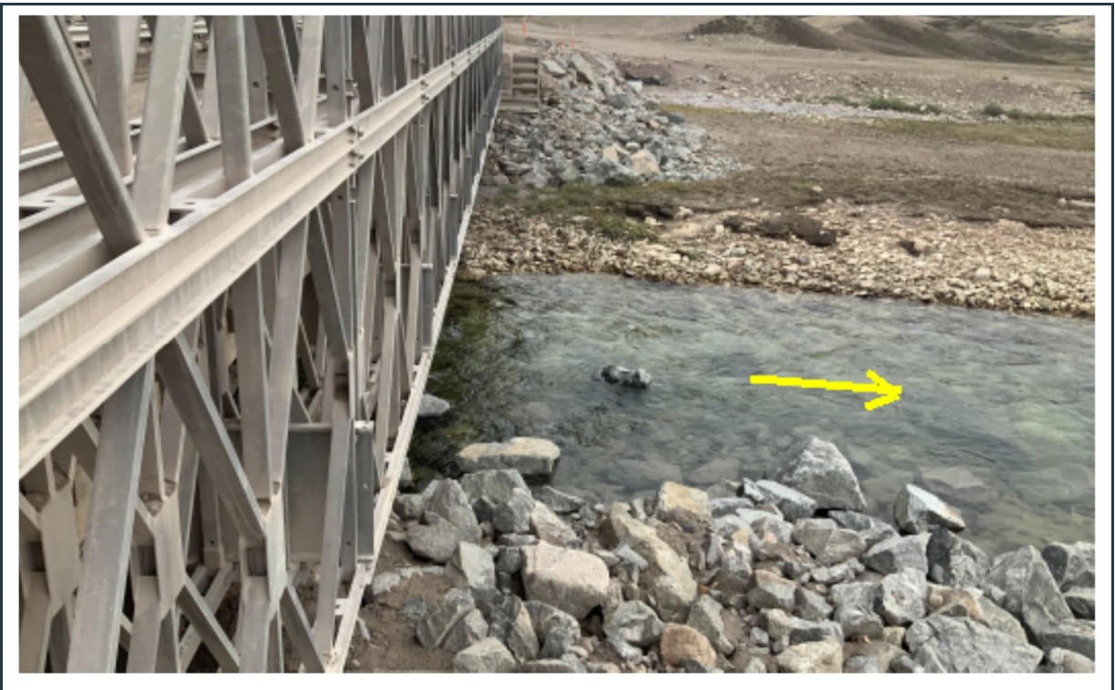
Figure 96: View of the west side of bridge 63, with stable abutments and riprap scour protection.
