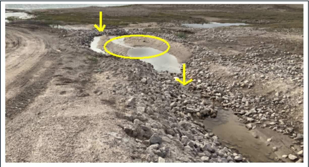
Figure 104: View of the ditch and check dams at KM 33+000. The ditch should be cleaned (yellow circle) and the crest of the check dams repaired/raised (yellow arrows) during culvert replacement.
