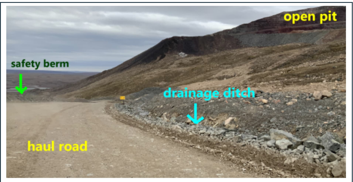
Figure 105: View of the well-maintained haul road between the crusher pad and the open pit around KM-107. Note the safety berm along the downslope side and the upgraded, erosion-controlled drainage ditch along the upslope side of the road with additional rock fill in critical areas.
