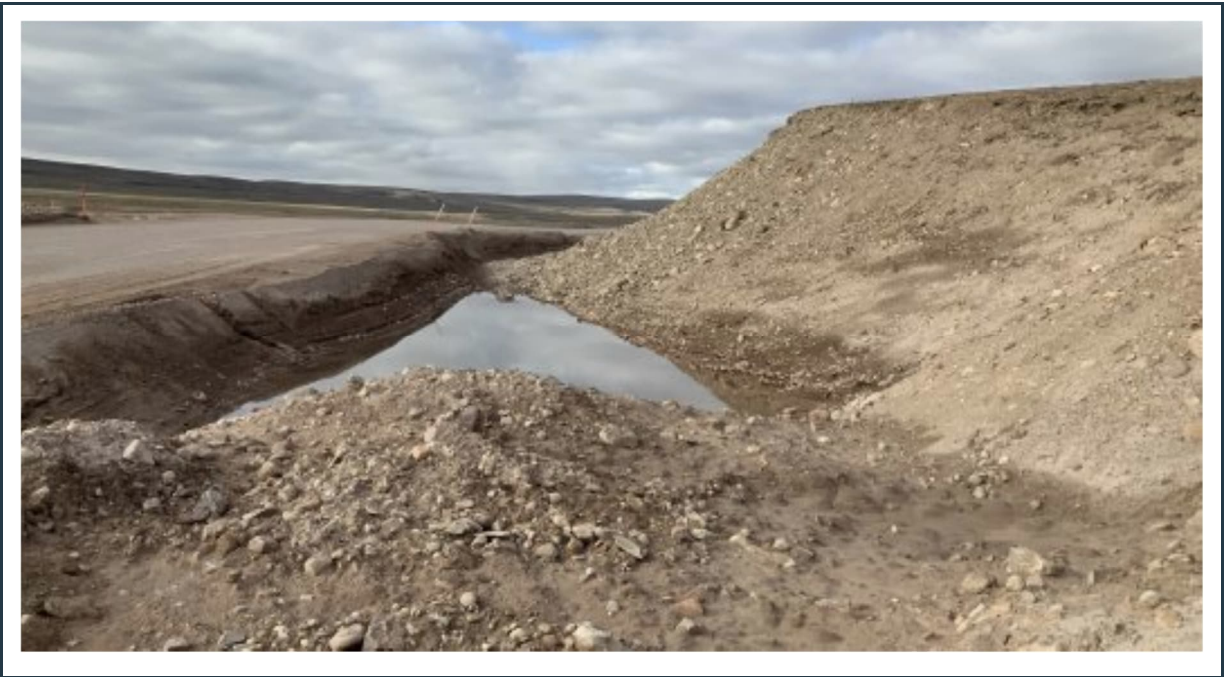
Figure 112: View of a generally stable slope in a cut area, and the adjacent road embankment with poor surface drainage at KM 28.9. - September 3, 2023.
