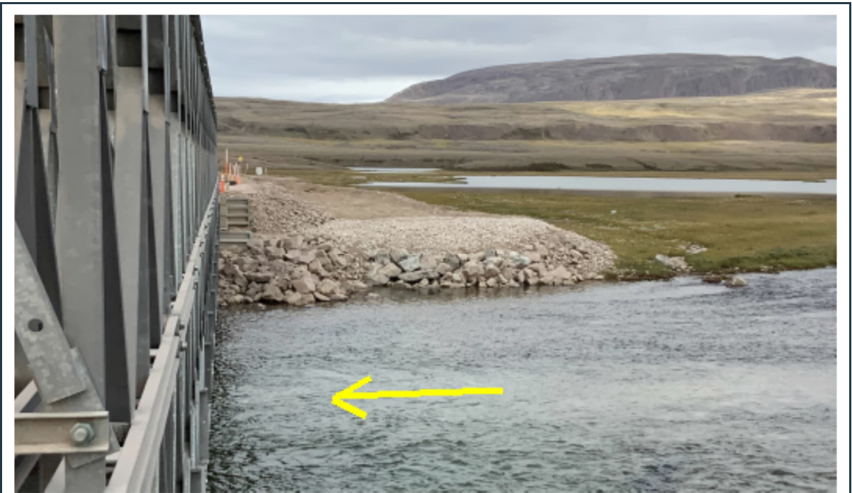
Figure 95: View of the east abutment, where the old metal crib has been removed and replaced with new riprap erosion protection at the south side of bridge KM17.
