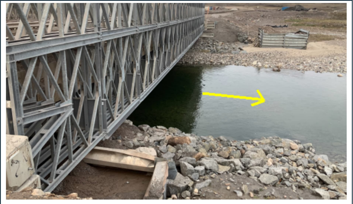
Figure 100: View of the stable abutments with riprap scour protection at the west side of bridge KM 97.
