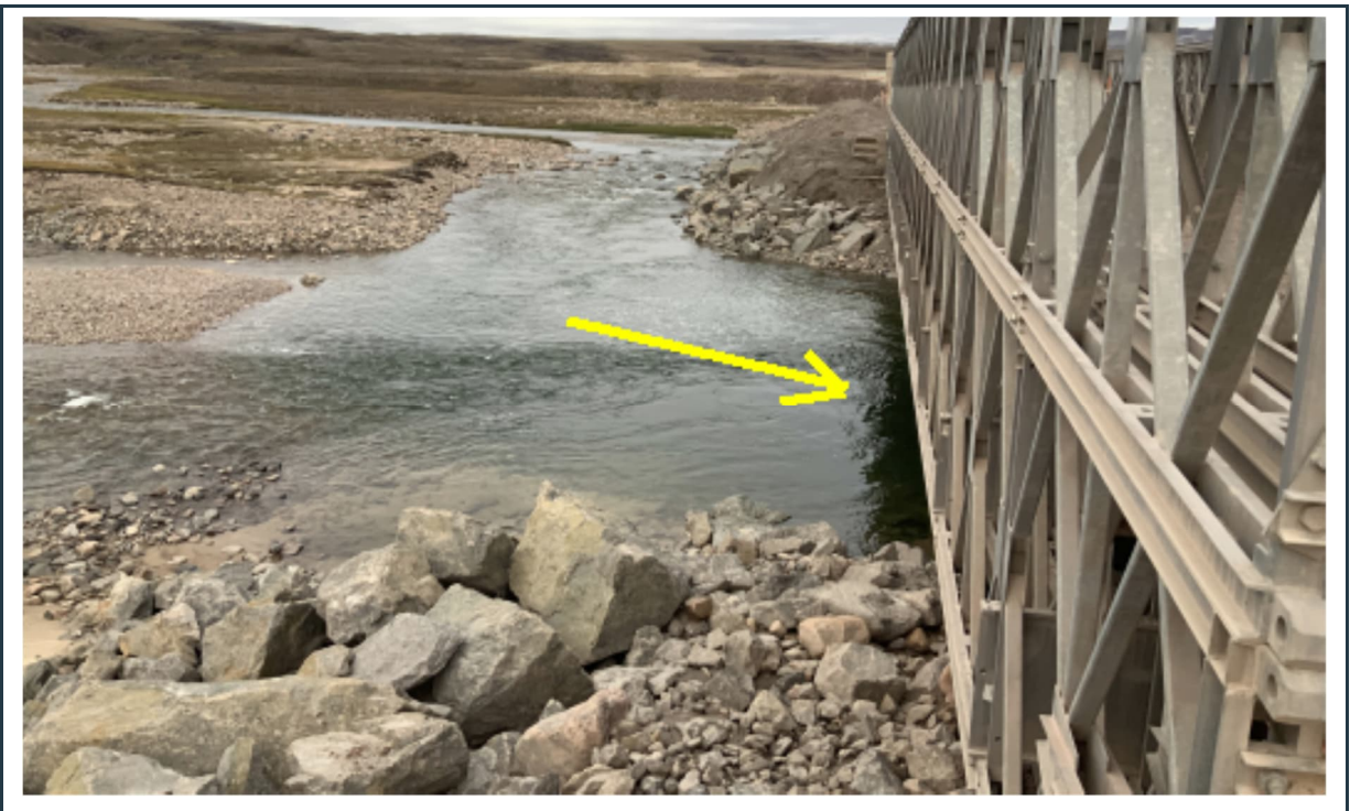
Figure 101: View of the two stable abutments with riprap scour protection at the east side of bridge KM97.
