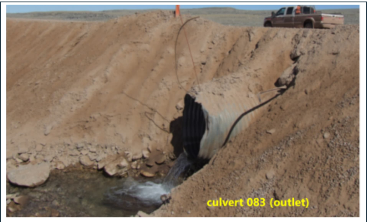
Figure 115: View of the most typical problems (short culvert and erosion at the toe of the embankment) along the Tote Road in a historic image from 2019.
