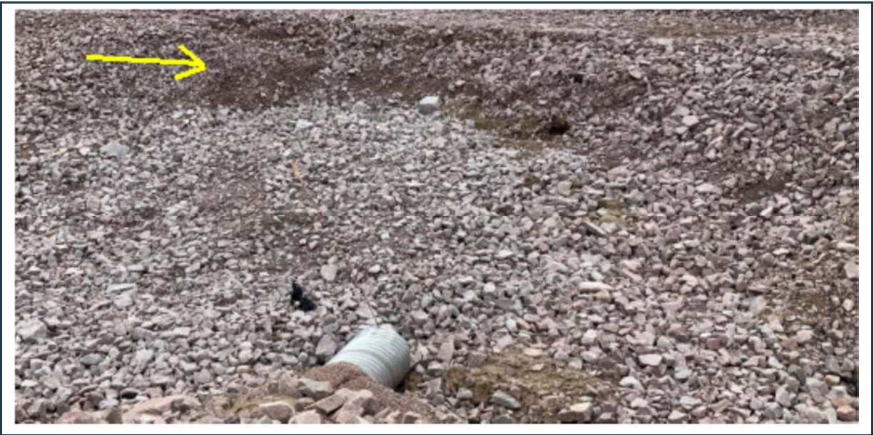
Figure 81: View of the “west end” of the PSC surface water collection ditch (red circle in Figure 8). Note the localized slope degradation due to frequent water seepage from the granular fill of the LP-2 laydown pad (yellow arrow). The culvert shown in the image can be removed.
