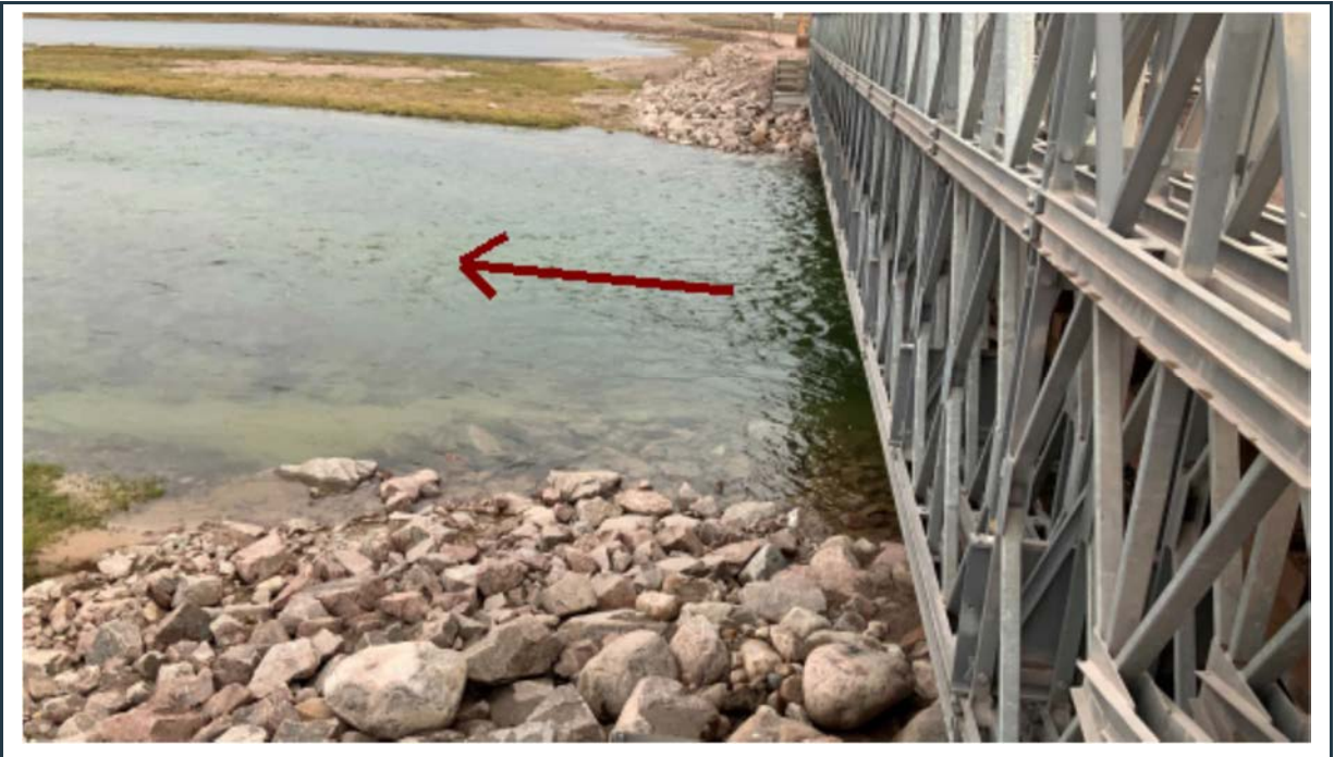
Figure 89: View of the stable abutments with riprap erosion protection at the north side of bridge KM17.
