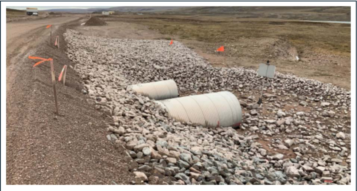
Figure 105: View of the outlet of the twin culverts at KM 33+100. No water was flowing through the culverts that show some sagging in their centre, under the weight of the road embankment.
