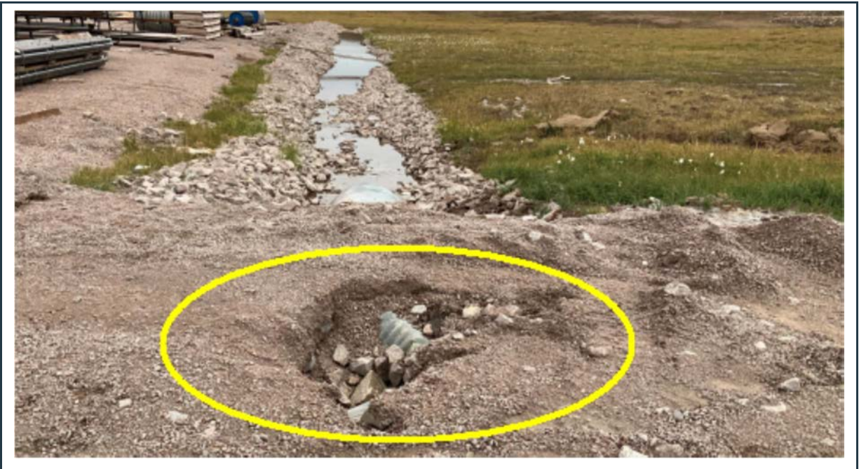
Figure 71: View of the damaged culvert (yellow circle) and the northern section of the P-SWD-3 surface water collection ditch with failed slopes and ponding water.
