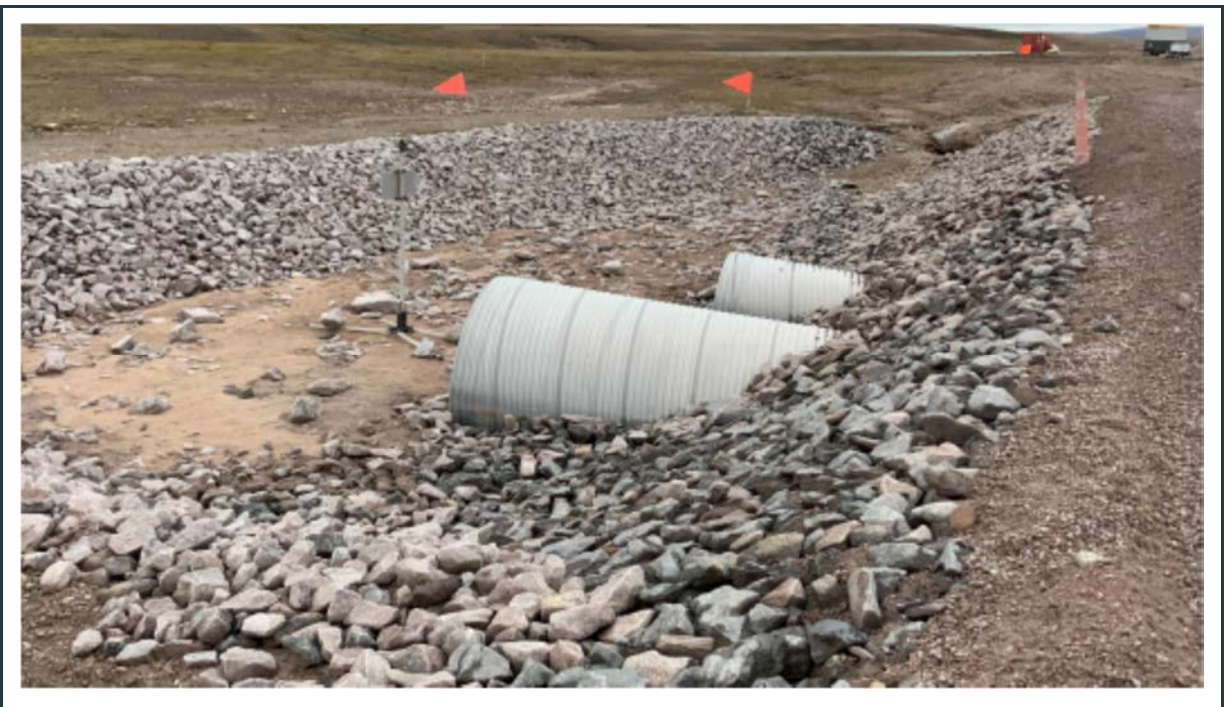
Figure 104: View of the inlet of the twin culverts at KM 33+100. No water was flowing through the culverts that show some sagging in their centre, under the weight of the road embankment.
