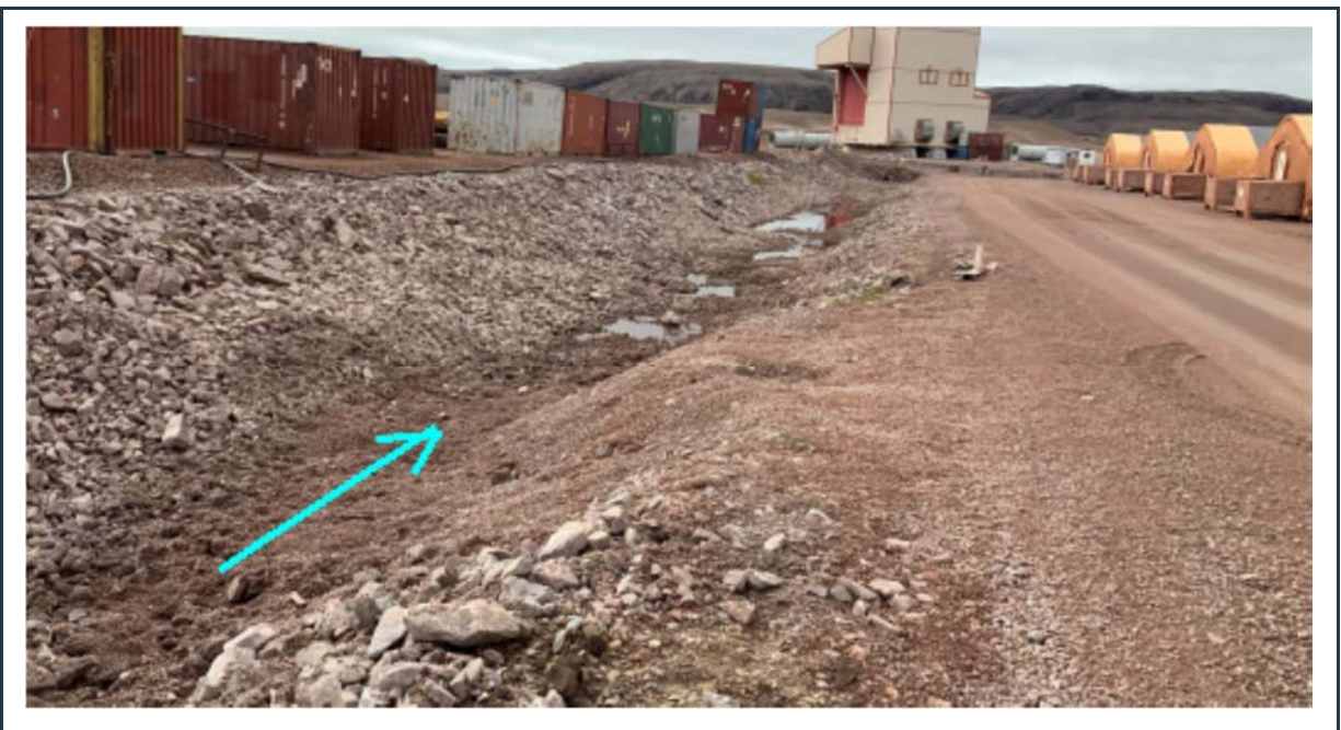
Figure 80: View of the east section of the 380-Person Camp surface water collection ditch in good condition.
