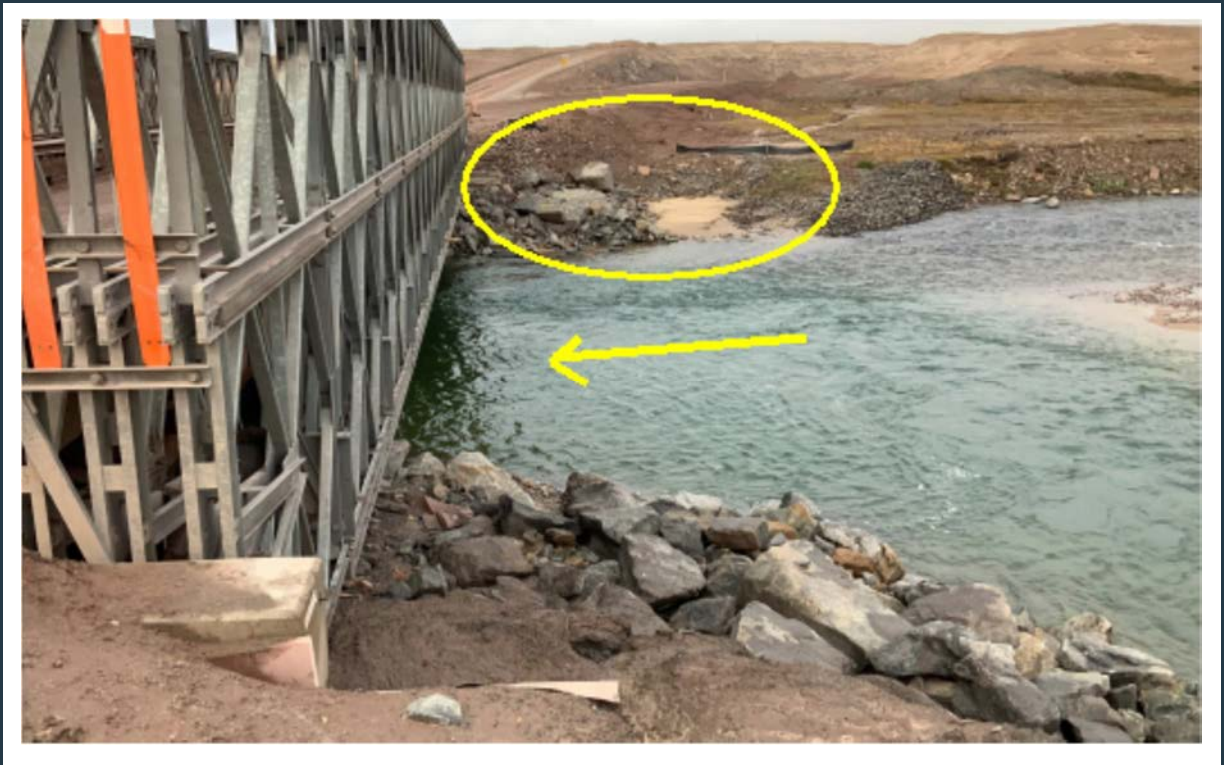
Figure 99: View of the stable abutments at the east side of bridge KM97. Note the area marked by the yellow circle where additional rock fill should be placed at the shore of the river and adjacent to the approach embankment to the bridge abutment, for erosion protection.
