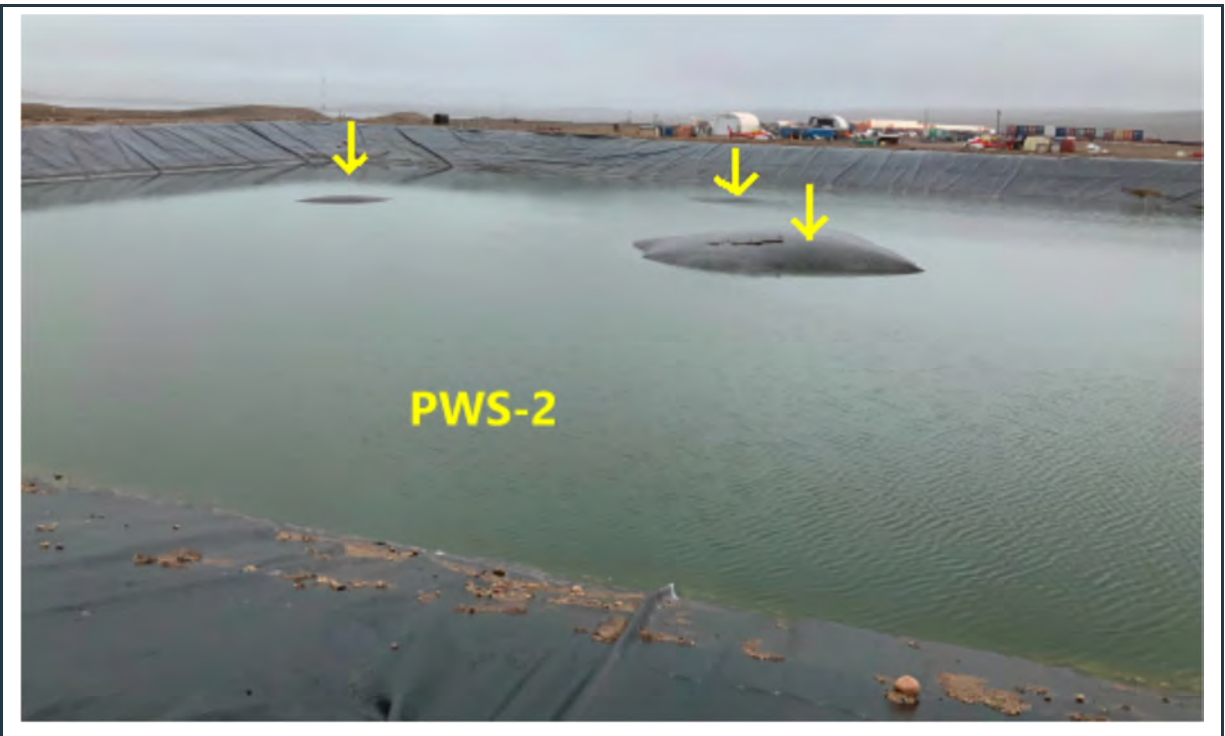
Figure 15: PWS pond #2 with stable, well-maintained berms and liner. – Sections of the liner (“whales”) are visible in the pond above the water (yellow arrows), which do not pose a risk to the integrity of the liner.
