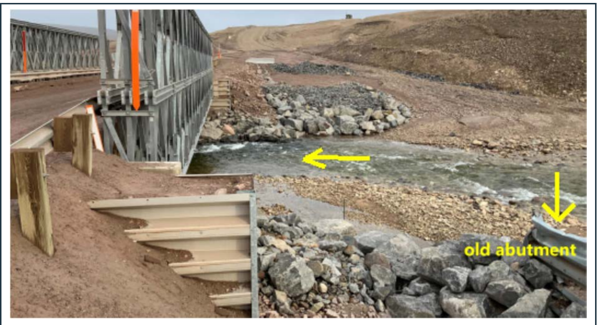
Figure 94: View of the stable abutments at the east side of bridge 63. Also note that one (south) of the two “old” crib abutments is still in place, while the north one has been removed and replaced with rock fill (cobbles and boulders).
