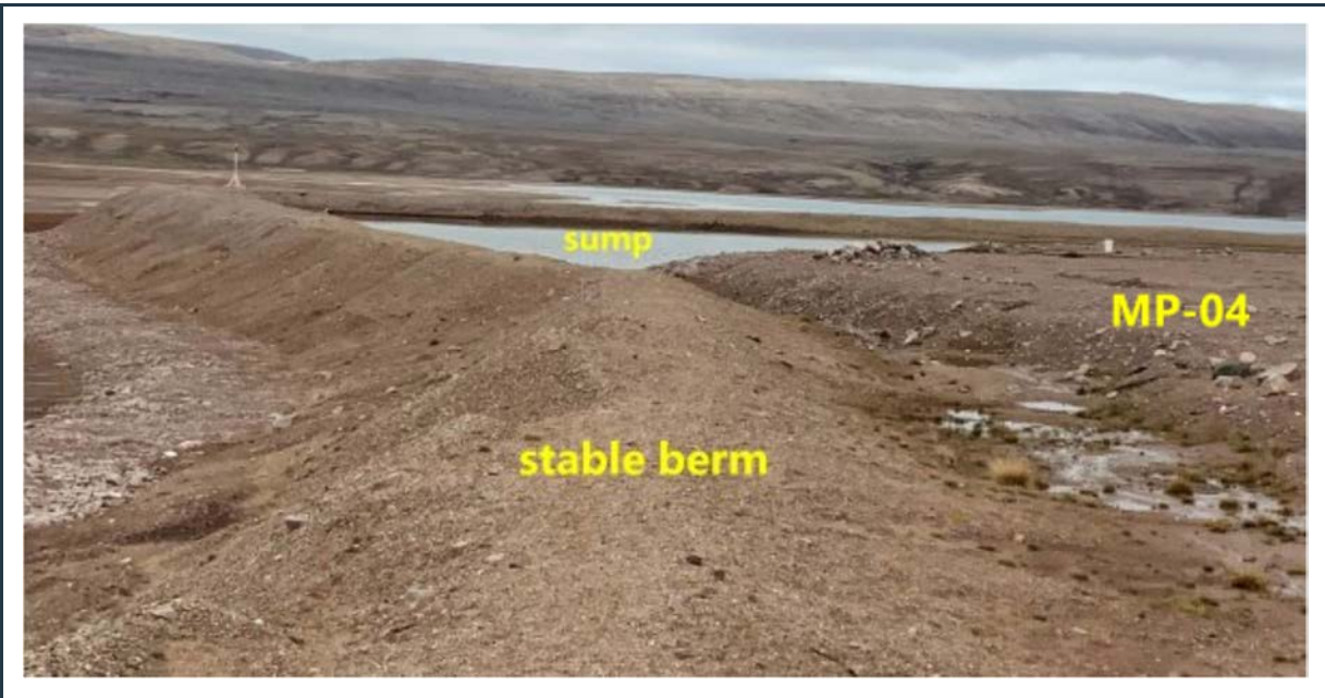
Figure 59: View of stable perimeter berm around the MP-04 landfarm, with ponding water in one corner of the cell (sump). Note the standard soil cover over the buried solid waste.
