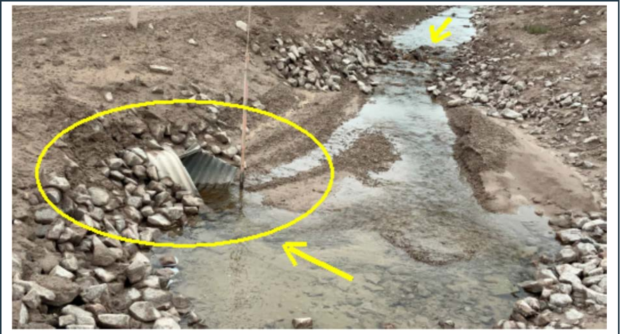
Figure 101: View of the damaged culvert at its inlet at KM 32+900. The culvert should be replaced as soon as practically possible. More rockfill should also be placed around the culvert's inlet.
