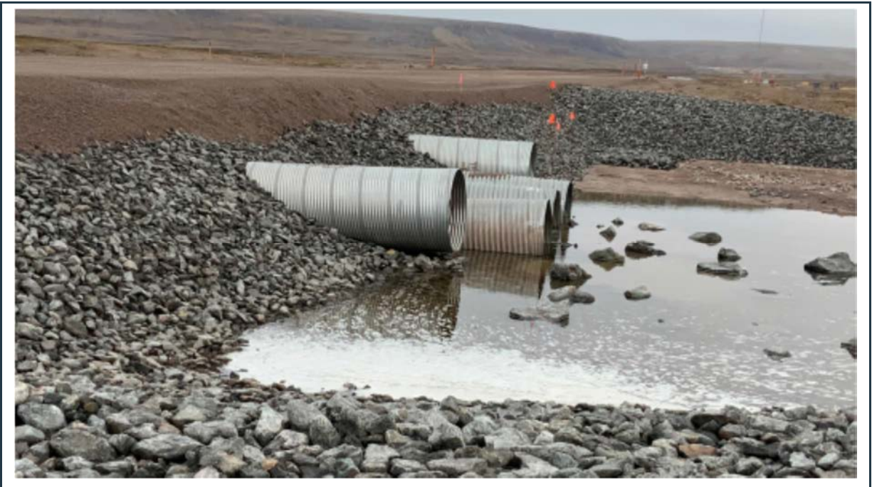
Figure 111: View of the outlet of five culverts at KM 80+500. All five culverts suffered serious differential settlements (sagging) and all of them will need to be replaced as soon as practically possible.
