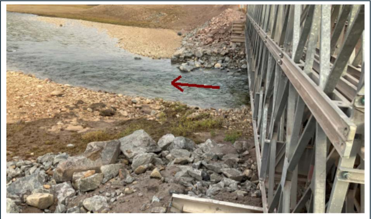
Figure 93: View of the west side of bridge 63, with stable abutments and riprap scour protection.
