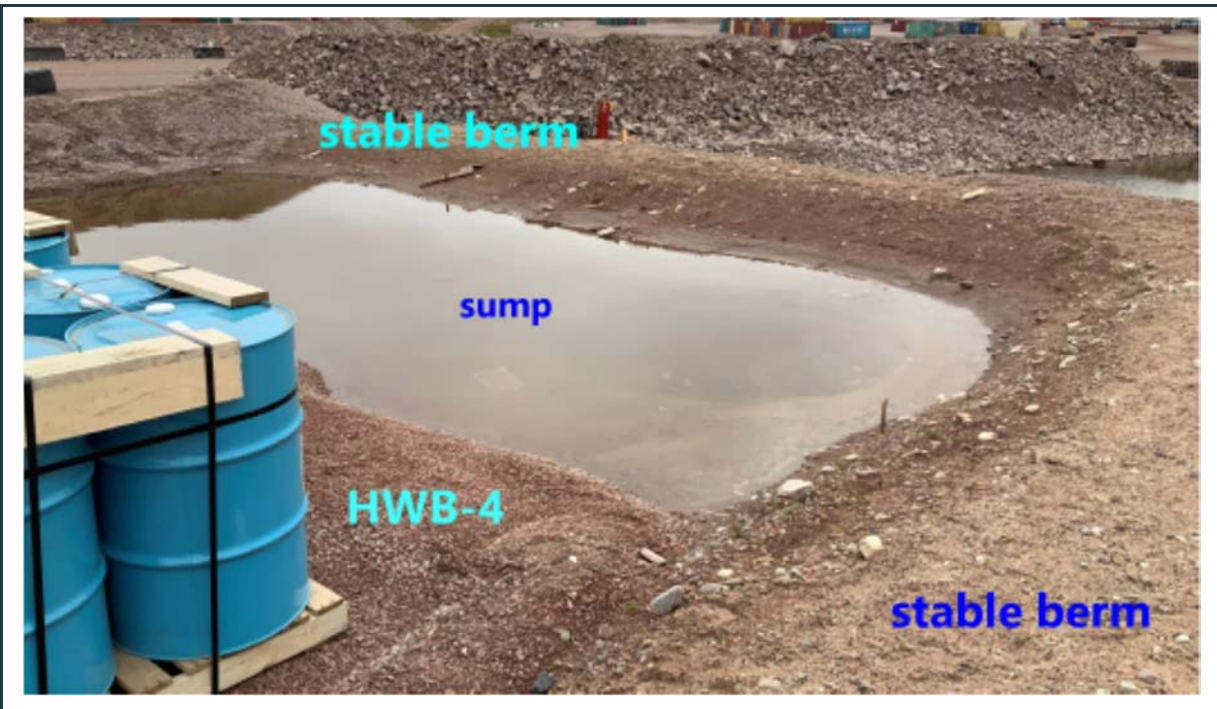
Figure 56: View of stable berm and the sump in the HWB-4 cell, storing jet fuel and shipping containers. Note the improved granular base within the cell, protecting the geomembrane liner.
