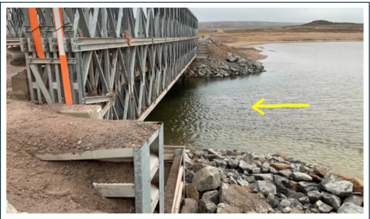
Figure 96: View of the abutments with riprap scour protection at the east side of bridge 80.
