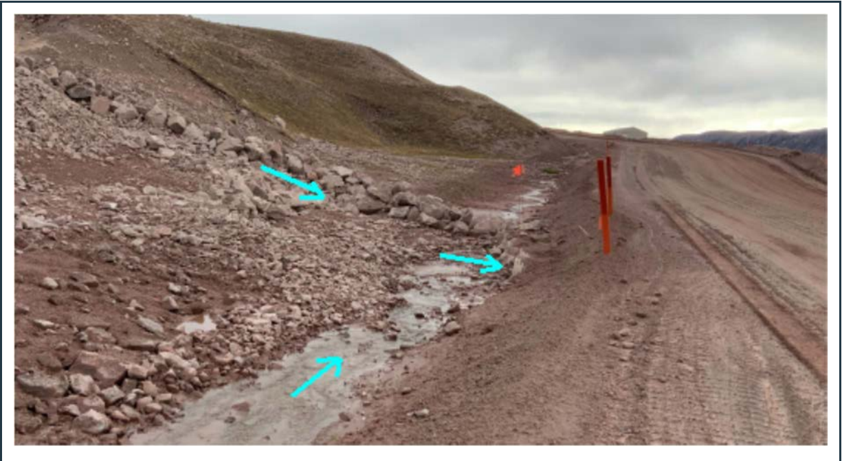
Figure 83: View the inlet of twin culverts draining surface water from the P-SWD-6 ditch and from the road's side-ditch, under the tote road.
