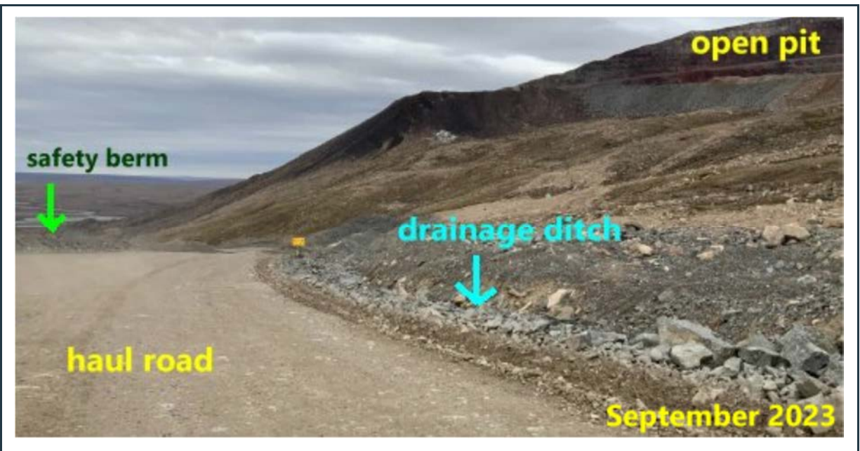
Figure 116: View of a 2023 image of the well-maintained haul road between the crusher pad and the open pit around KM-107. Note the safety berm along the downslope side and the upgraded, erosion-controlled drainage ditch along the upslope side of the road with additional rock fill in critical areas.
