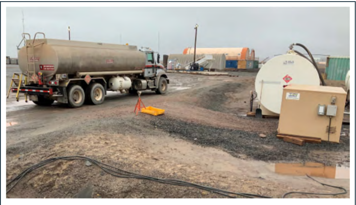
Figure 38: View of the well-maintained sand and gravel berm and access ramp at the lined jet-fuel storage facility. Ponding water in the cell indicates good liner performance.
