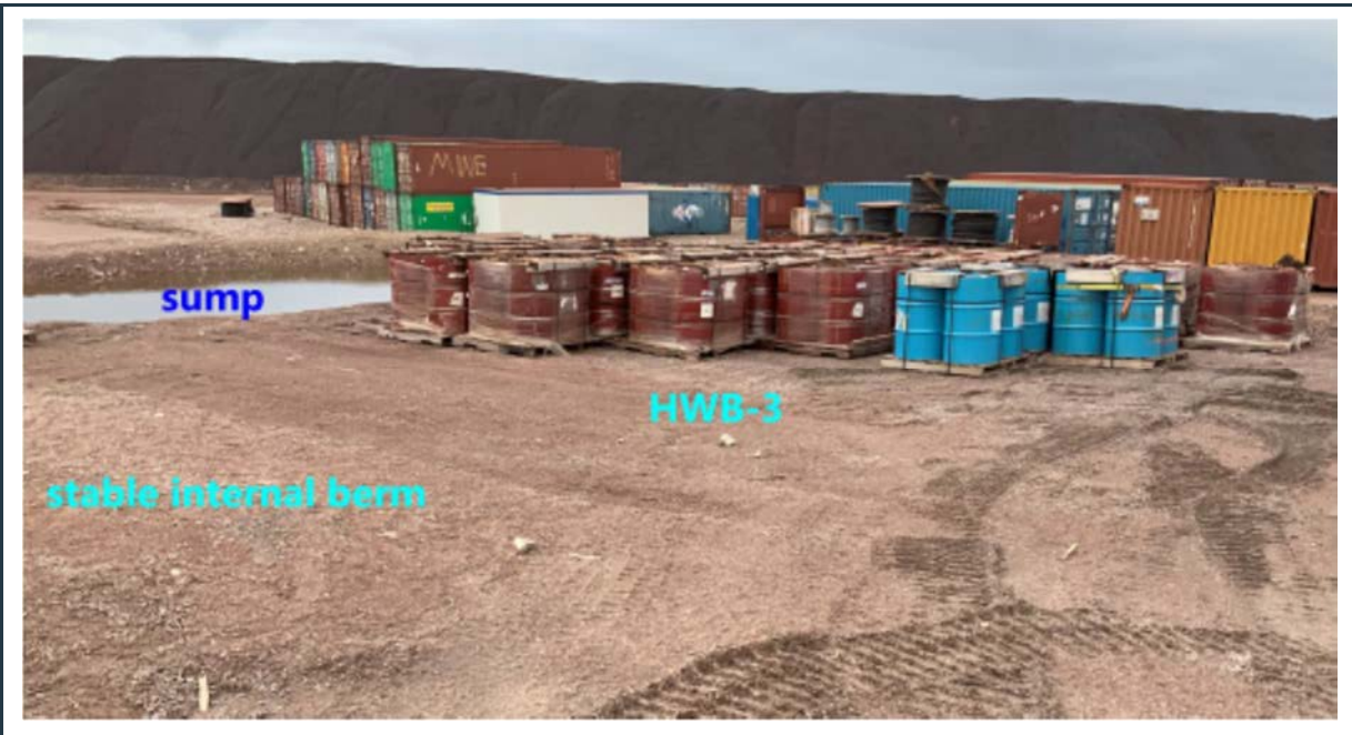
Figure 55: View of the well-maintained HWB-3 cell with stable berm, containing fuel barrels. The interior subgrade in the two cells had been regraded recently using clean sand and gravel fill.
