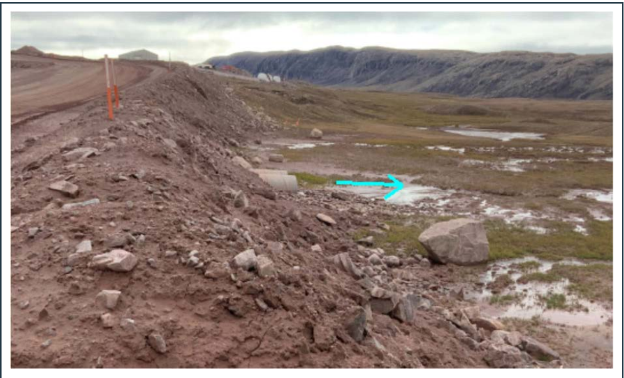
Figure 84: View of the outlet of the twin culverts, installed within the road embankment.
