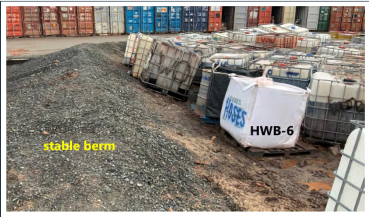
Figure 22: View of the recently regraded stable berm at the HWB-6 cell. The presence of ponding water in the cell indicates good liner performance. This cell is almost always filled to its capacity.
