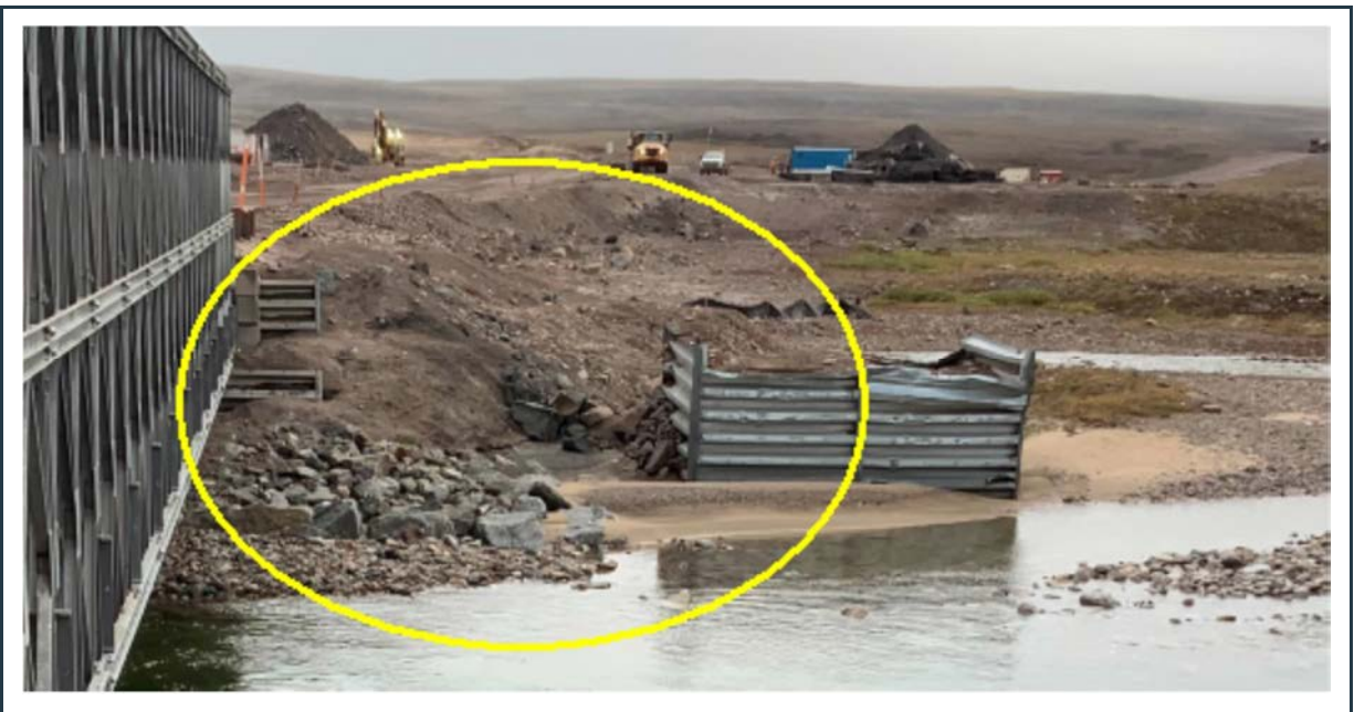
Figure 98: View the enlarged image of the area between the old and new abutments (yellow circle) where additional rock fill should be placed for erosion protection.
