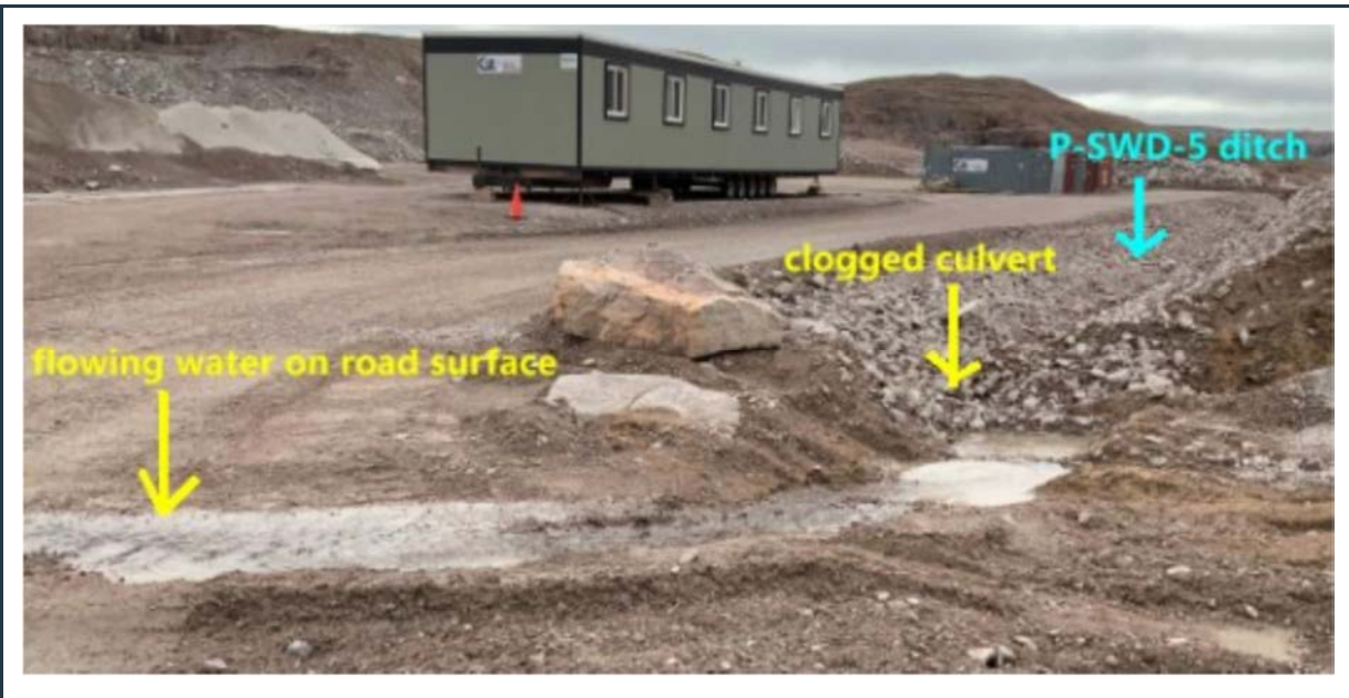
Figure 69: Poor surface water control in many areas of the lower (main) level of the Q01 rock quarry.
