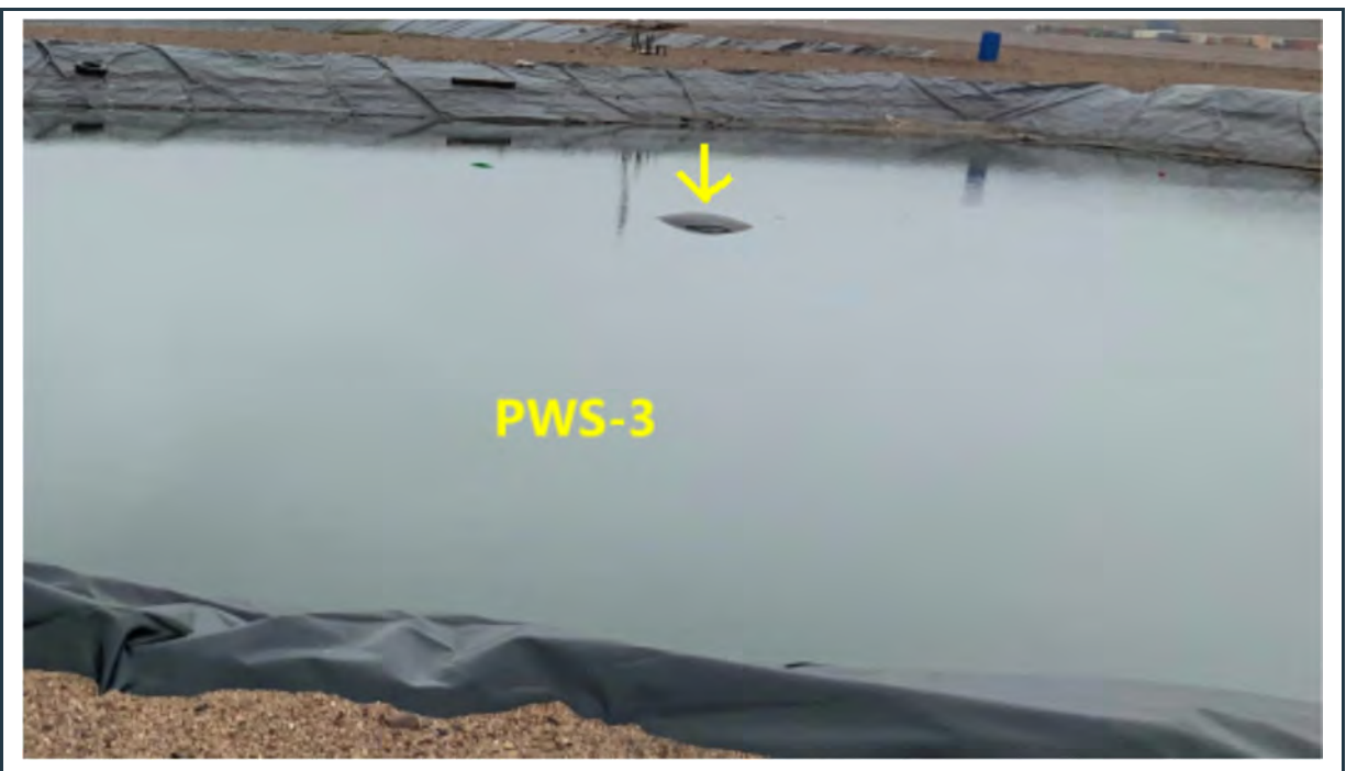
Figure 16: Robust, stable perimeter berms and intact liner at the PWS-3 pond. Note a “whale” in the pond, similar to the ones present in the neighbouring PWS-2 pond.
