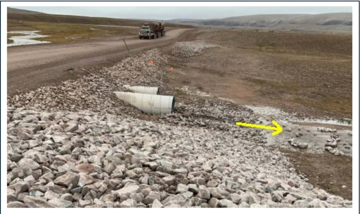
Figure 107: View of the outlet of the twin culverts at KM 36+000, in good condition.
