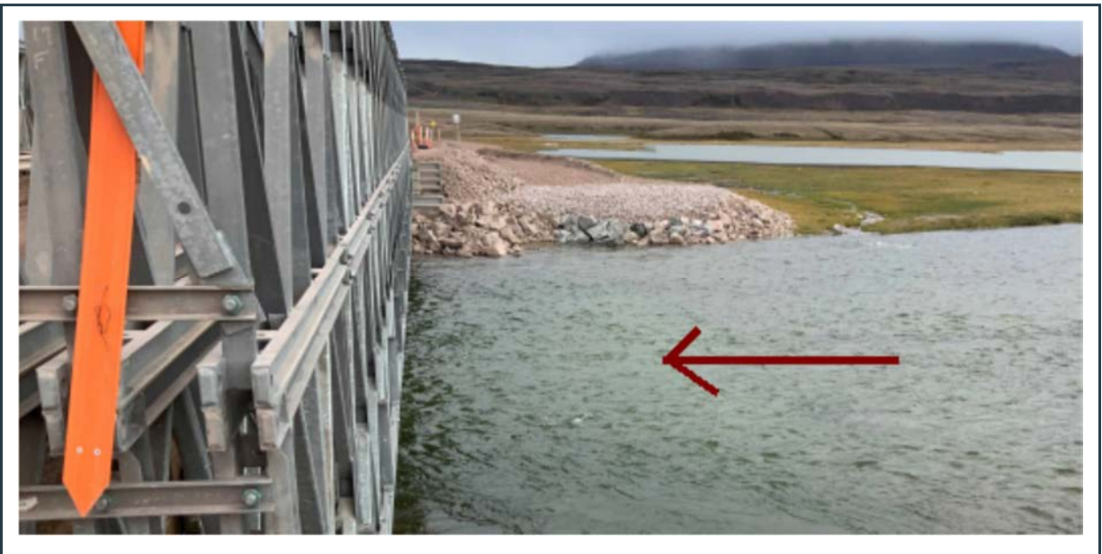
Figure 92: View of the east abutment, where the old metal crib has been removed and replaced with new riprap erosion protection at the south side of bridge KM17.
