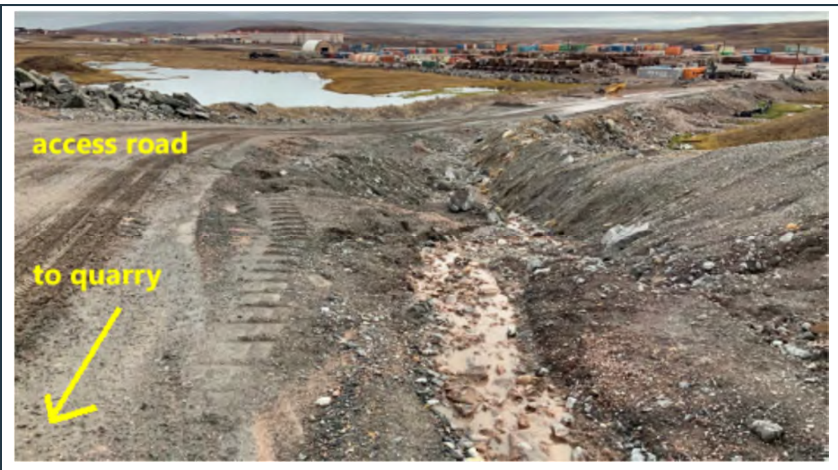
Figure 49: Serious erosion problem still exists along the edge of the access road to the quarry.
