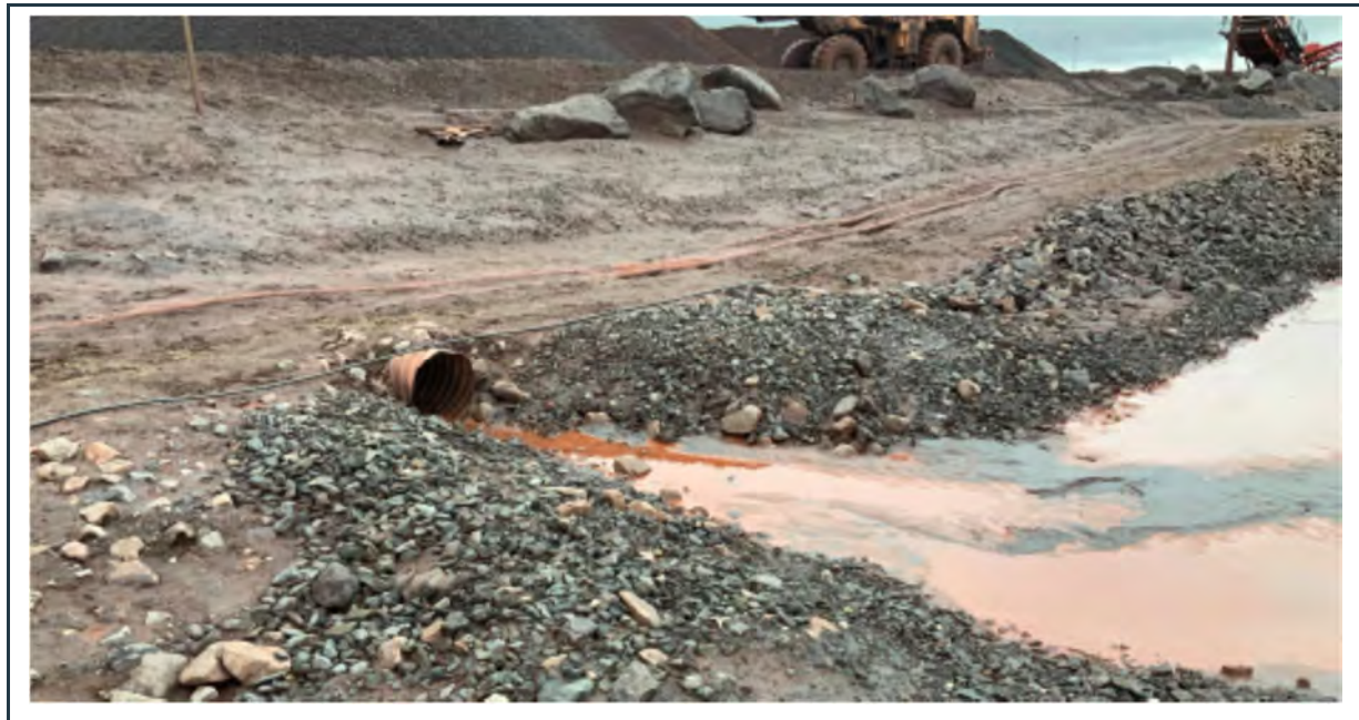
Figure 24: View of the discharge end of the recently cleaned culvert, draining the collected surface water from the crusher pad area to the MS-06 pond.
