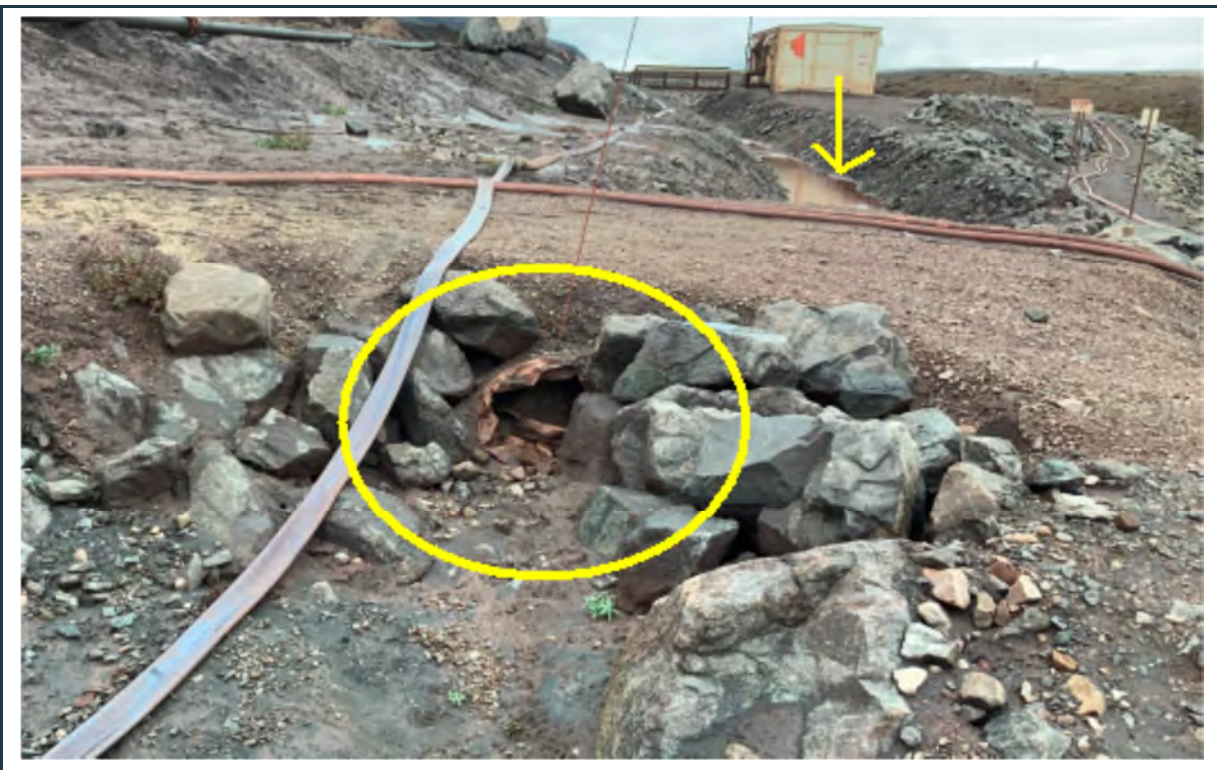
Figure 26: View of one of the side-ditches and a culvert leading to the MS-06 pond. As shown by the yellow circle, the culvert is damaged and clogged, preventing the collected water from the upstream section of the ditch (yellow arrow) reaching the pond.
