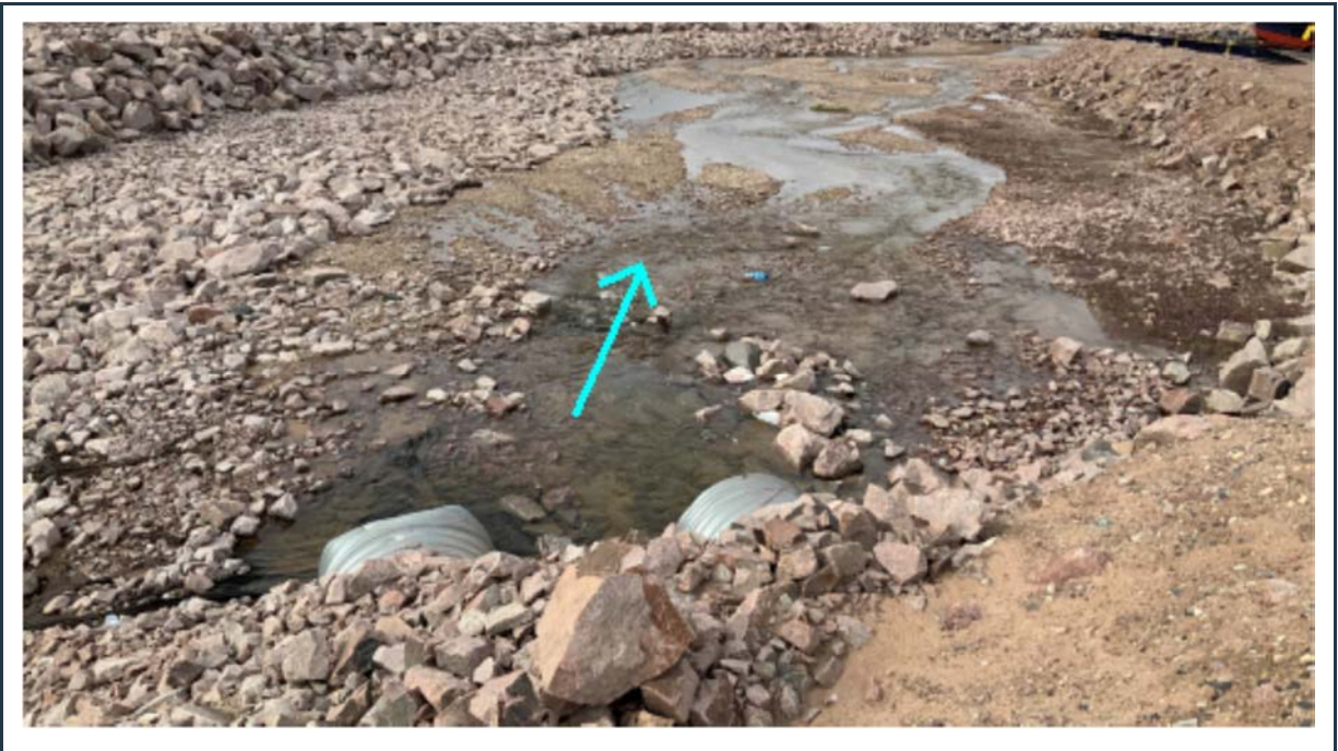
Figure 77: View of the well-maintained P-SWD-7 surface water collection ditch and culverts (outlet).
