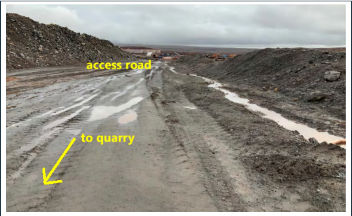
Figure 48: Drainage problems still exist at the first quarry level. Surface drainage shall be rectified.
