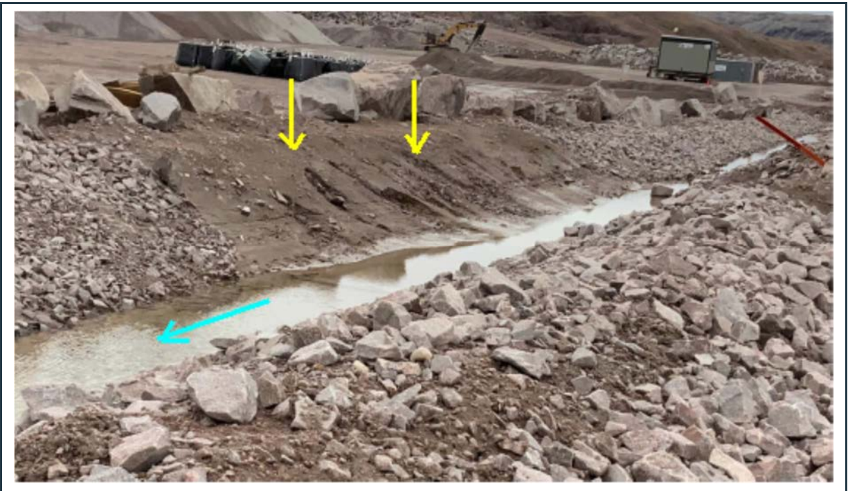
Figure 72: P-SWD-5 – “Q01-North” surface water collection ditch with missing riprap at one section of the ditch. Note the continuous seepage from the granular fill pad of the quarry’s lower level.
