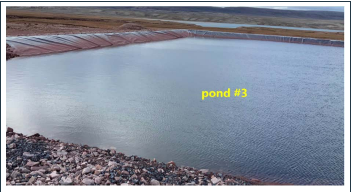
Figure 61: View of surface water management pond #3, with lined, stable berms.
