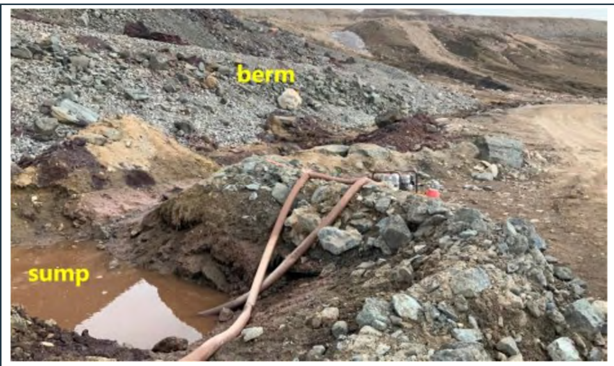
Figure 50: View of a historic image (2022) of the diversion berm, drainage ditch/swale and sump in poor conditions, south of the KM-106 ore stockpile area. See these recently upgraded infrastructure components in Figures 51 and 52 (next page).
