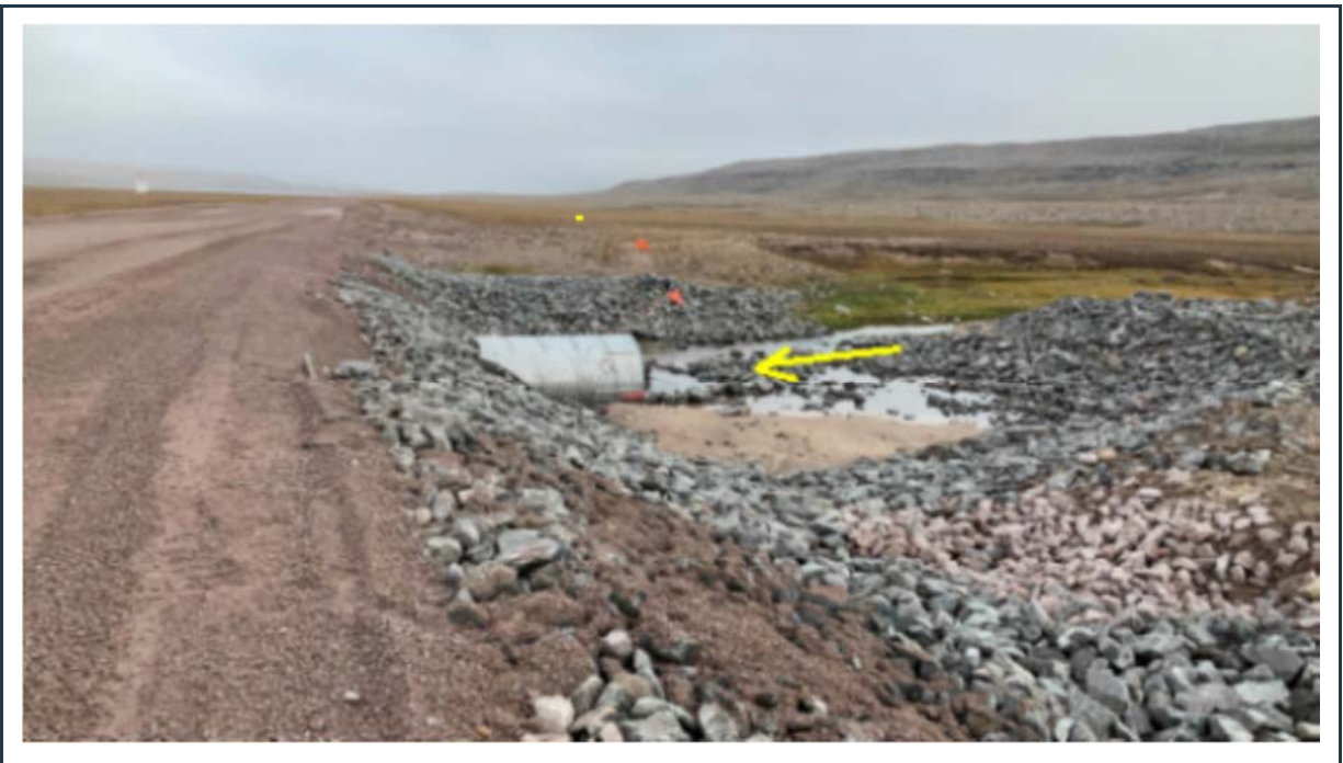
Figure 108: View of the inlet of the twin culverts at KM 59+800, in good condition.
