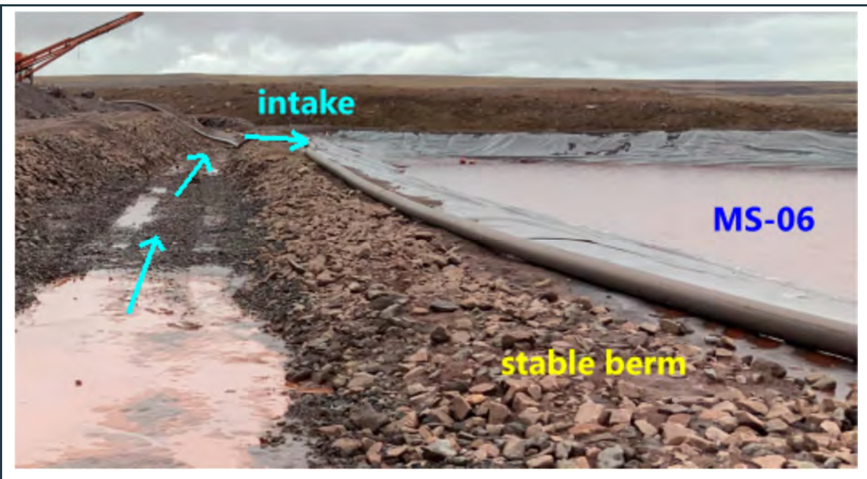
Figure 25: View of the robust, stable berm around the MS-06 pond, with intact liner.
