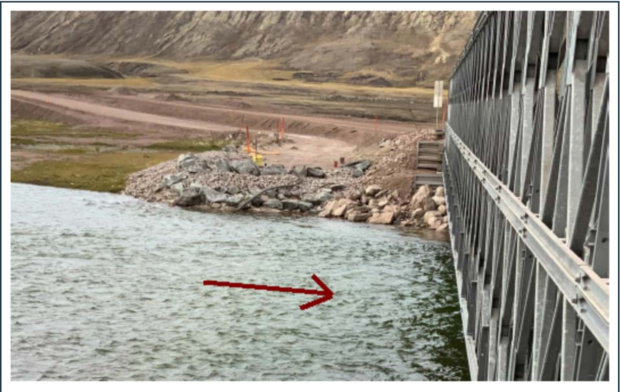
Figure 91: View of the west abutment, where the old metal crib has been removed and replaced with new riprap erosion protection at the south side of bridge KM17.
