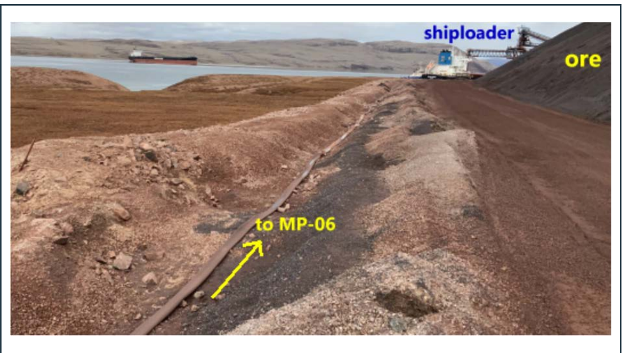
Figure 66: View of the 2023 condition of the “west” surface water collection ditch adjacent to the ore storage area, draining water from pond #3 to the MP-06 pond. This photograph was taken in 2023. Note the changes in ditch condition in Figure 67, which was taken in August 2024.
