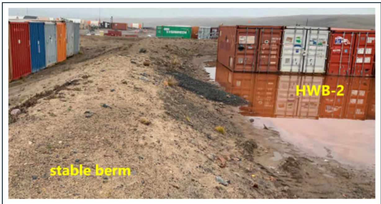
Figure 18: View of the robust, stable berm around HWB-2. The presence of water in the cell indicates good liner performance.
