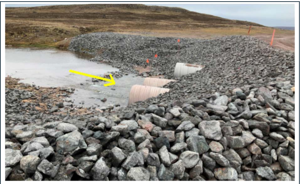
Figure 114: View of the inlet of three culverts at KM 94+060, in good condition.
