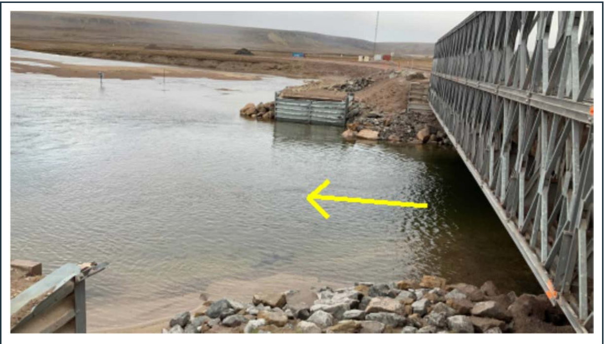
Figure 95: View of the west side of bridge 80, with riprap scour protection around the abutments.
