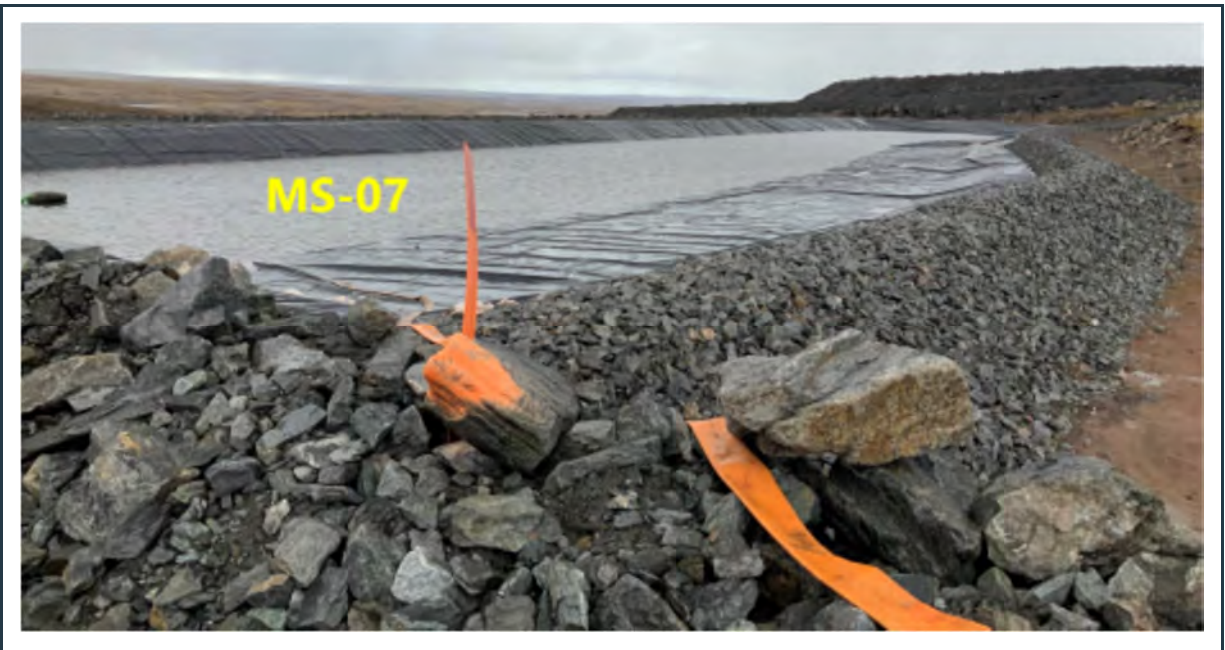
Figure 27: View of the robust, stable perimeter berm and intact liner at the MS-07 surface-water management pond at KM106.
