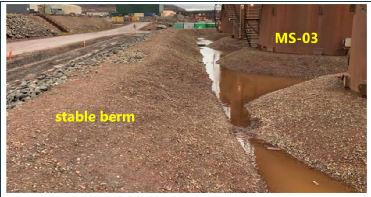
Figure 39: Well-maintained, stable berm around the MS-03 diesel fuel farm, with some ponding water, which is indication of good liner performance. Note the rock fill on the downstream slope of the berm for additional protection against erosion.
