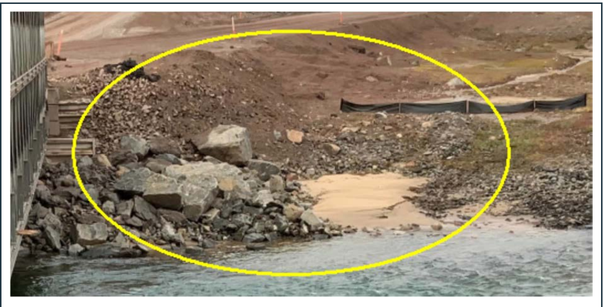
Figure 100: View of the enlarged image of the area marked by the yellow circle in Figure 99, where additional rock fill should be placed for erosion protection.
