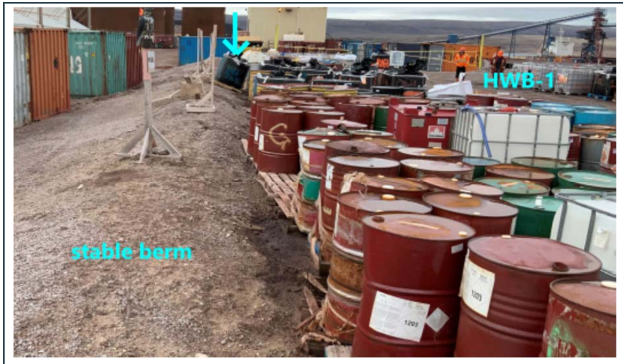
Figure 53: View of the stable perimeter berm around the lined HWB-1 cell with various materials and two shipping containers stored within the cell. Materials on pallets should be stored within the cell, not on the berms (note the container marked by the blue arrow).
