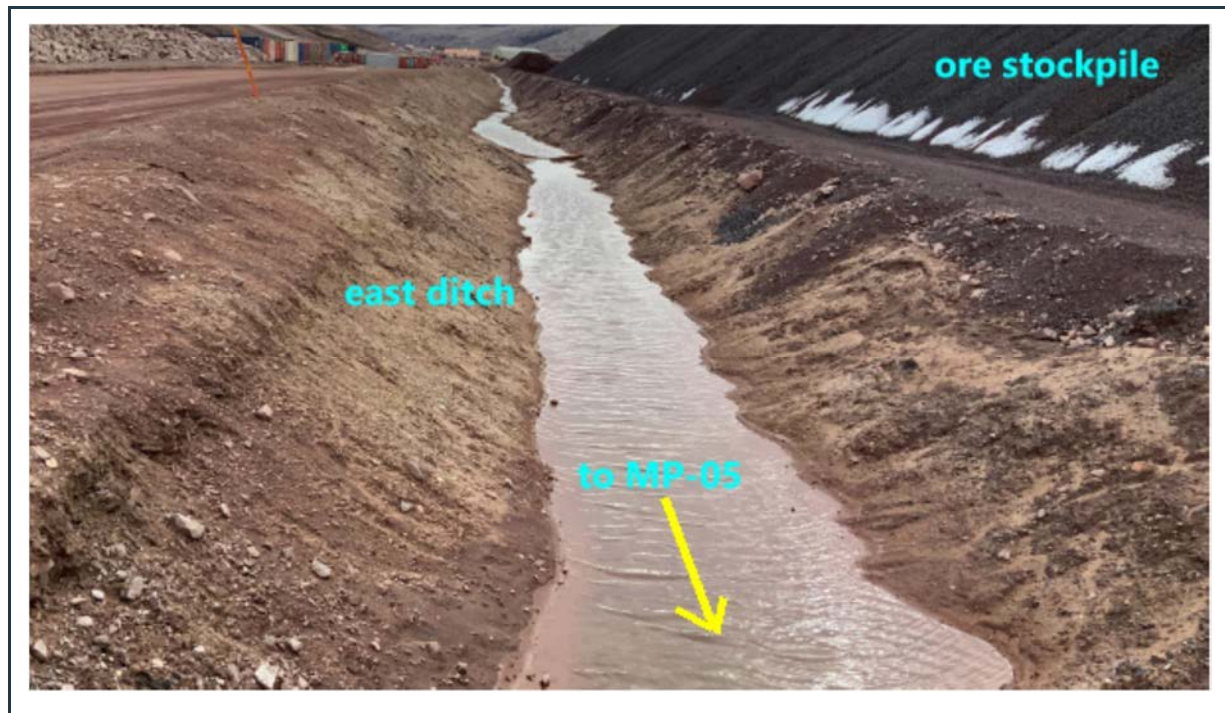
Figure 63: View of the "east" surface water collection ditch adjacent to the ore storage area, draining to the MP-05 pond.
