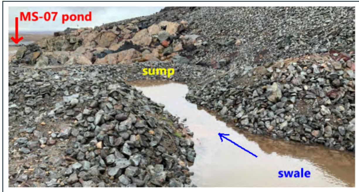
Figure 52: View of the new drainage ditch/swale and sump pit south of the KM-106 ore stockpile area, collecting local run-off. Note the recently completed riprap erosion protection along the sides of the swale and sump. Water from the sump is pumped into the nearby MS-07 pond.
