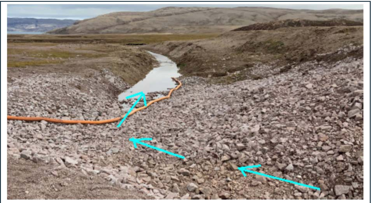
Figure 82: View of the “east end” of the PSC surface water collection ditch (also shown by green circle B in Figure 8). Additional riprap and a check dam should be installed along this section of the ditch.
