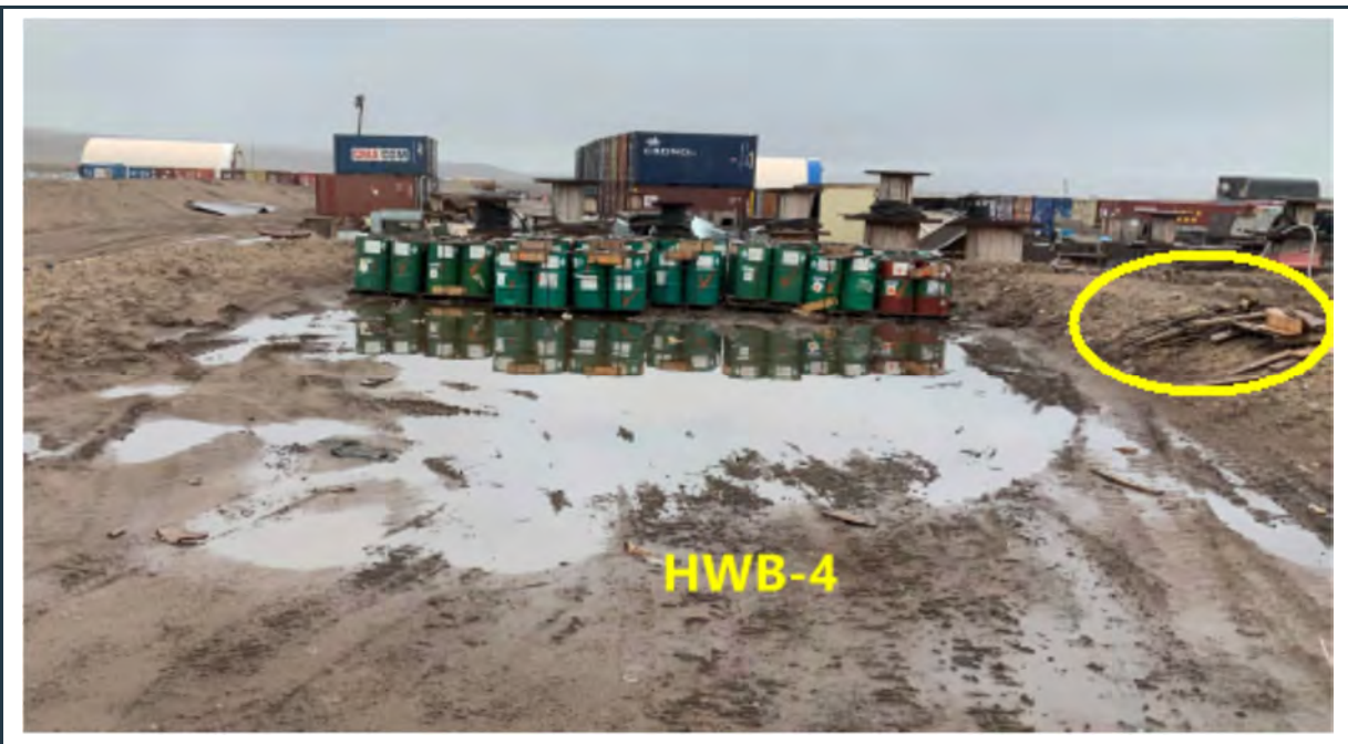
Figure 20: View of stable perimeter berm around the HWB-4 cell, with fuel barrels on wooden pallets stored in the cell. The presence of water in the cell indicates good liner performance. The debris, visible on the right berm, should be removed and disposed (yellow circle).
