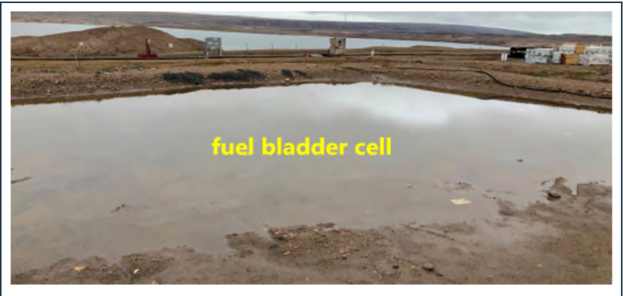
Figure 37: View of the stable perimeter berm around the empty “fuel bladder” cell. The ponding water in the cell indicates good liner performance.
