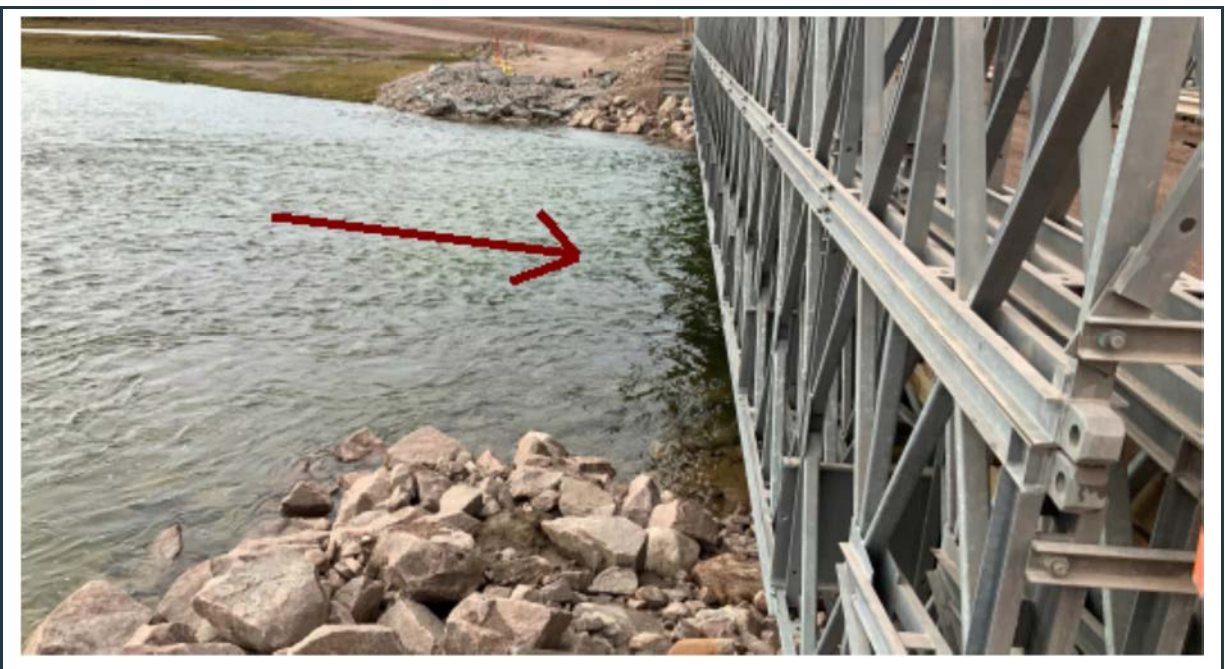
Figure 90: View of the stable abutments with riprap scour protection at the south side of bridge KM-17.
