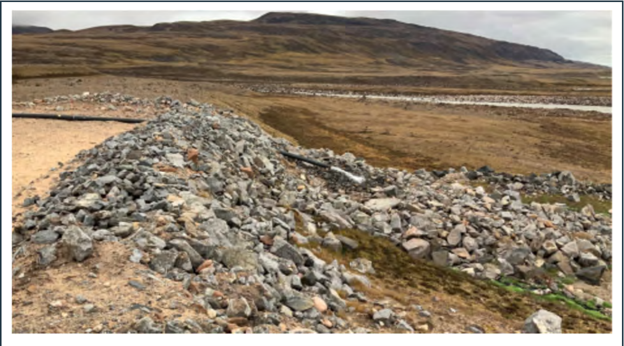
Figure 47: View of the stable slope with rockfill erosion protection at the water discharge area.
