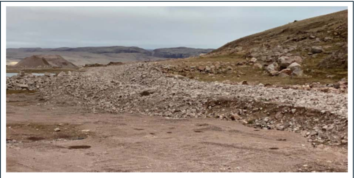
Figure 74: View of the P-SWD-6 surface water collection ditch. As opposed to the original design intent, no water is drained from the quarry in this ditch with its invert level constructed above the current (lower) level of the quarry (see Figure 75 as well).
