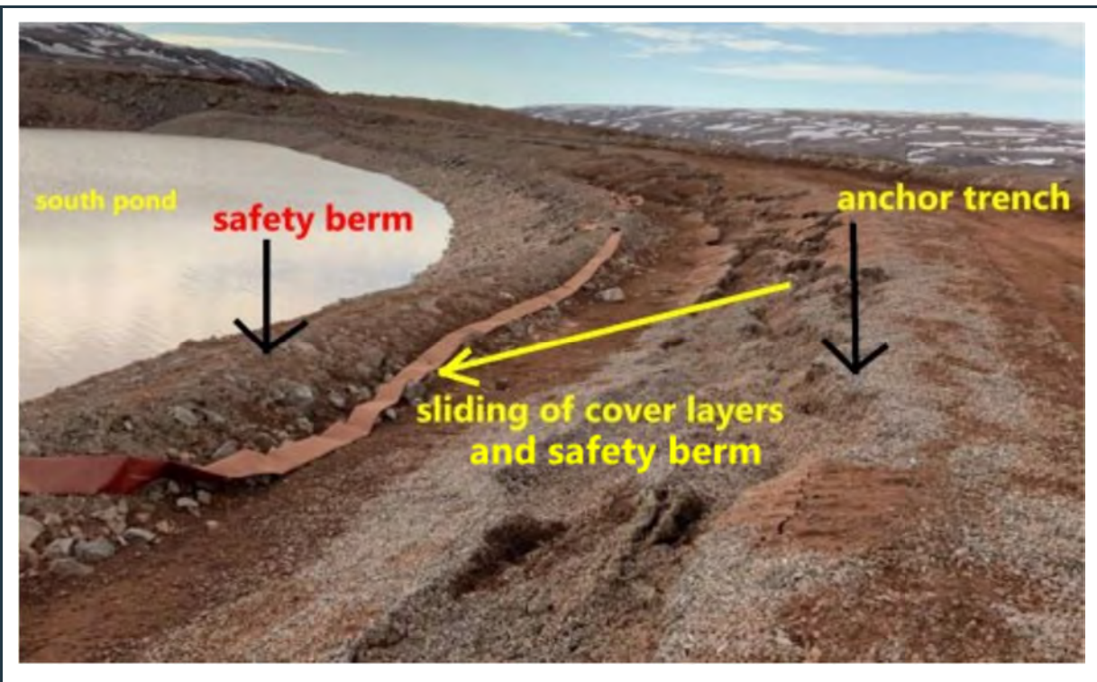
Figure 35: Sliding of the cover layers and safety berm above the liner in the south pond (image was taken on June 22, 2022).
