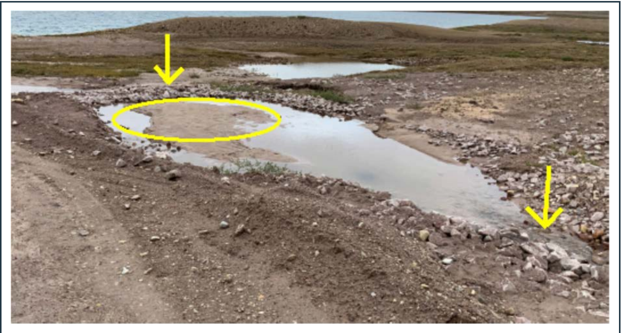
Figure 103: View of the ditch and check dams at KM 32+900. The ditch should be cleaned (yellow circle) and the crest of the check dams repaired/raised (yellow arrows) during maintenance work.
