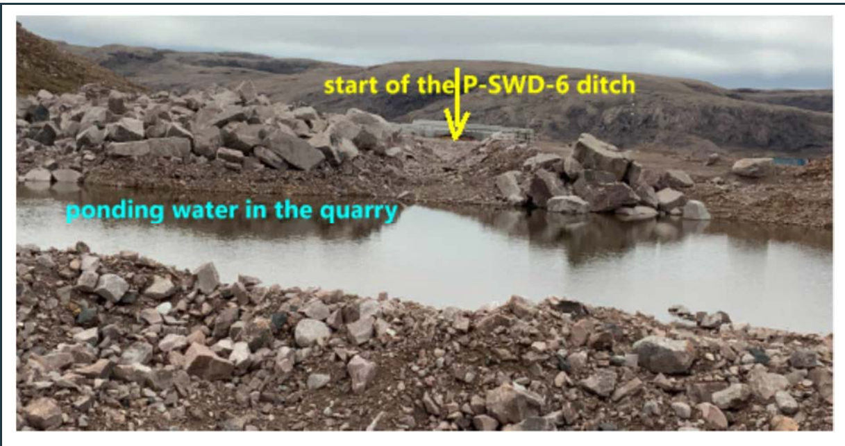
Figure 75: View of the over-excavated southern area of the Q01 quarry with ponding water (see Figure 11 for location). Note the start of the P-SWD-6 ditch in the image, with its invert level well above the new ground level in the area (bottom of the pond).
