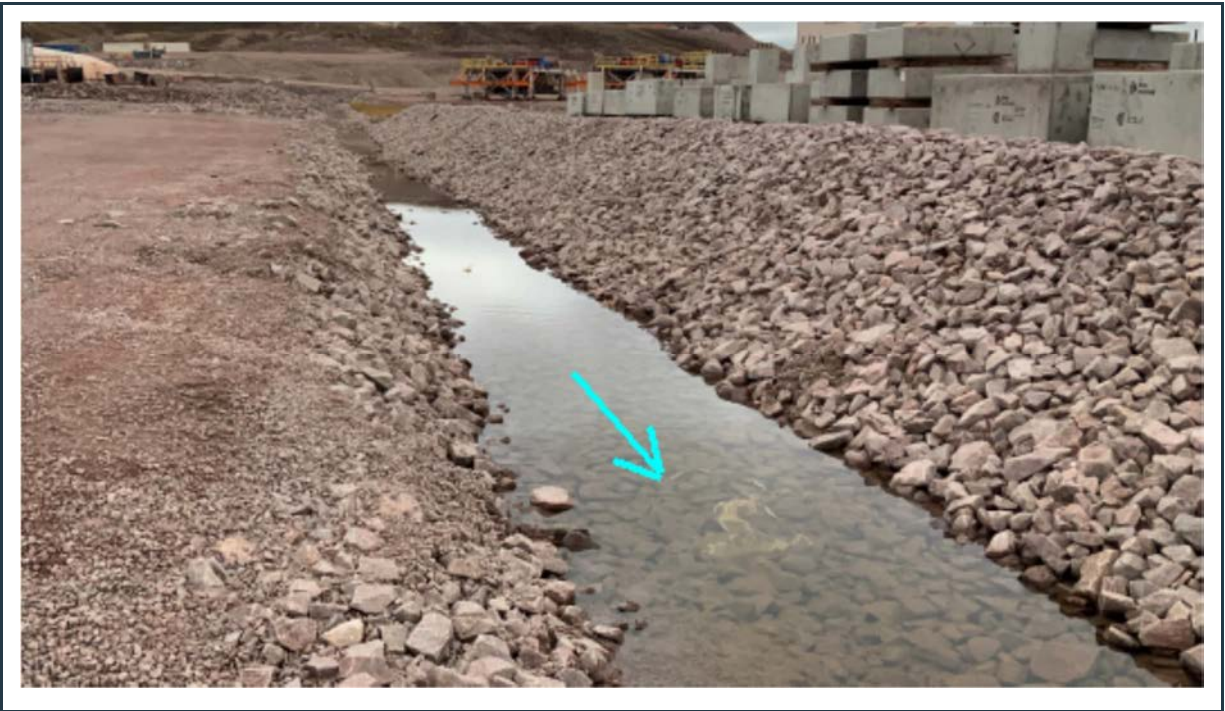
Figure 79: View of the well-maintained south section of the 380-Person Camp surface water collection ditch.
