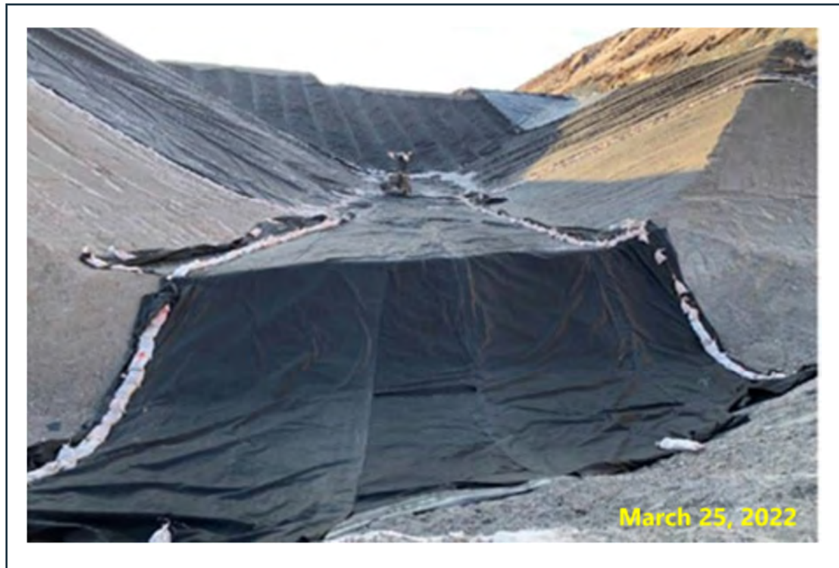
Figure 33: Installation of HDPE liner into the anchor trench at the toe of the main dam at MS-11.
