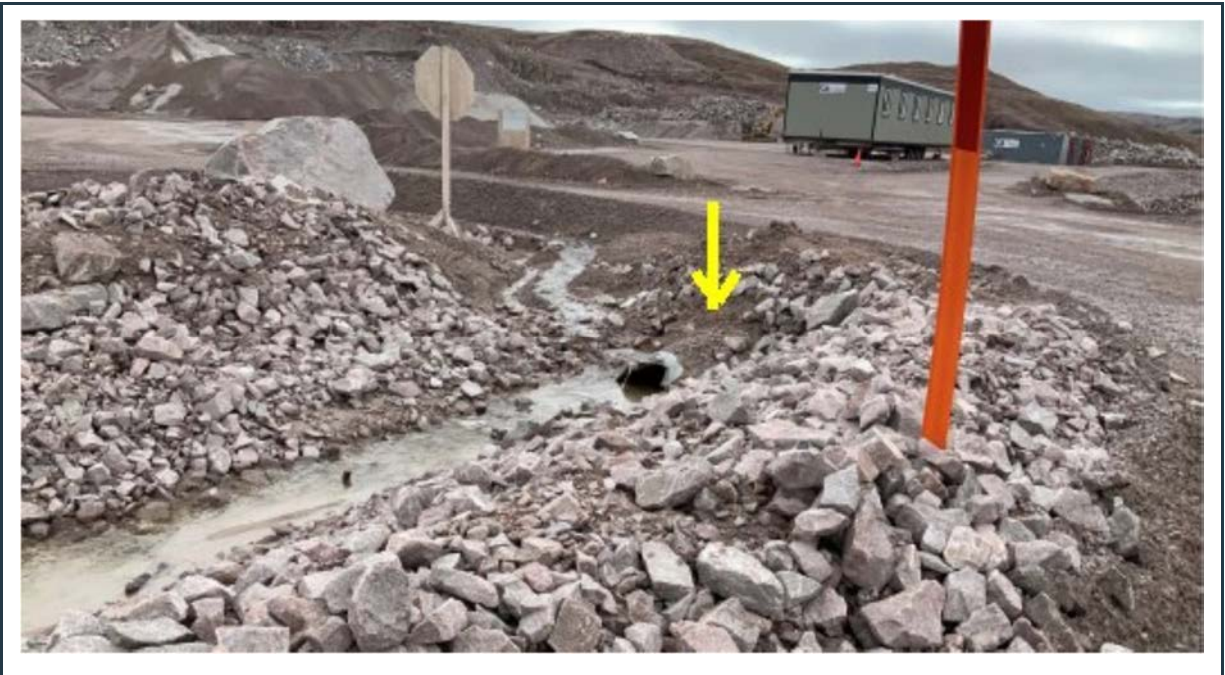
Figure 73: View of the clogged, undersized culvert beneath the access road to the Q01 rock quarry. This culvert should be removed and replaced with a larger diameter pipe.
