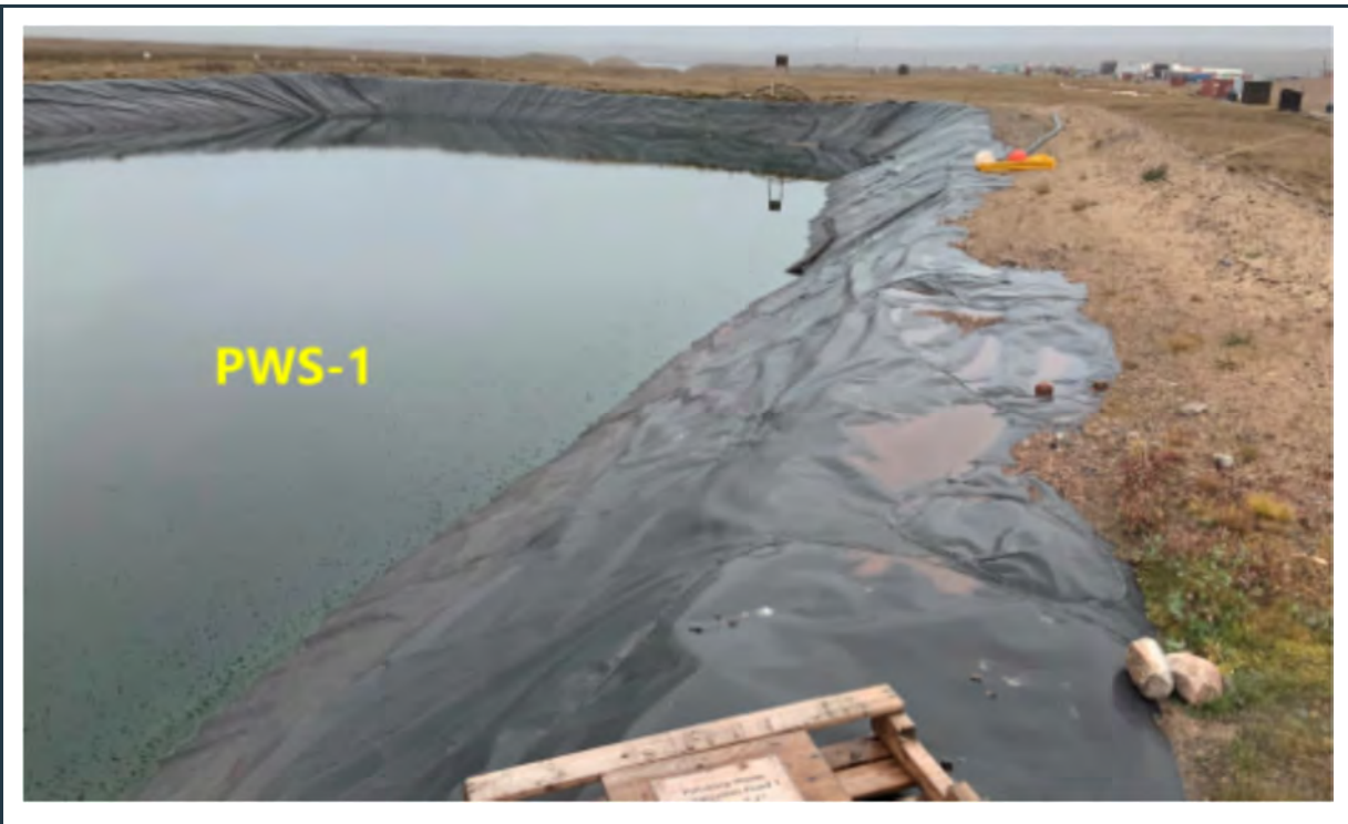
Figure 14: PWS pond #1. Well-maintained, stable perimeter berm and intact liner at the pond.
