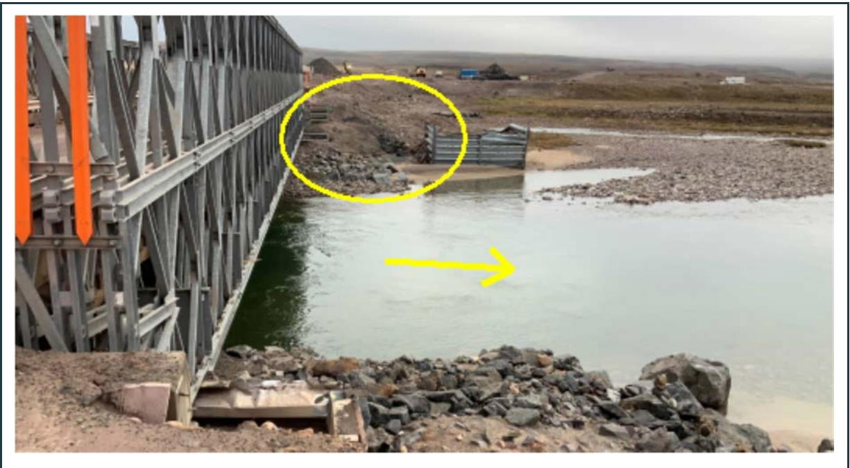
Figure 97: View of the stable abutments at the west side of bridge KM 97. As shown, there is only one remaining old crib abutment present at this bridge. Note the area between the old and new abutments (yellow circle) where additional rock fill should be placed for erosion protection.
