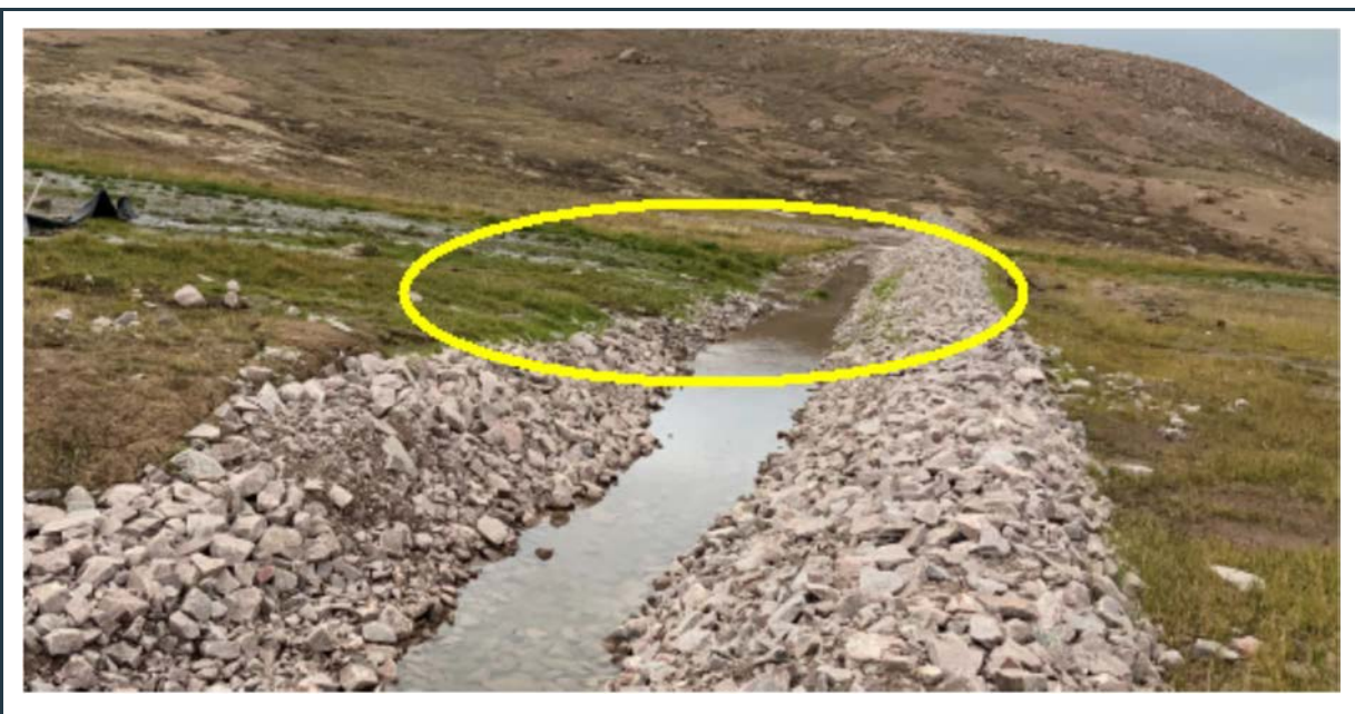
Figure 70: View of the southern section of the P-SWD-3 surface water collection ditch with failed slope sections and ponding water due to inadequate longitudinal channel slope.
