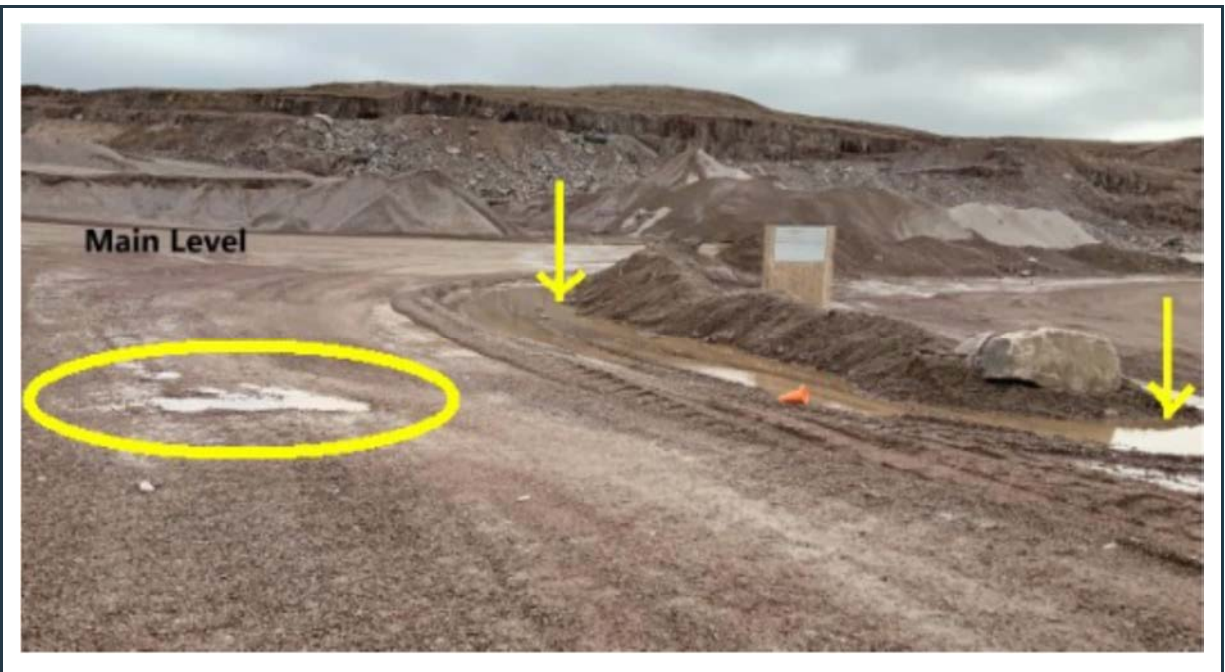
Figure 68: View of ponding and flowing water at many areas of the lower (main) level of the Q01 rock quarry. The drainage problem should be rectified prior to restarting the operation in the quarry.
