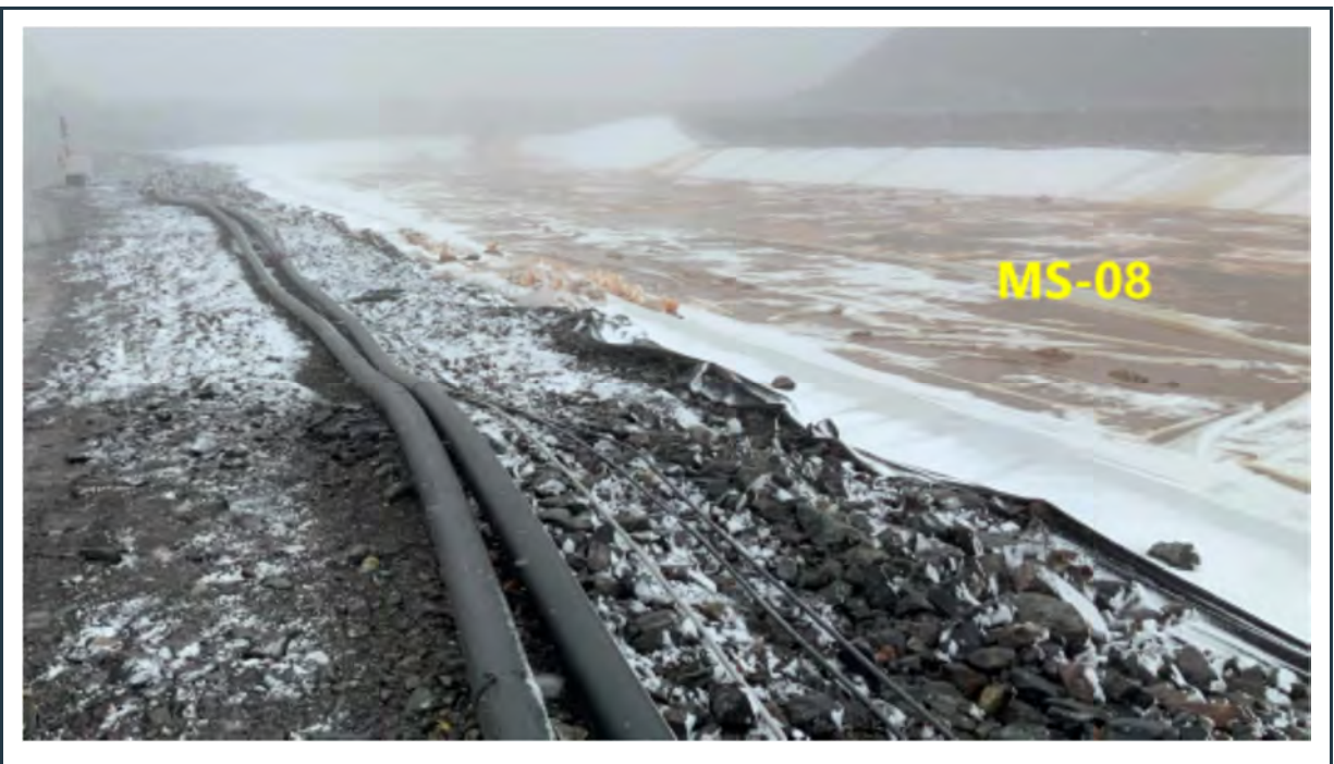
Figure 28: View of the stable, robust berm and intact liner at the MS-08 pond, which was almost empty at the time of the August 2024 visit. Note the snow already on the ground in August.
