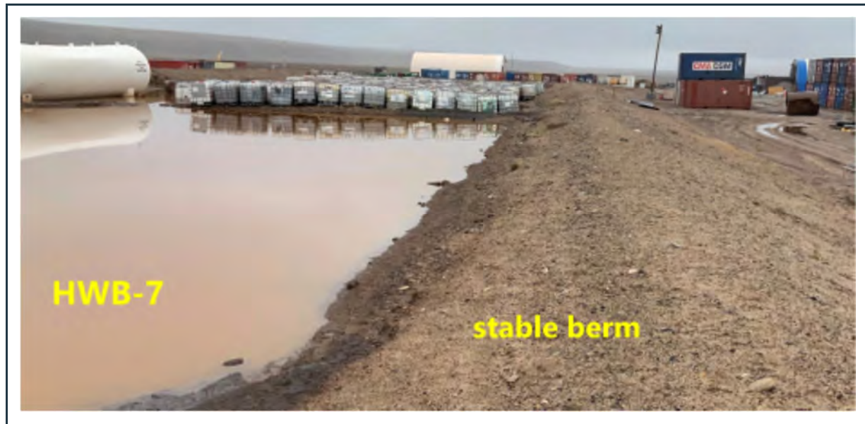
Figure 23: View of the stable berm around the HWB-7 cell, with an old fuel tank and oil filled plastic containers stored in the cell. The ponding water indicates good liner performance.
