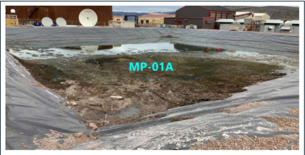
Figure 57: View of the robust, stable berm and intact liner at the practically empty MP-01A pond.
