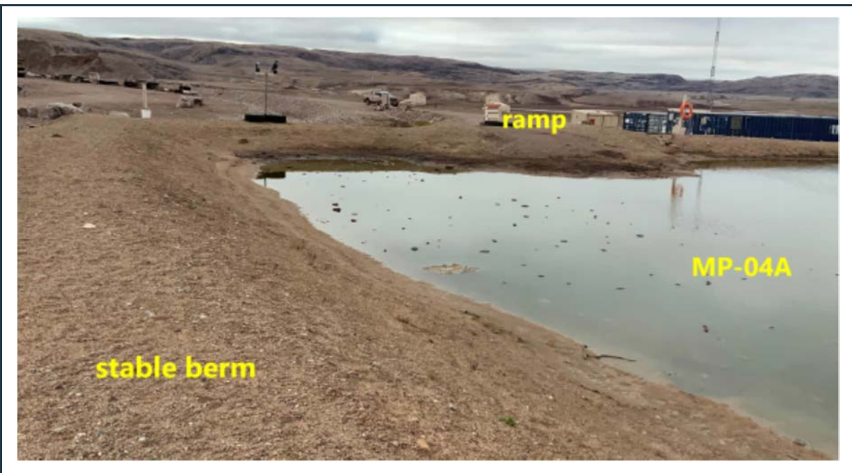
Figure 60: View of the lined MP-04A contaminated snow disposal cell with robust, stable perimeter berm. The ponding water (melted snow) indicates good liner performance. Additional protective layer of sand and gravel fill was placed recently over the access ramp.
