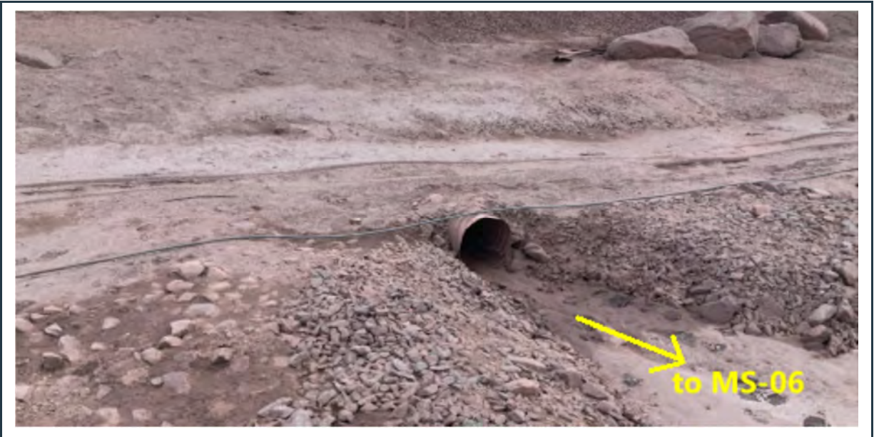
Figure 24: View of the discharge end of the recently cleaned culvert, draining the collected surface water from the crusher pad area to the MS-06 pond. See culvert A in Figure 2 for location.
