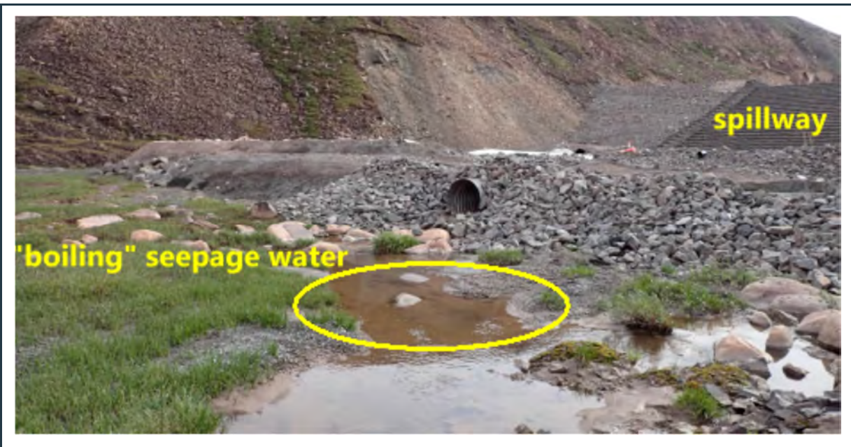
Figure 33: View of the location of "boiling" seepage water at the downstream toe of the spillway of the main dam at MS-11.
