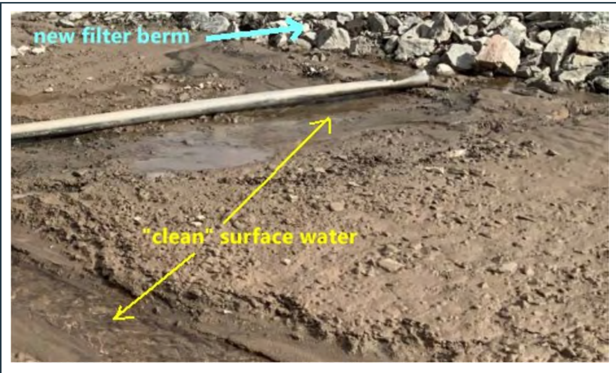
Figure 37: View of the "clean" surface water past the new filter berm in the south pond.
