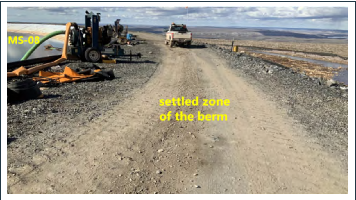
Figure 30: View of a settled zone of the berm, where two pumps are located. The anchor trench of the liner is still in its original position. The crest of the berm along this zone should be raised to its original crest elevation by crushed aggregate.
