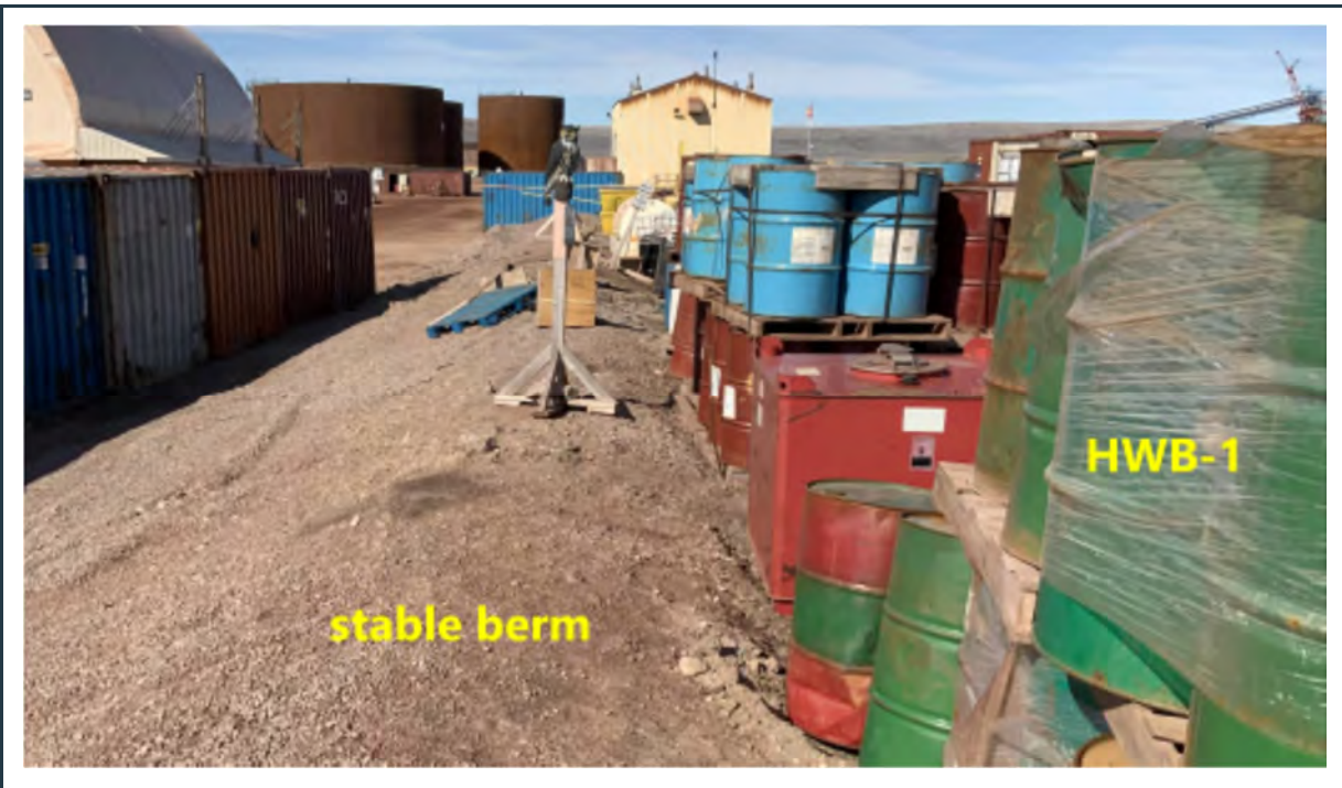
Figure 48: View of the stable perimeter berm around the lined HWB-1 cell with various materials and seven shipping containers stored within the cell. Materials on pallets should be stored within the cell, not on the berms.
