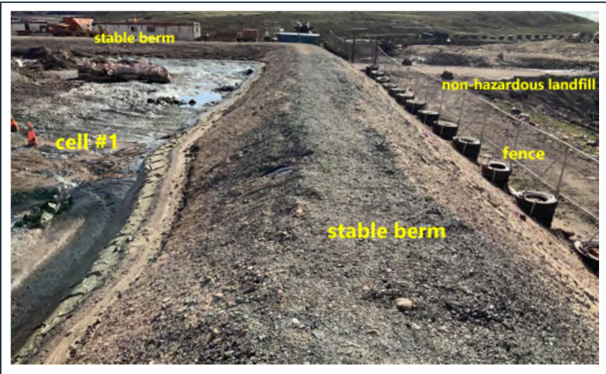
Figure 43: View of a section of the stable berm at the lined landfarm's cell #1.
