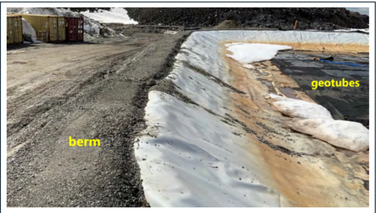
Figure 31: View of the refurbished perimeter berm and new liner at the geotube pond, located adjacent to the water treatment plant.
