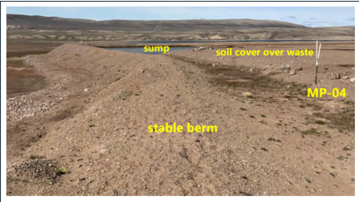
Figure 54: View of stable perimeter berm around the MP-04 landfarm, with ponding water in one corner of the cell (sump). Note the standard soil cover over the buried solid waste.
