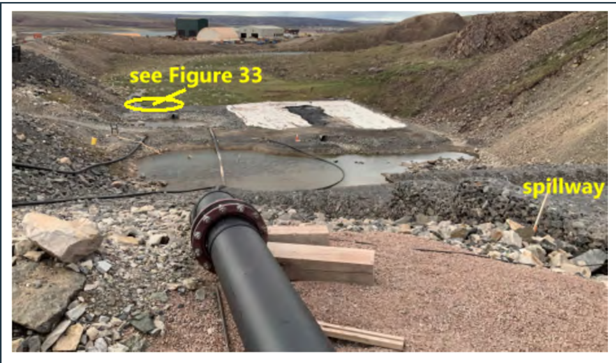
Figure 32: View of the downstream side of the spillway at the main dam of the KM105 sedimentation control pond. The presence of water at the toe is the result of "piping" beneath the dam. See the enlarged image of the location marked by the yellow circle in Figures 33 and 34.
