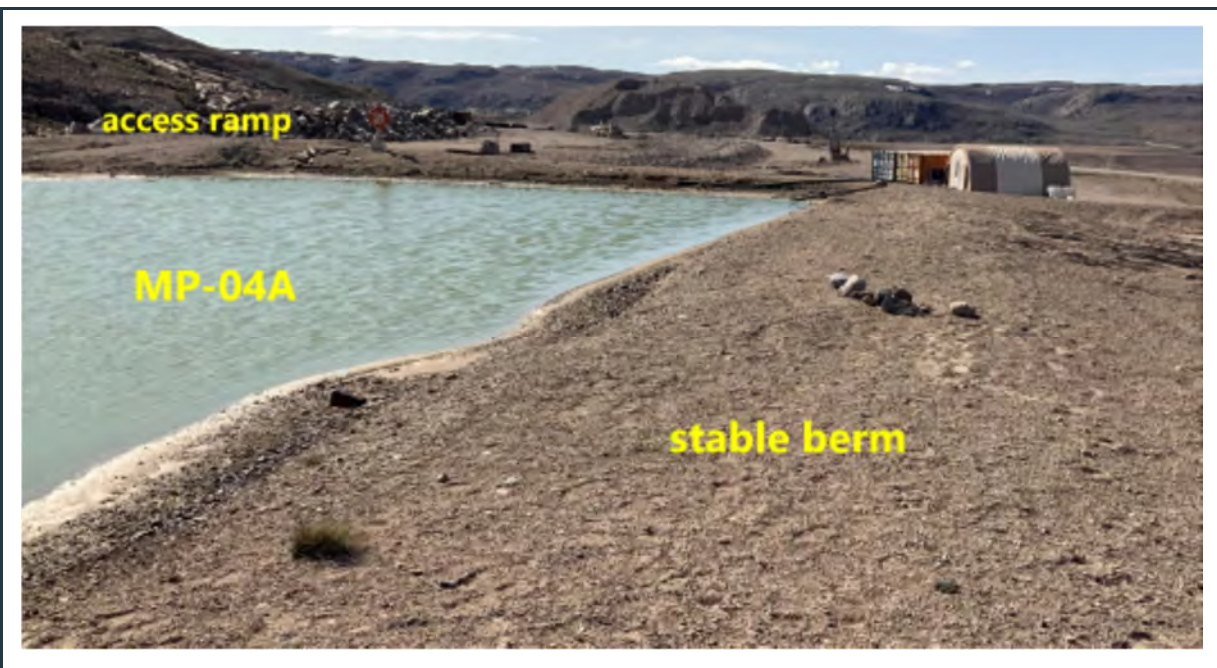
Figure 55: View of the lined MP-04A contaminated snow disposal cell with robust, stable perimeter berm. The ponding water (melted snow) indicates good liner performance.
