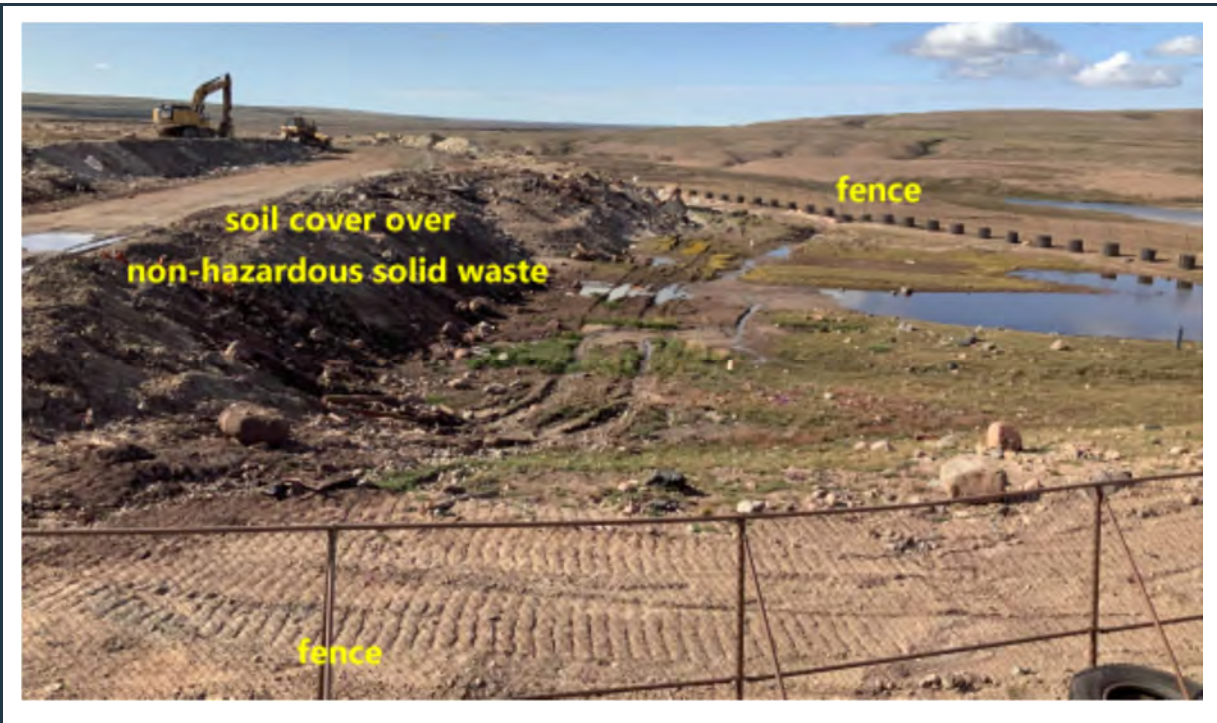
Figure 42: View of soil cover over non-hazardous solid waste in the fenced-in, gated landfill facility.
