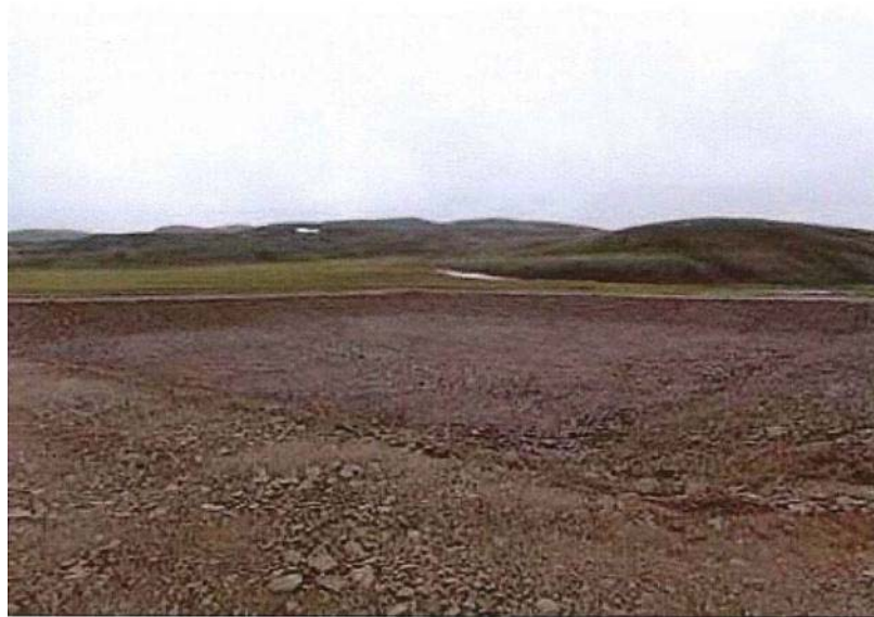
Figure 1: Before – Sub-grade Prepared
