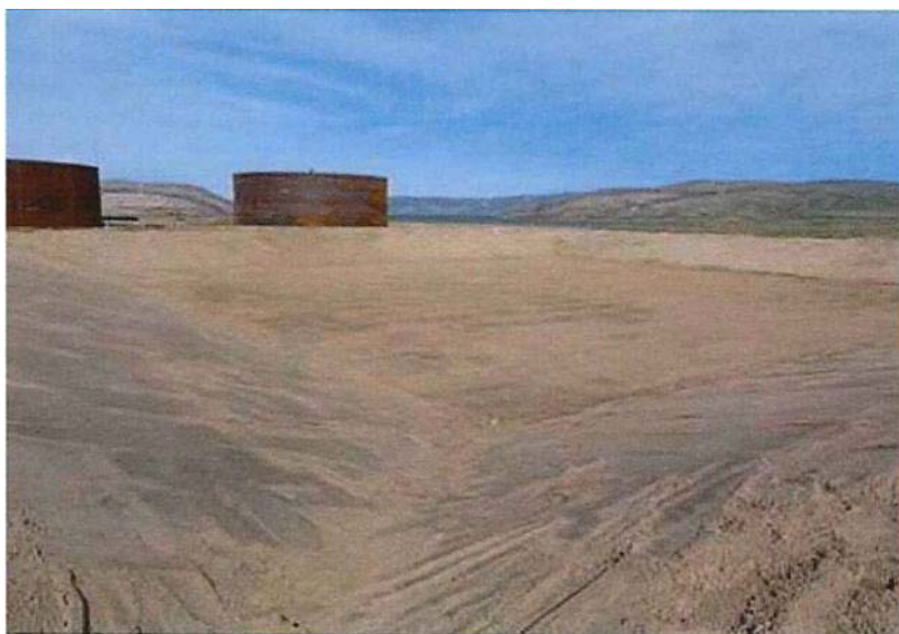
Figure 3: During - Liner Installed
