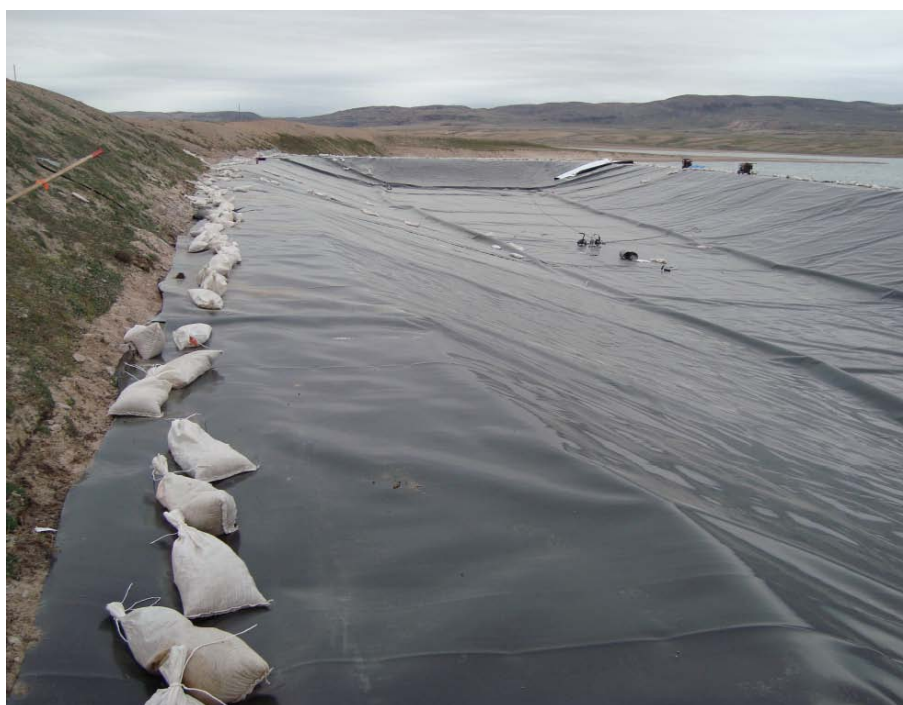
Figure 2: Pond No. 1 (west pond) placing the liner [southwest view].
