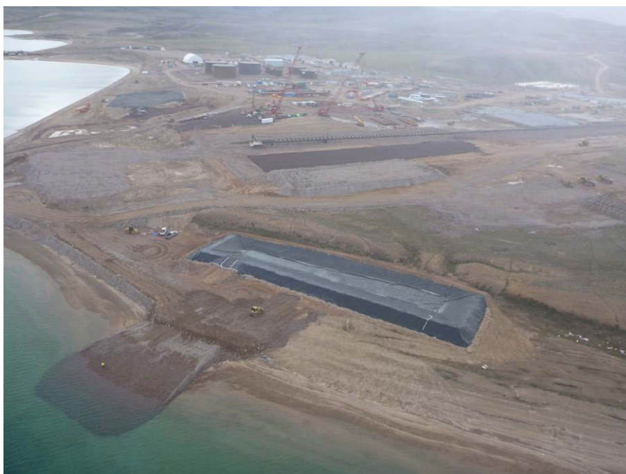
Figure 4: Aerial photo of in-progress Pond No. 1 (west pond) with liner in place [east view].
