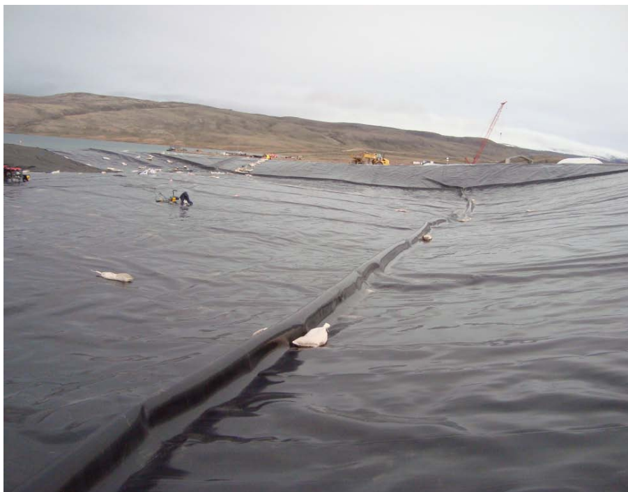
Figure 9: Pond No. 2 (east) placing the liner [southeast view].
