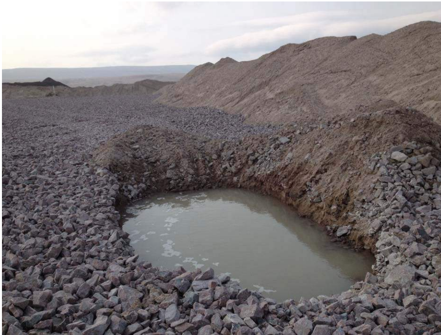
Figure 7: Pond No. 2 (east) high moisture sub-grade soils encountered during excavation. Discussed further in Section 5 Field Decisions, below.
