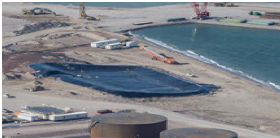
Figure 11: Aerial photo of in-progress Pond No. 2 (east pond) liner being sealed [north view].
