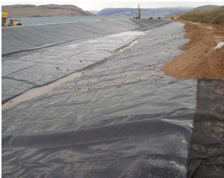
Figure 3: Pond No. 1 (west pond) liner installed [northeast view].
