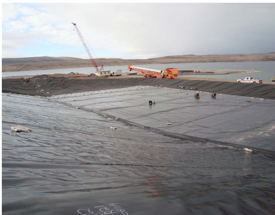
Figure 10: Pond No. 2 (east pond) liner installed [northwest view].
