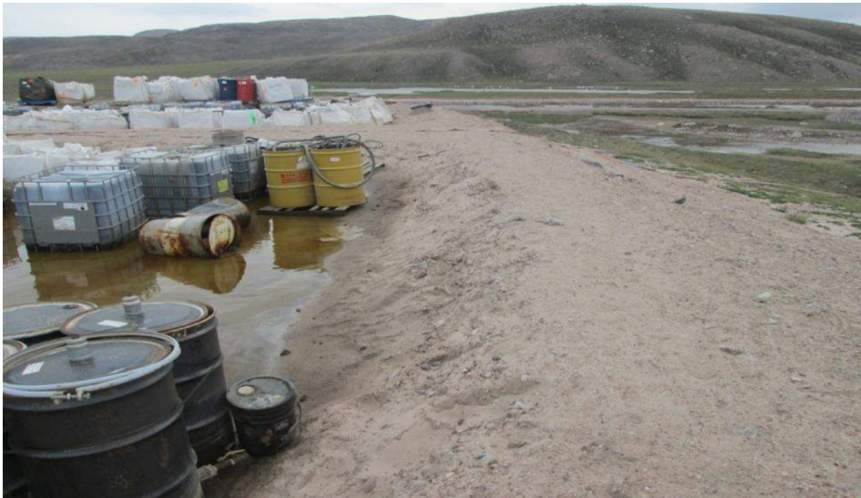
Photos taken along rear dyke at hazardous waste storage area. Note water contained within dyke.
