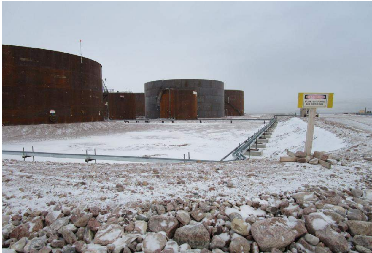
Fuel tank farm containment
