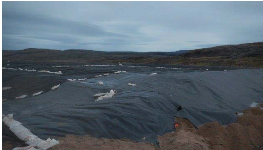
Figure 9: Contaminated Snow Containment - Liner ballasted in place with sand bags ready for seam sealing.
