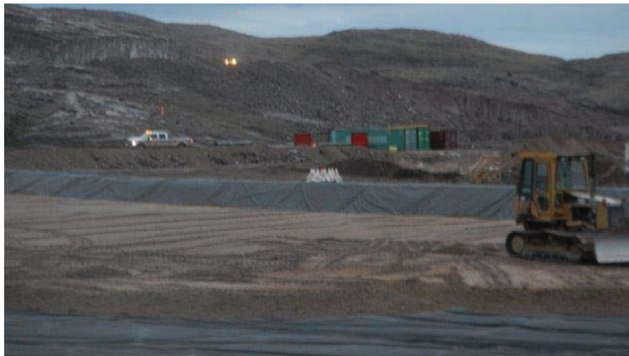
Figure 8: Landfarm - Smoothing fill layer.
