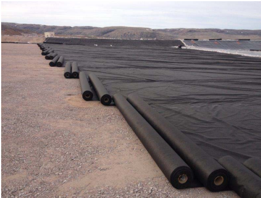
Figure 4: Laying out the liner for installation in landfarm package.
