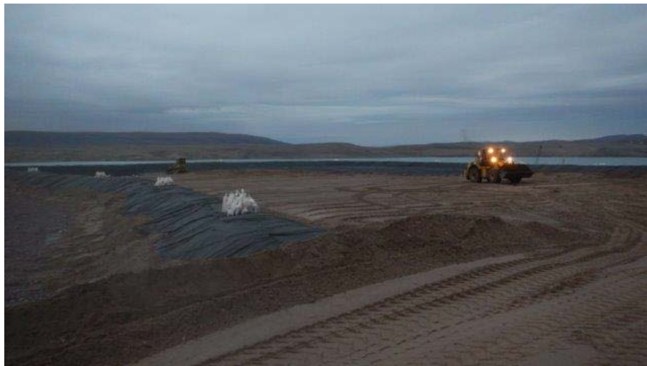
Figure 6: Landfarm – Installation of fill layer on top of installed liner layers.
