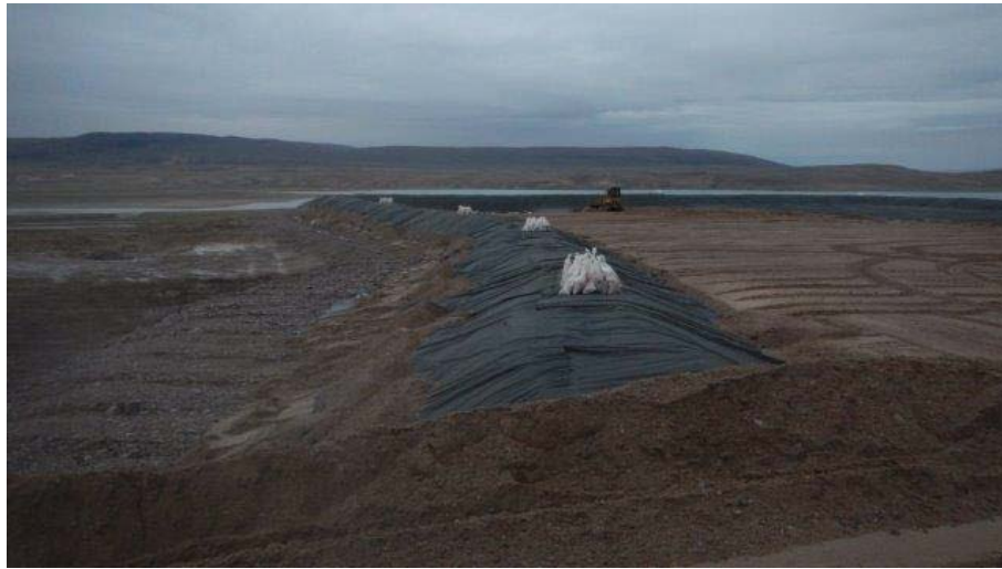
Figure 7: Landfarm – Finishing installation of fill layer on top of liner layers (showing berm between landfarm and contaminated snow area).
