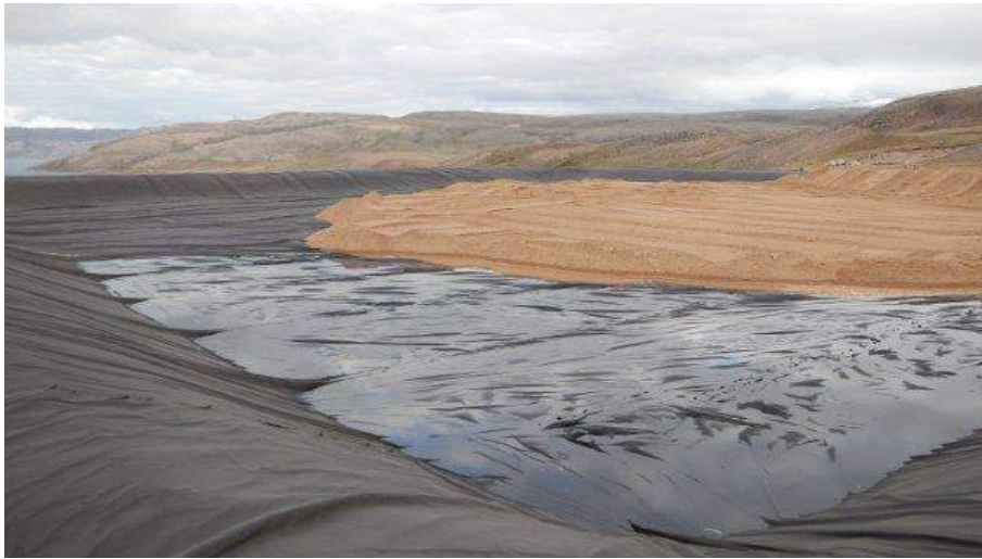
Figure 11: Contaminated Snow Containment - Liner installation complete.
