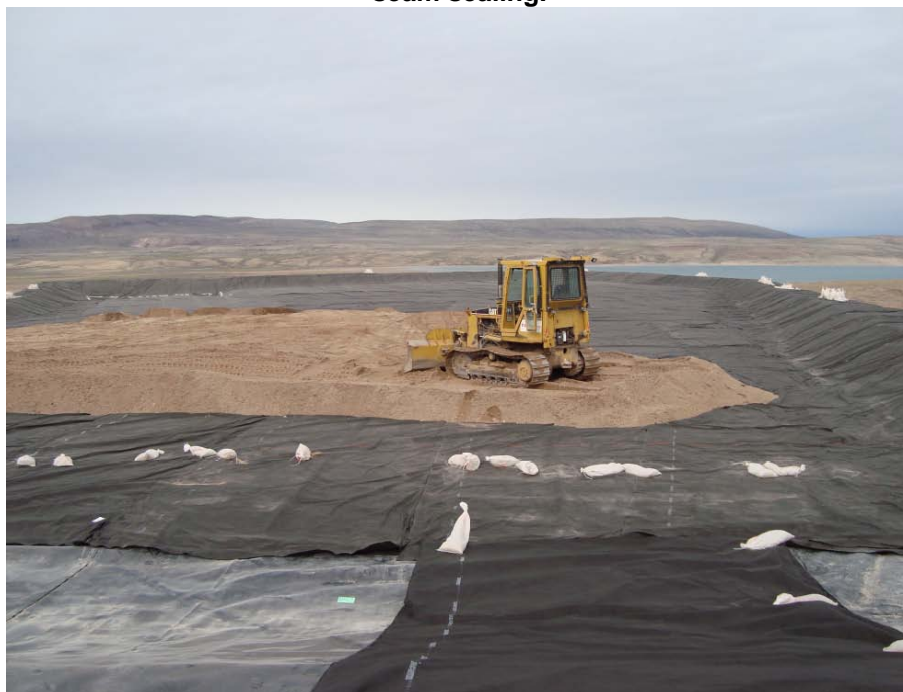
Figure 10: Contaminated Snow Containment – Placing fill on liner.
