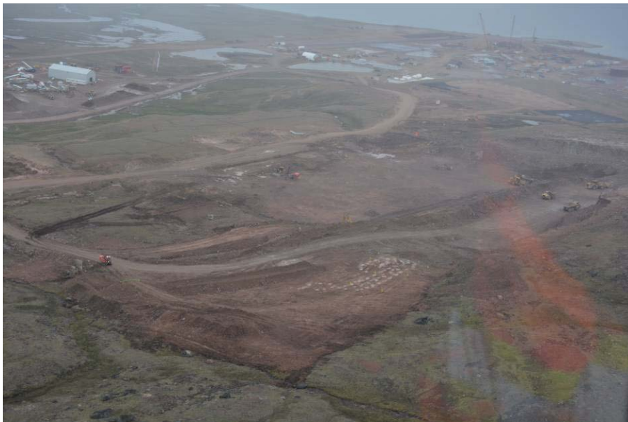
Figure 2: Landfarm package earthworks in-progress, preparing sub-base [northwest view].
