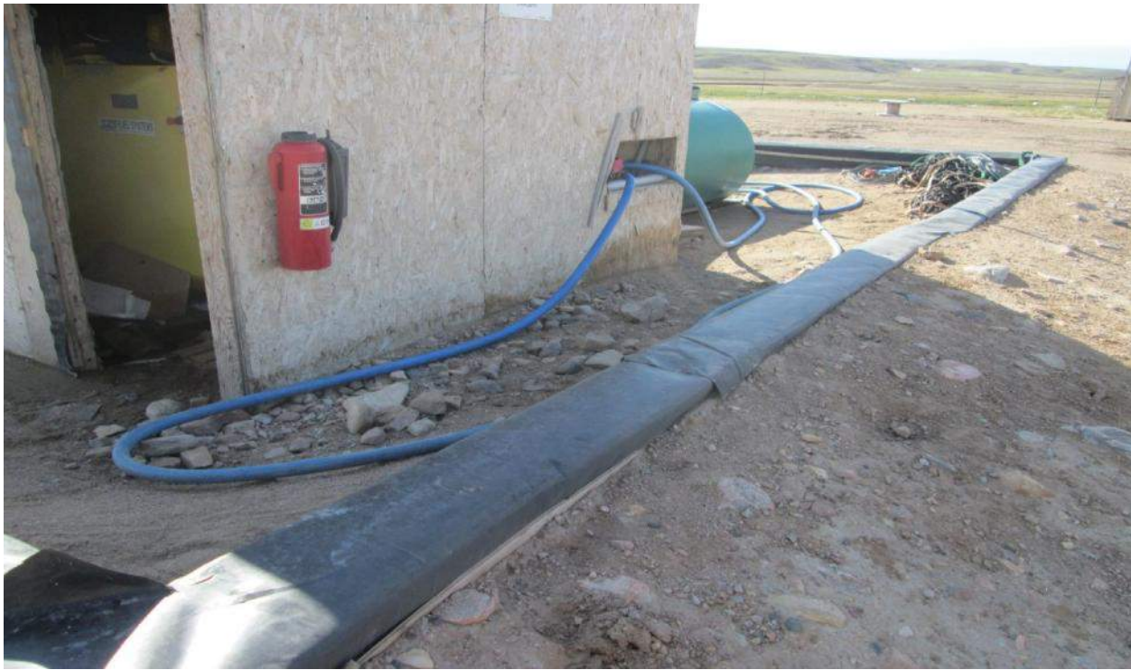
Helicopter Fuel Tank Containment.
