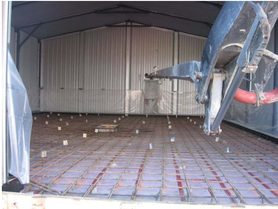
Figure 4: Installation of floor insulation and reinforcing rebar
