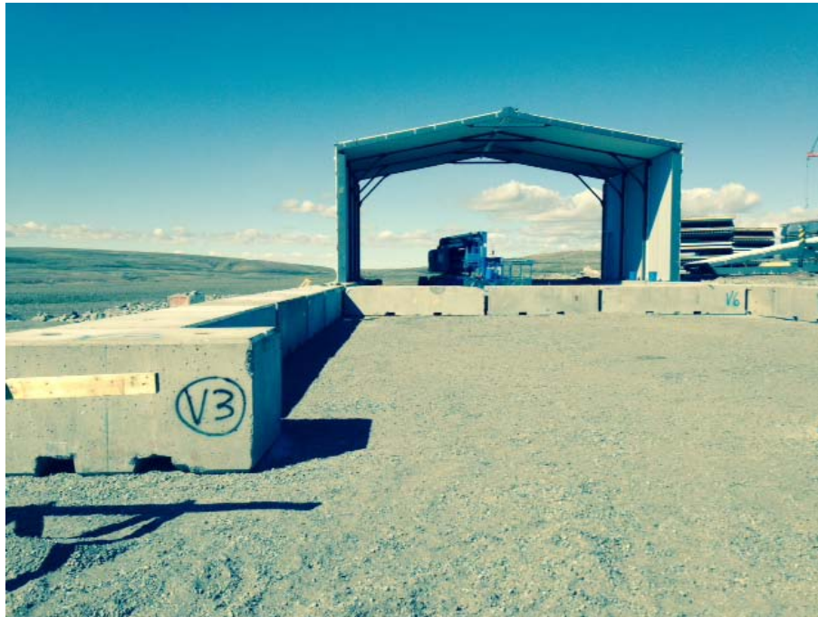
Figure 2: Precast foundation blocks and fold out building erection
