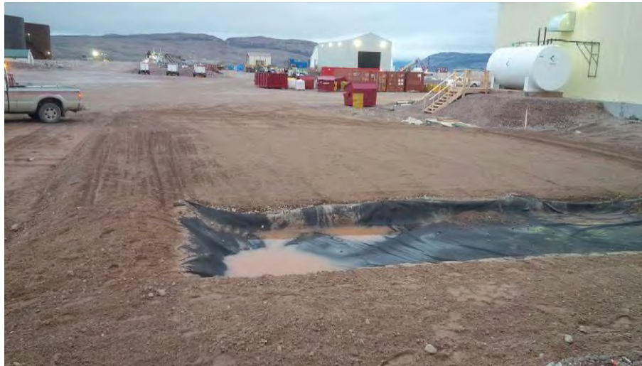
Figure 19: South hazardous containment area: Liner installed and berm shaped
