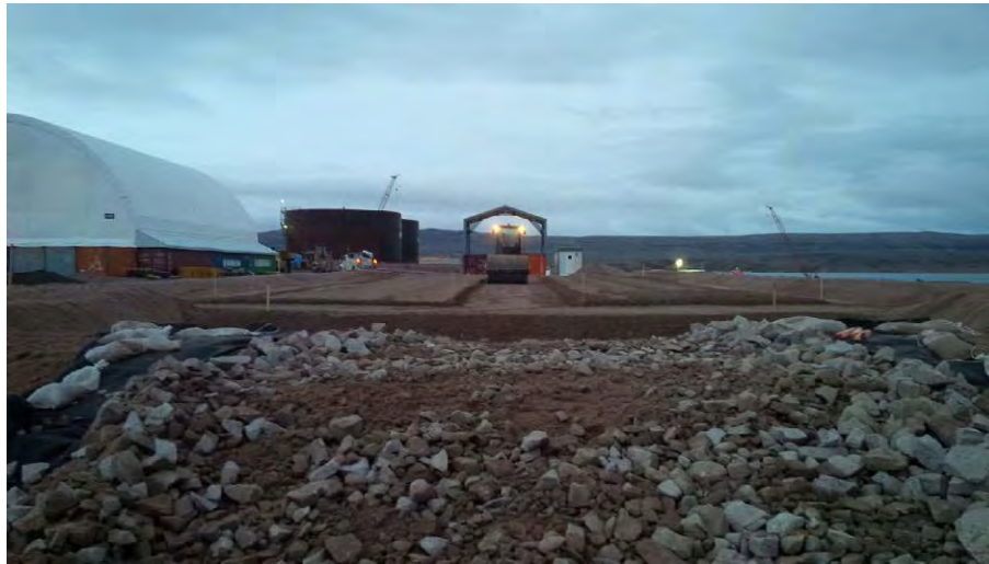
Figure 15: North hazardous waste containment area: Shaping the container pad earthworks [west view]
