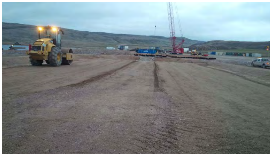
Figure 14: North hazardous waste containment area: Shaping the container pad earthworks (facing east) [west view]
