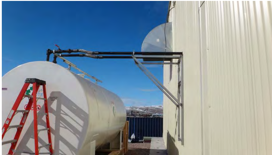
Figure 7: Waste Management Building: Incinerator fuel day tank installation
