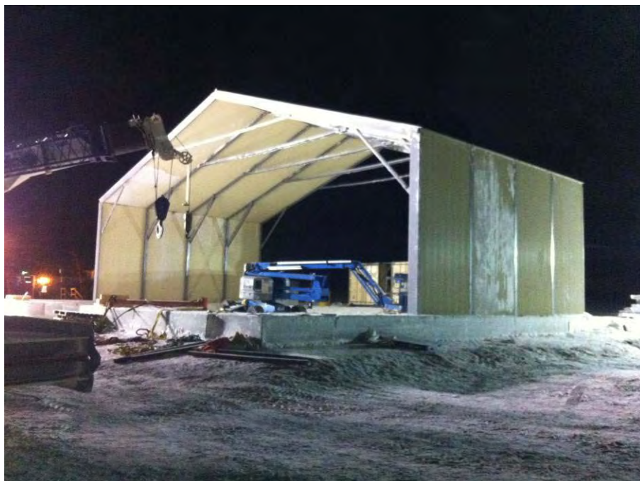
Figure 5: Waste Management Building: Erecting the fold away building
