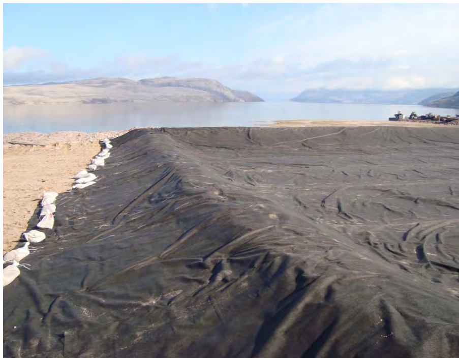
Figure 12: North hazardous waste containment area: placing liner [north view]
