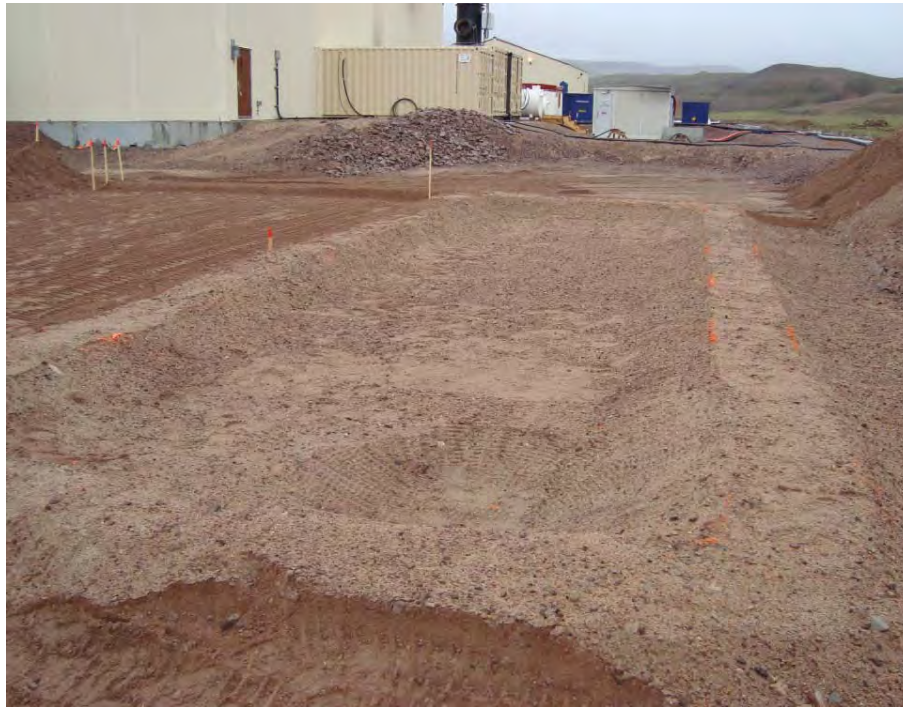
Figure 17: South hazardous containment area: Sub-base complete
