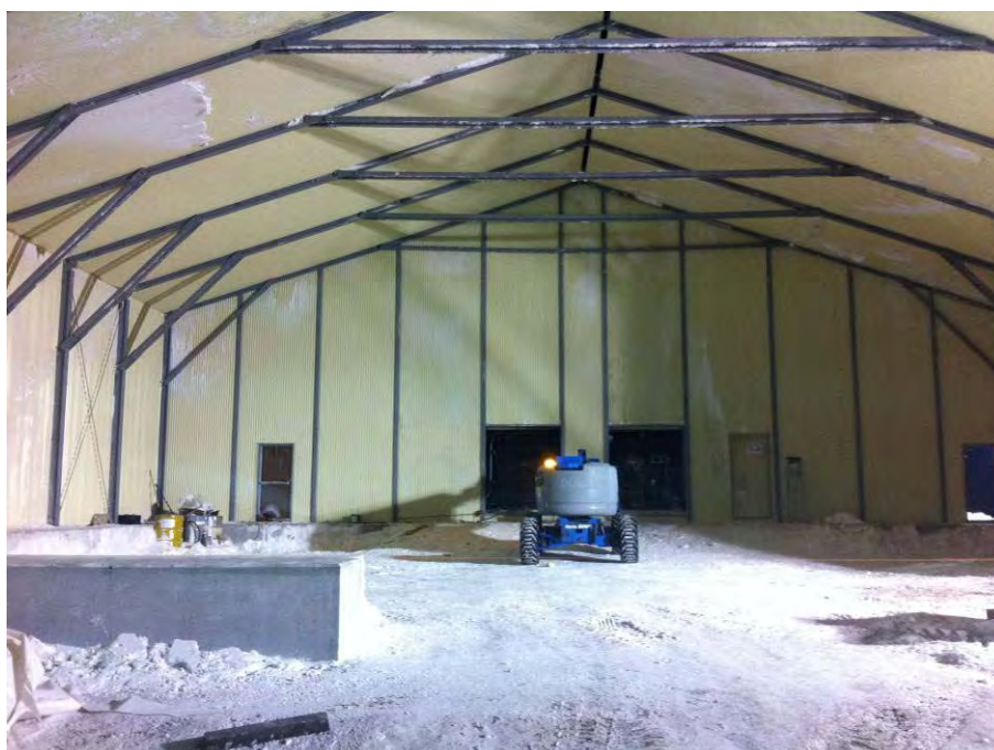
Figure 6: Waste Management Building: Installing the end walls (incinerator access ports on rear wall)
