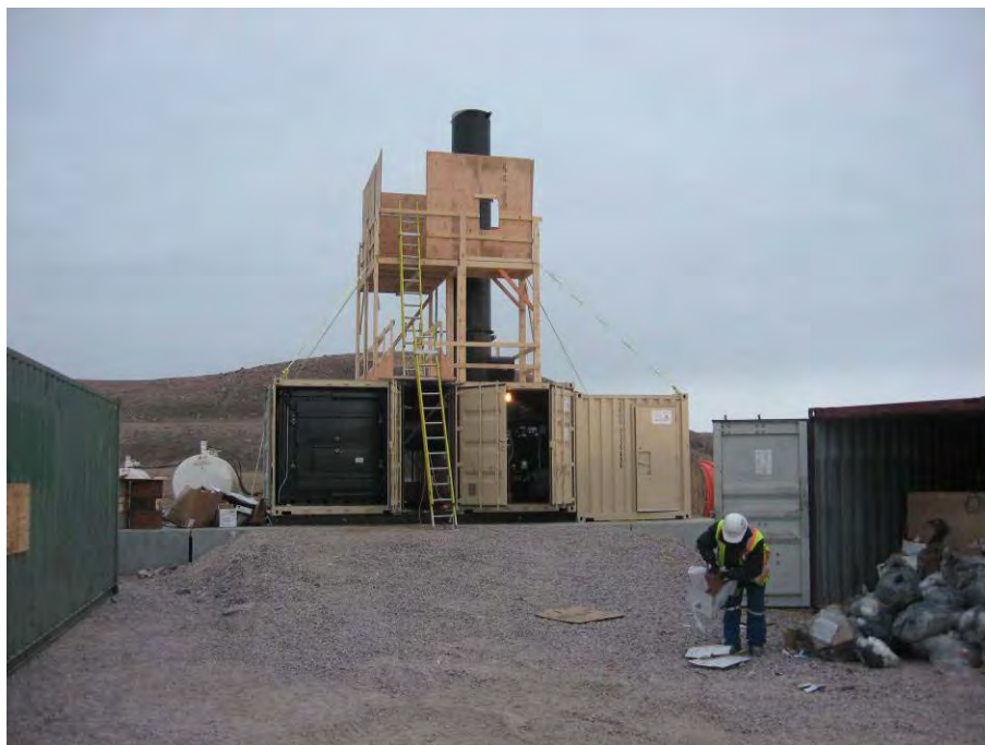
Figure 4: Waste Management Building: Installation of the incinerator equipment with temporary access platform for stack emissions testing
