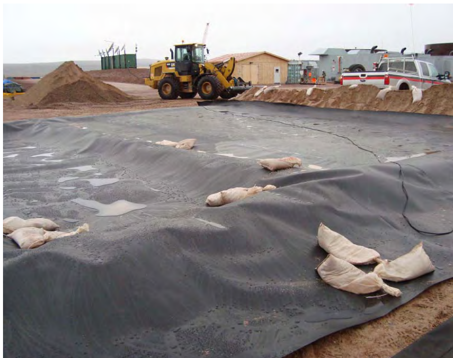
Figure 18: South hazardous containment area: Liner installation
