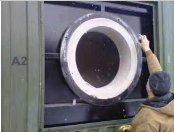
Gasket adhesive spray being applied
