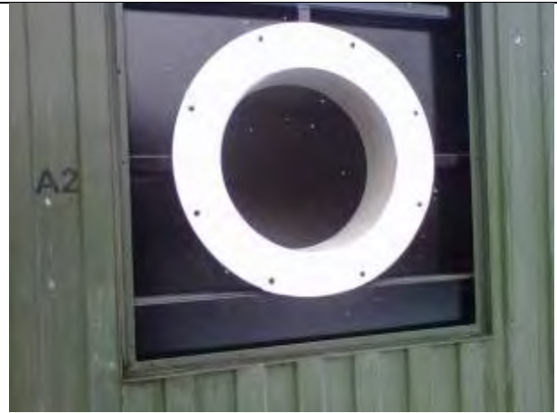
Correctly Installed Gasket
