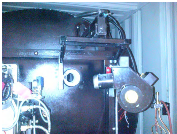
Swing the burner open
