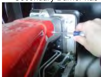
Secondary Burner has 4 screws (2 on each side)
