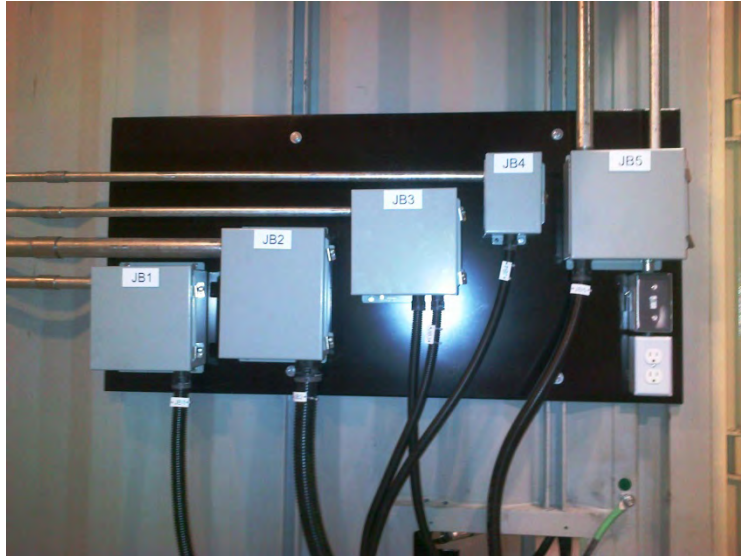
Junction Boxes in container 3 (control container)
