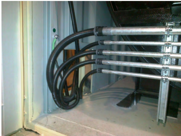
Flexible conduit in Container 2 (secondary chamber)
