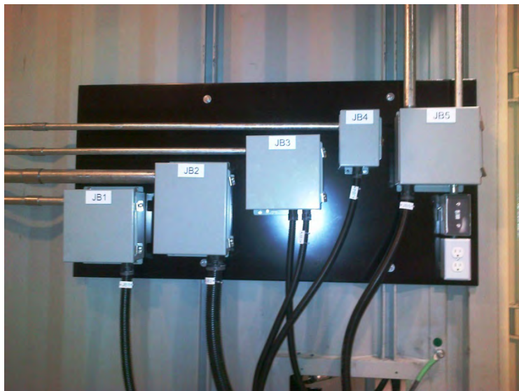
Junction Boxes in container 3 (control container)
