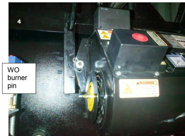
Waste oil burner secured with pin
