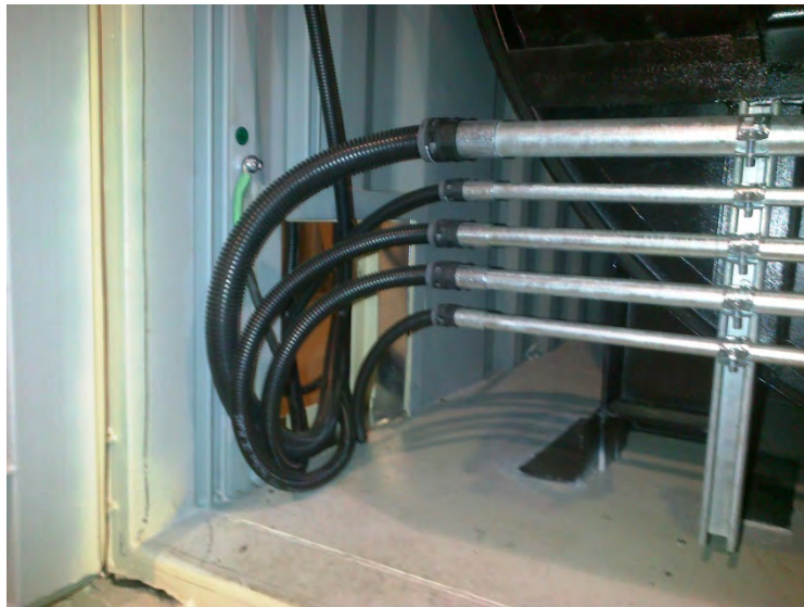
Flexible conduit in Container 2 (secondary chamber)
