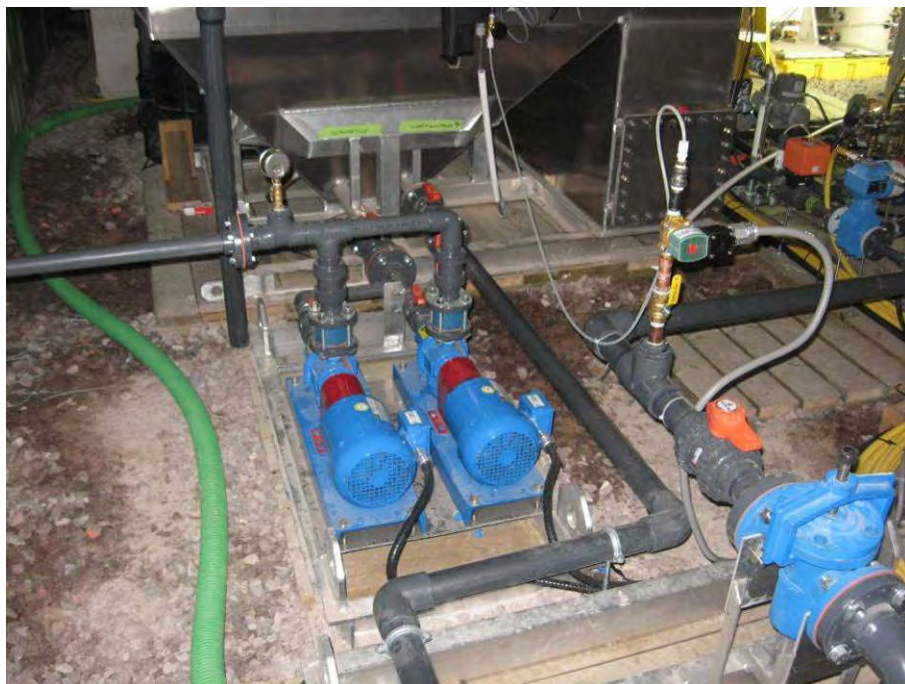
Figure 5: Water system – water treatment pumps and clarifier
