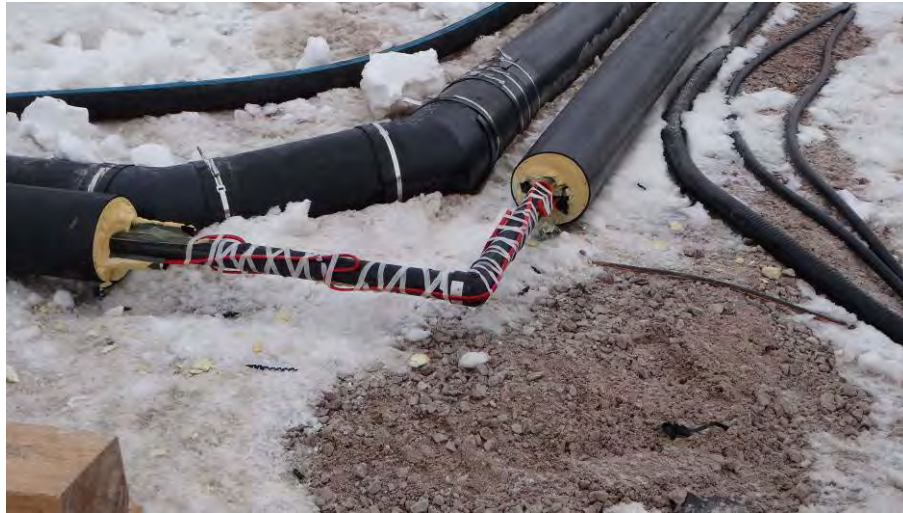
Figure 18: Installation of heat trace lines along an elbow of treated effluent discharge piping
