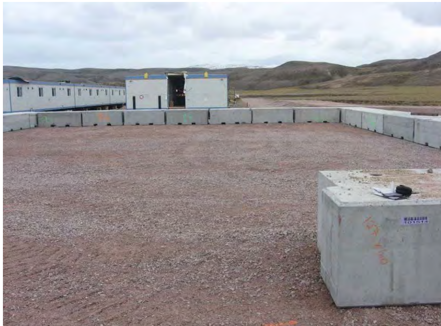
Figure 2: Water building pad and pre-cast concrete foundation blocks
