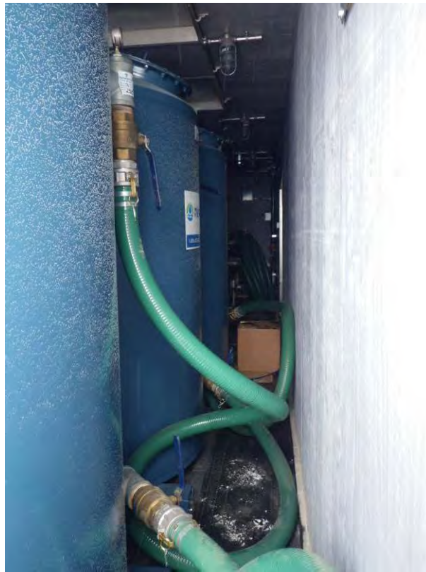
Figure 16: Treated effluent tanks inside the sewage treatment facility
