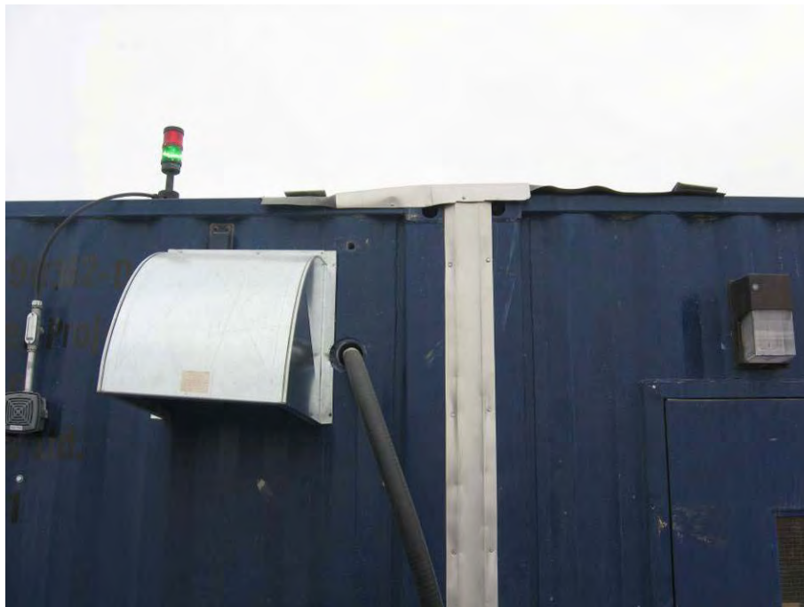
Figure 13: Weather sealing of connection joint between two of the six sea containers that combined are the sewage treatment building
