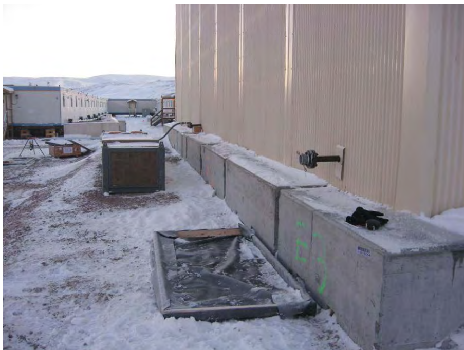
Figure 11: Water building - water truck connection
