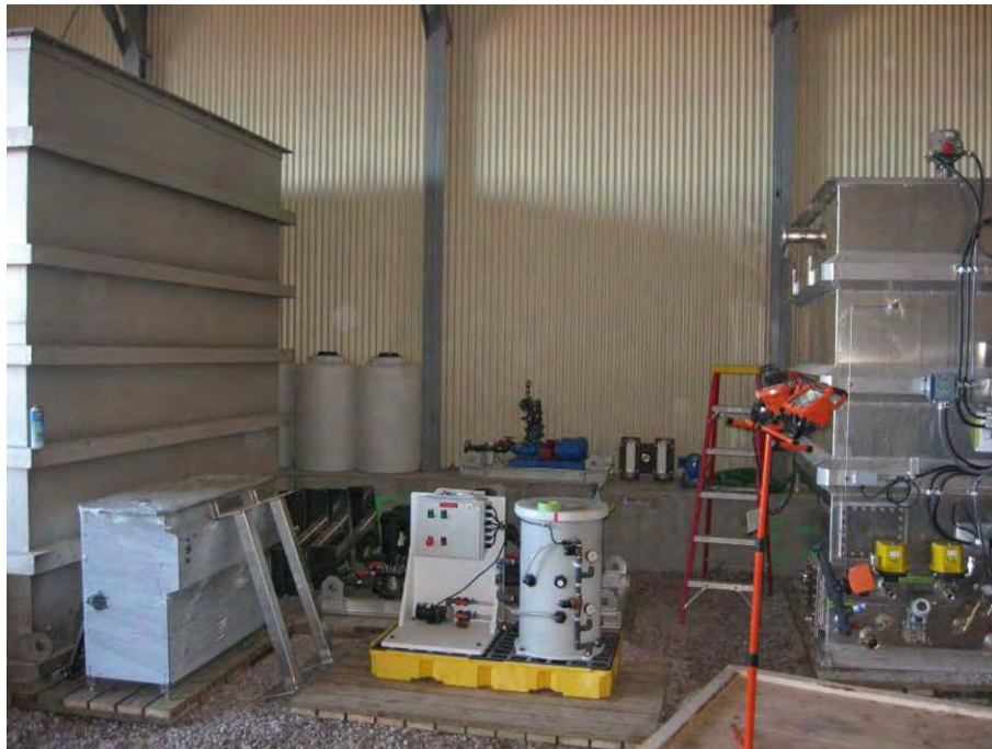
Figure 4: Water system – raw water tank, chlorine dosing system and clarifier
