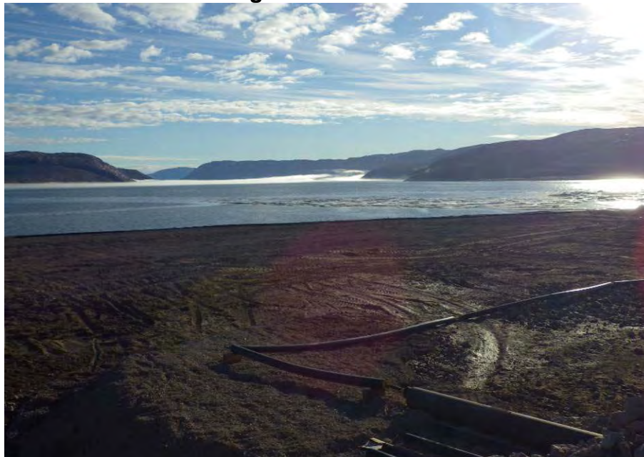
Figure 17: Treated effluent discharge piping laid out for fusing [north view]
