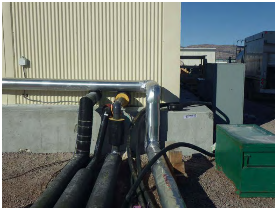
Figure 9: Piping out of the water building (to accommodation facilities, to sewage treatment, and for firewater)
