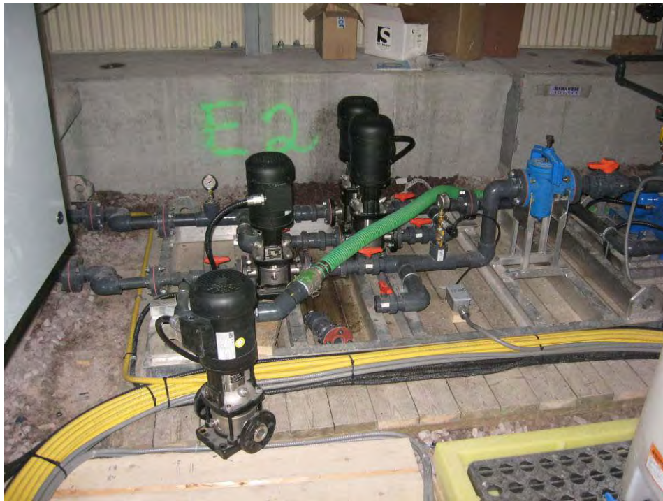
Figure 8: Water system – water treatment pumps
