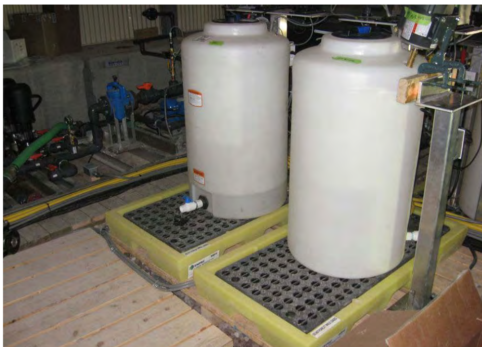
Figure 7: Water system – chemical mixing / dosing tanks
