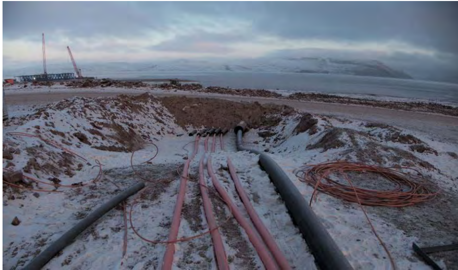
Figure 20: Road crossing with cables and piping routing through schedule 80 pipe sleeves for protection
