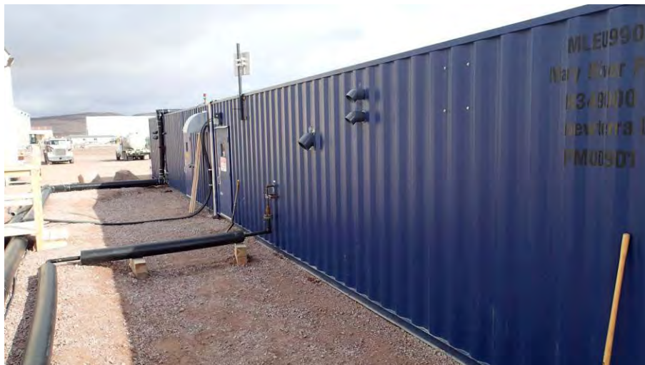
Figure 15: Installation of interconnecting piping to and from the sewage treatment building
