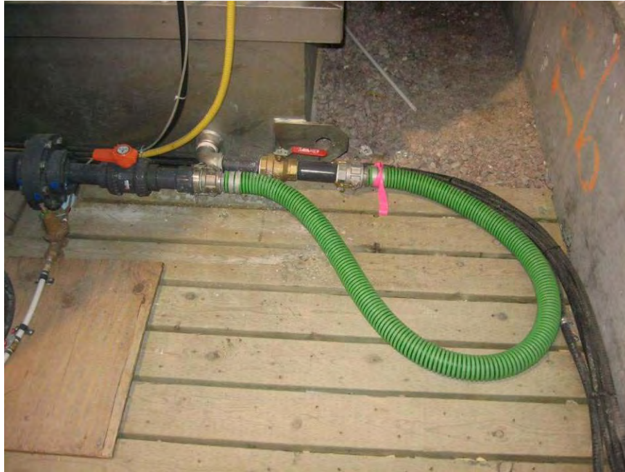
Figure 22: Location of cracked pipe in Milne Port Water Building, fixed infield with flexible hose connection as shown [27Apr2014].
