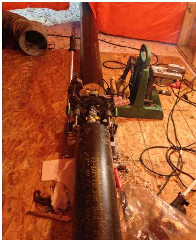
Figure 19: Preparing to fuse two HDPE piping lengths (activity enclosed in protective tenting to retain heat required for fusing)
