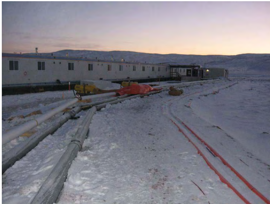
Figure 10: Piping between accommodation facilities, water treatment plant, and sewage treatment facility [northeast view]
