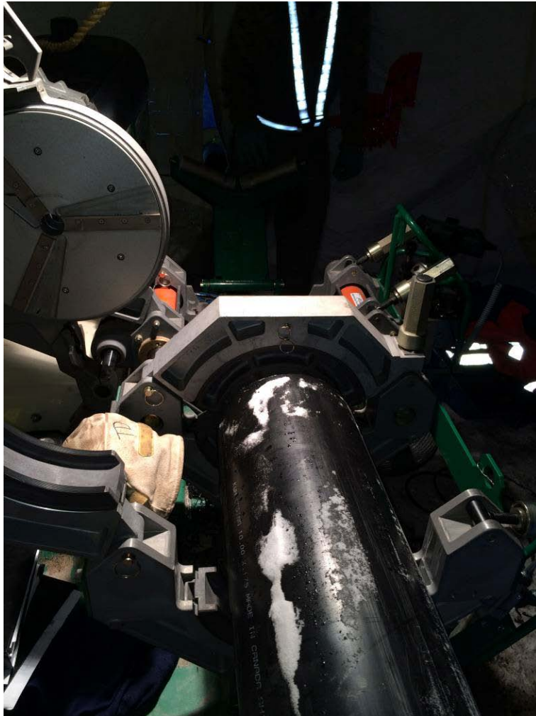
Figure 28: Preparing to fuse two HDPE piping lengths (activity enclosed in protective tenting)
