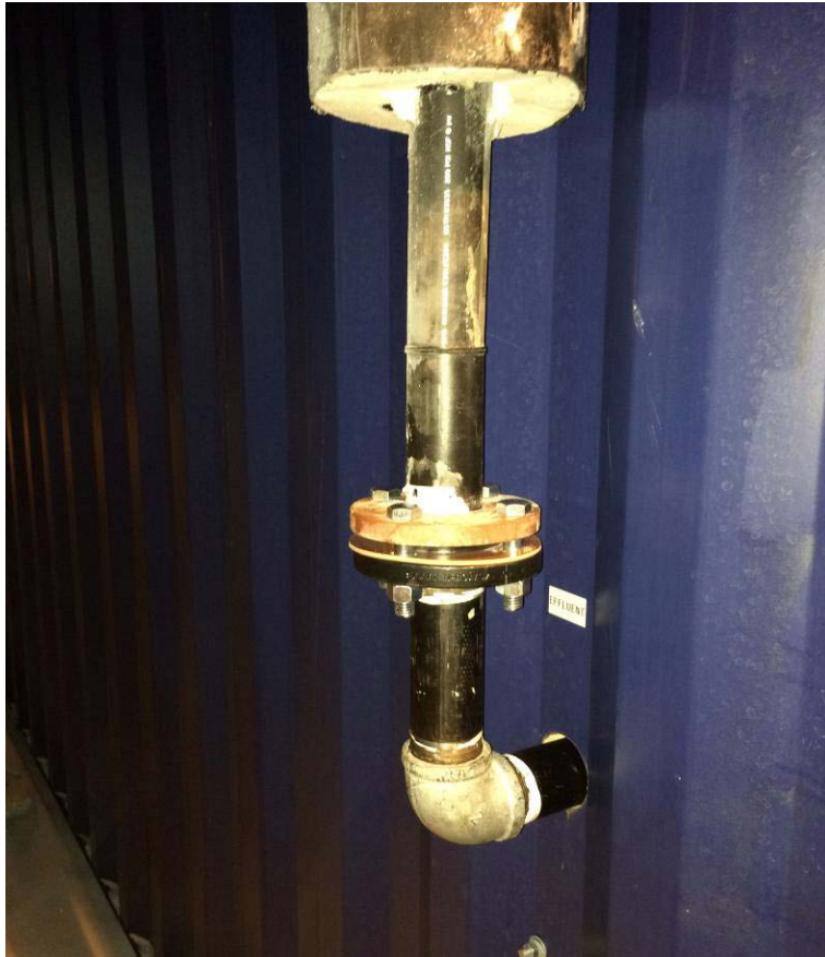
Figure 25: Treated effluent discharge connection on north side of sewage treatment plant
