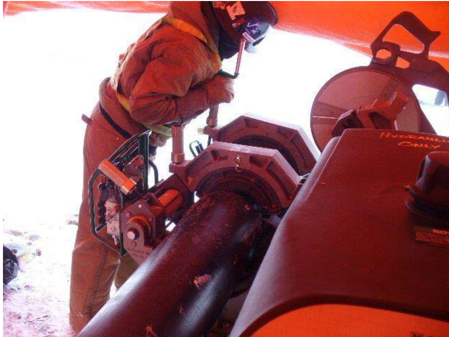
Figure 13: Pipe fusing inside the tent shelter (activity enclosed in protective tenting to retain heat required for fusing)
