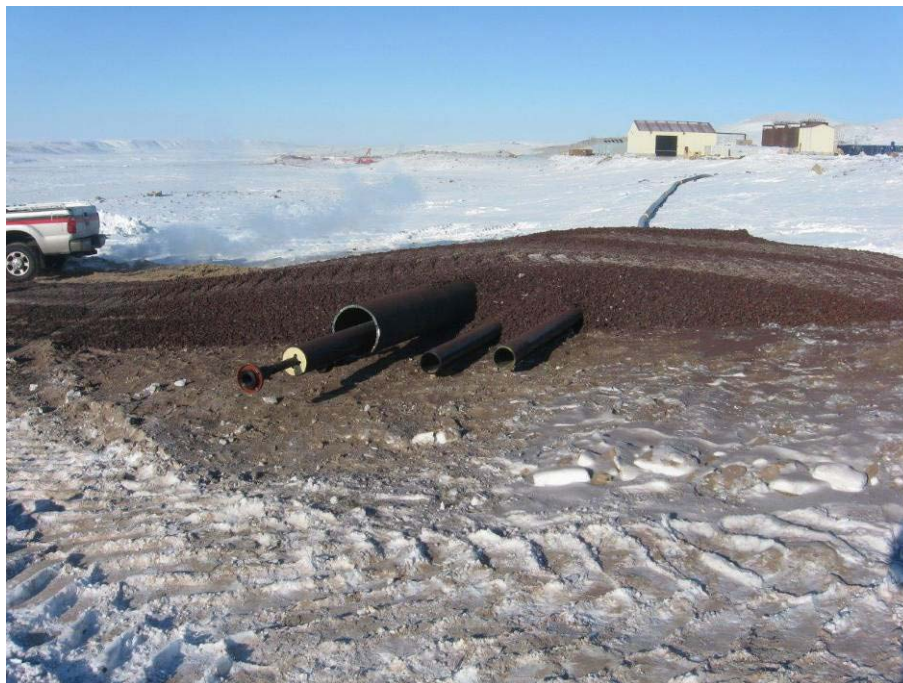
Figure 30: Treated effluent discharge road crossing construction
