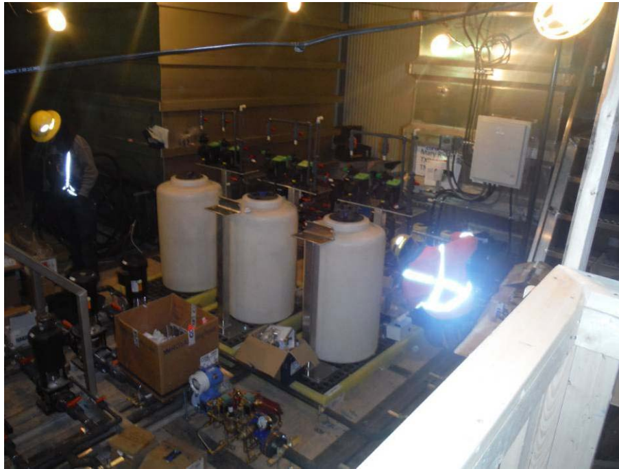
Figure 20: Installation of skid mounted tanks, piping, valving and equipment
