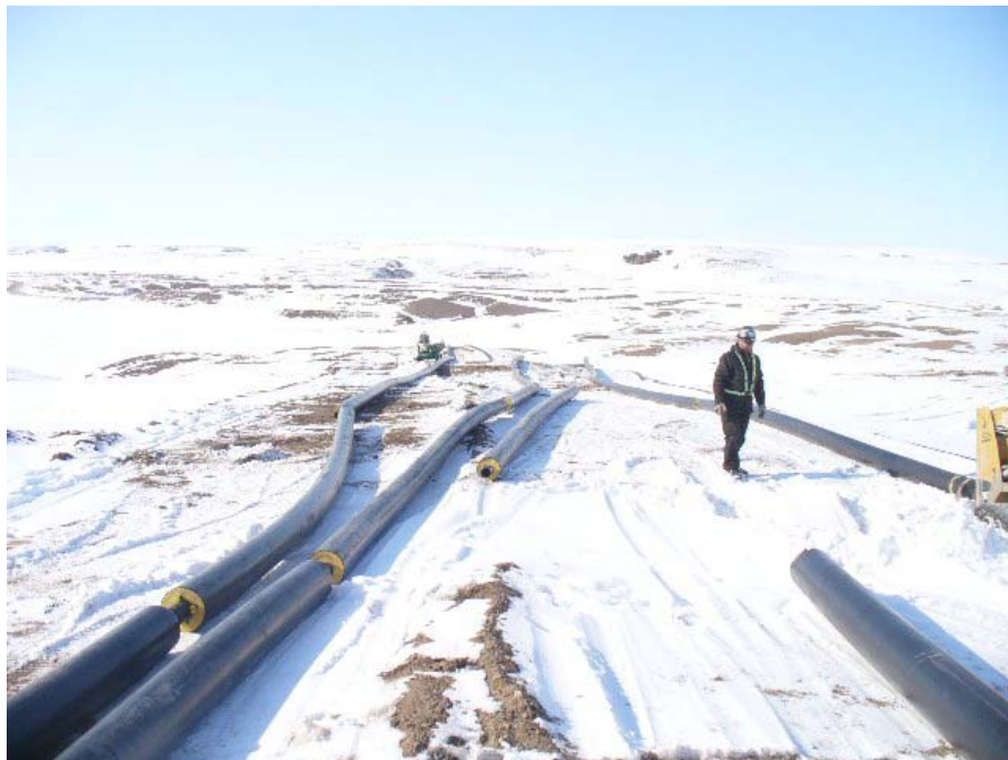
Figure 8: Laying out the piping lengths
