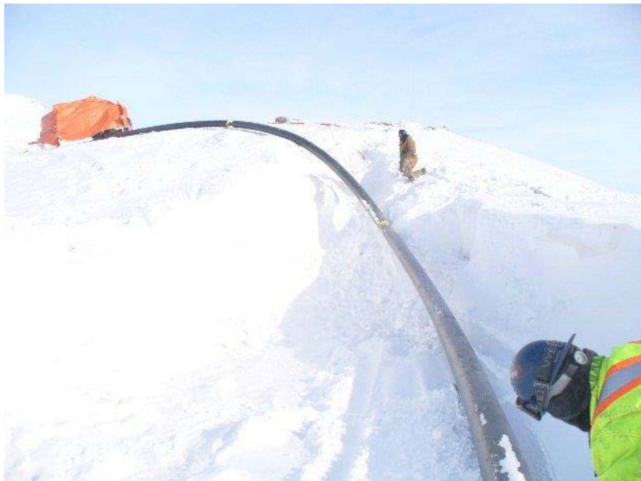
Figure 12: Laying out the piping route (tent shelter for pipe fusing activities in back left)
