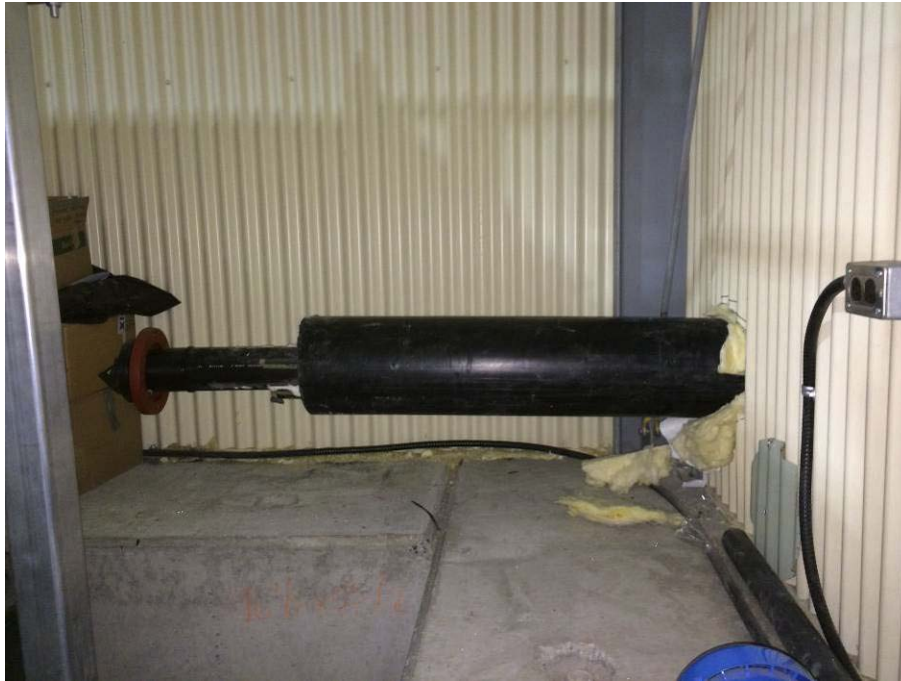
Figure 16: Raw water pipeline entering the water building
