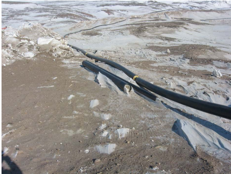
Figure 9: Raw water line "snaking" across the tundra
