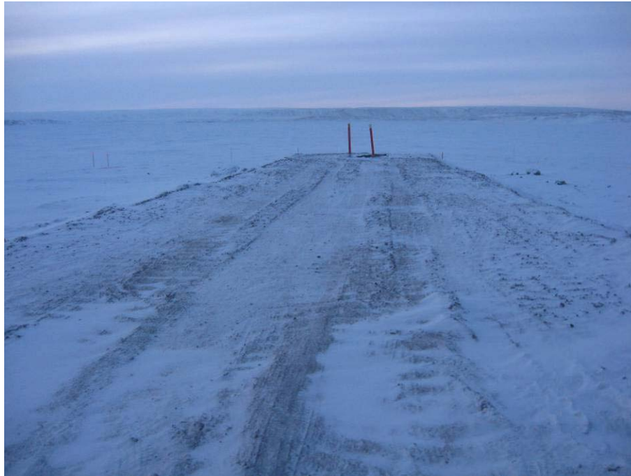
Figure 4: Raw water jetty earthworks complete [west view]
