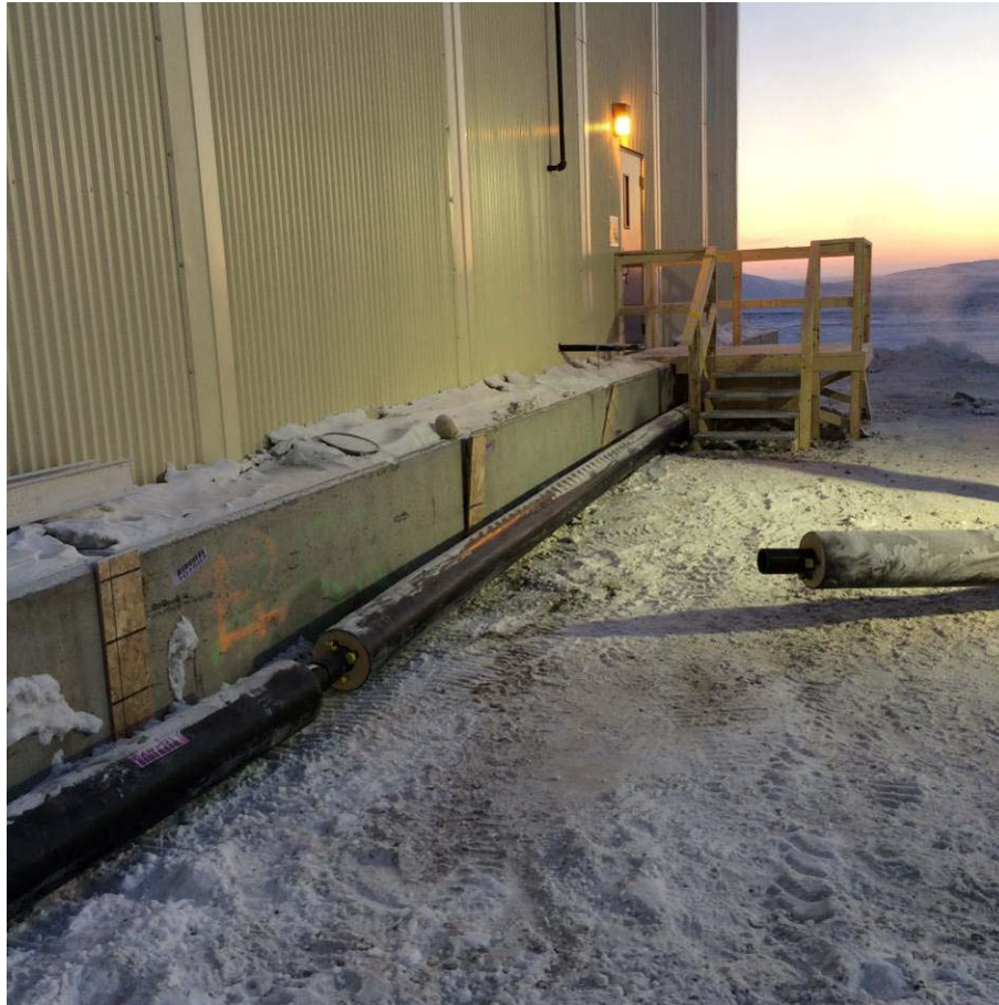
Figure 15: Raw water intake piping entering the water building
