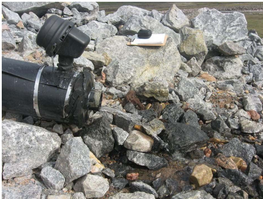
Figure 33: All-weather treated effluent discharge point over rip rap
