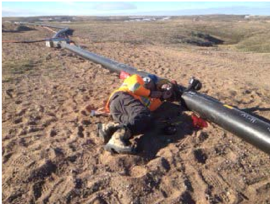
Figure 14: Testing of the finished line
