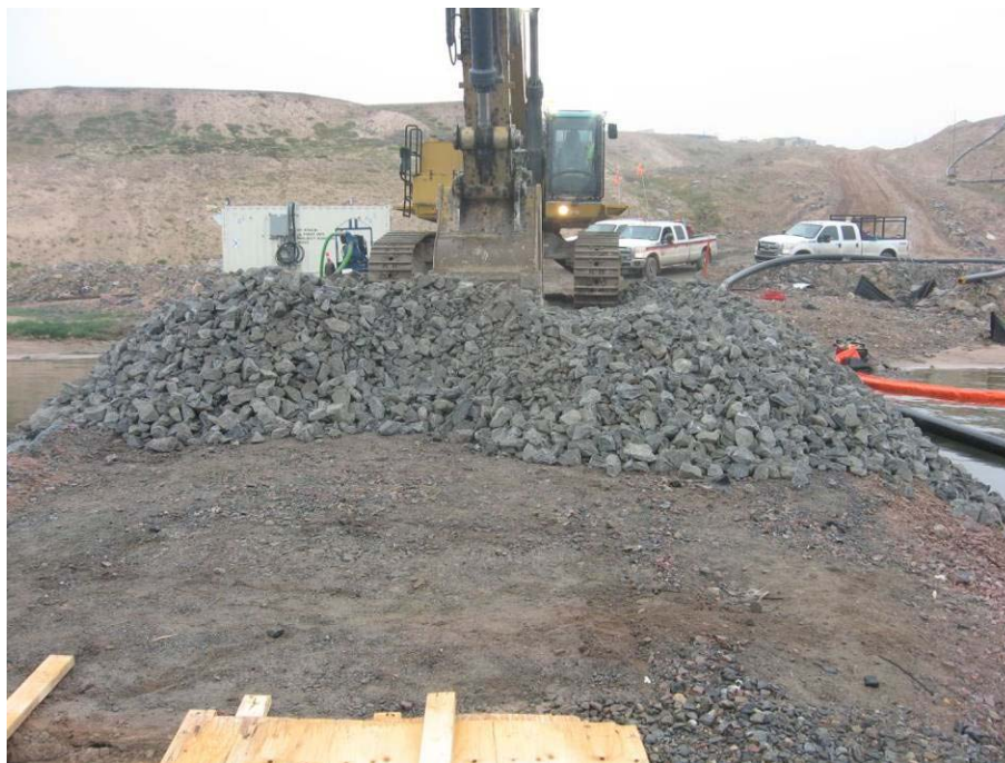
Figure 3: Installing armour stone at raw water jetty [east view]
