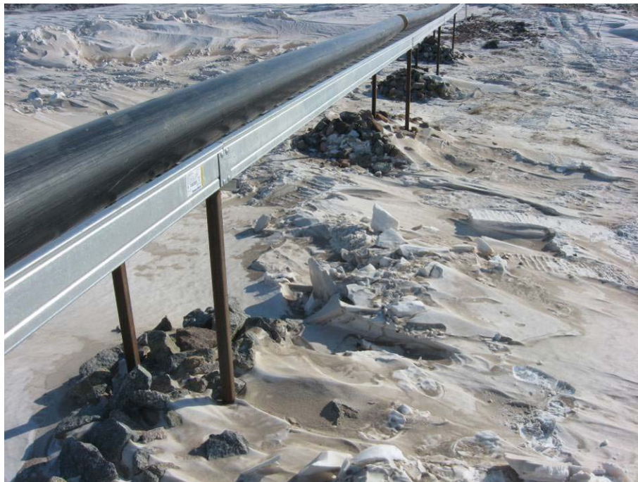
Figure 10: Raw water line raised to cross a low point
