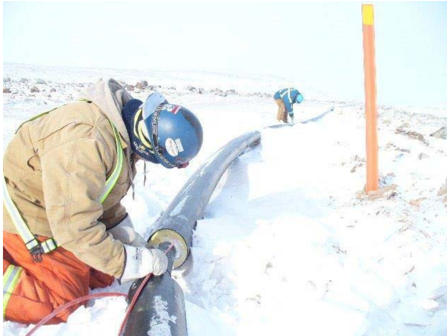
Figure 11: Feeding the heat trace cable through sleeve in the insulation
