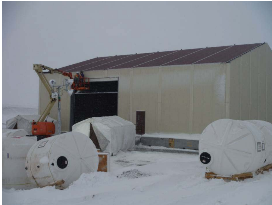
Figure 18: Preparing water building for water treatment equipment (fire water tanks shown outside)
