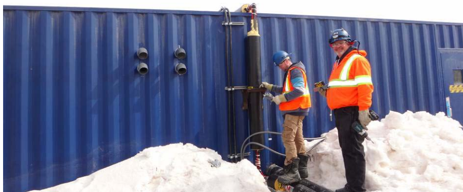
Figure 26: Installation of heat trace lines on treated effluent discharge piping
