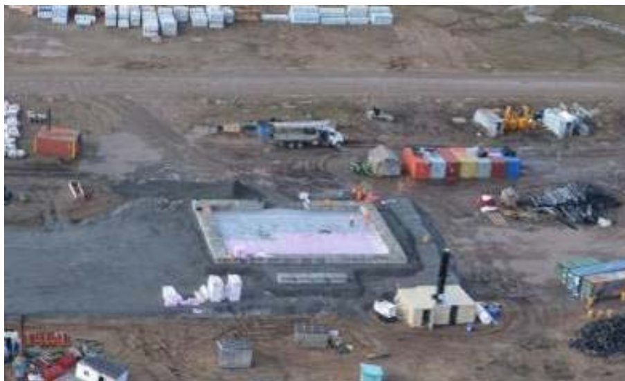
Figure 4: Waste Management Building: Slab on grade installation in progress. Incinerator temporary location north-west of foundation as shown until foundation complete [south view]
