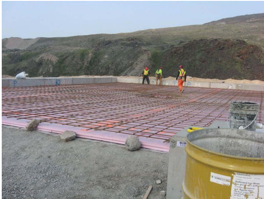
Figure 5: Waste Management Building: Laying the insulation and rebar within the boundaries of the pre-cast foundation blocks, ready to pour the concrete slab on grade [north view]
