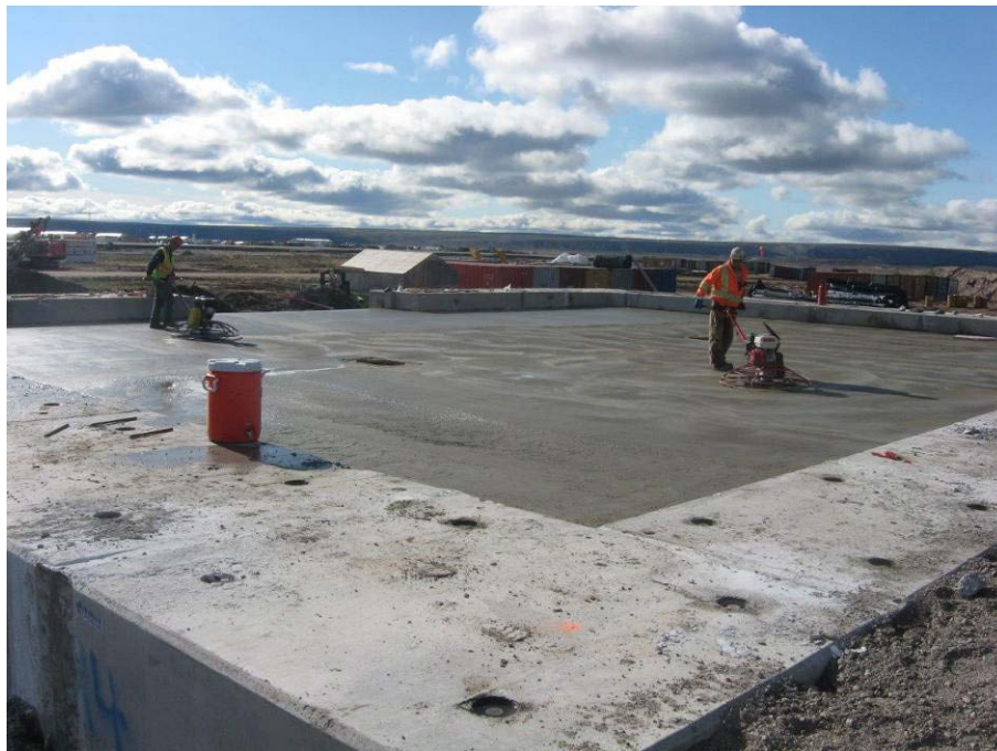
Figure 6: Waste Management Building: Steel trowel finishing the concrete pad in the boundaries of the pre-cast foundation blocks [southwest view]
