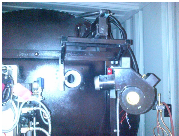
Swing the burner open
