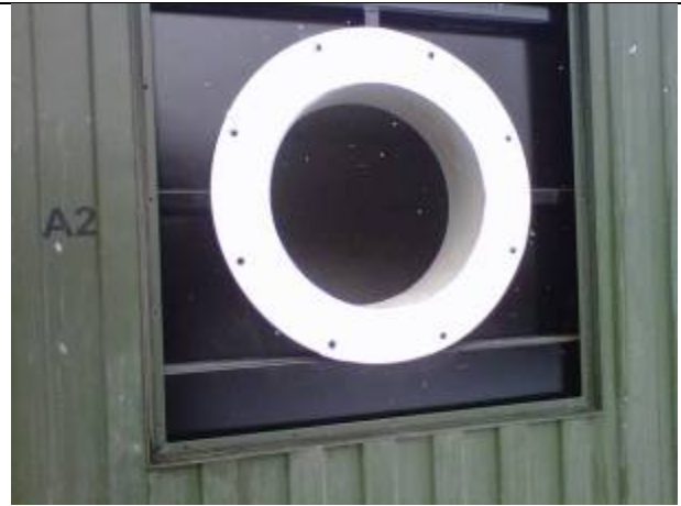
Correctly Installed Gasket
