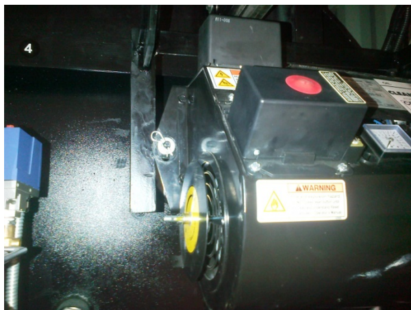
With the burner all the way out remove pin
