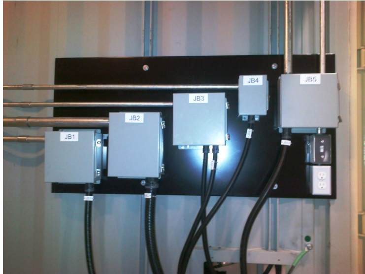
Junction Boxes in container 3 (control container)
