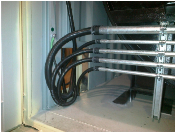
Flexible conduit in Container 2 (secondary chamber)
