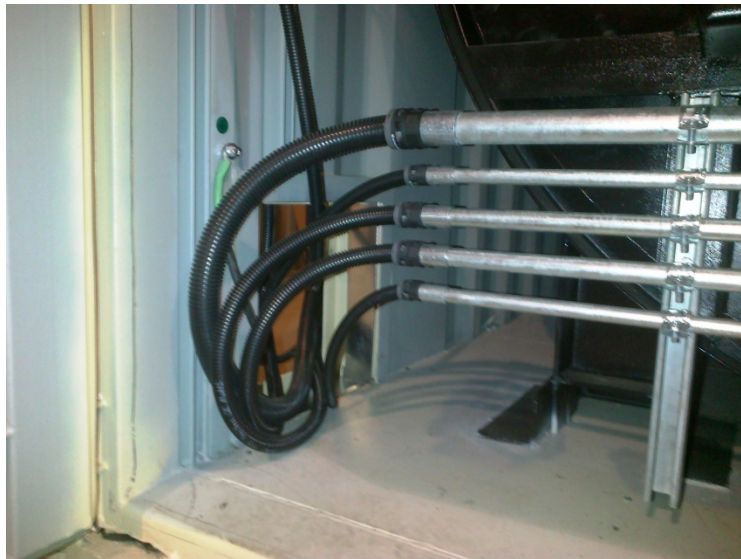
Flexible conduit in Container 2 (secondary chamber)
