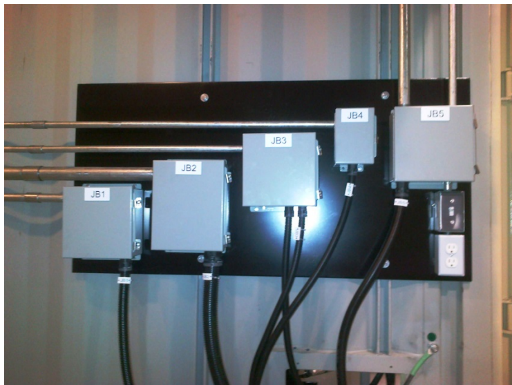
Junction Boxes in container 3 (control container)
