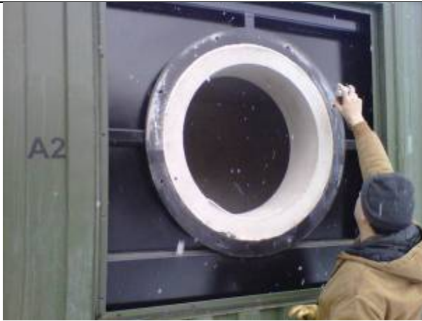
Gasket adhesive spray being applied
