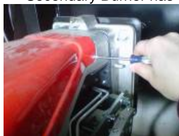
Secondary Burner has 4 screws (2 on each side)
