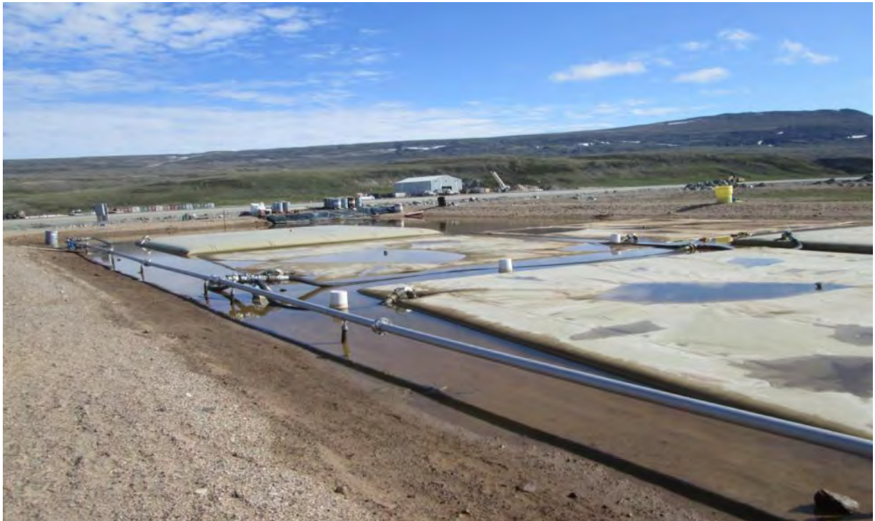
Bulk Fuel Storage Containment.
