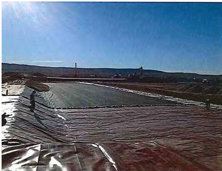
Figure 5: Installation of liner
