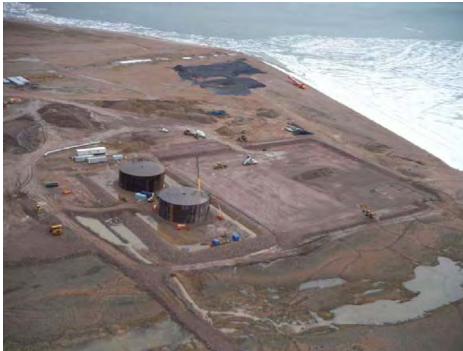
Figure 4: Preparation for liner installation [northwest view]
