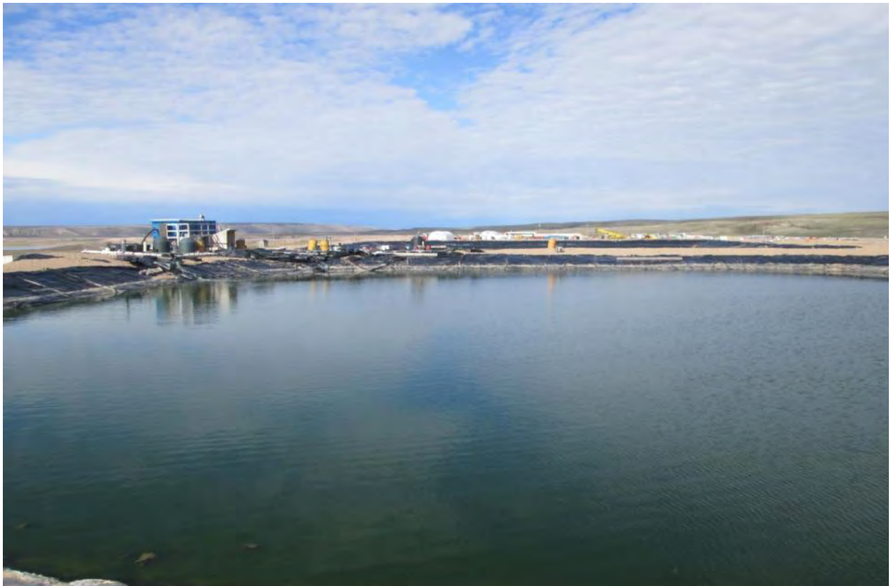
Polishing/Waste Stabilization Ponds #2 and #3.
