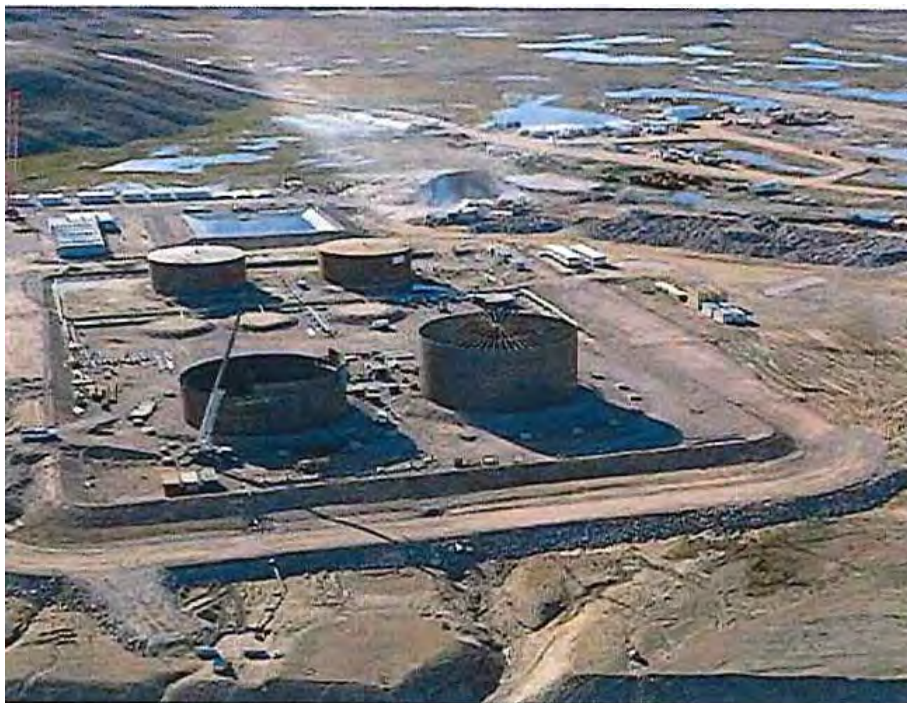
Figure 8: Containment earthworks completed [south view]
