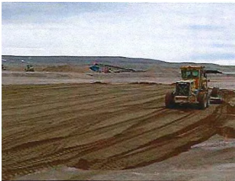
Figure 3: Placement of sand layer below liner
