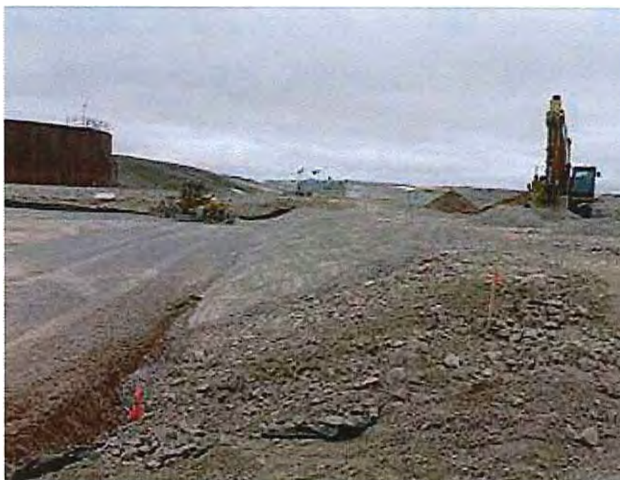
Figure 7: Berm construction
