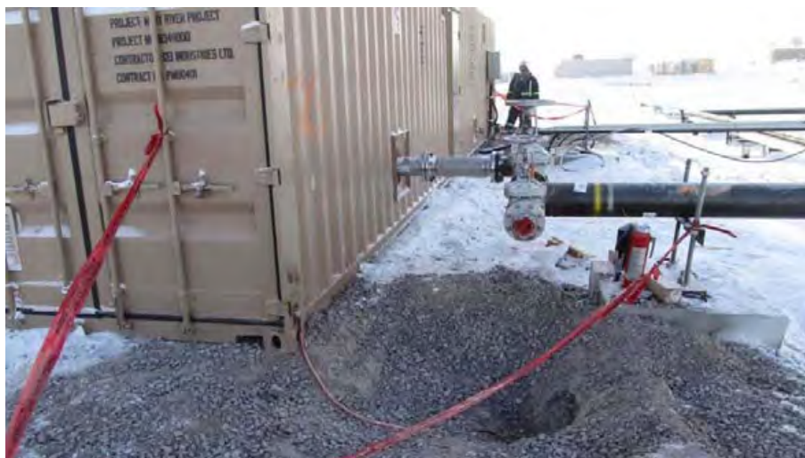
Figure 12: Dispensing module inlet piping from tanks
