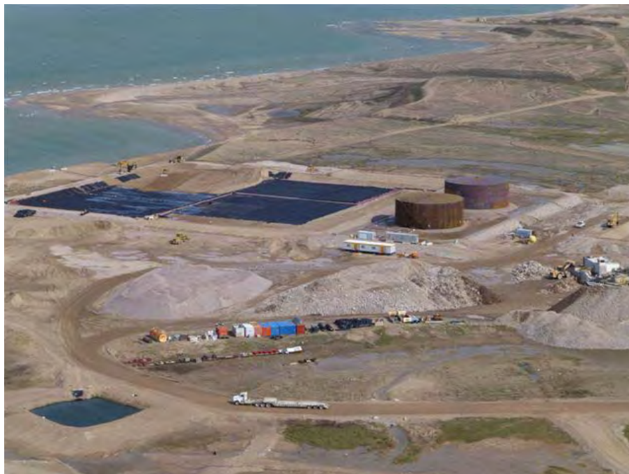
Figure 6: Liner installation in-progress [northeast view]
