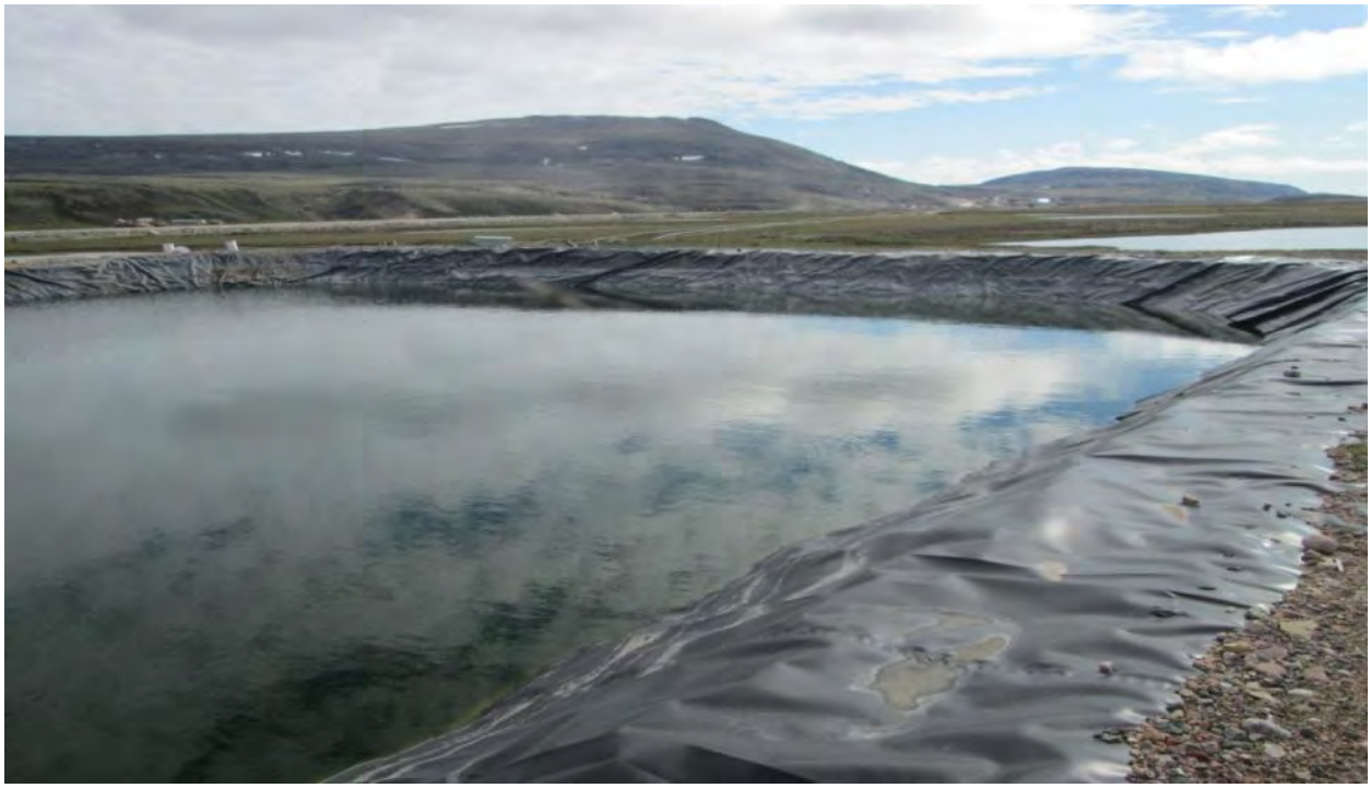
Polishing/Waste Stabilization Pond #1.
