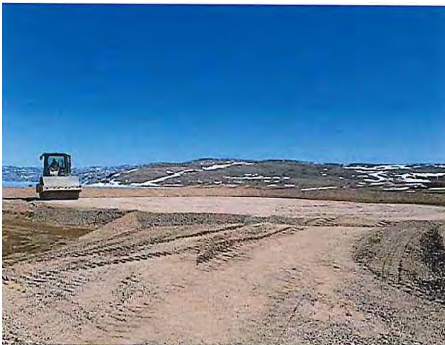
Figure 2: Preparation of sub-base
