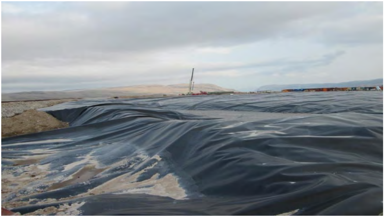
Photo taken looking north at the covered contaminated granular from the bulk fuel storage facility undergoing decommissioning.
