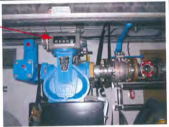
Tanker truck fuel meter
