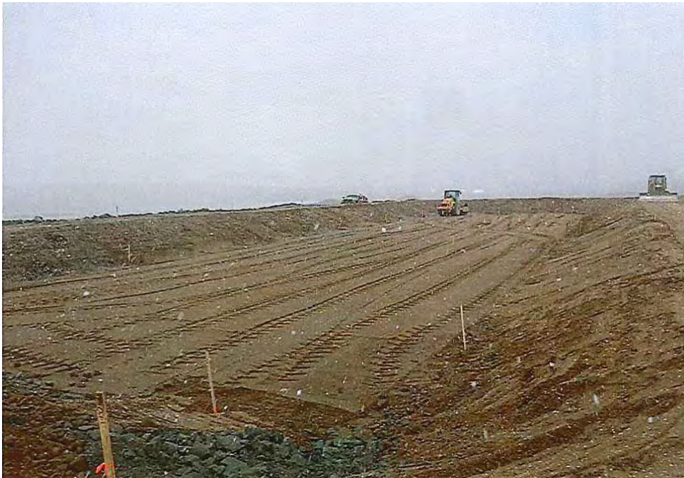
Figure 4: Compaction of sand layer
