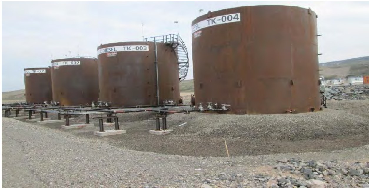
Minesite Steel Fuel Tank Farm Containment
