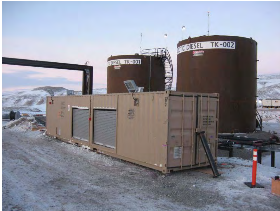
Figure 11: Fuel dispensing module and overhead piping tray
