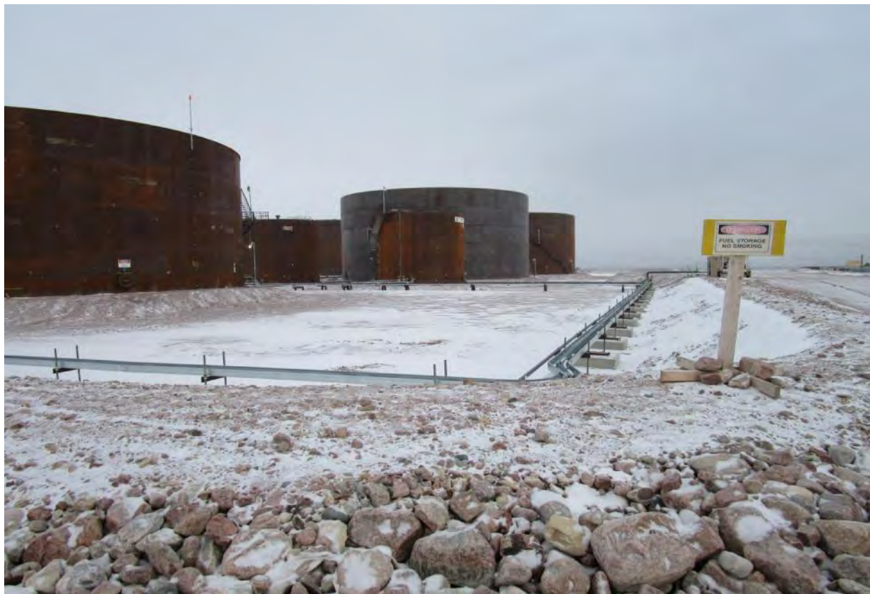
Fuel tank farm containment
