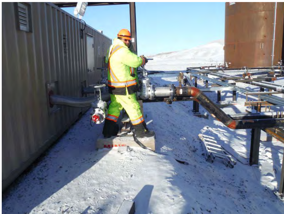
Figure 12: Valves and piping between tanks and dispensing module (at dispensing module)
