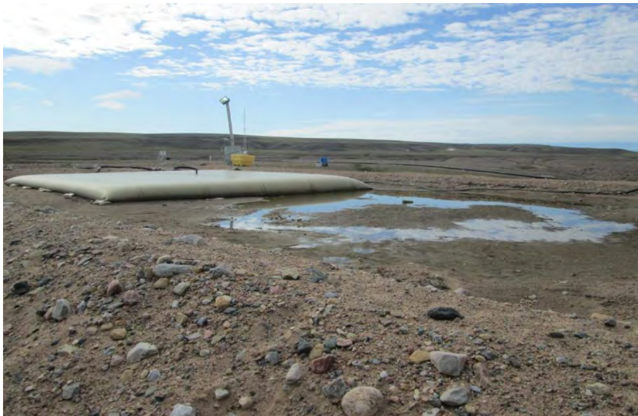
Generator Fuel Storage Facility Containment
