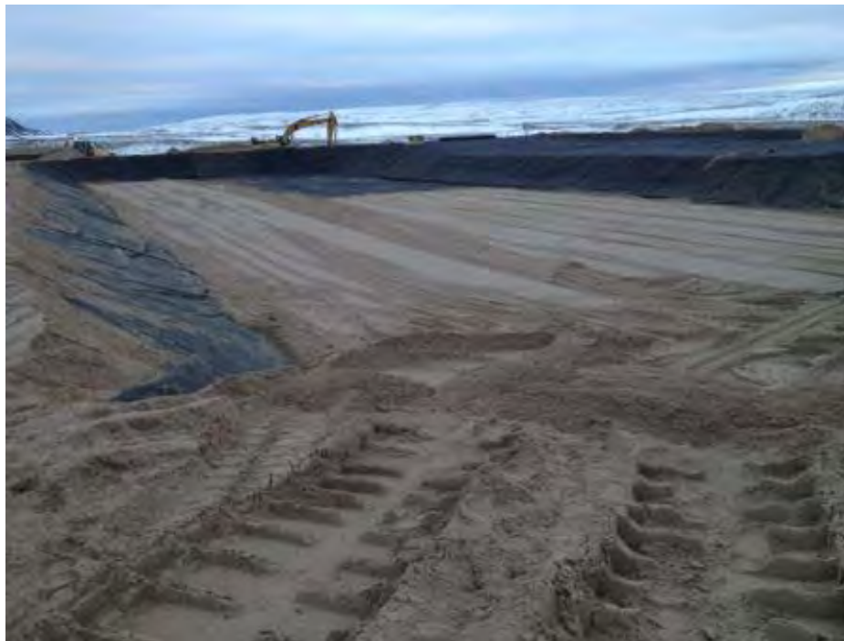
Figure 8: Installation of cover material over liner
