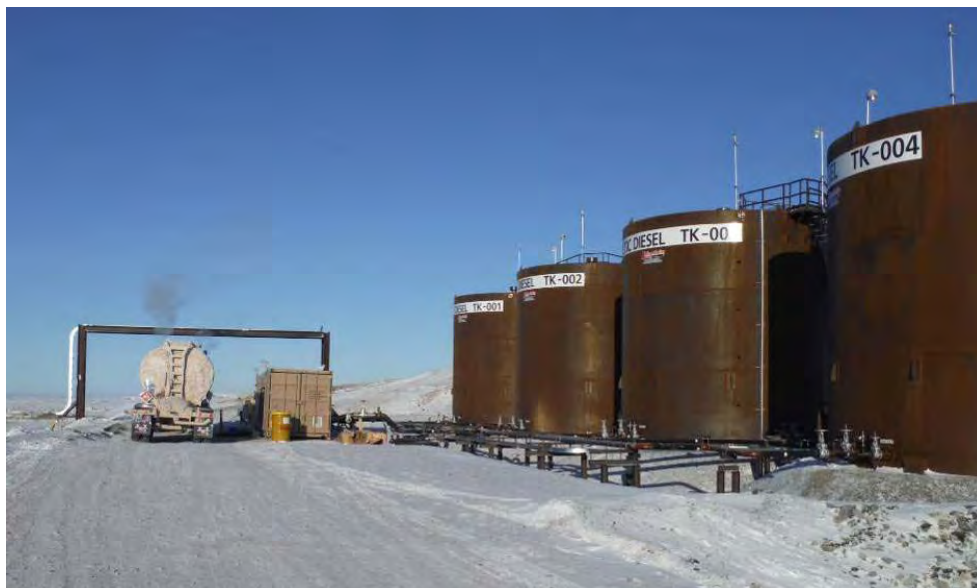
Figure 13: Tanks, piping, dispensing module, and overhead piping tray [northwest view]
