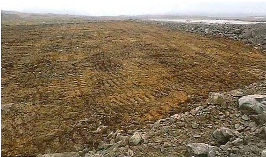
Figure 2: Graded sub-base
