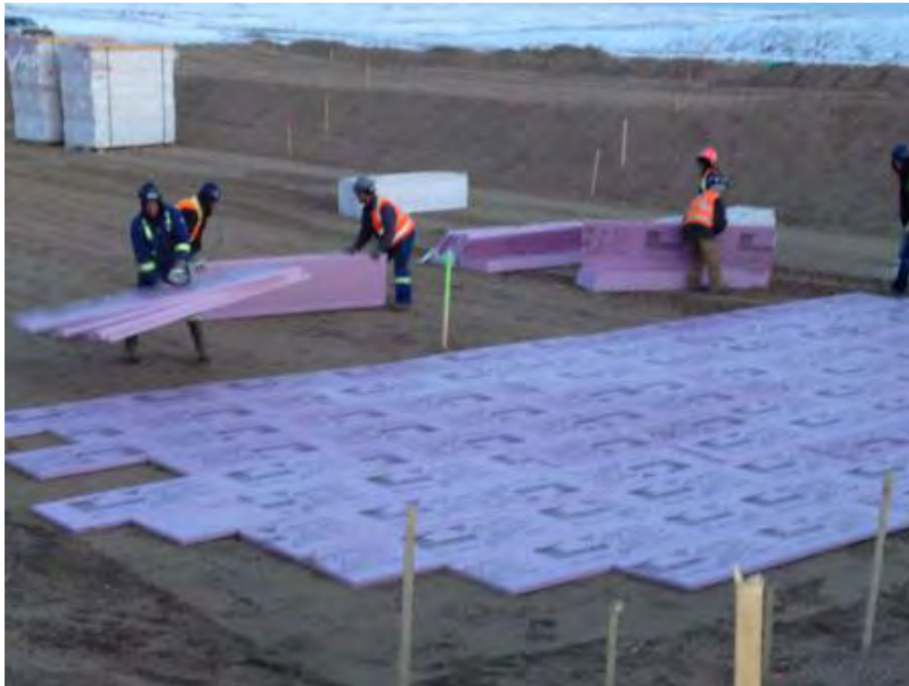
Figure 5: Installation of insulation layer
