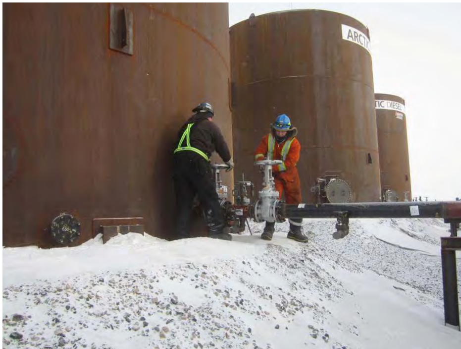
Figure 10: Valves and piping between tanks and dispensing module (at tanks)
