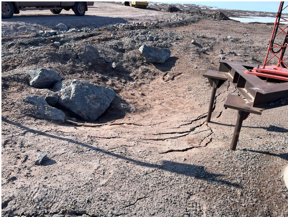
Photo 4 Subsidence north of the access road and adjacent airstrip lighting
