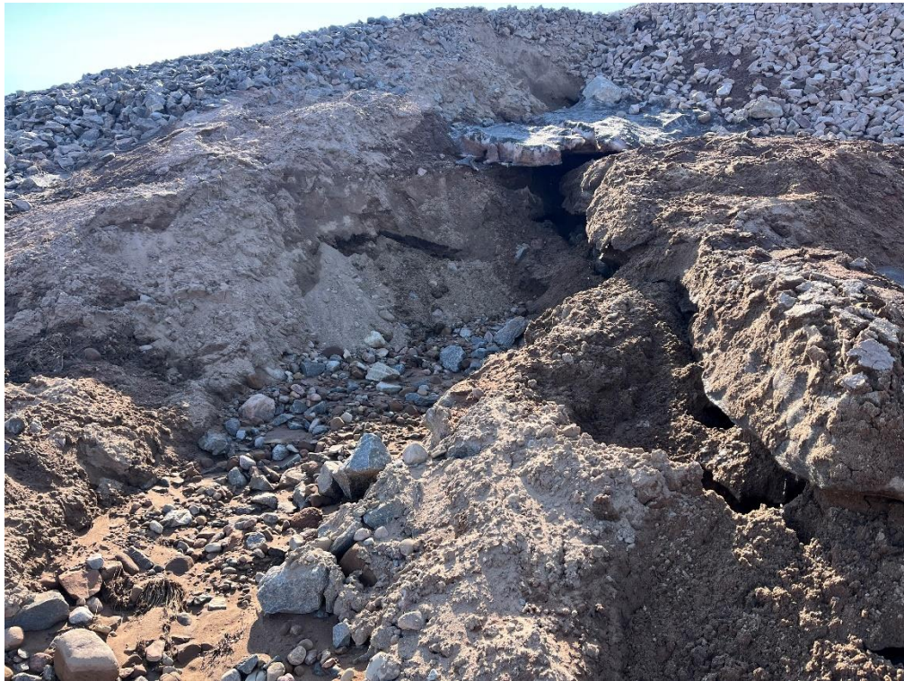
Photo 3 Eroded slope beneath the low area requiring drainage
