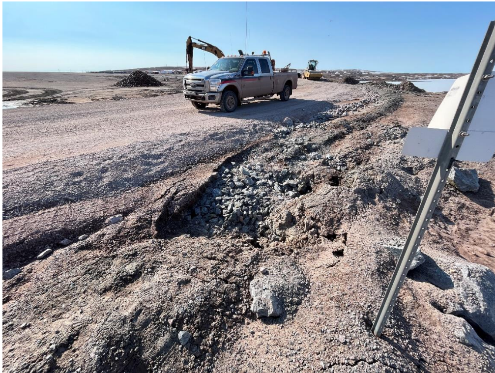
Photo 5 Subsidence north of the access road and adjacent airstrip lighting
