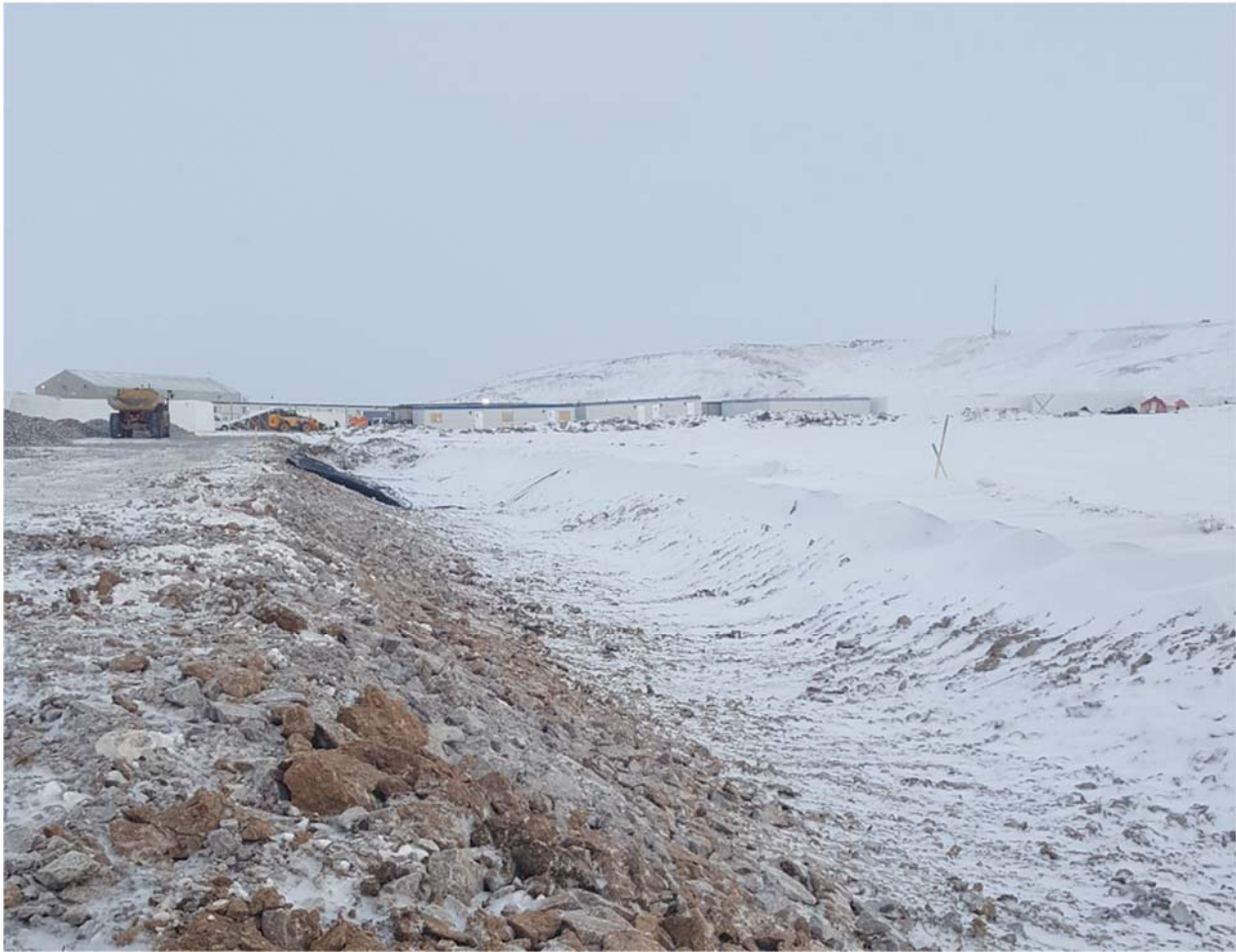
Figure 2: An overview of a completed section, in the background, the inlet plug can be seen to remain with riprap placement required and geotextile already installed.
