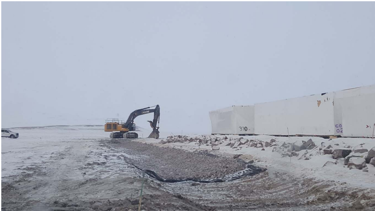
Figure 1: JD850 Excavator completing a segment of the ditch with geotextile and riprap placement. In the foreground, excavated ditch can be seen, which will be the next section for slope and grade final cut, along with geotextile and riprap placement.
