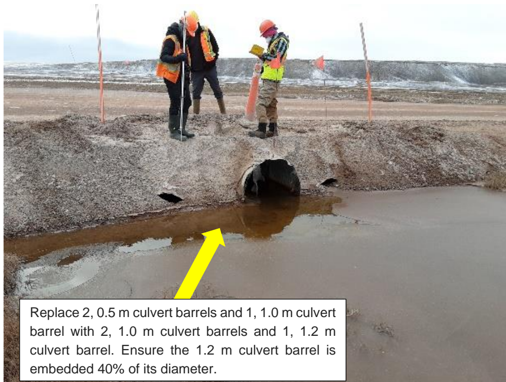
Photo B17.1 CV-001 Culvert Inlet
