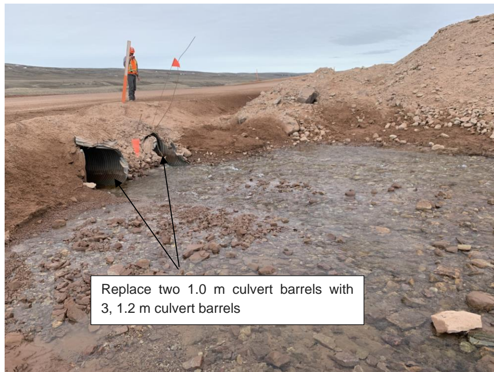
Photo B1.1 CV-114 Culvert Inlet
