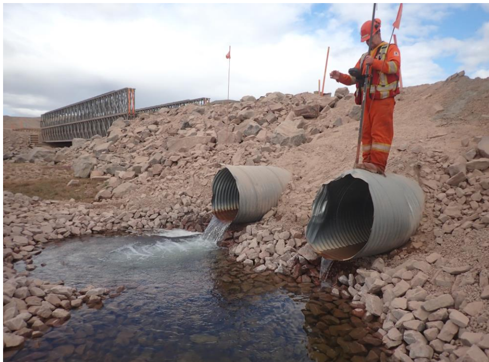
Photo B10.2 BG-50 Culvert Outlet
