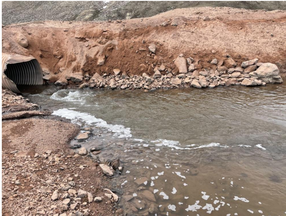
Photo B15.3 BG-17 Culvert Downstream Bank Erosion
