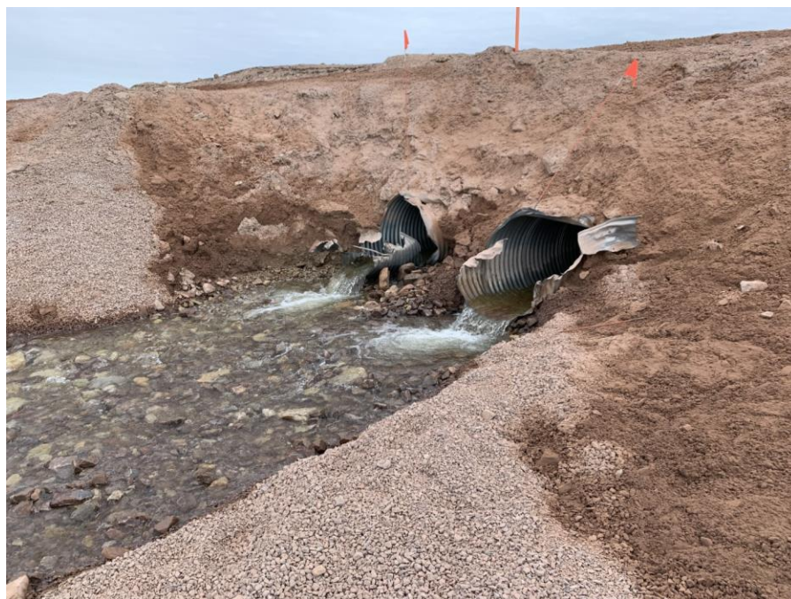
Photo B1.2 CV-114 Culvert Outlet
