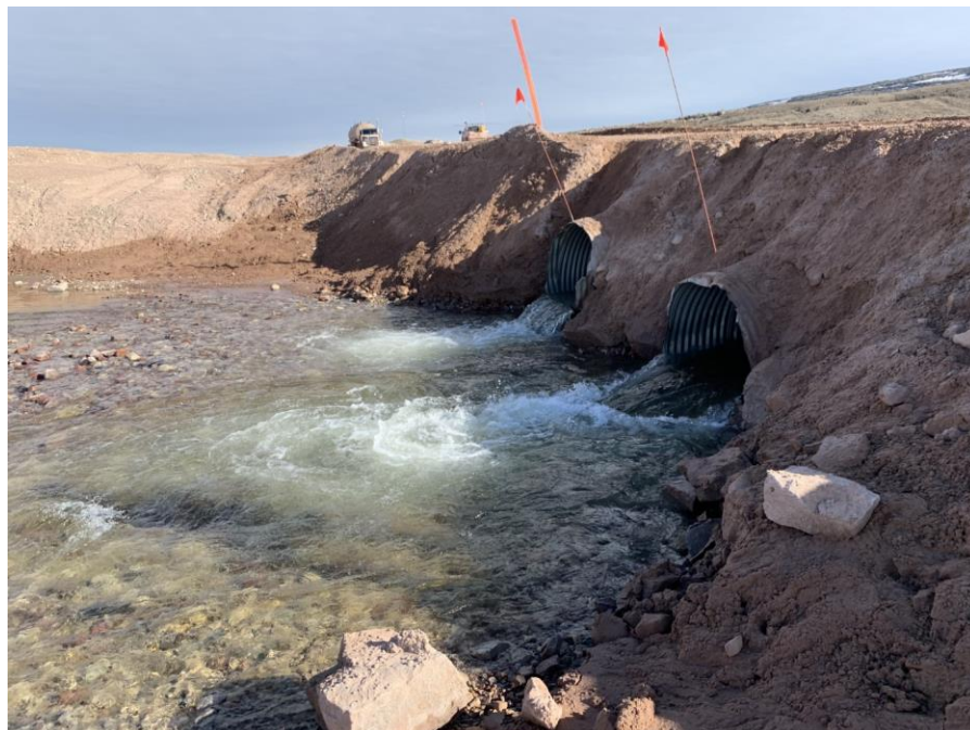
Photo B6.2 CV-079 Culvert Outlet
