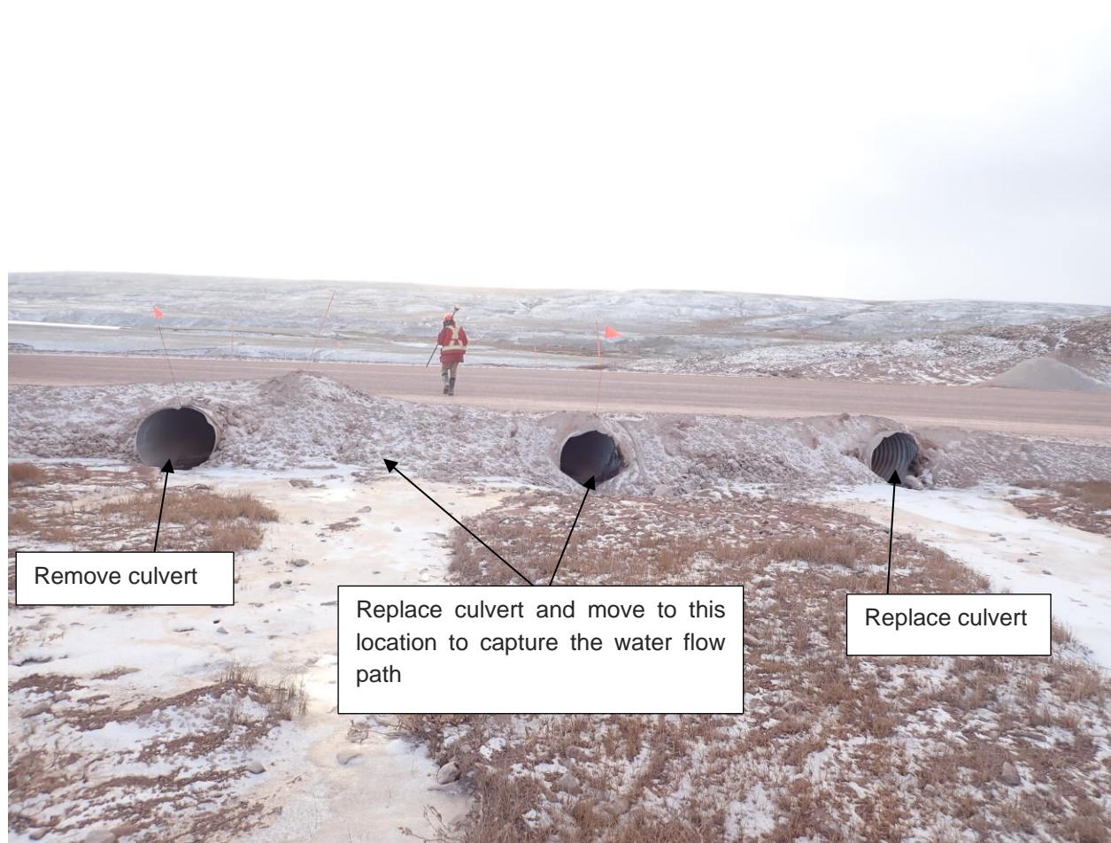
Photo B2.1 CV-112 Culvert Inlet
