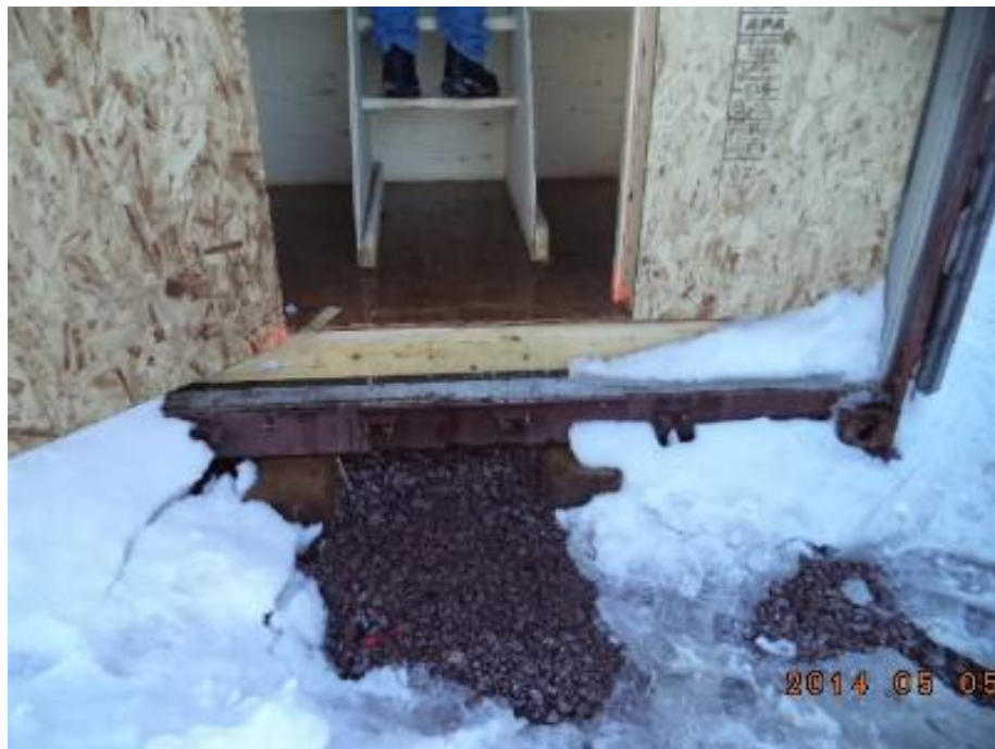
Figure 2. Sewage leak from Main Lift Station
