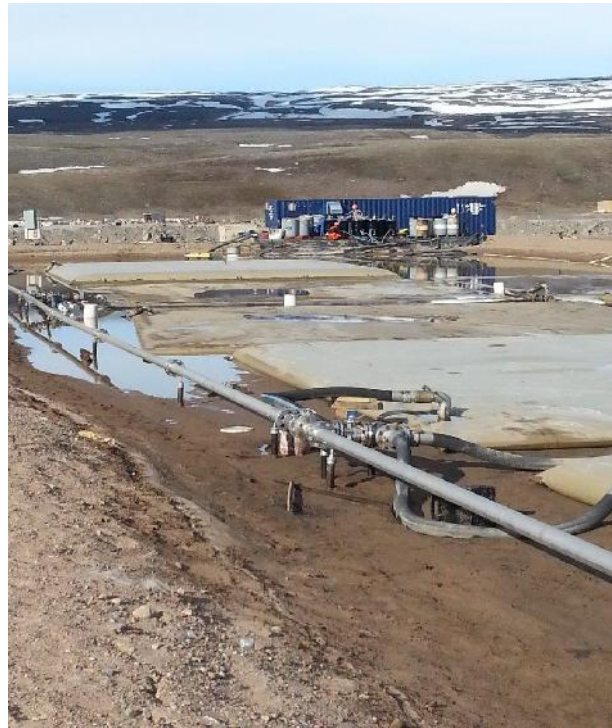
Photo 5: View of north end of facility showing oily water treatment plant and low levels of water and bladders remaining in facility. June 28.
