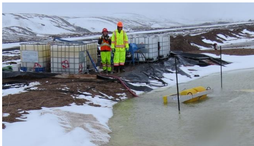
Photo 3: View of south end of facility, using drum skimmer to remove product. Operation conducted on a liner that drains back to the facility. June 1.
