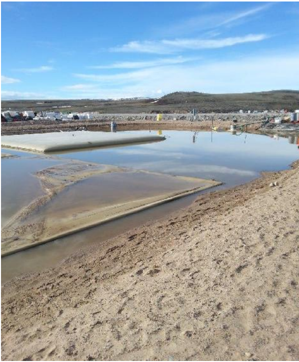
Photo 4: View of north end of facility on June 28, bladders no longer underwater allowing access to bladders to view remaining fuel and to inspect.
