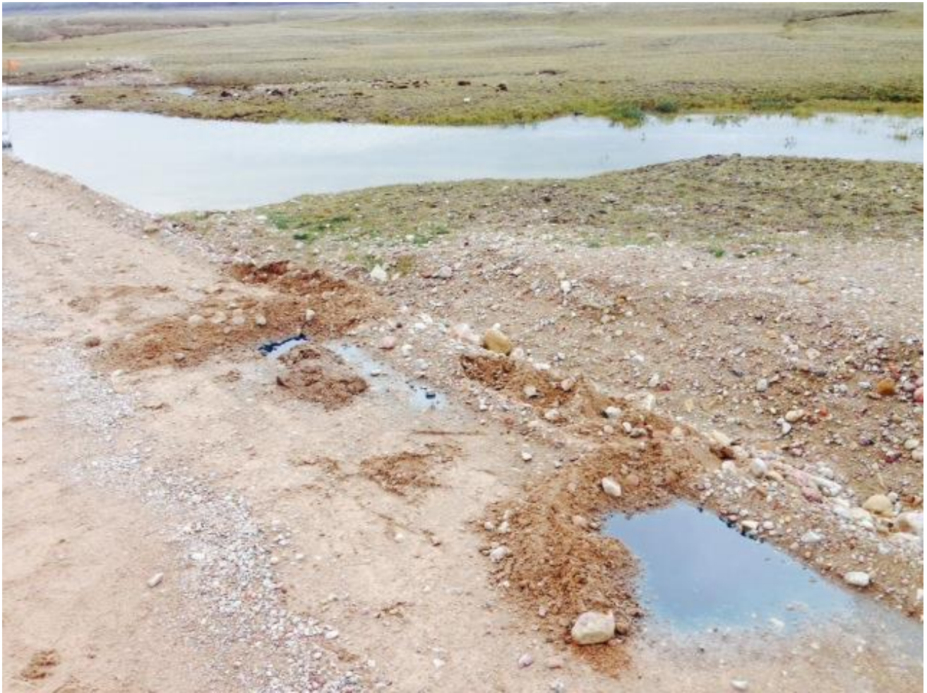
Figure 1: Earthen berms preventing oil from entering waterway
