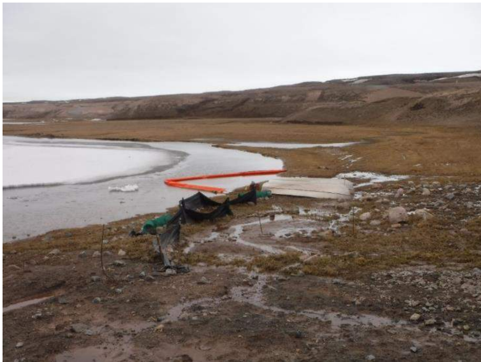
June 11, 2017 – Installation of silt curtain on the outlet of Camp Lake Sedimentation Ponds. Spring berms and silt fences installed.
