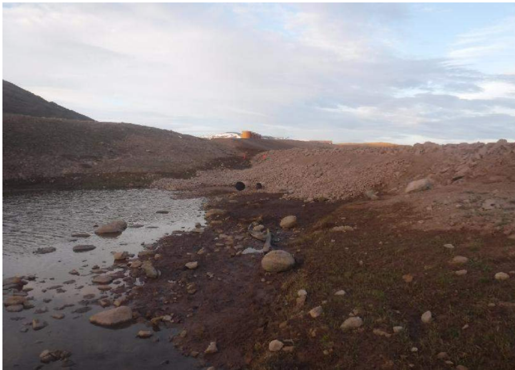
July 2, 2017 - Downstream of CV-187 (Upgraded in April 2017)
