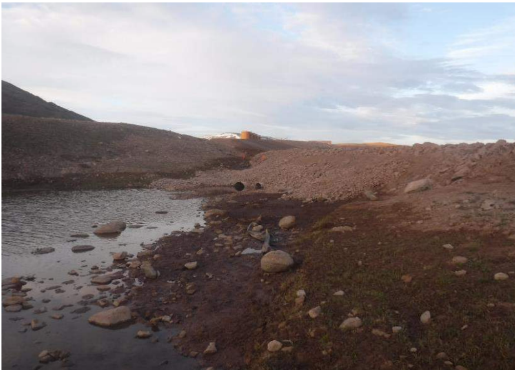
July 2, 2017 - Downstream of CV-187 (Upgraded in April 2017)
