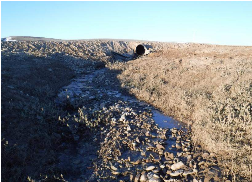
July 1, 2017 - Downstream of CV-106
