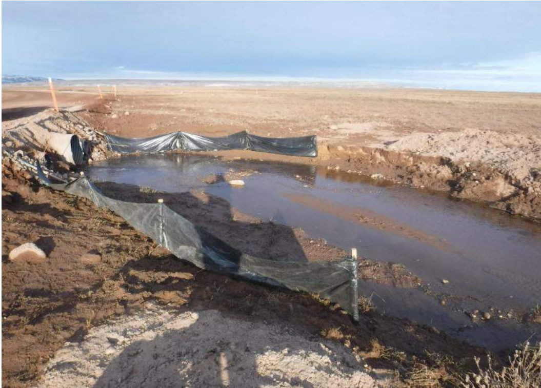
June 25, 2017 – Silt fences installed near CV-001 (downstream)
