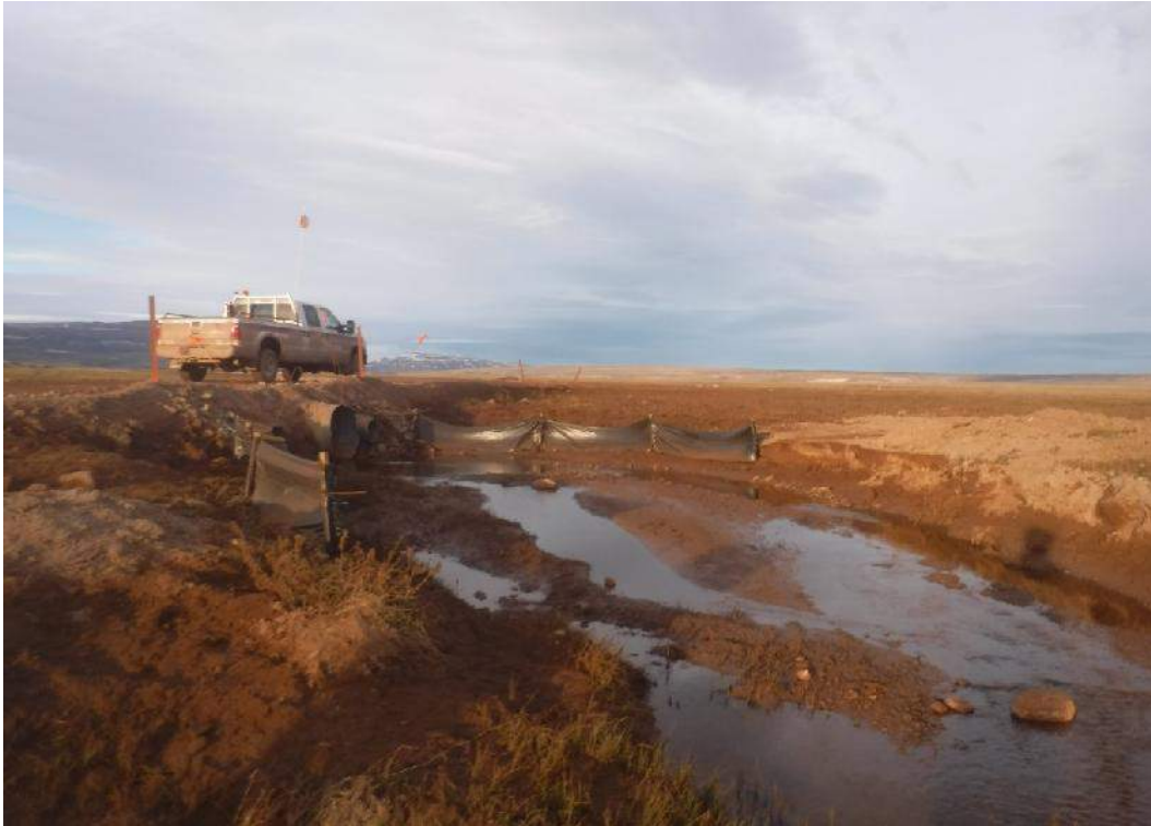
July 1, 2017 - Downstream of CV-001
