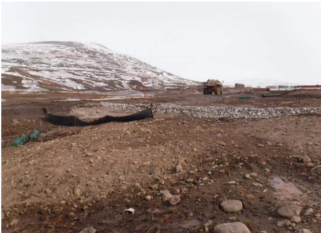
May 16, 2017 - Construction of check dam north of culvert CV-186 (Sheardown Lake Tributary 1)
