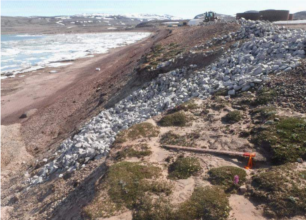
July 1, 2017 - Additional rip-rap placed downstream of MP-05
