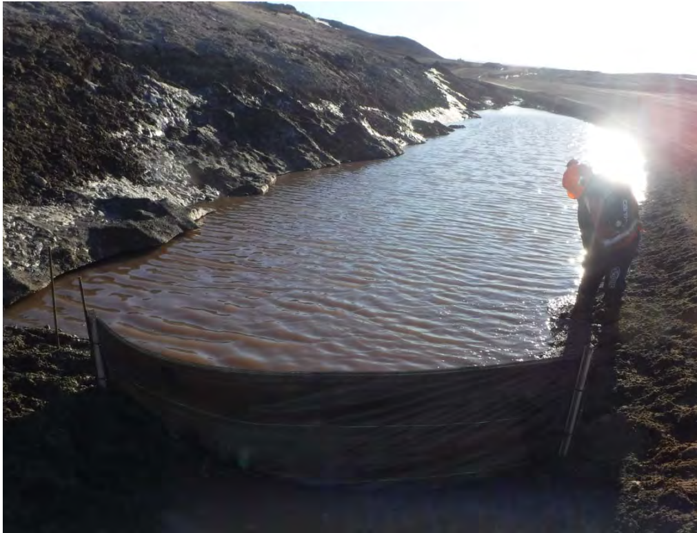
Photo 5. June 6, 2018: Silt fence being installed upstream of crossing
