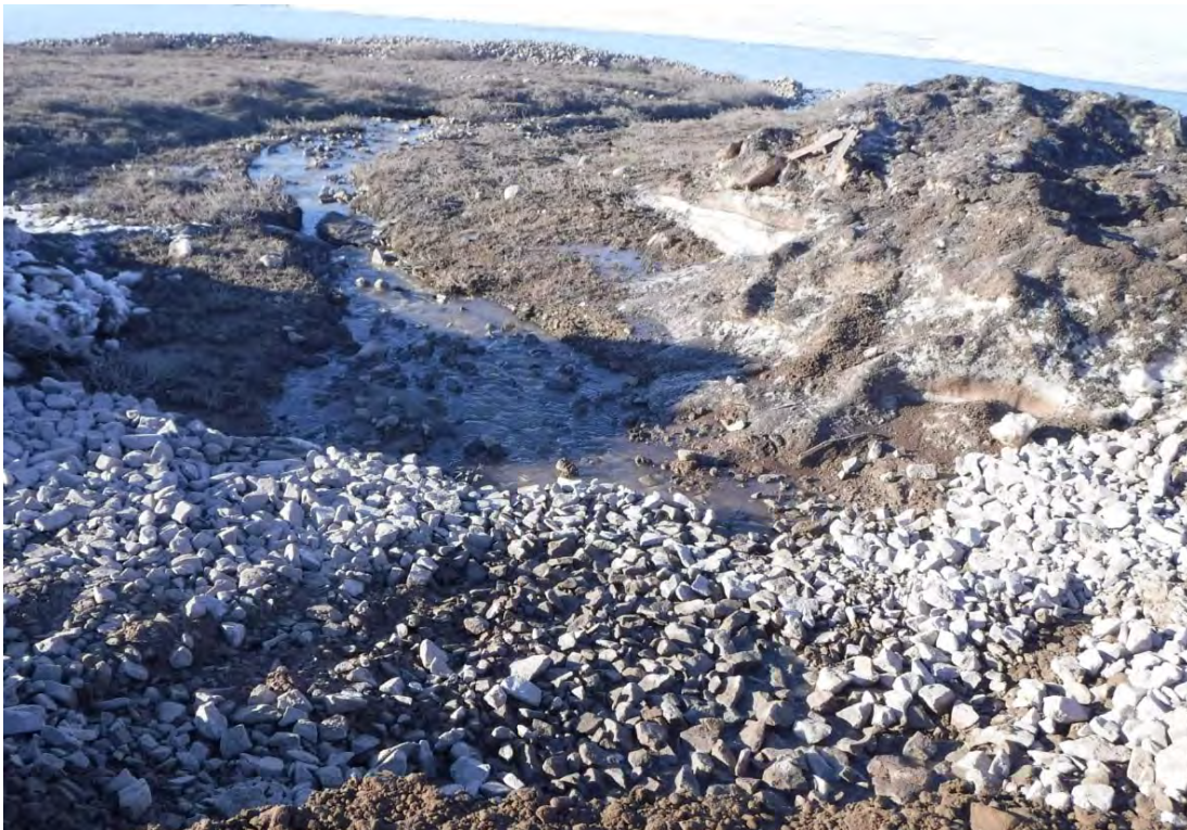
Photo 4. June 6, 2018: Bank armoring with riprap
