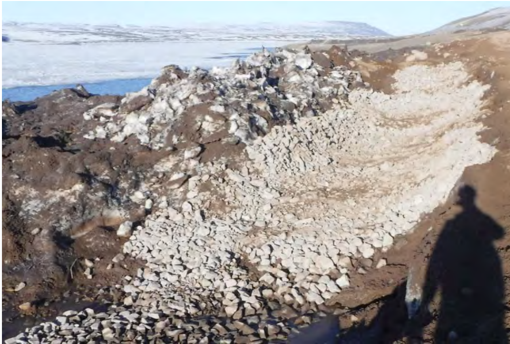
Photo 3. June 6, 2018: Bank armoring with riprap
