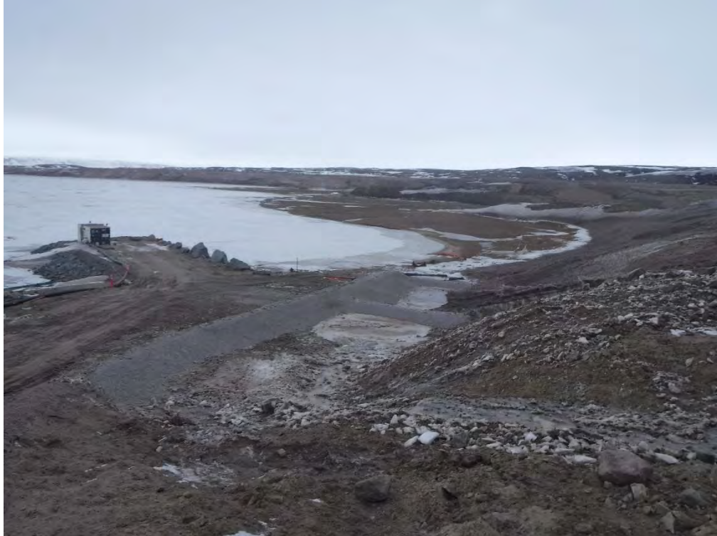
Photo 3. May 22, 2018: Camp Lake Jetty access road drainage channel check dams and berm
