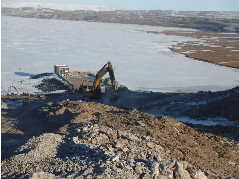
Photo 5: May 21, 2018: Reinforcement of berms/check dams at Camp Lake Jetty, during frozen conditions
