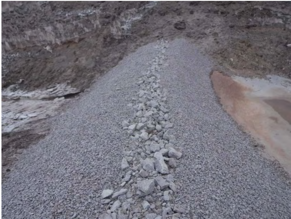
Photo 4. May 22, 2018: Typical check dam/berm cross section
