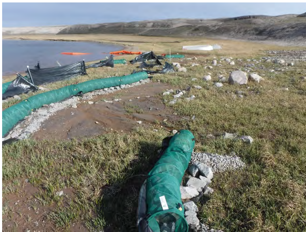
June 23, 2018: Downstream view of CLSP-OUT
