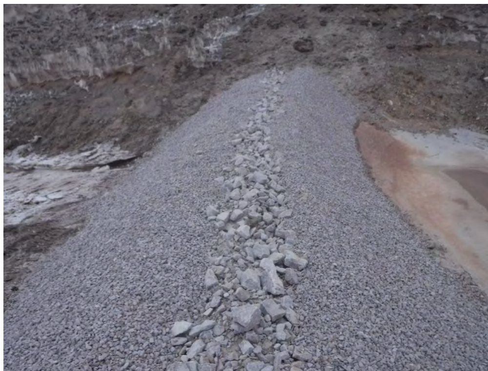
May 22, 2018: Typical Check Dam Cross Section After Construction
