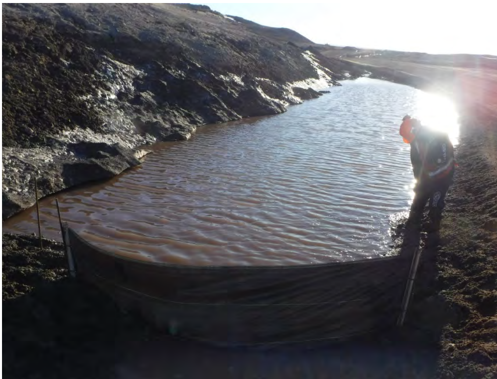
June 6, 2018: Silt Fence Installation Upstream of Crossing
