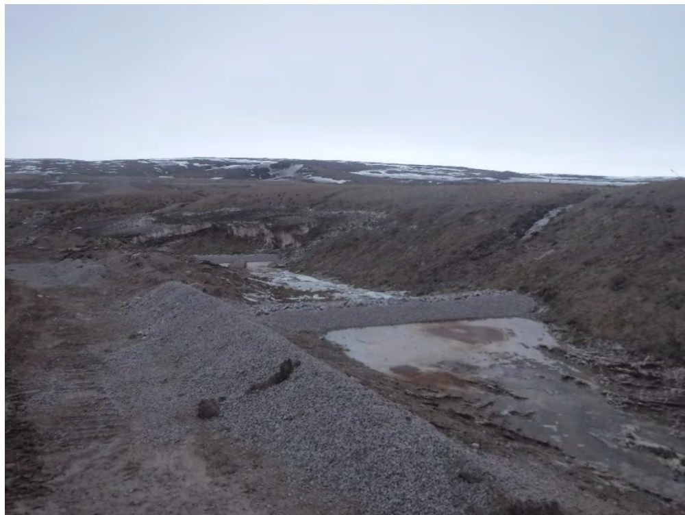
May 22, 2018: Check Dams in Camp Lake Settling Pond Drainage Channel After Construction Upgrades
