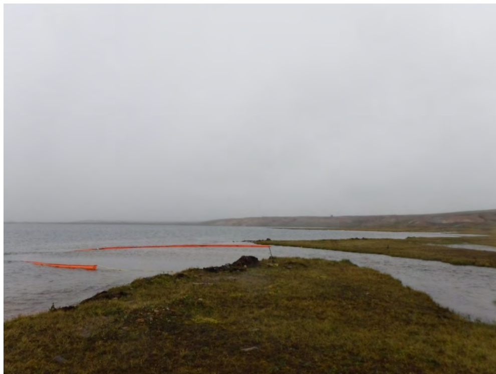
August 7, 2018: Silt Curtain Installation at CLT-OUT
