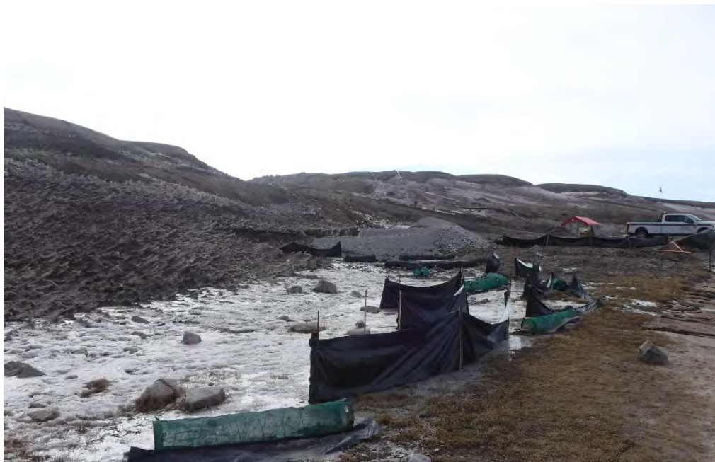
May 28, 2018: Downstream view of CLSP-OUT
