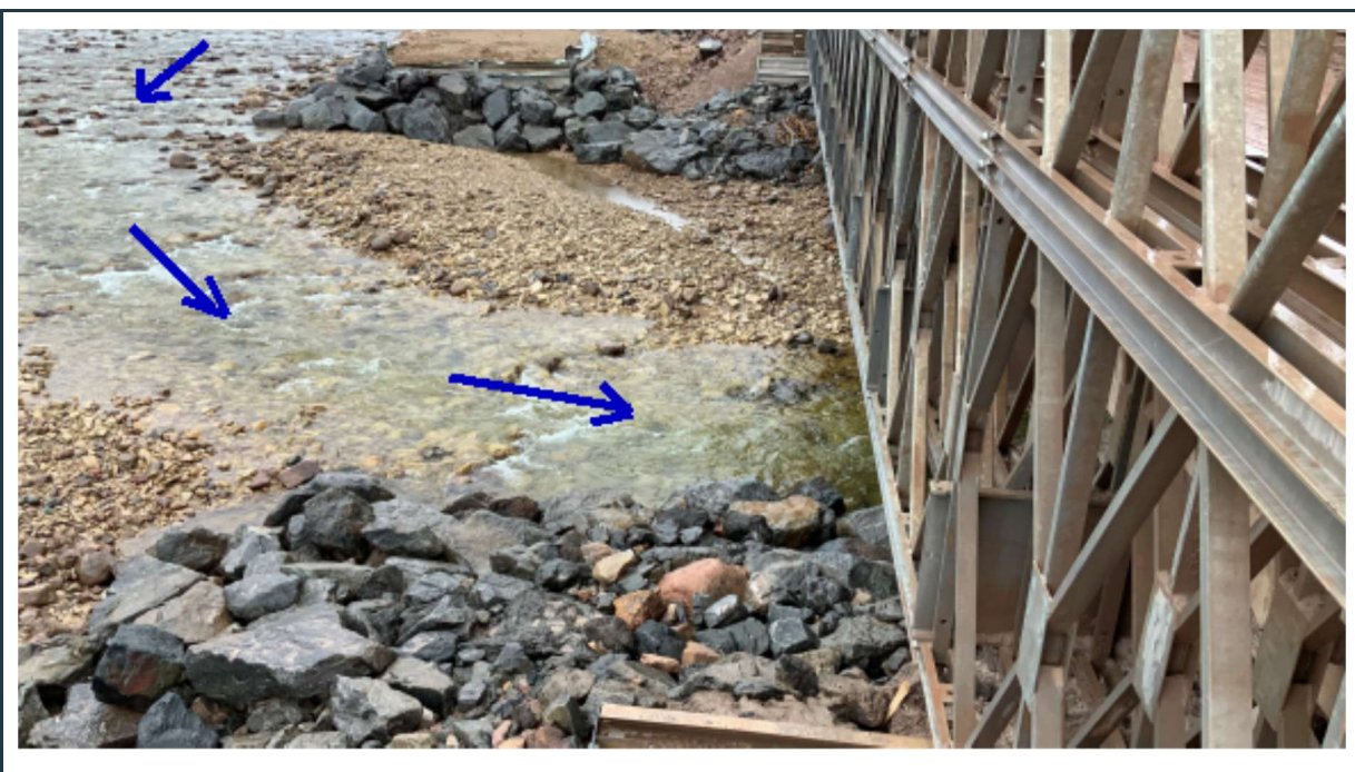
Figure 84: View of the stable abutments with low flow at the east side of bridge 63. Also note one of the two “old” abutments with riprap erosion protection.
