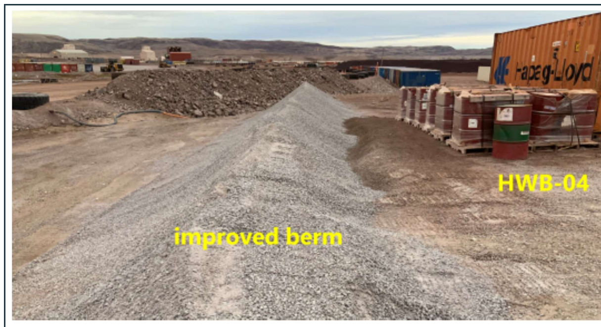
Figure 52: Recently improved (raised) berm at the HWB-4 cell, storing jet fuel and shipping containers.
