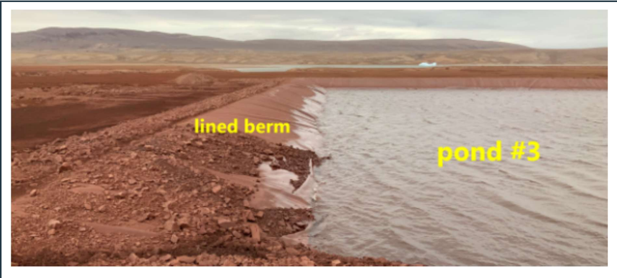
Figure 58: View of surface water management pond #3, with lined, stable berms along three sides of the pond.
