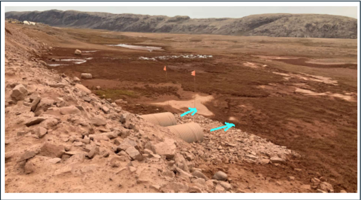
Figure 78: View of twin culverts, draining surface water from the quarry area (outlet).
