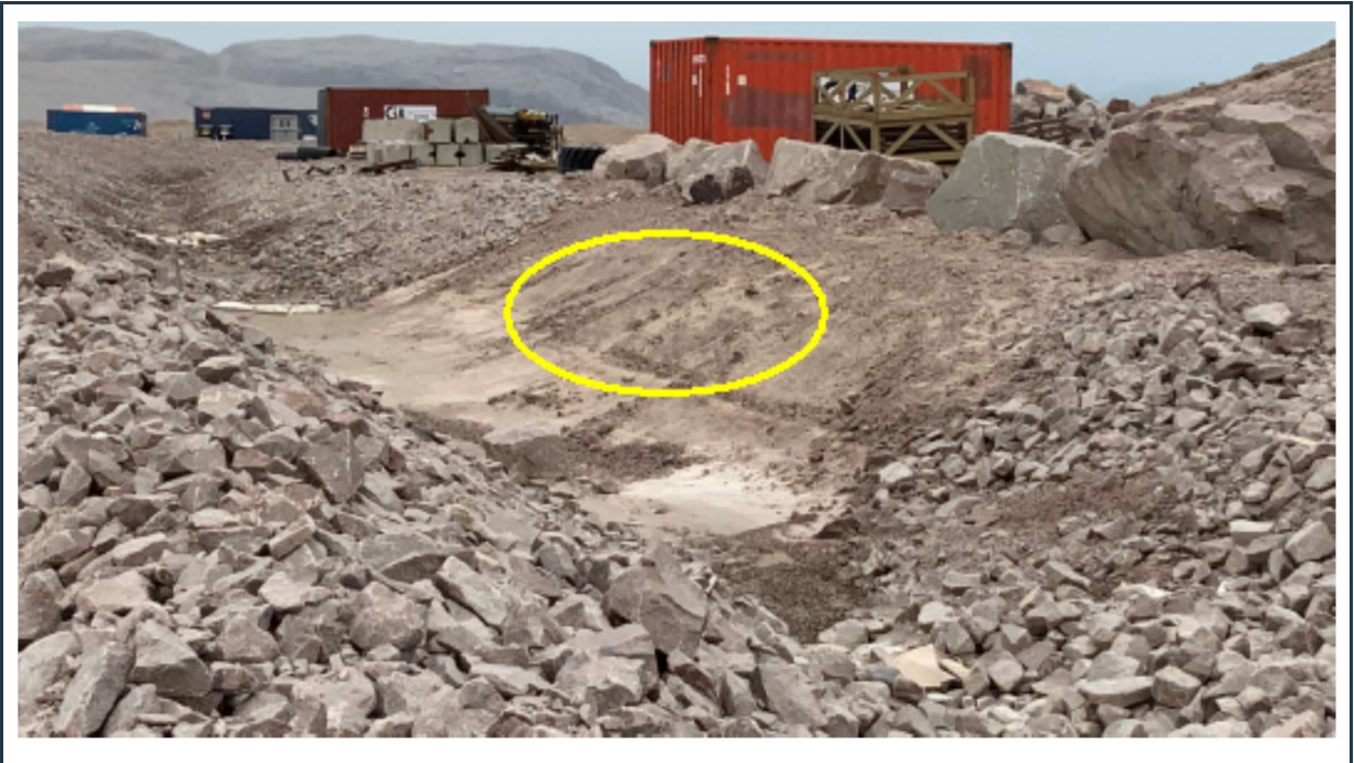
Figure 68: P-SWD-5 – “Q01-North” surface water collection ditch with missing riprap at a short section.
