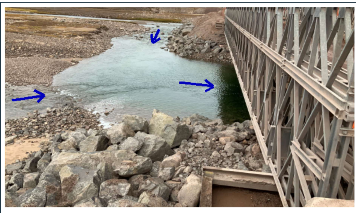
Figure 88: View of the two stable abutments with riprap scour protection at the east side of bridge 97.
