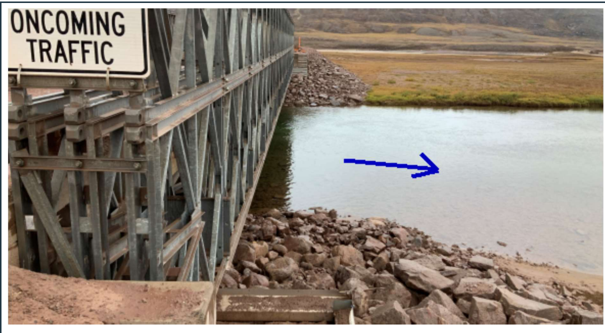
Figure 81: View of the north side of "bridge 17", with stable riprap scour protection at the abutments.
