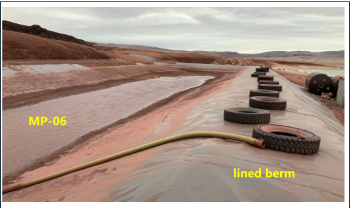
Figure 63: View of the lined MP-06 pond with robust, stable berms.
