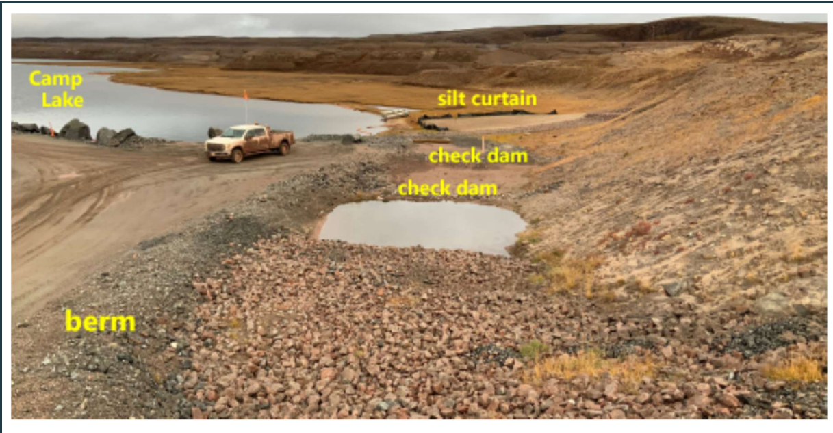
Figure 41: Camp Lake berm and check dams, constructed to form effective silt sedimentation cells. Note the silt curtain at the base of the slope for additional protection.
