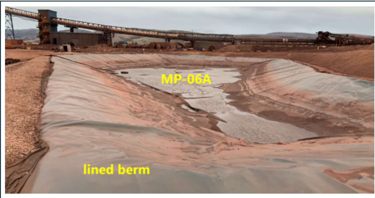
Figure 64: View of the lined MP-06A overflow pond with robust stable berms, adjacent to the ship loader.
