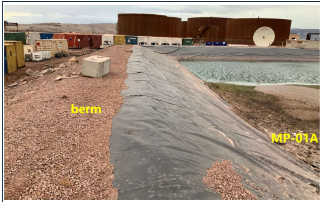
Figure 53: View of the robust, stable berms and intact liner in the MP-01A pond.
