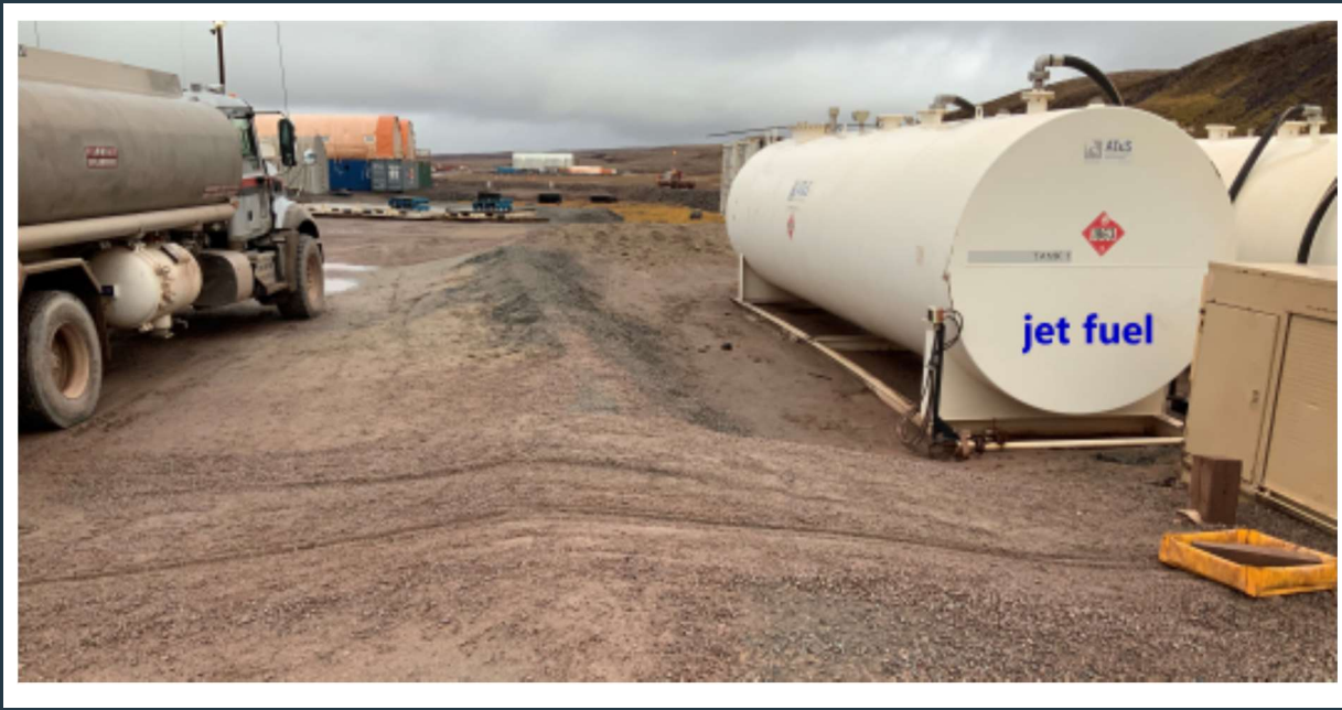
Figure 33: View of the well-maintained sand and gravel berm and access ramps at the lined jet-fuel storage facility.
