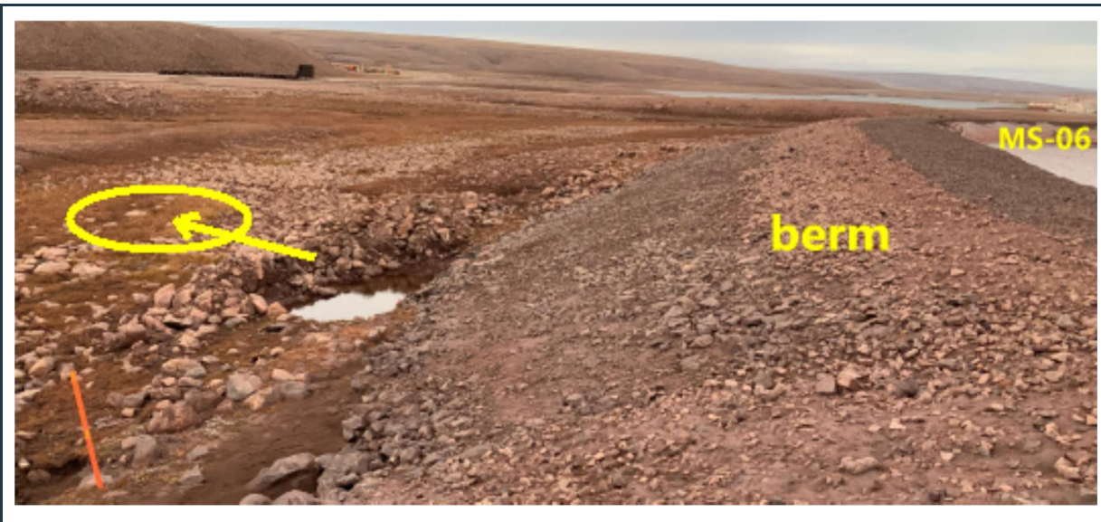
Figure 22: Seepage water within the permeable, cobbly overburden adjacent to the area of the crusher pad and the MS-06 pond's berm. The excavated temporary sump at the toe of the berm should be filled and "relocated" away from the toe of berm (to the area of the yellow circle).
