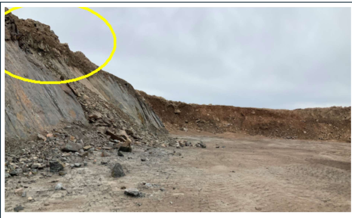
Figure 46: View of the exposed stable slope of the rock quarry with some boulders rolling down on the slope from the overburden. The soil cover on the top of the rock slope should be scaled back.
