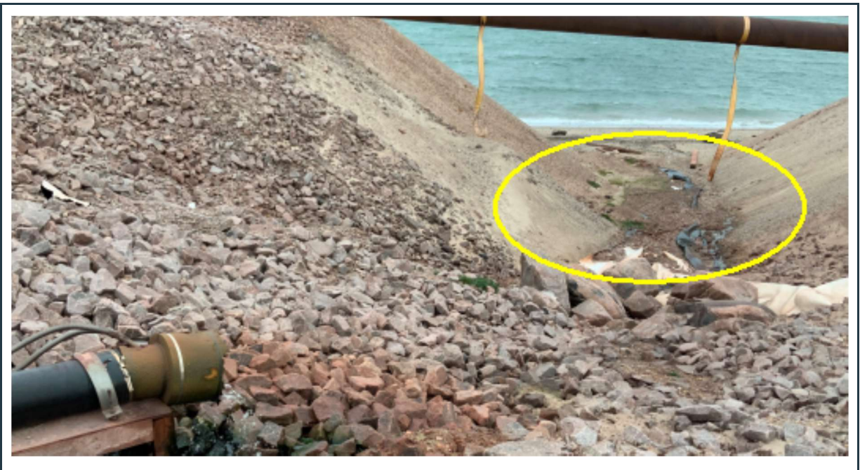
Figure 79: View of the water discharge pipe with rockfill riprap on the adjacent stable slope. More well-graded rockfill riprap should be placed over geotextile along the valley floor (yellow circle), to prevent erosion of finer soil from that area.
