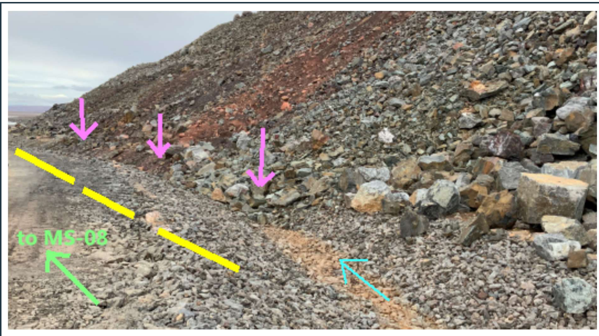
Figure 25: Drainage ditch around the west side of the waste rock facility. Note a short section of the ditch blocked by waste rock (purple arrows). It is suggested to excavate the ditch along the yellow line to facilitate easier flow of surface water within the ditch to the pond.
