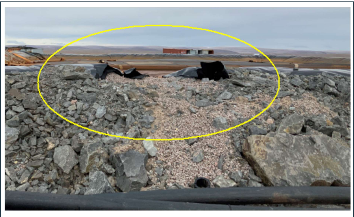
Figure 28: Damaged rock fill berm and liner at the south-west section of the berm at the geotube pond, located adjacent to the treatment plant and waste rock disposal facility.
