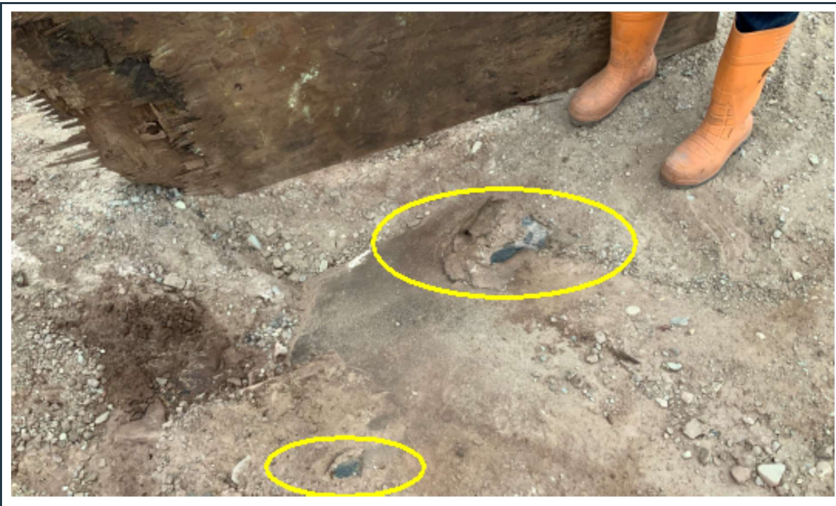
Figure 57: View of damaged geotextile at the access ramp to the MP-04A cell. The liner is still intact, but the geotextile should be repaired, and granular fill should be placed over the ramp.
