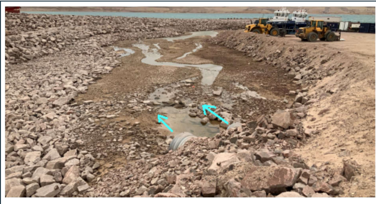
Figure 72: View of the well-maintained P-SWD-7 surface water collection ditch and culverts (outlet).
