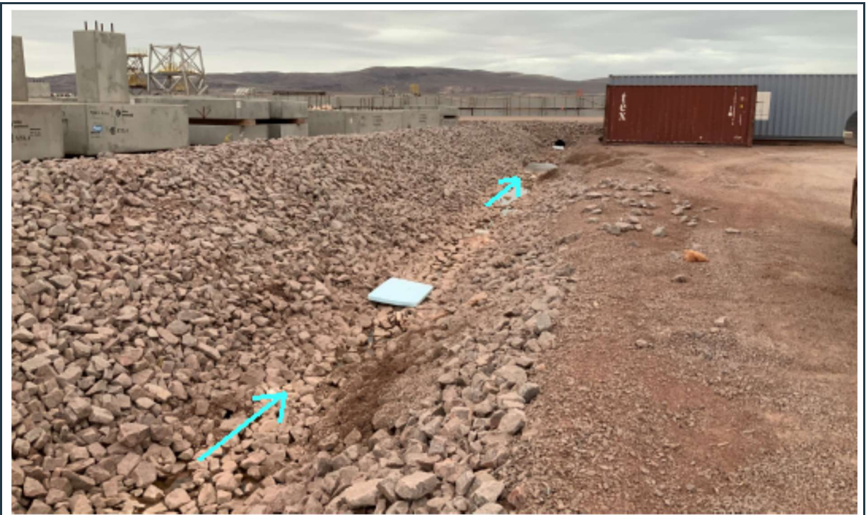
Figure 74: View of the south section of the 380-Person Camp surface water collection ditch.
