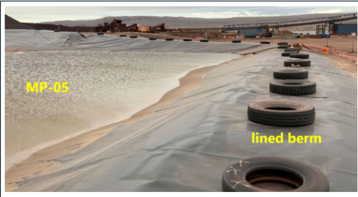
Figure 60: View of the robust, stable berms and intact liner at the MP-05 pond.
