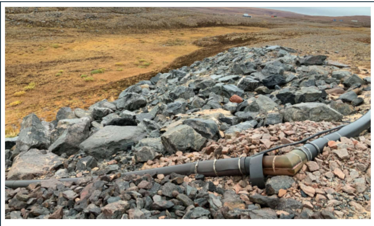
Figure 42: View of the stable rock fill riprap slope at the water discharge area.
