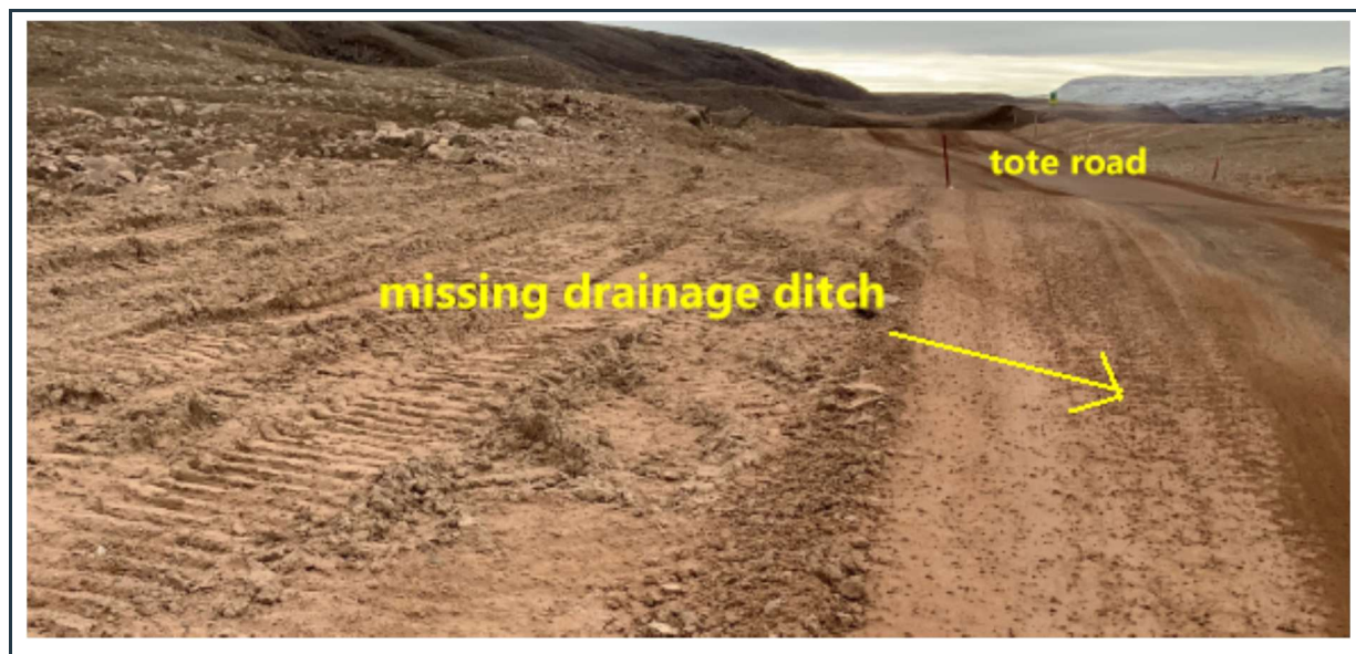
Figure 90: View of a section of the tote road around KM 07+700. No drainage ditch is provided although the ground adjacent to the road is higher than the road level and sloping toward the road.
