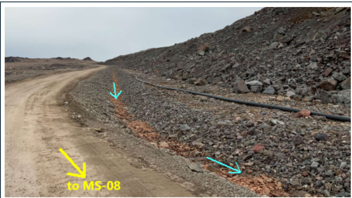
Figure 26: View of the clean drainage ditch around the east side of the waste rock facility, leading to the MS-08 pond.
