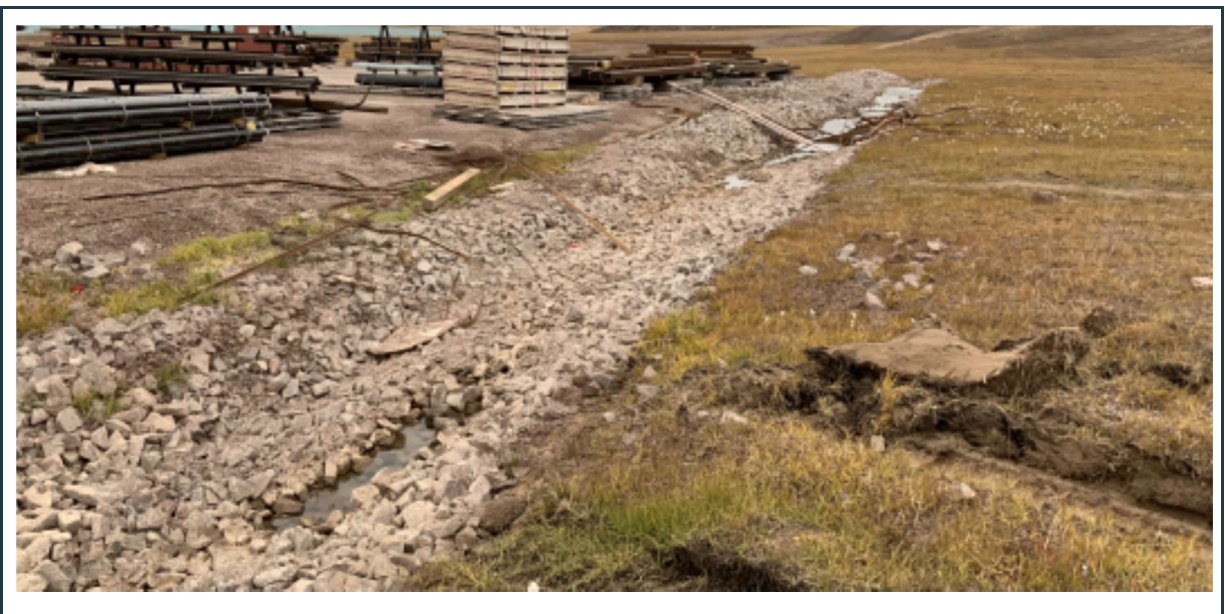
Figure 67: View of the northern part of the P-SWD-3 surface water collection ditch with failed slope sections and some debris left in the channel, which should be removed.
