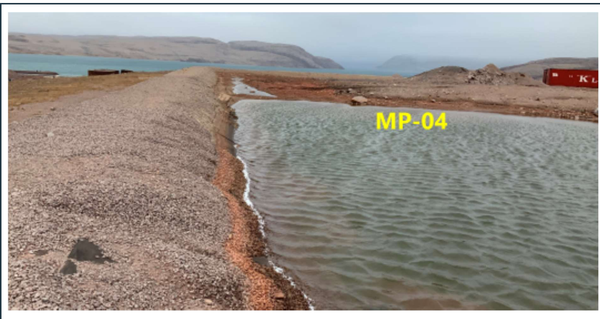
Figure 55: View of stable berm around the MP-04 land-farm, with ponding water in one corner of the cell.
