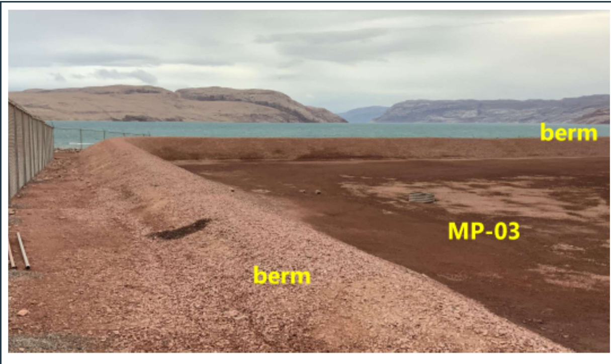
Figure 54: View of the well-maintained stable berms around the MP-03 fuel tank farm.
