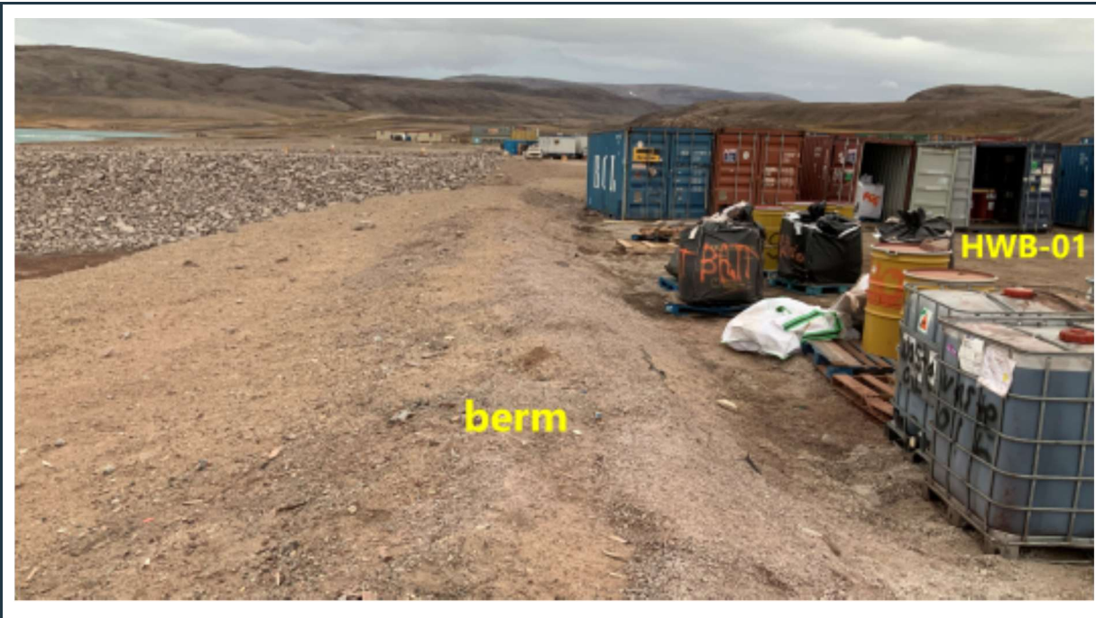
Figure 48: View of the robust, stable berm around the HWB-1 cell.
