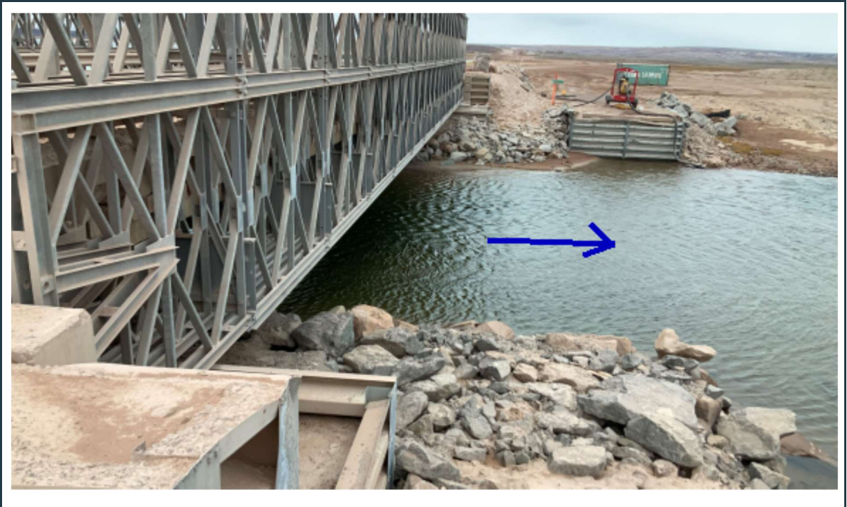
Figure 85: View of the west side of bridge 80, with stable abutments and riprap scour protection.
