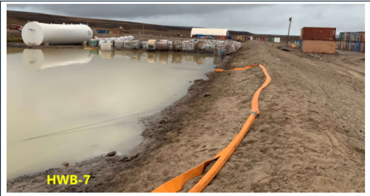
Figure 19: View of the stable berm around the HWB-7 cell, with an old fuel tank and some plastic containers stored in the cell. The ponding water is being currently removed and treated.
