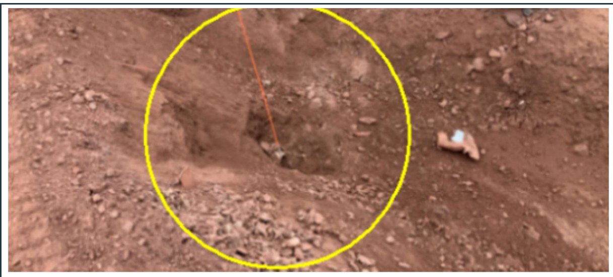
Figure 20: Drainage ditch next to the crusher plant leading to the MS-06 pond. The yellow circle indicates that the entry to the culvert that should drain the collected surface water from the ditch to the MS-06 pond is partly clogged (should be cleaned). Extending the culvert is also suggested.
