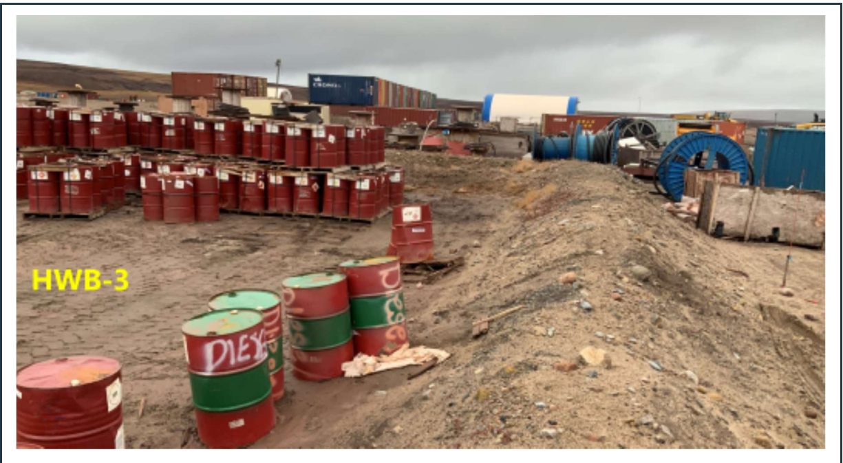
Figure 15: View of stable berms and stored fuel barrels in HWB-3.
