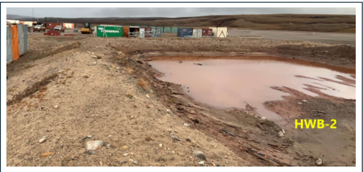
Figure 14: View of the robust, stable berms around HWB-2. The presence of water in the cell indicates good liner performance. No material is currently stored in this cell.
