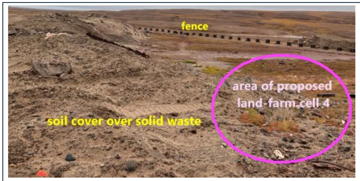
Figure 38: View of soil cover over solid waste in the landfill facility. Note the proposed area for land-farm Cell 4 (see Figure 34 for the entire land-farm cell layout).
