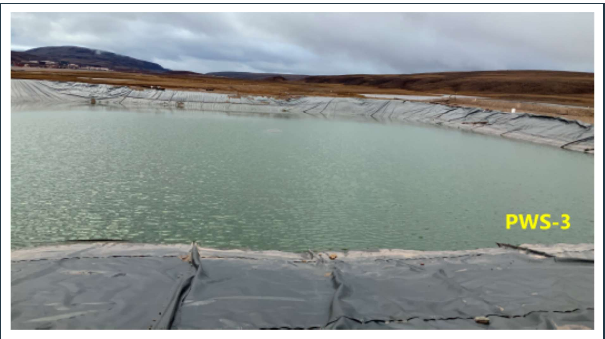
Figure 12: Robust, stable perimeter berms around PWS pond #3 – Wrinkles are common on exposed liners, but they do not pose a risk to the integrity of the high-strength HDPE liners.
