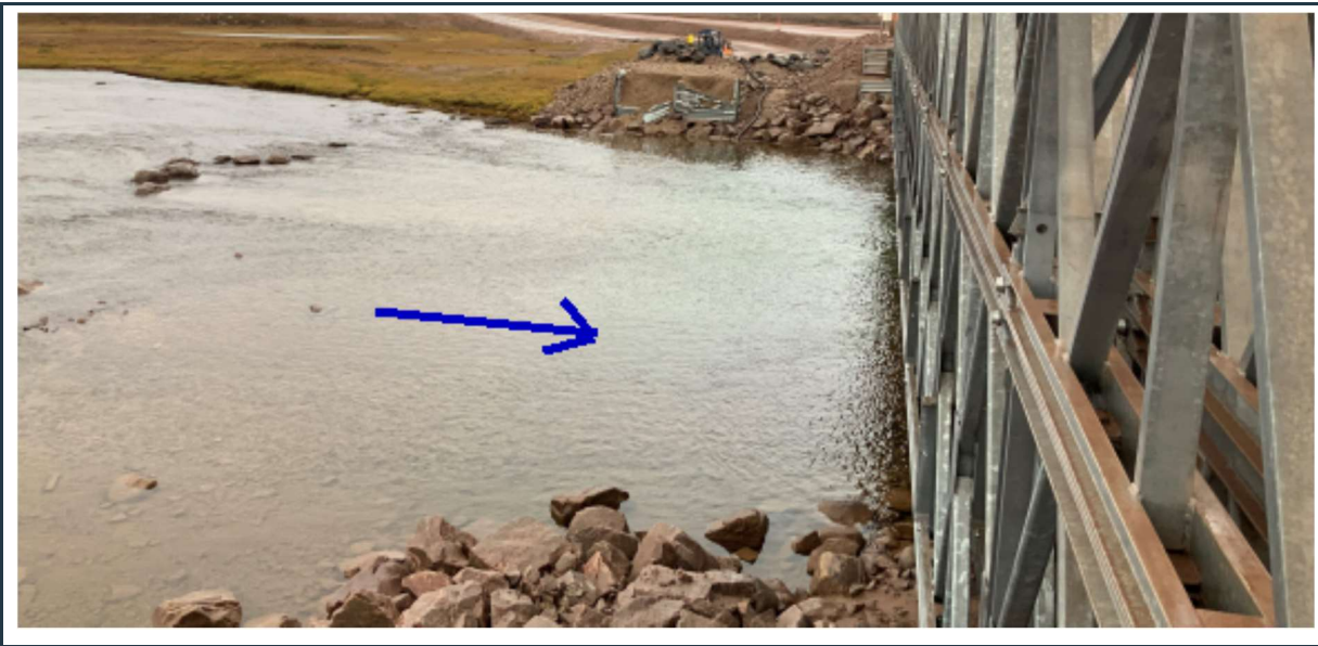
Figure 82: View of the stable abutments with riprap erosion protection at the south side of "bridge 17".
