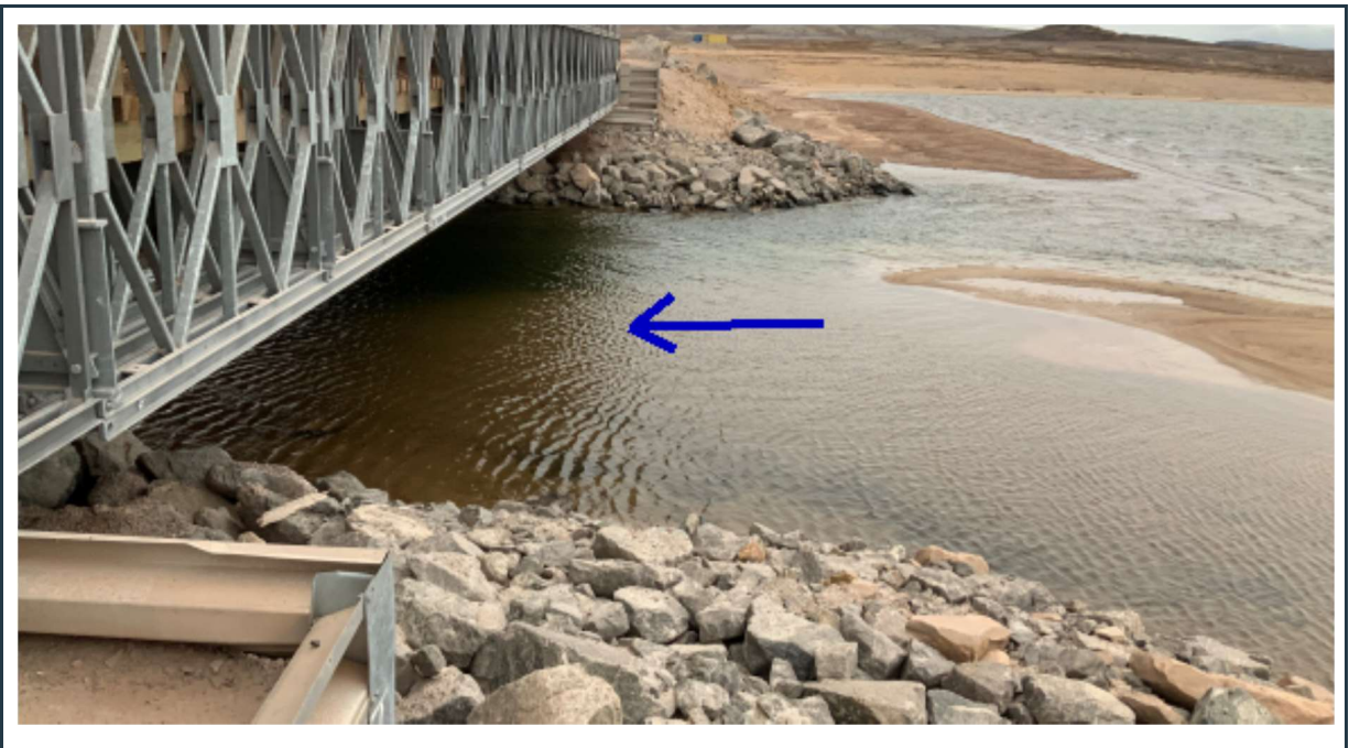
Figure 86: View of stable abutments with riprap scour protection at the east side of bridge 80.
