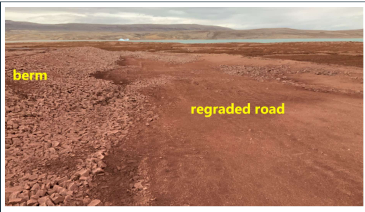
Figure 59: View of the north berm at settling pond #3, with the road regraded adjacent to the berm.
