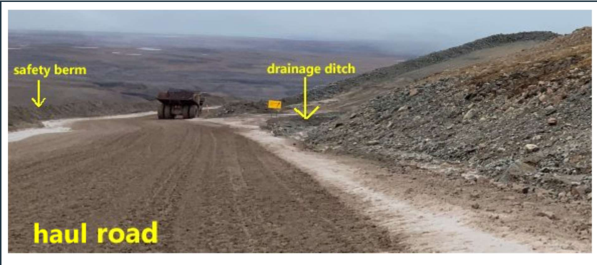
Figure 95: View of the haul road between the crusher pad and the open pit around KM-107. Note the standard road components in the image, the safety berm along the fill (left) side of the road and the drainage ditch along the cut side (right) of the road.
