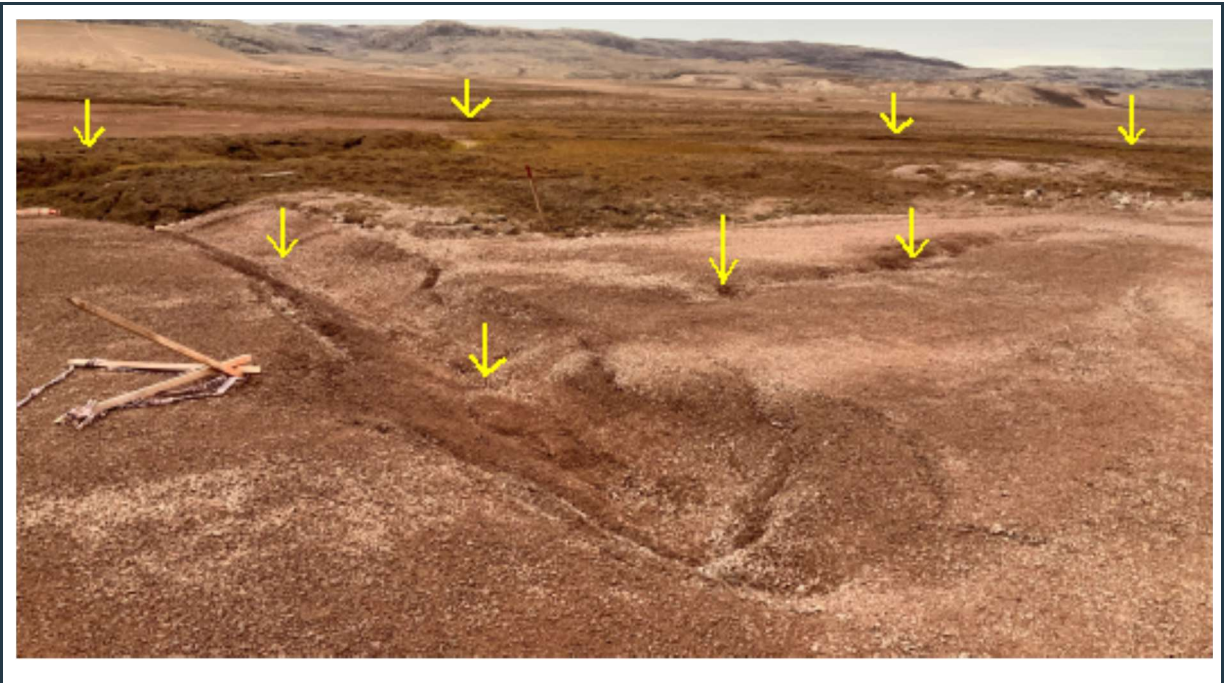
Figure 80: View of a network of natural cracks and depressions on the surface in the area at and adjacent to the LP-5 storage area. The depressions across the storage area should be filled with more sand and gravel and the surface shall be regraded.
