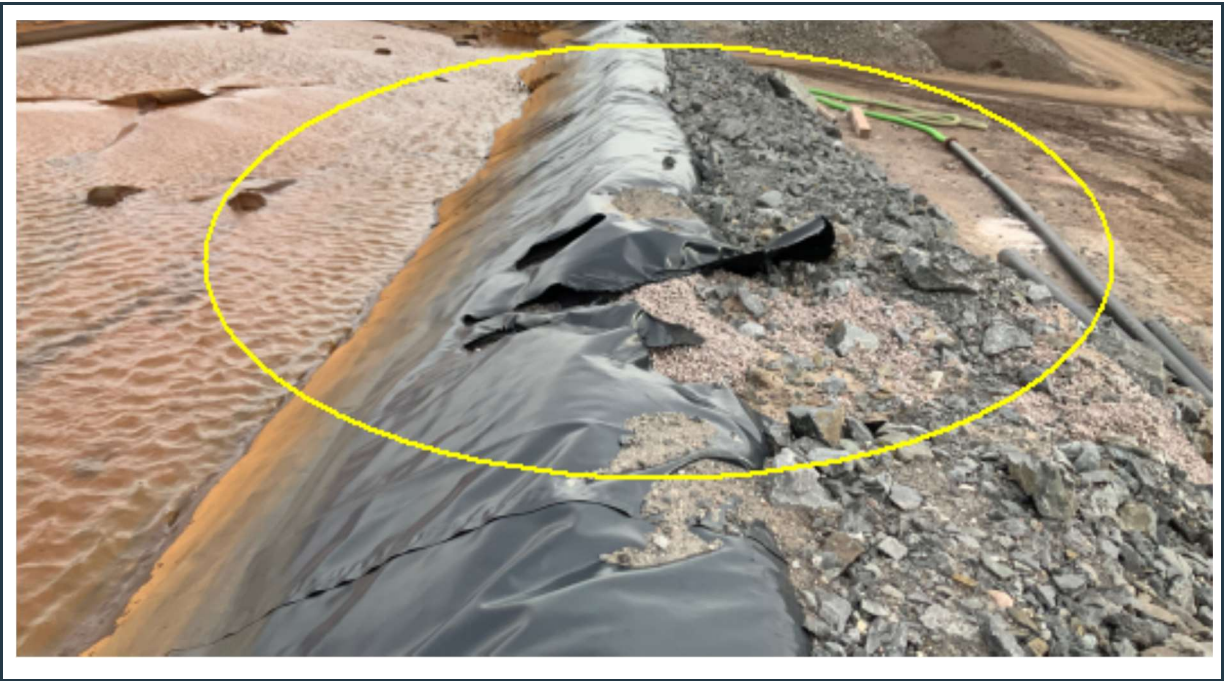
Figure 27: Damaged liner at the south-west section of the berm (yellow circle) at the geotube pond, located adjacent to the treatment plant and waste rock disposal facility.
