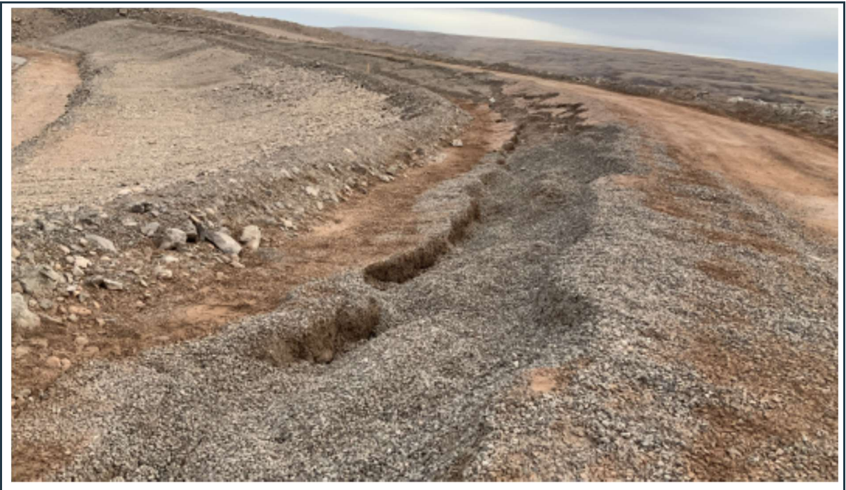
Figure 31: View of freeze/thaw related ground movement along the road next to the MS-11 slope. The area of the cracks should be regraded/compacted to minimize water infiltration into the ground next to the slope.
