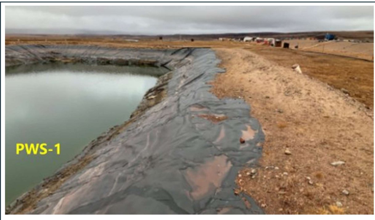
Figure 10: PWS pond #1. Well-maintained, stable perimeter berm and liner at the pond.
