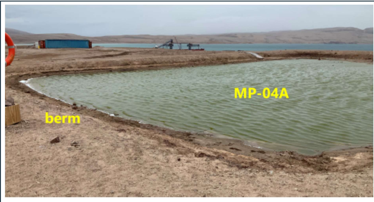
Figure 56: View of the MP-04A cell with stable berms. The ponding water indicates good liner performance.
