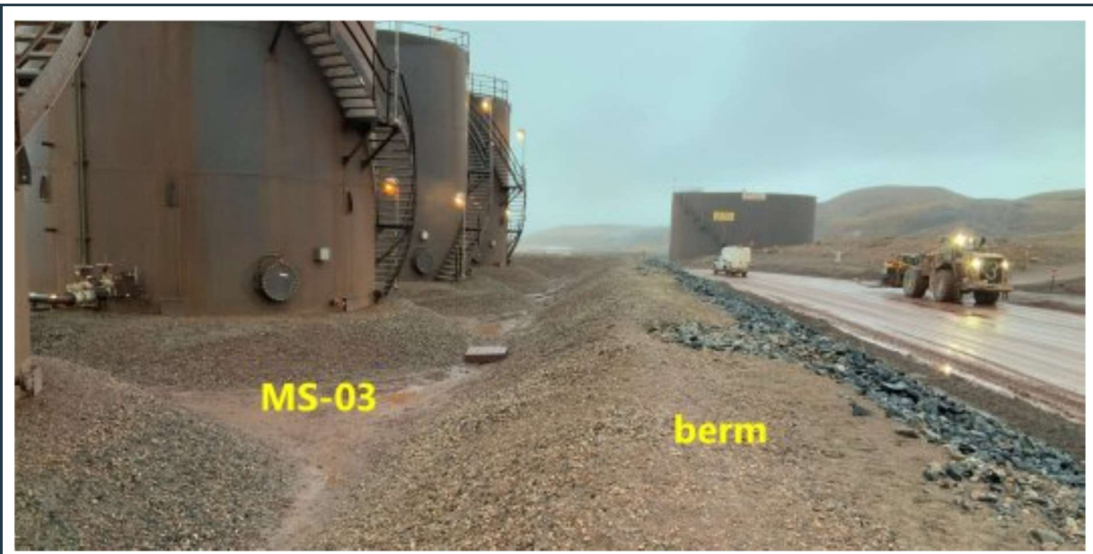
Figure 34: Well-maintained, stable berm around the MS-03 diesel fuel farm, with some ponding water. No problems with the liner were noted anywhere in this facility.
