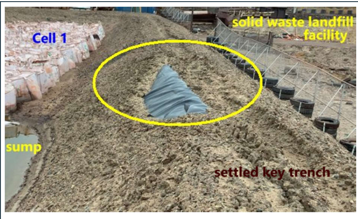
Figure 39: View of a section of the recently constructed berm at the land-farm's Cell 1. Note the exposed liner above the sump area and the settled anchor trench along the top of the berm.
