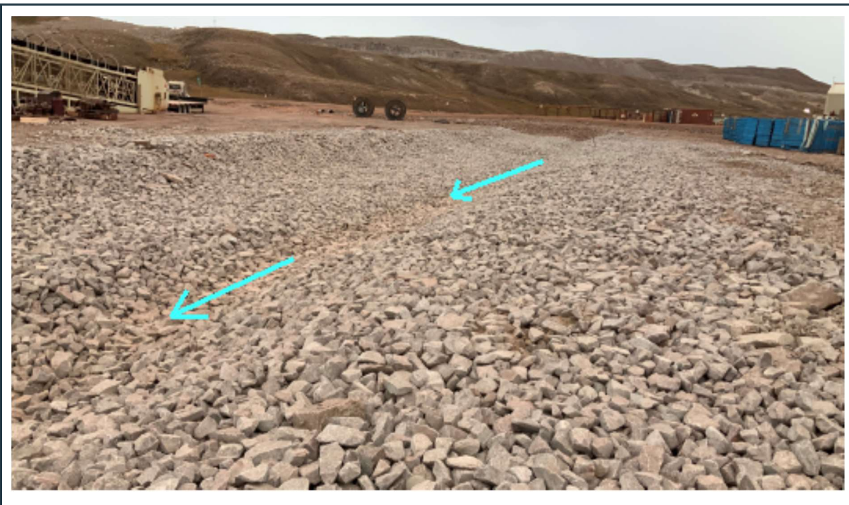
Figure 73: View of the recently completed W3/W14 surface water collection ditch with crushed rock riprap slope protection.
