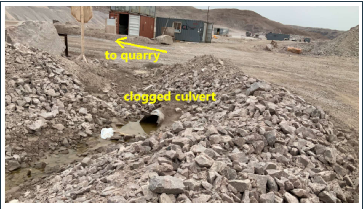
Figure 69: Clogged culvert at the entrance to the quarry in P-SWD-5/Q01-North surface water collection ditch. Should be replaced with a new, larger diameter culvert.
