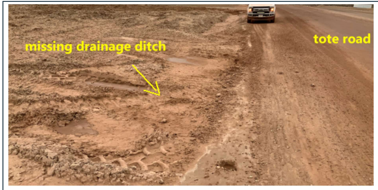
Figure 89: View of a section of the tote road around KM 06+900. No drainage ditch is provided although the ground level adjacent to the road is higher than the road level.
