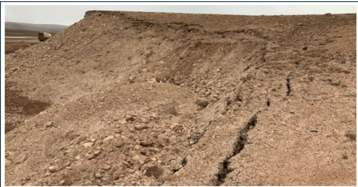
Figure 94: View of the slope at a cut section of the road at KM 28+900. Note the tension cracks on the crest of the slope due to freezing and thawing action in the ground. The slope is located somewhat closer to the road, but at this stage it may not present any risk to the traffic on the road or to the stability of the road. However, the slope should be monitored and reshaped to shallower inclination if necessary.
