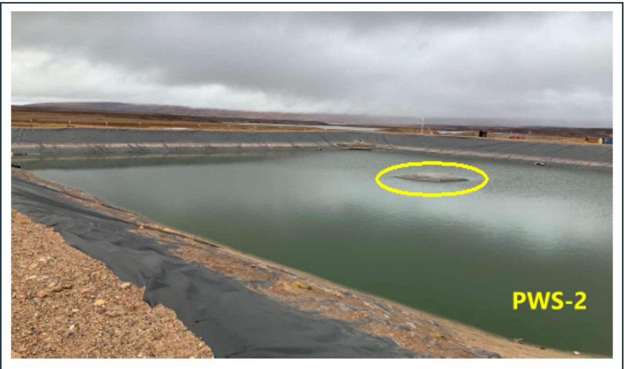
Figure 11: PWS pond #2 – Stable, well-maintained berm and liner. – A small section of the liner is visible in the center of the pond (yellow circle), which does not pose a risk to the integrity of the liner.
