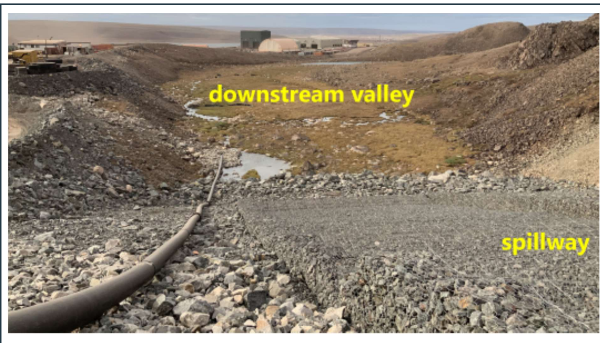
Figure 30: View of the robust and stable emergency spillway (gabion baskets and blankets filled with crushed rock) at KM105. Note the water seepage at the toe of the spillway.
