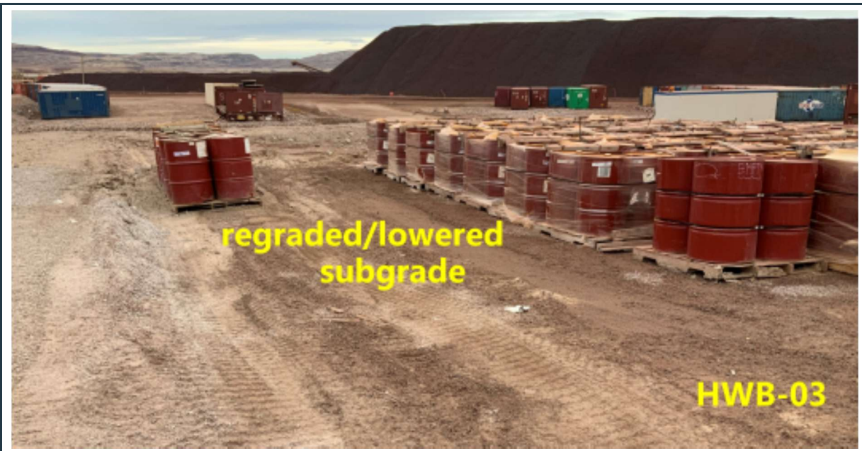
Figure 51: View of the HWB-3 cell with stable berms, containing fuel barrels. The interior subgrade has been regraded/lowered, as specified in the previous inspection report.
