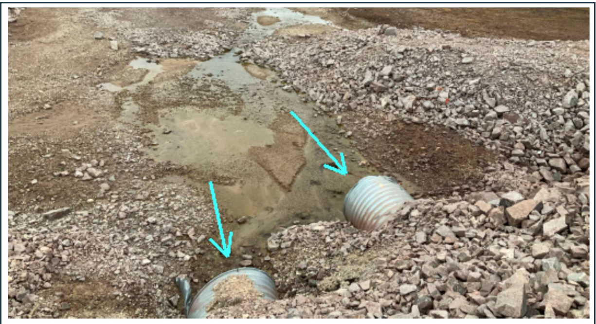
Figure 71: View of the P-SWD-7 surface water collection ditch and culverts (inlet).
