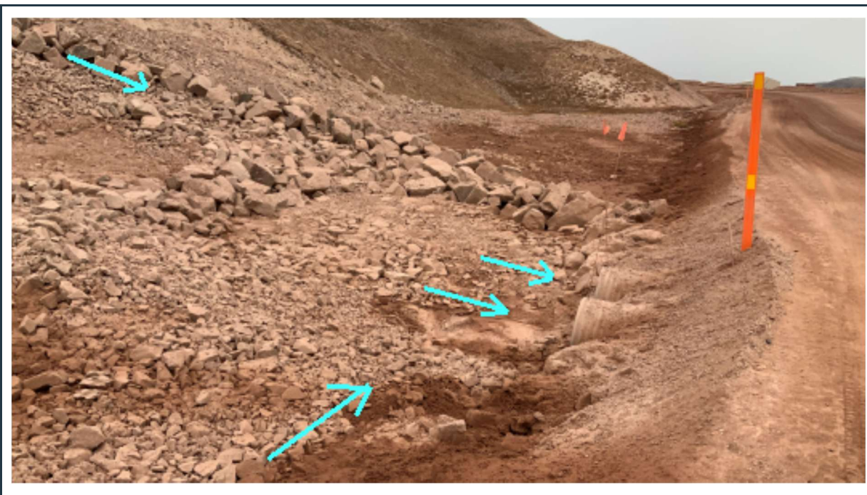
Figure 77: View of twin culverts, draining surface water from the quarry area under the tote road (inlet).
