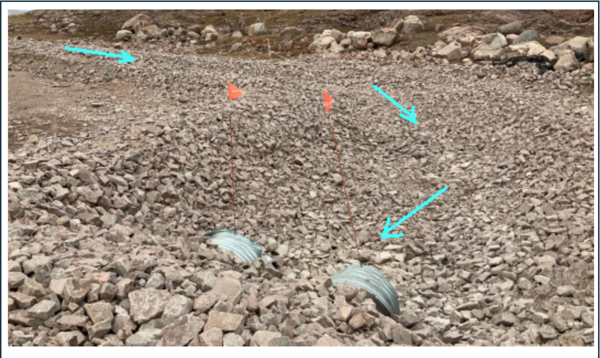
Figure 70: View of the south end of the rock fill lined P-SWD-6 surface water collection ditch.
