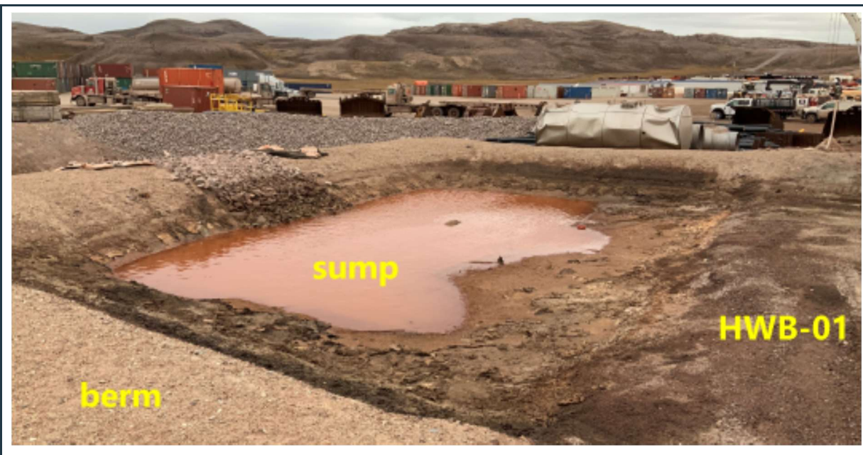
Figure 49: View of the sump at the back of the HWB-01 cell with stable berms.
