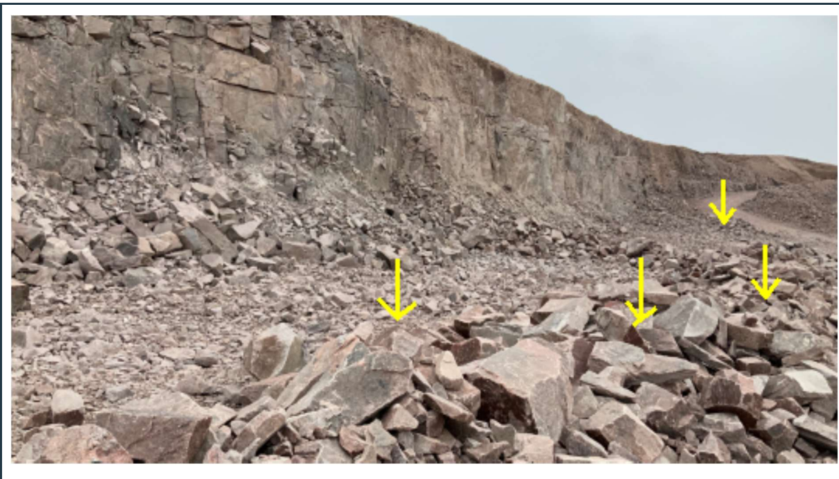
Figure 65: View of stable highwalls with minor weathering and bench erosion in the Q01 rock quarry. Note the safety berm between the access road and the face of the rock wall (yellow arrows).
