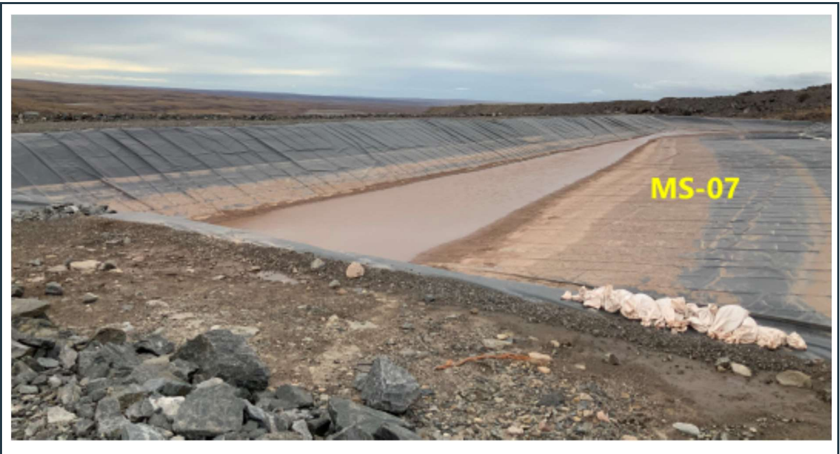
Figure 23: View of the robust, stable berms and intact liner at the MS-07 surface-water management pond. The pond was almost empty at the time of the September visit.
