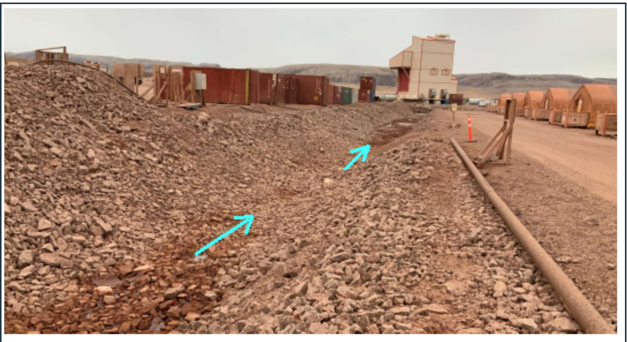
Figure 75: View of the east section of the 380-Person Camp surface water collection ditch in good condition.
