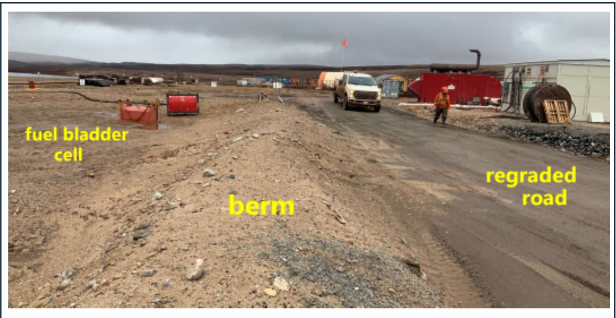
Figure 32: View of the stable berm around the "fuel bladder" cell. The adjacent road next to the east berm was recently regraded to improve surface drainage in the area.
