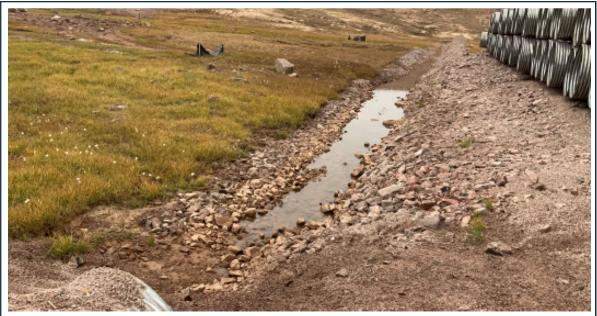
Figure 66: View of the southern part of the P-SWD-3 surface water collection ditch with failed slope sections, and ponding water due to inadequate longitudinal channel slope.
