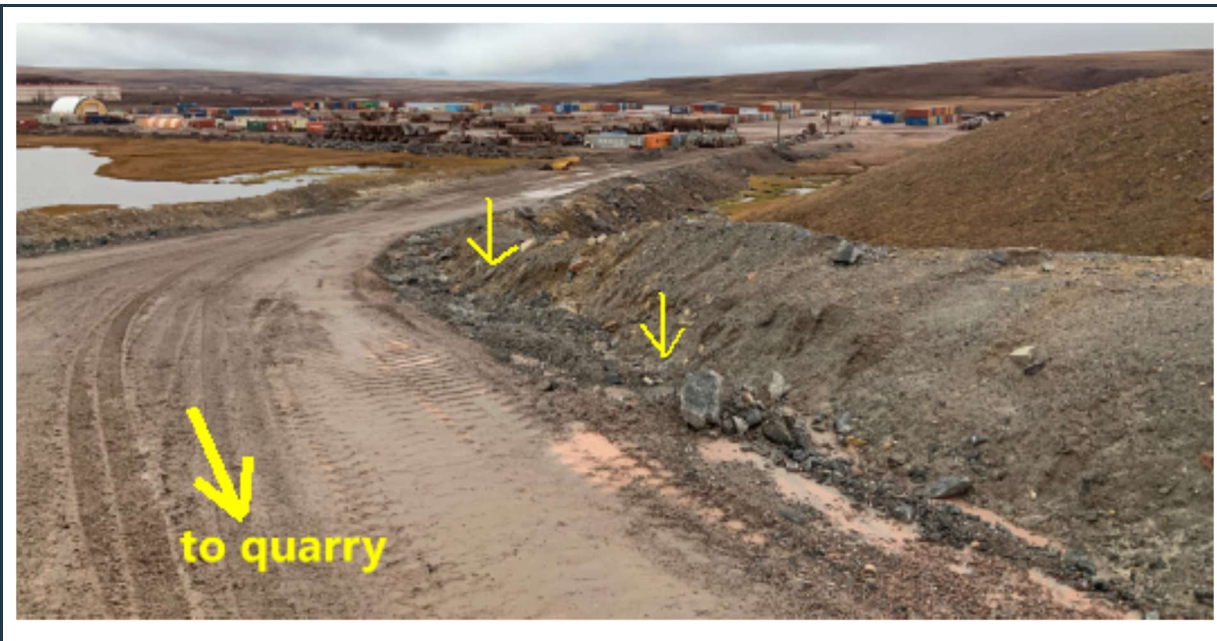
Figure 45: Erosion problem still exists along the edge of the access road to the quarry.
