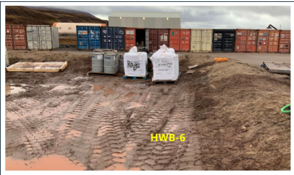
Figure 18: View of stable berms around, and the regraded granular fill within the HWB-6 cell. The ponding rainwater in the cell indicates good liner performance.
