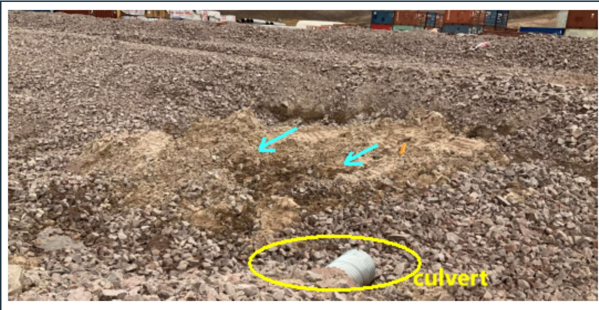
Figure 76: View of the PSC surface water collection ditch. Note the localized slope degradation due to frequent water seepage from the granular fill of the LP-2 laydown pad (blue arrows).
