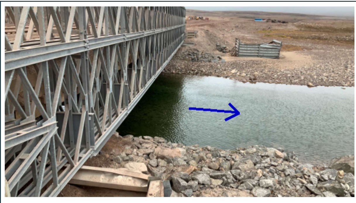
Figure 87: View of the stable abutments with riprap scour protection at the west side of bridge 97.
