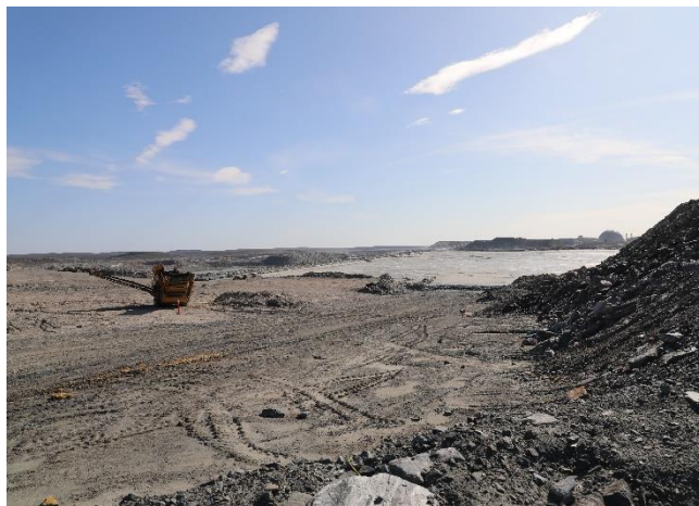
Photo 28: Tailings Storage Facility – South Cell
