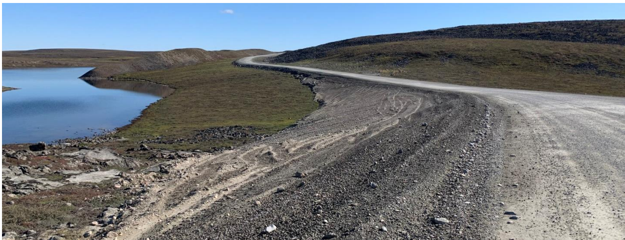
Photo 69: Whale Tail Haul Road Resloped
