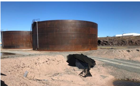
Photo 37: Exposed Liner at Fuel Tanks
