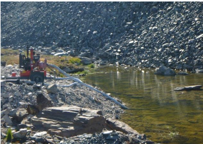
Photo 21: Seepage from Portage Waste Rock Storage Facility
