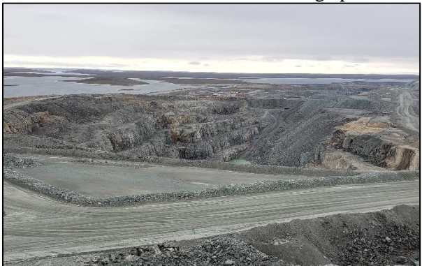
Goose Pit being used for in-pit tailings disposal
