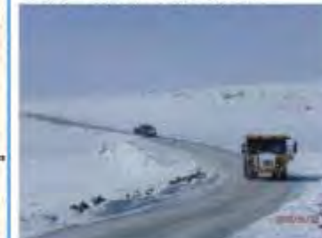
Protection berm along curve
