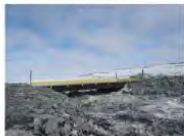
Temporary bridge km 3.4
