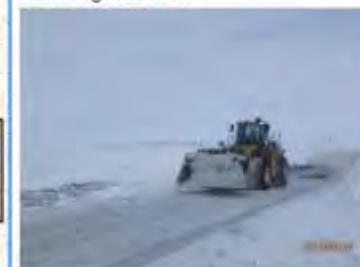
Road maintenance with loader
