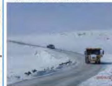
Protection berm along curve
