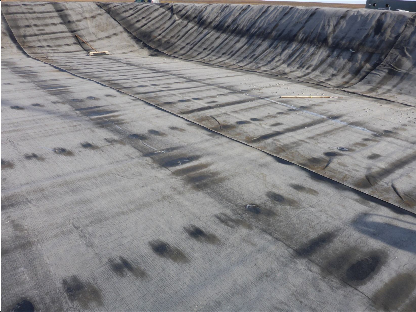
Description: Close up of the Coletanche geomembrane used in the construction of the powerhouse secondary containment.
