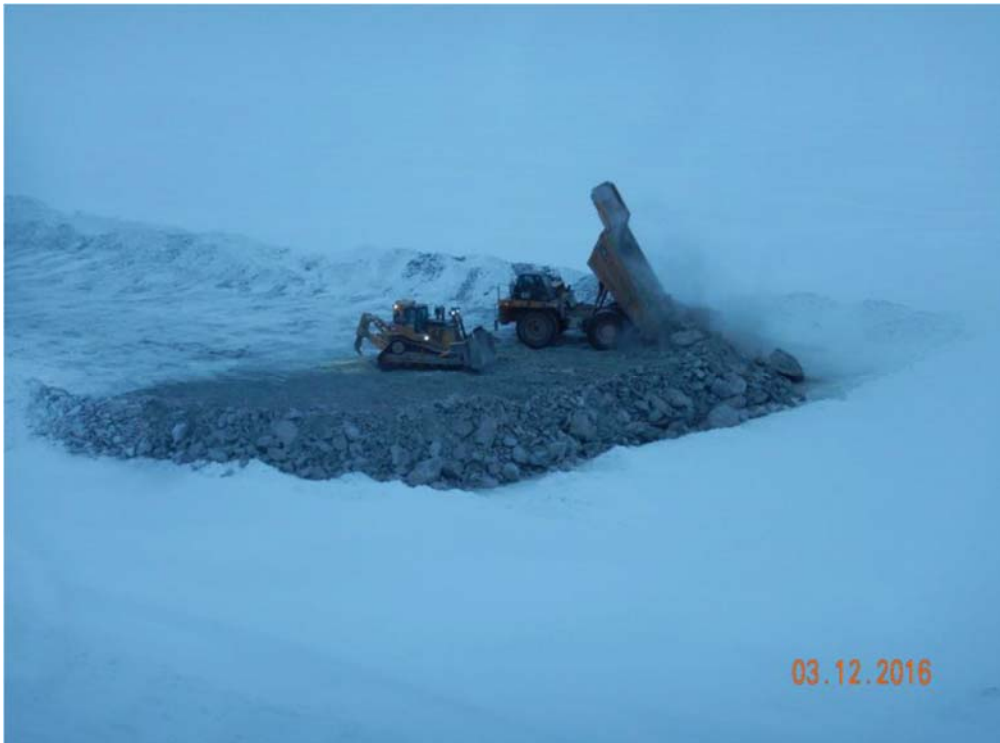
Photo 9: TSF North Cell, NPAG Cover construction, winter 2016
