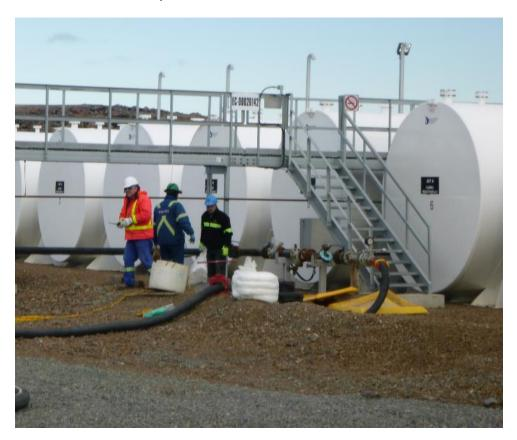
Intertek and AEM crew installing the secondary containment and spill supplies
