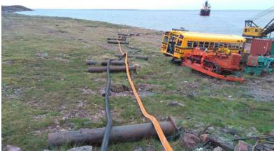
Figure 2: Diesel Transfer - Connection between shipper transfer hoses and Agnico permanent pipeline
