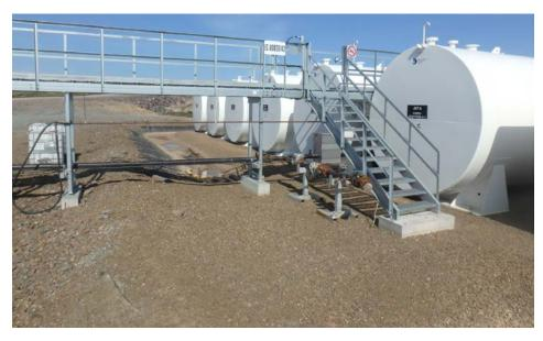
Photo 3: Jet-A Transfer - Connection between shipper transfer hoses and Agnico permanent pipeline
