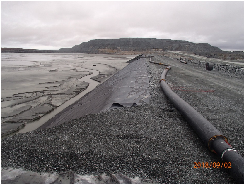
Photograph B7-9 Central Dike and Saddle Dam 5
