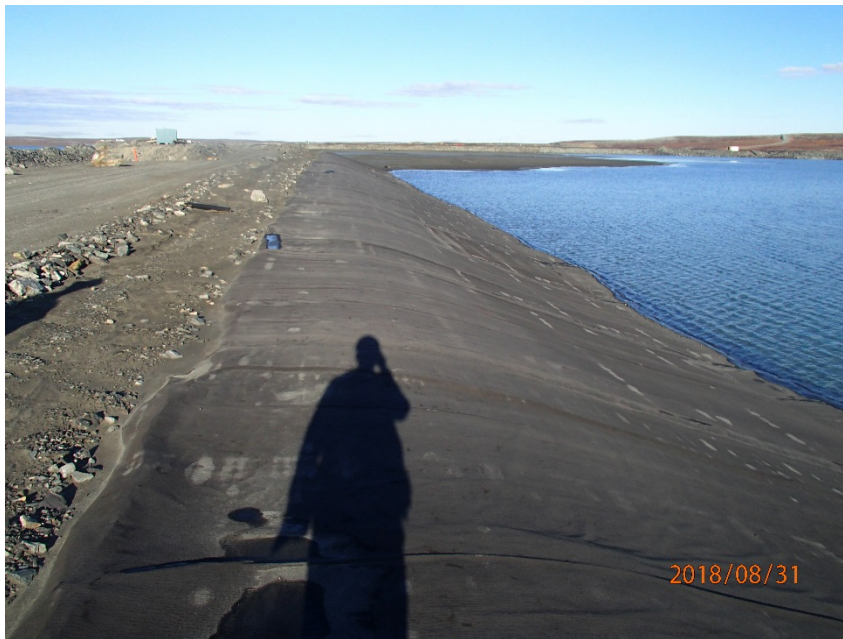
Photograph B4-16 Stormwater Dike
