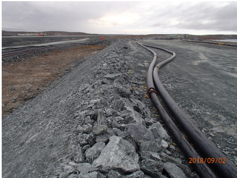
Photograph B7-16 Central Dike and Saddle Dam 5
