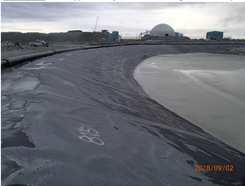
Photograph B7-14 Central Dike and Saddle Dam 5
