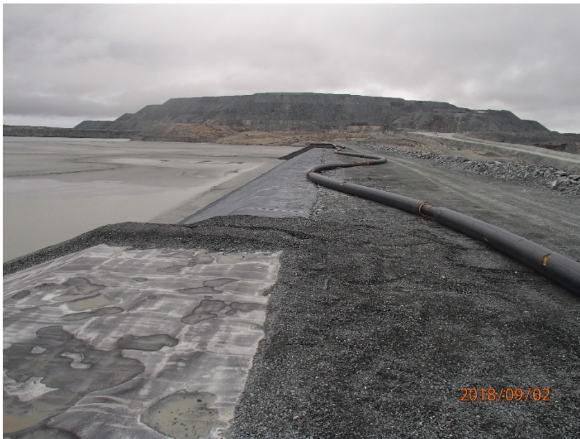
Photograph B7-2 Central Dike and Saddle Dam 5
