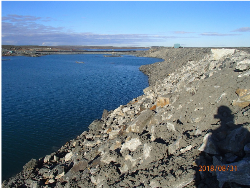
Photograph B4-13 Stormwater Dike
