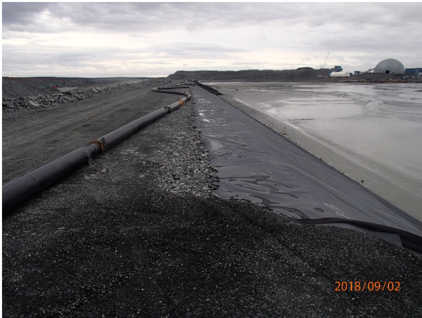
Photograph B7-3 Central Dike and Saddle Dam 5
