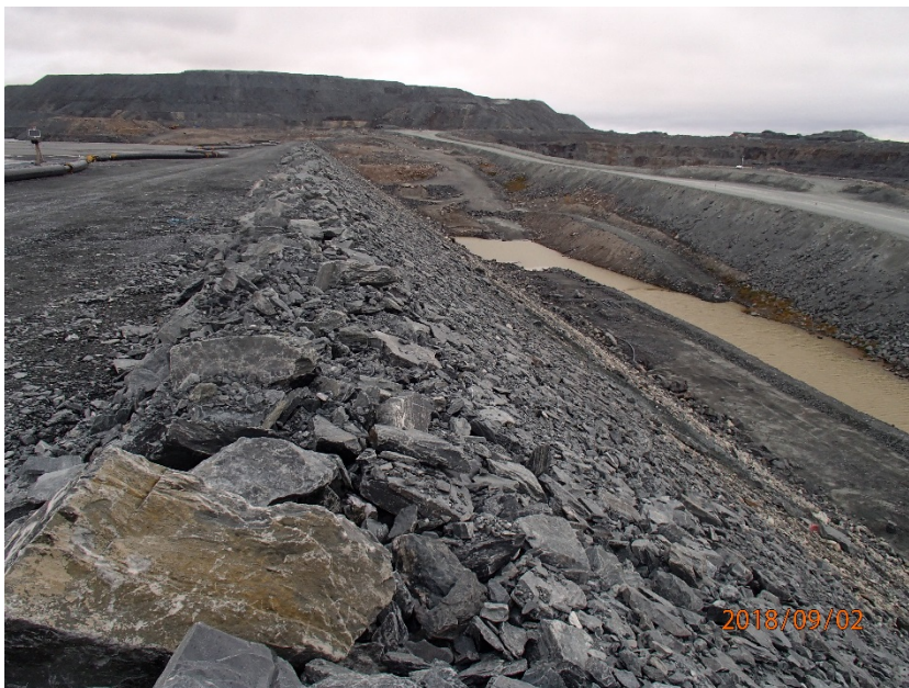
Photograph B7-6 Central Dike and Saddle Dam 5
