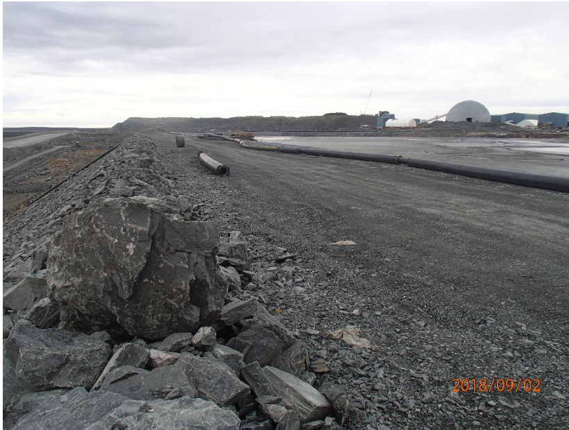
Photograph B7-7 Central Dike and Saddle Dam 5
