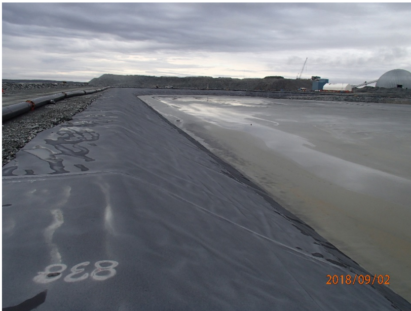
Photograph B7-10 Central Dike and Saddle Dam 5
