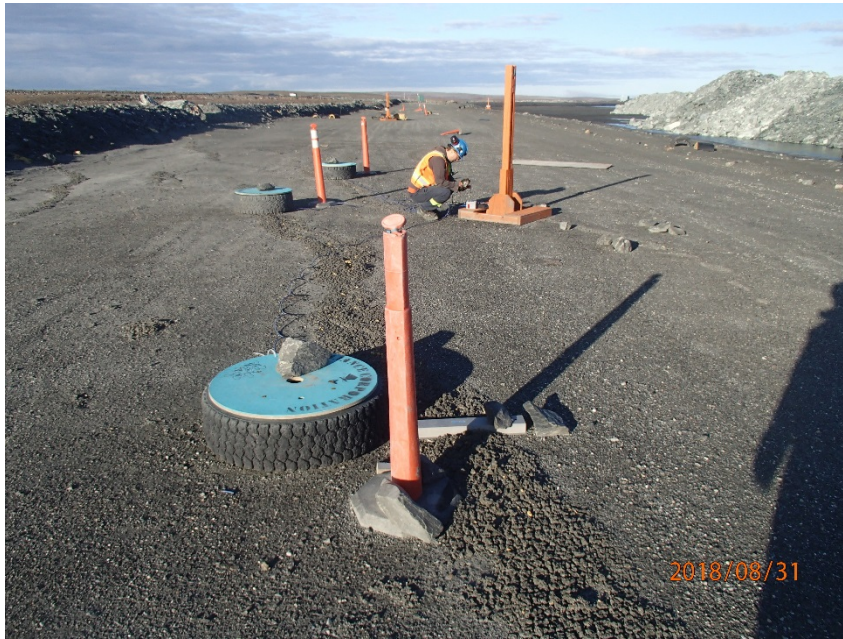
Photograph B4-17 Stormwater Dike
