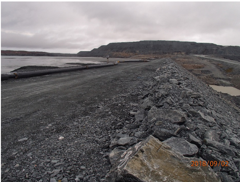
Photograph B7-8 Central Dike and Saddle Dam 5
