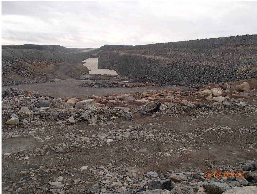
Photograph B7-1 Central Dike and Saddle Dam 5
