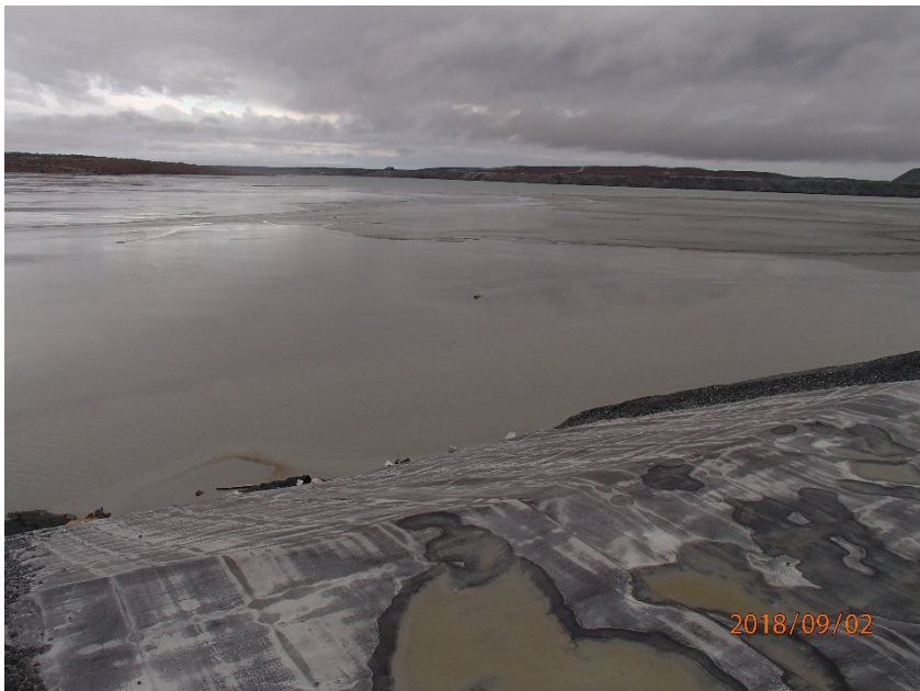
Photograph B7-4 Central Dike and Saddle Dam 5
