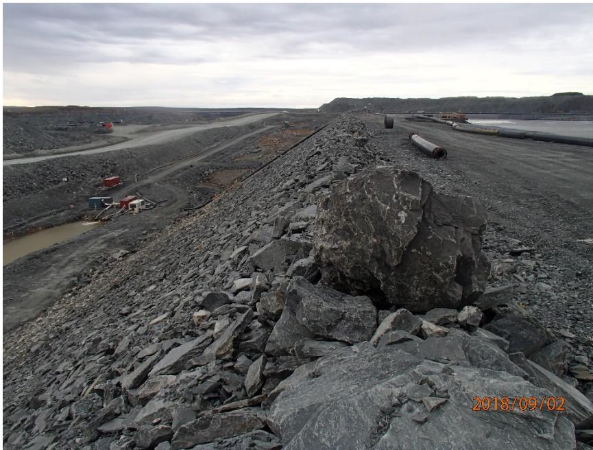
Photograph B7-5 Central Dike and Saddle Dam 5
