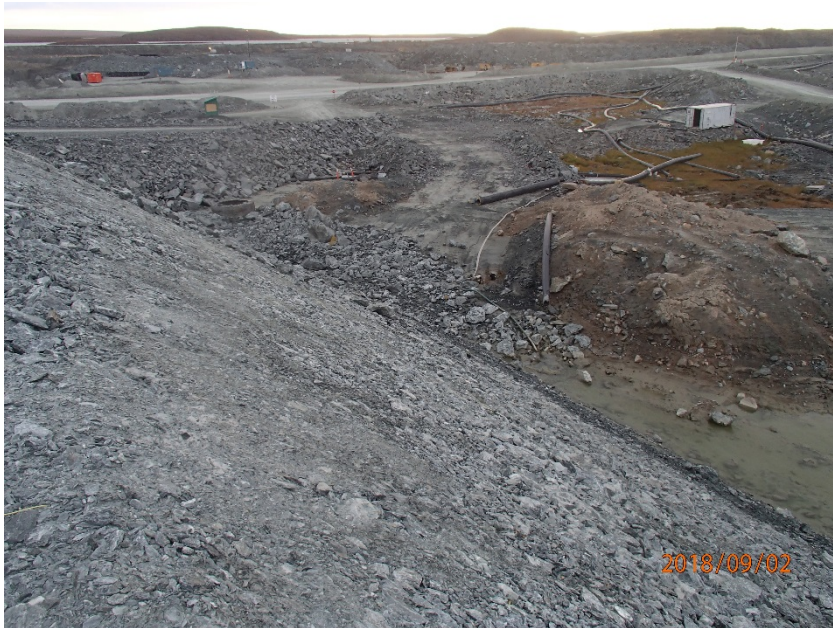
Photograph B7-15 Central Dike and Saddle Dam 5
