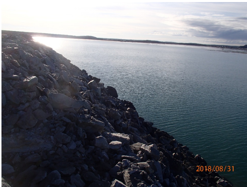
Photograph B4-14 Stormwater Dike
