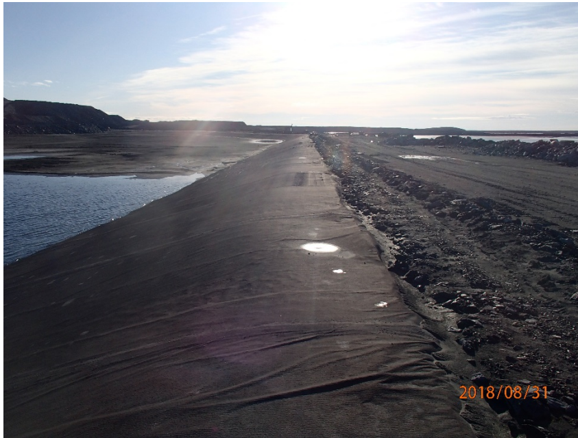
Photograph B4-15 Stormwater Dike
