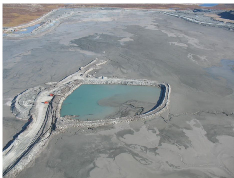
Photo No. 8 Meadowbank. Water collection sump in the North Cell of the TSF
