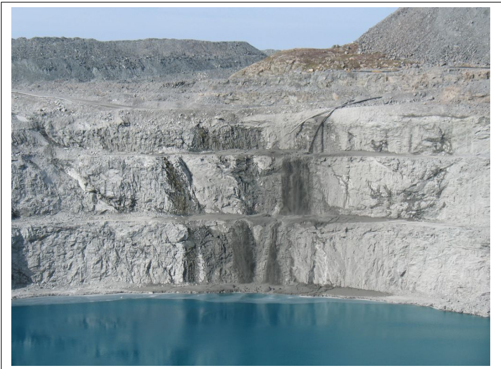
Photo No. 6 Meadowbank, In-Pit deposition of tailings. Pit E
