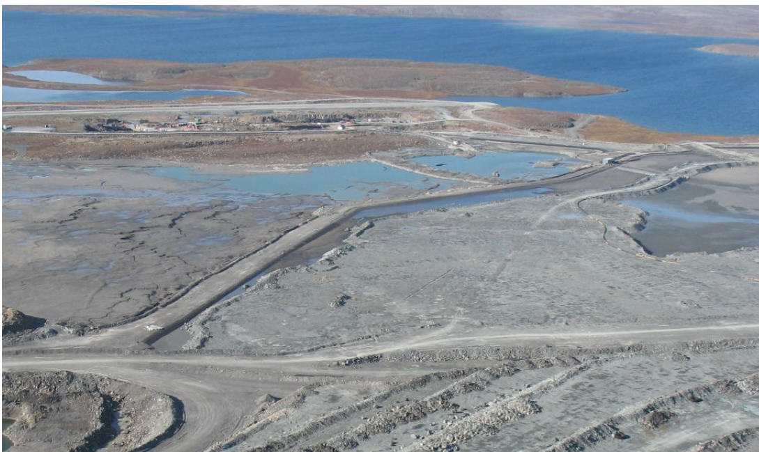
Photo No. 7 Meadowbank. Stormwater Dike and North (right) and South Cells of the TSF
