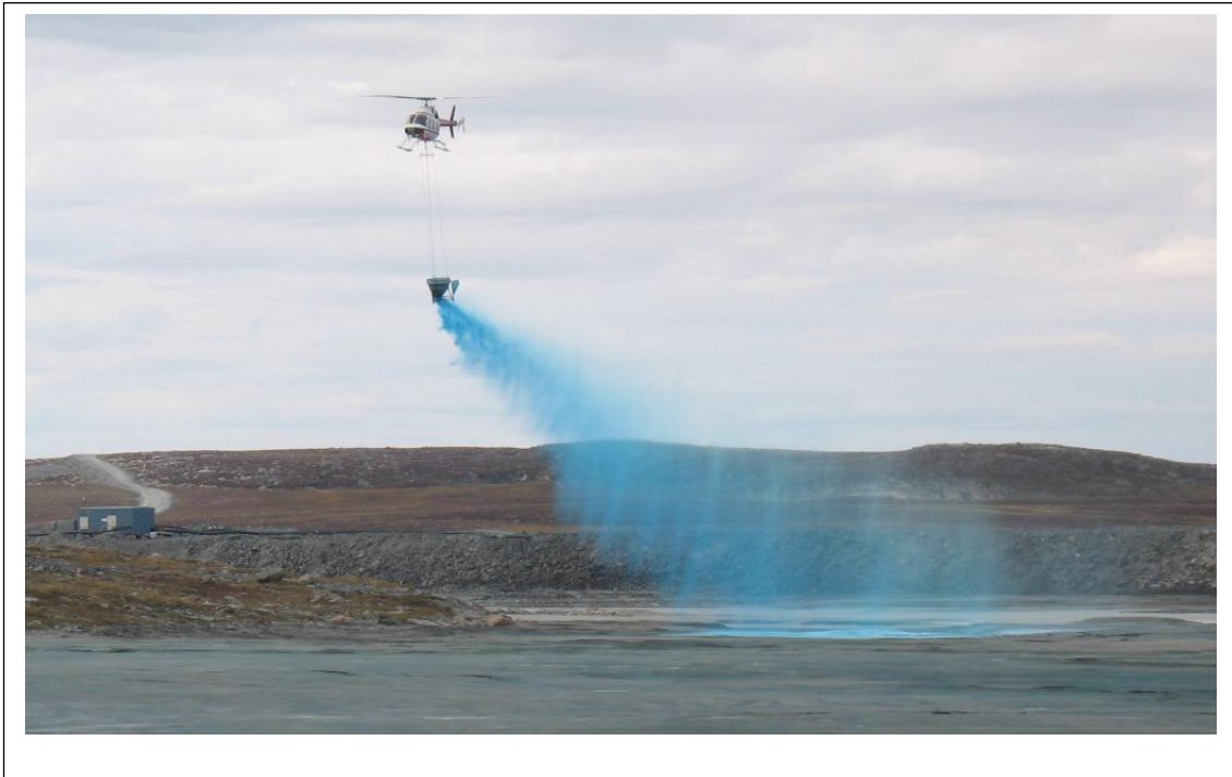
Photo No. 3 Meadowbank TSF, sealant spreading
