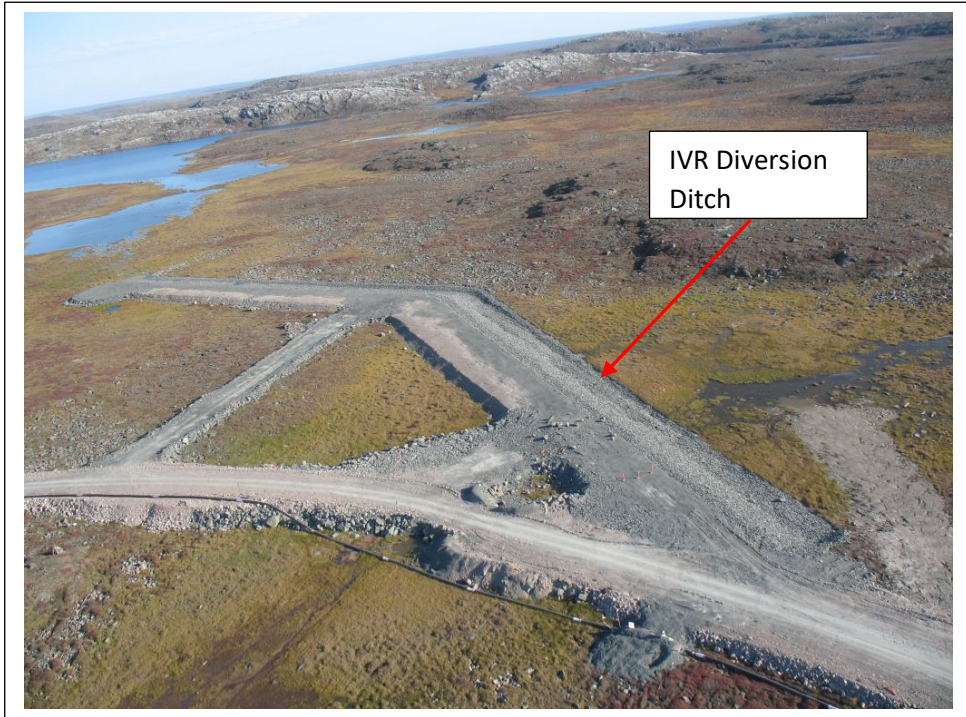
Photo No. 15 Amaruq. IVR Diversion Ditch and retaining berm
