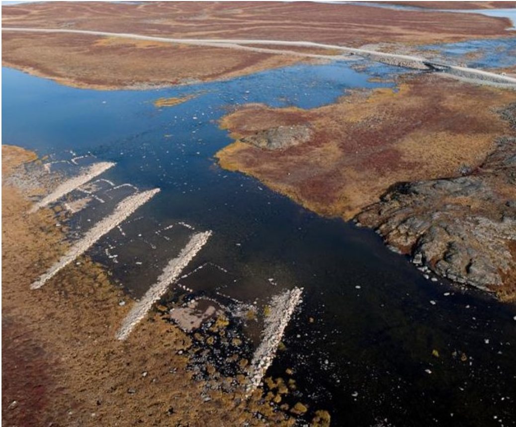
Figure 1. Arctic Grayling spawning pads constructed at Meadowbank all weather road crossing R02.
