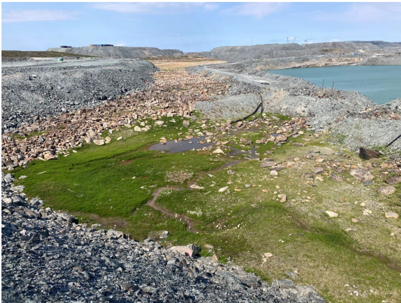
Photograph A3-14 Bay Goose Dike
