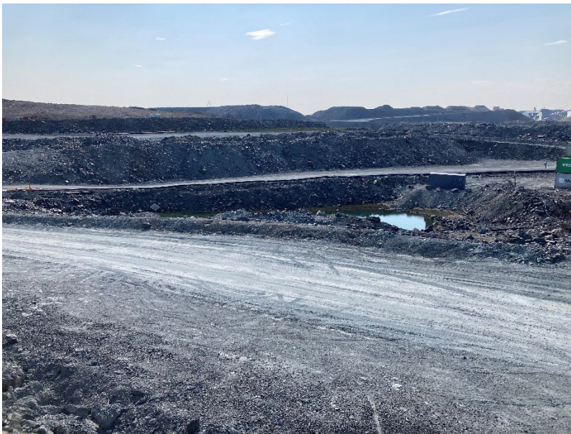
Photograph A1-14 East Dike
