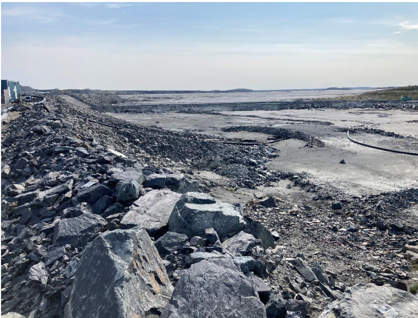
Photograph B4-12 Stormwater Dike
