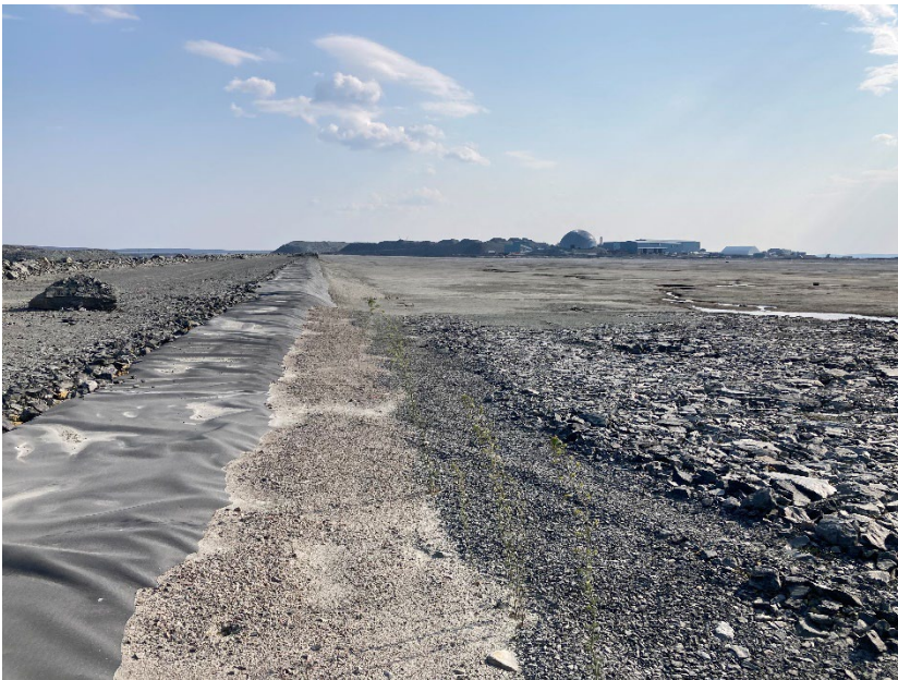
Photograph B7-12 Central Dike and Saddle Dam 5
