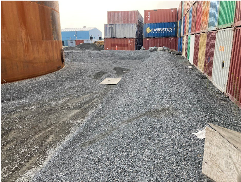
Photograph G2-03 Meadowbank Tank Farm
