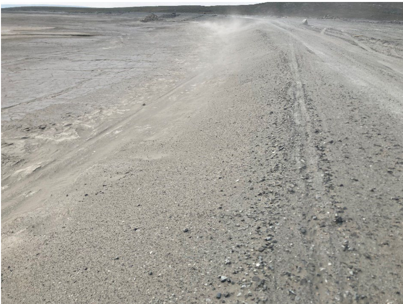
Photograph B1-06 Tailings Storage Facility
