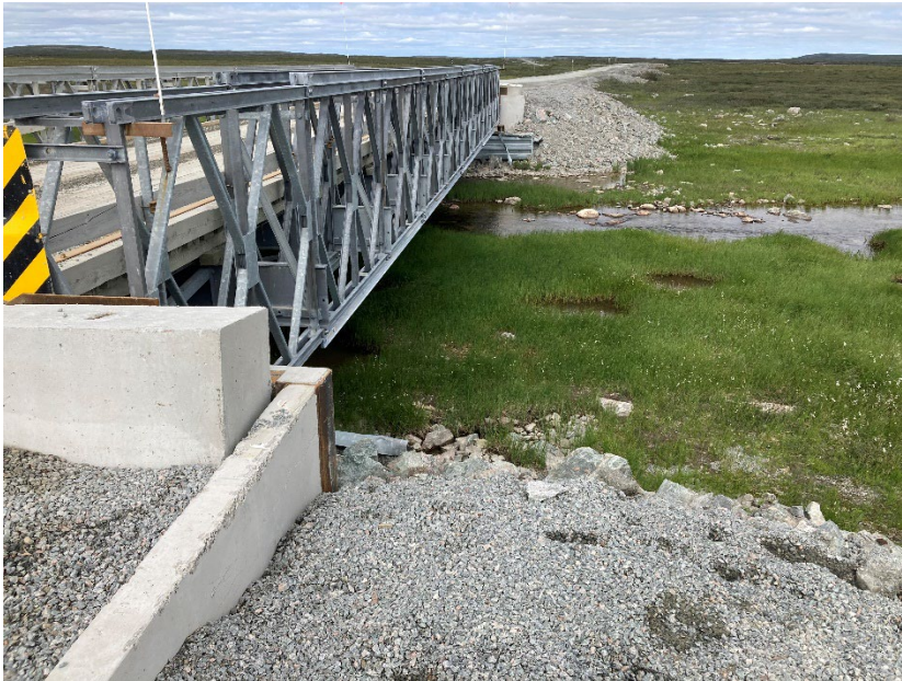
Photograph D3-3 Bridges 2 – R05 km 17+600
