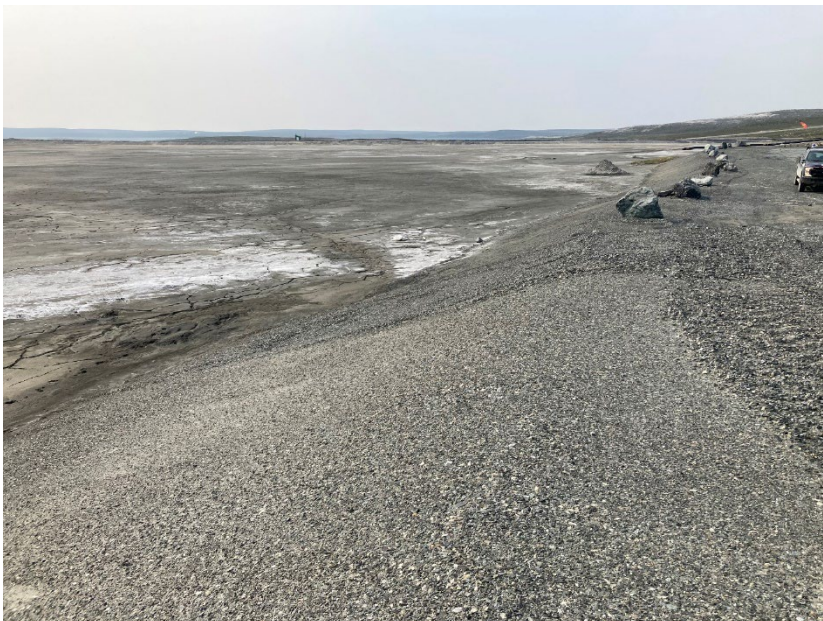
Photograph B1-02 Tailings Storage Facility
