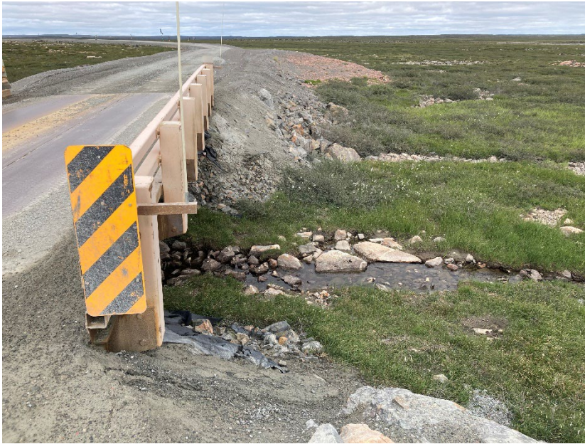
Photograph D3-13 Bridges 7 – R16 km 73+800
