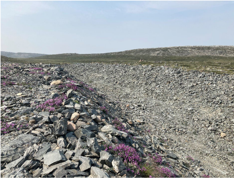
Photograph H2-09 Diversion Ditch and its Sediment and Erosion Protection Structure
