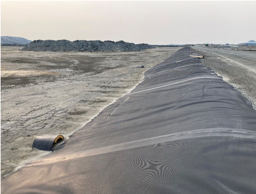
Photograph B3-05 Saddle Dam 2
