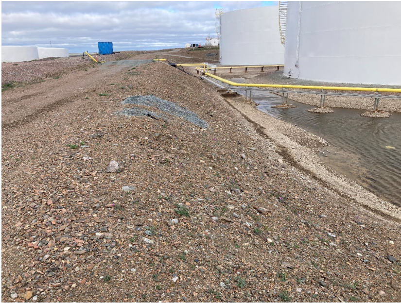
Photograph G1-23 Baker Lake Tank Farm
