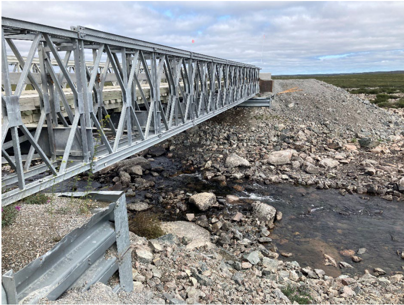
Photograph D3-1 Bridges 1 – R02 km 8+750
