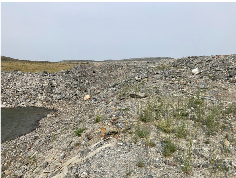
Photograph H2-20 Diversion Ditch and its Sediment and Erosion Protection Structure
