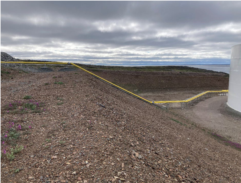
Photograph G1-21 Baker Lake Tank Farm
