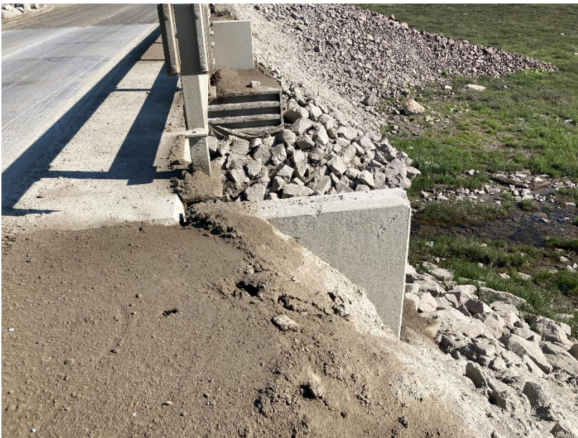
Photograph E2-8 Bridges 4 – km 136+000
