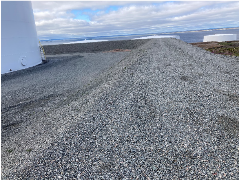
Photograph G1-27 Baker Lake Tank Farm
