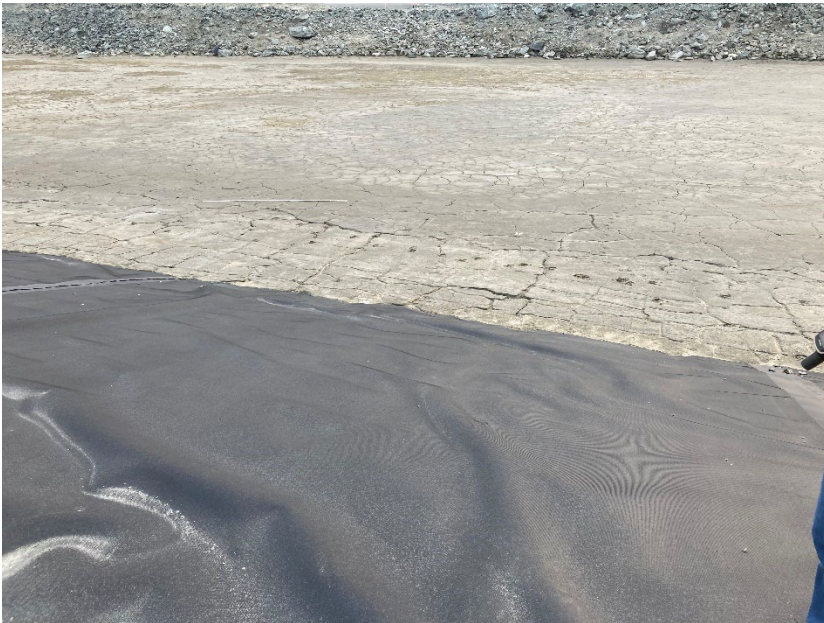
Photograph B3-02 Saddle Dam 2
