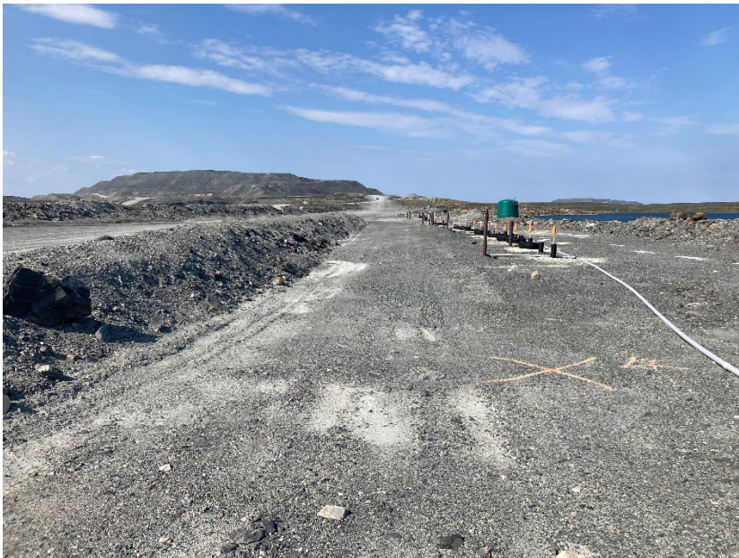
Photograph A1-06 East Dike
