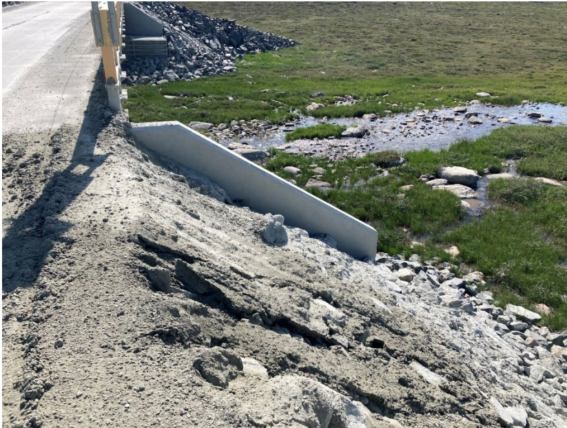
Photograph E2-20 Bridges 9 – km 160+800
