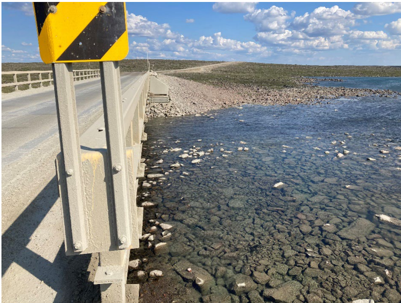
Photograph E2-11 Bridges 5 – km 139+900
