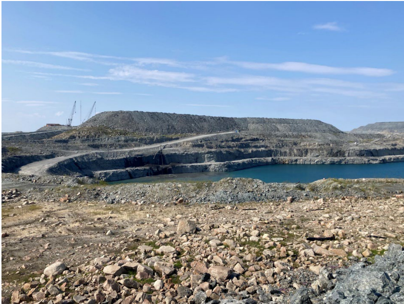
Photograph A3-33 Bay Goose Dike
