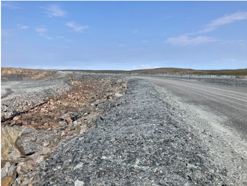
Photograph A3-39 Bay Goose Dike
