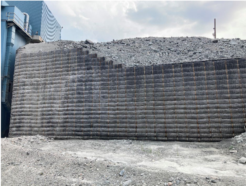
Photograph H6-01 Meadowbank Crusher Retaining Wall
