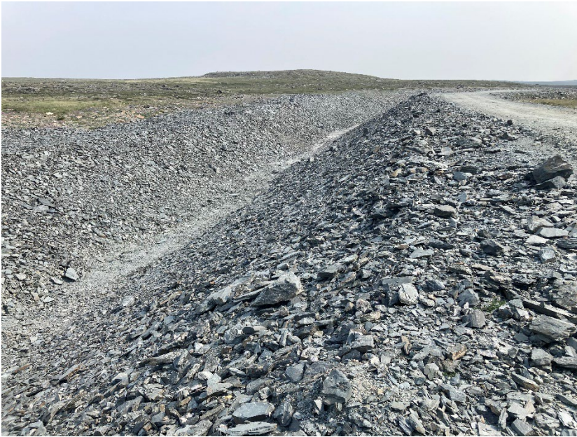
Photograph H2-07 Diversion Ditch and its Sediment and Erosion Protection Structure
