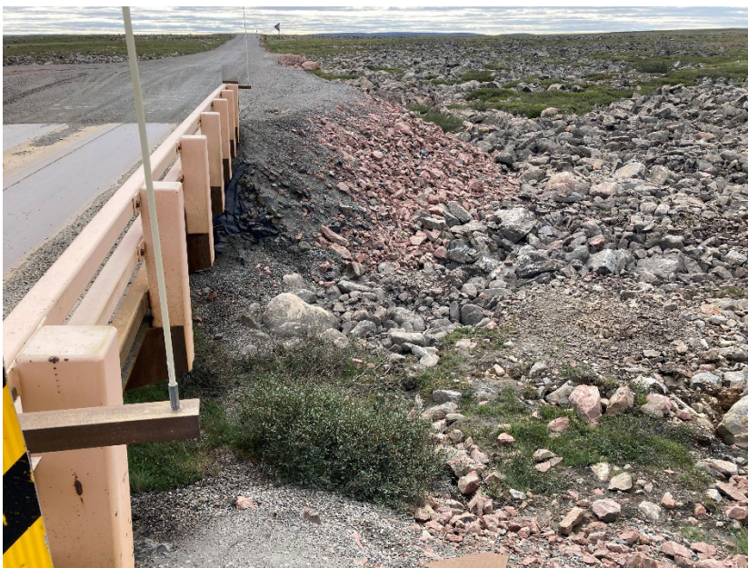
Photograph D3-16 Bridges 8 – R18 km 79+500
