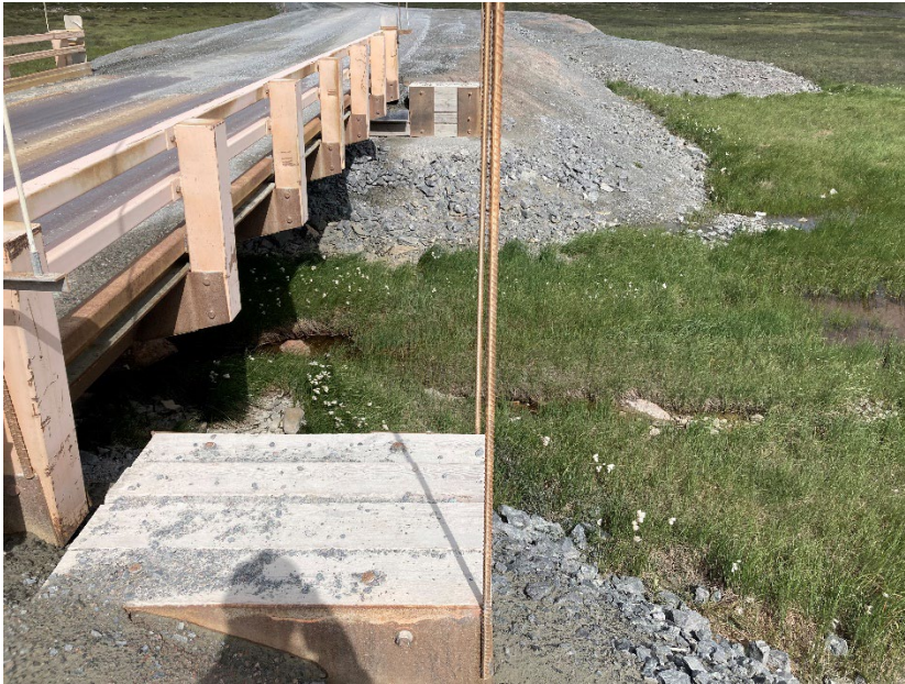
Photograph D3-9 Bridges 5 – R13 km 62+060
