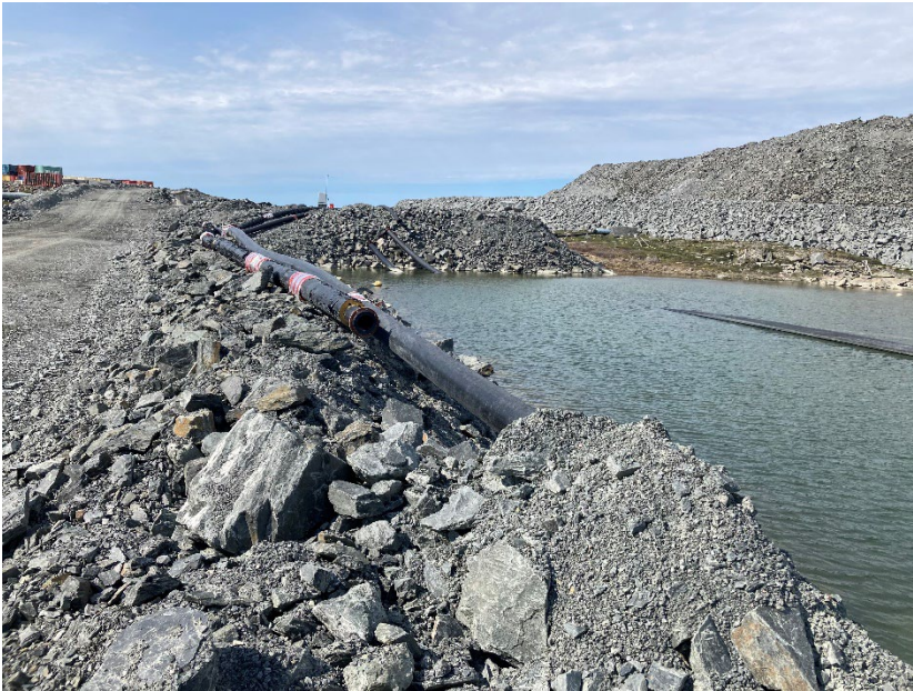
Photograph H8-01 IVR Attenuation Pond Jetty
