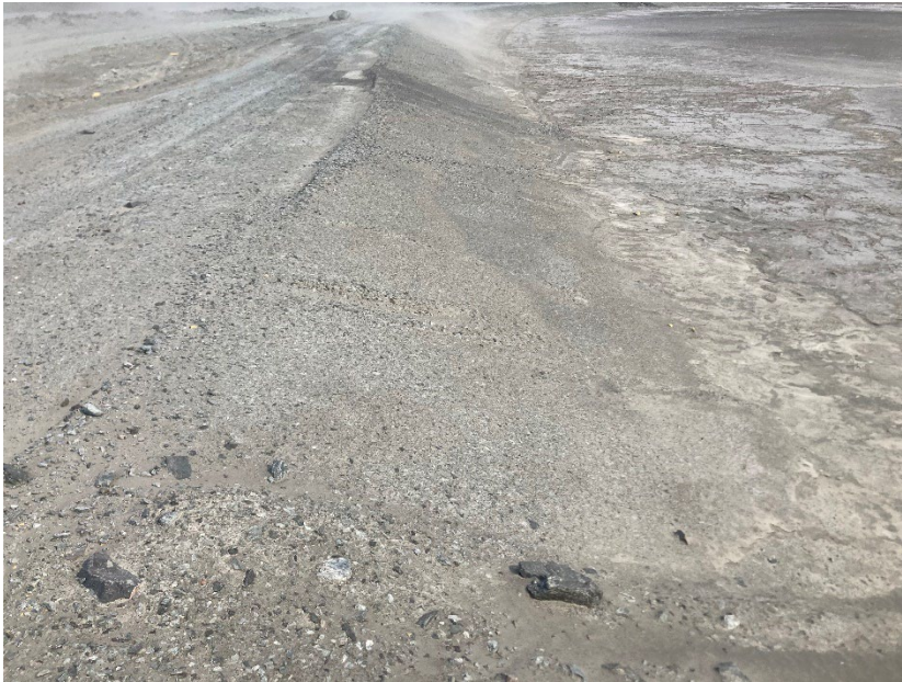
Photograph B1-07 Tailings Storage Facility
