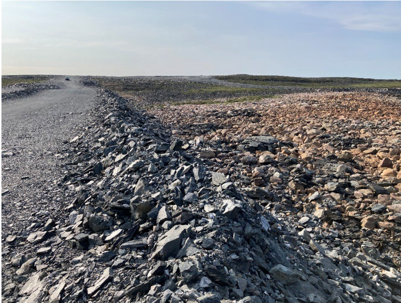
Photograph A4-5 Vault Dike
