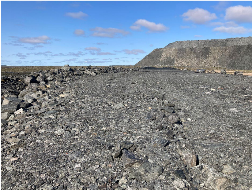
Photograph A7-3 WRSF Dike
