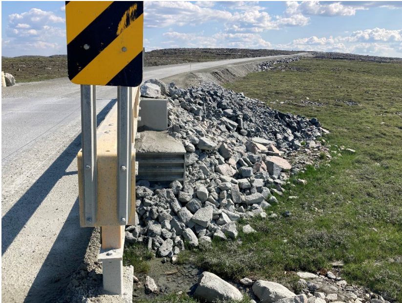
Photograph E2-18 Bridges 8 – km 159+500
