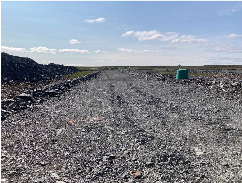
Photograph A8-3 Mammoth Dike
