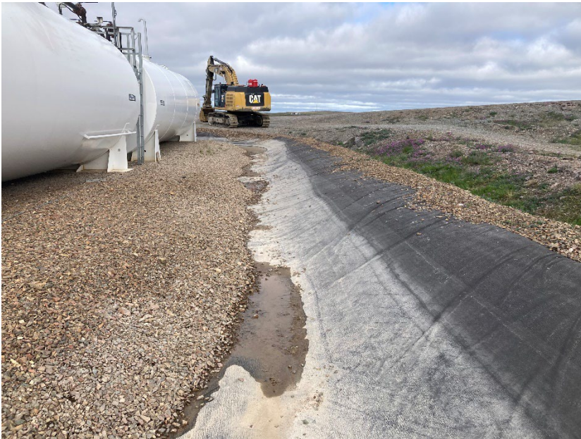
Photograph G1-18 Baker Lake Tank Farm
