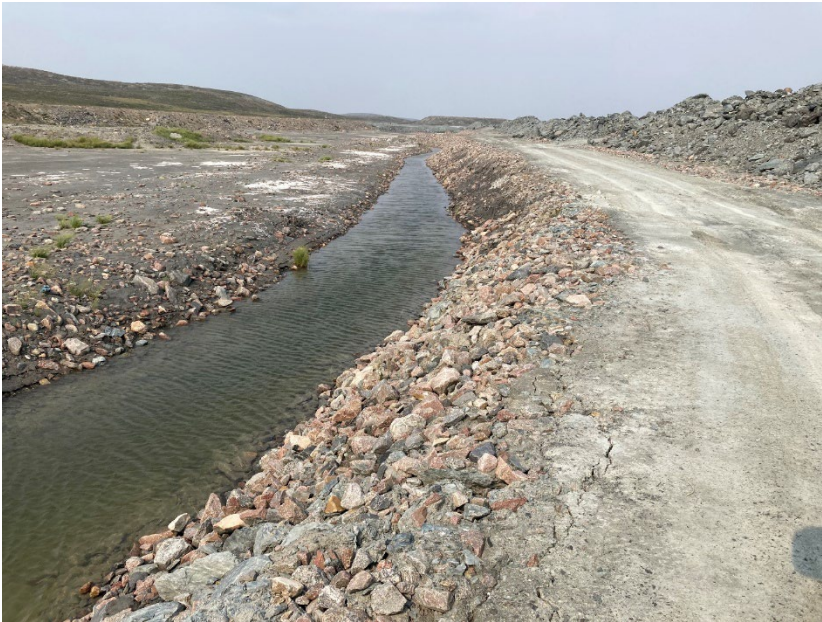
Photograph B1-03 Tailings Storage Facility
