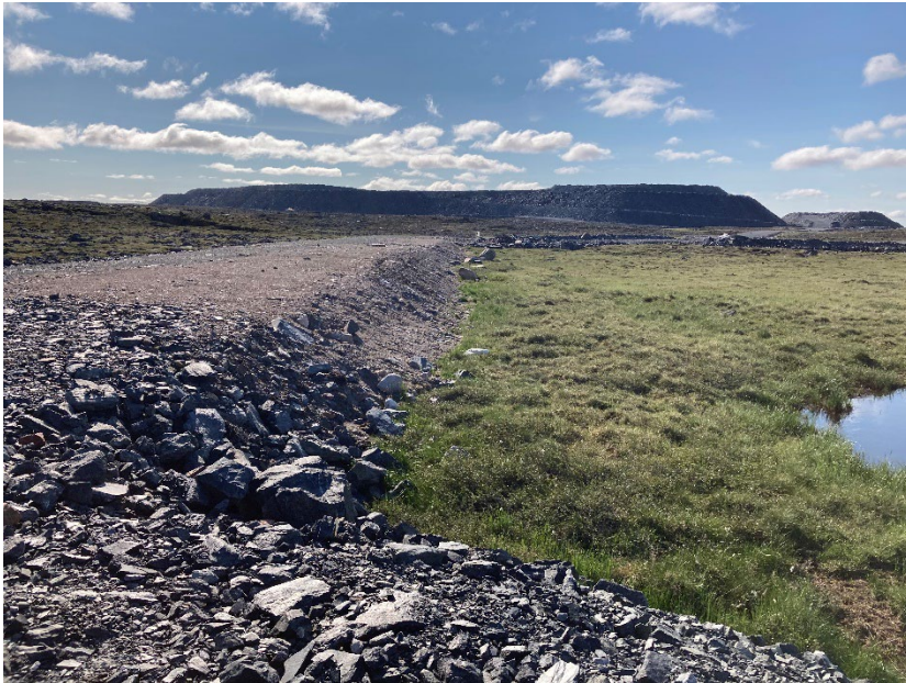
Photograph H13-7 IVR Diversion Channel
