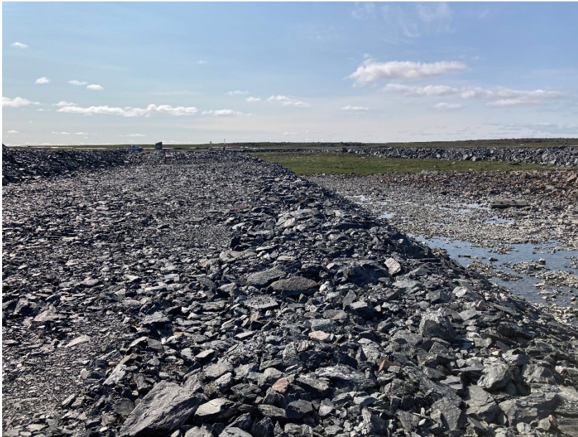
Photograph A8-7 Mammoth Dike
