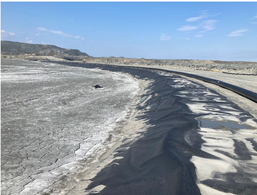
Photograph B7-02 Central Dike and Saddle Dam 5
