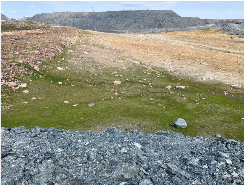
Photograph A3-04 Bay Goose Dike
