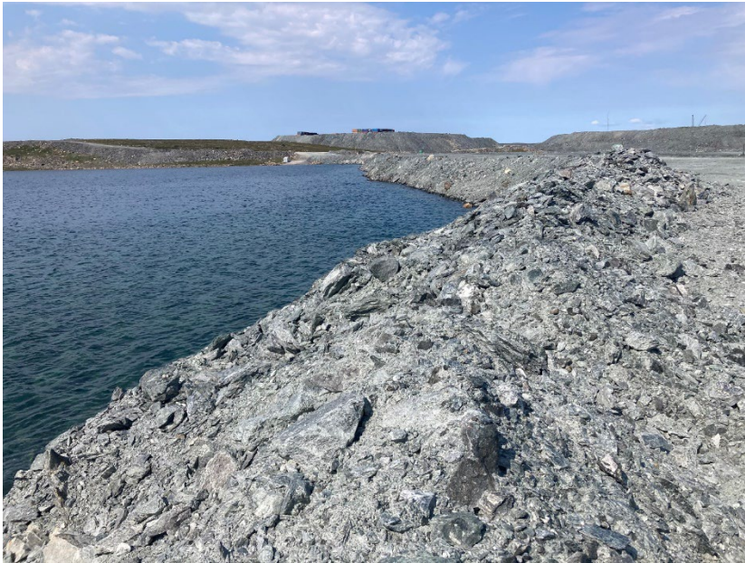
Photograph A3-11 Bay Goose Dike
