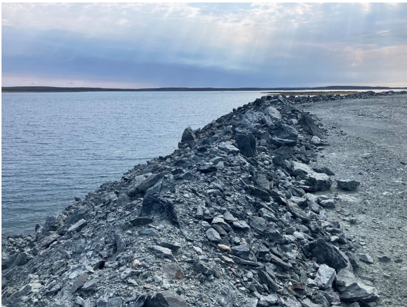
Photograph A3-28 Bay Goose Dike
