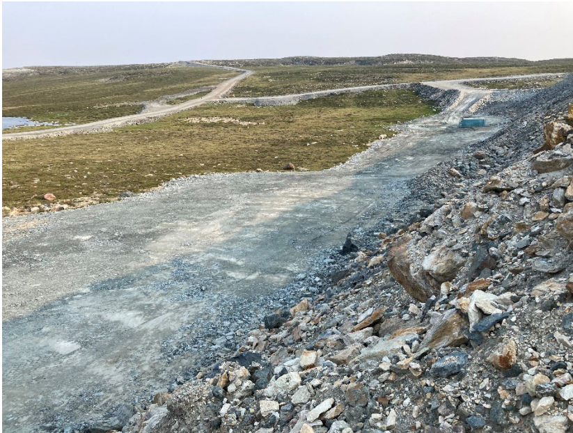
Photograph B2-11 Saddle Dam 1
