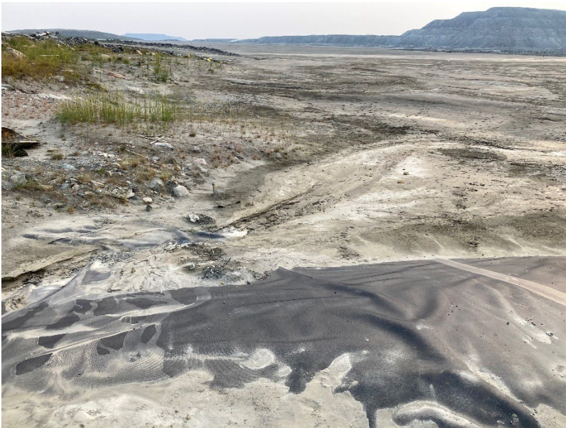
Photograph B3-06 Saddle Dam 2
