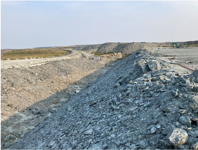
Photograph B5-01 Saddle Dam 3
