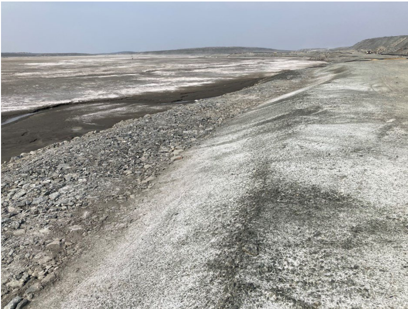
Photograph B1-13 Tailings Storage Facility
