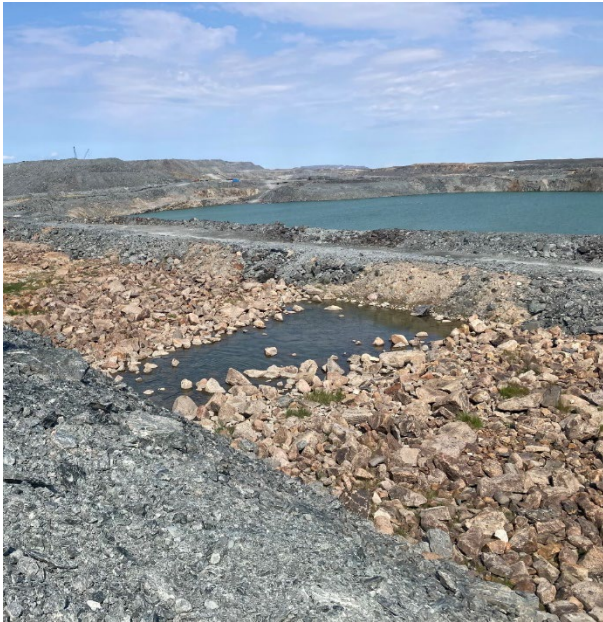
Photograph A3-09 Bay Goose Dike
