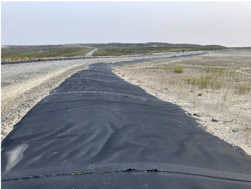
Photograph B2-02 Saddle Dam 1
