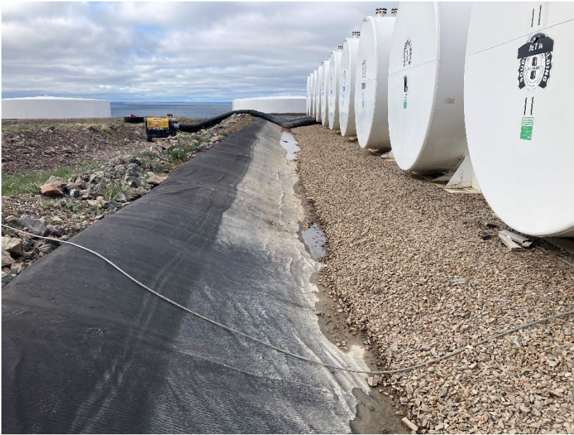
Photograph G1-17 Baker Lake Tank Farm
