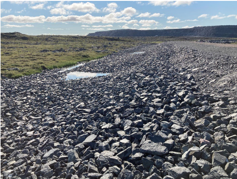
Photograph H13-6 IVR Diversion Channel
