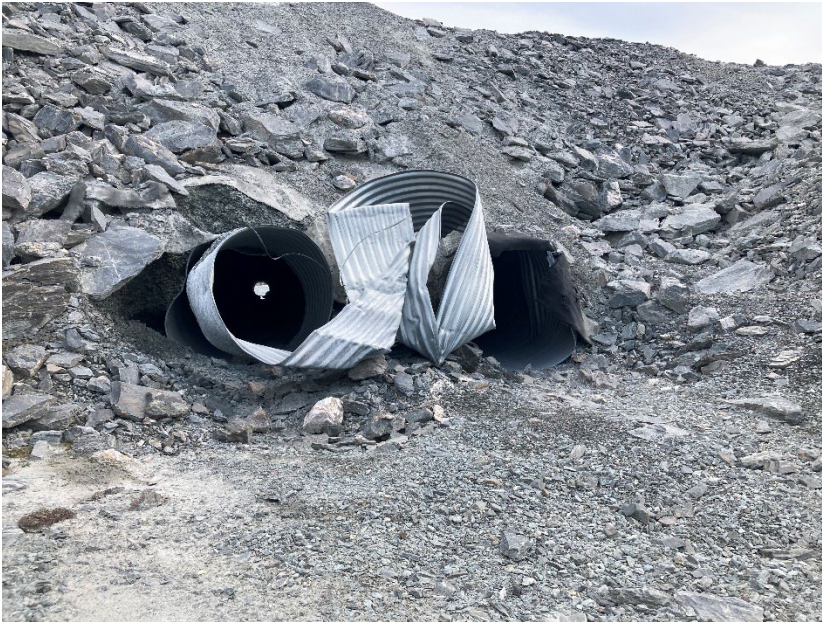
Photograph H2-03 Diversion Ditch and its Sediment and Erosion Protection Structure
