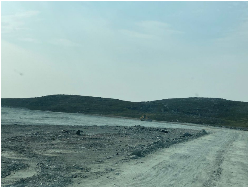
Photograph H2-14 Diversion Ditch and its Sediment and Erosion Protection Structure
