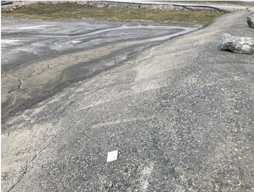
Photograph B1-01 Tailings Storage Facility
