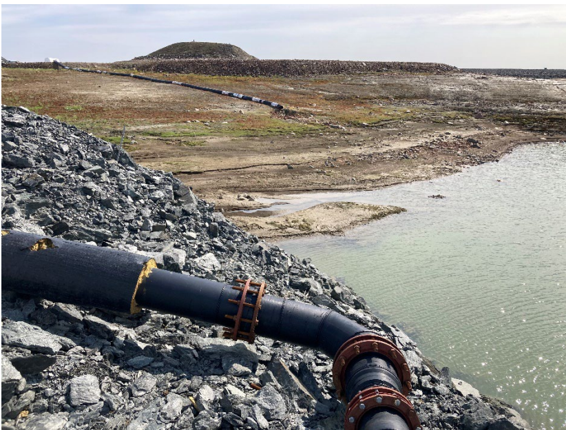
Photograph H7-02 Whale Tail Mine Site Attenuation Pond Jetty
