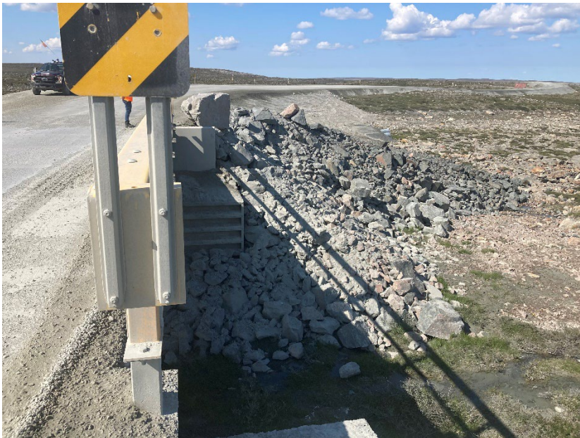
Photograph E2-17 Bridges 8 – km 159+500
