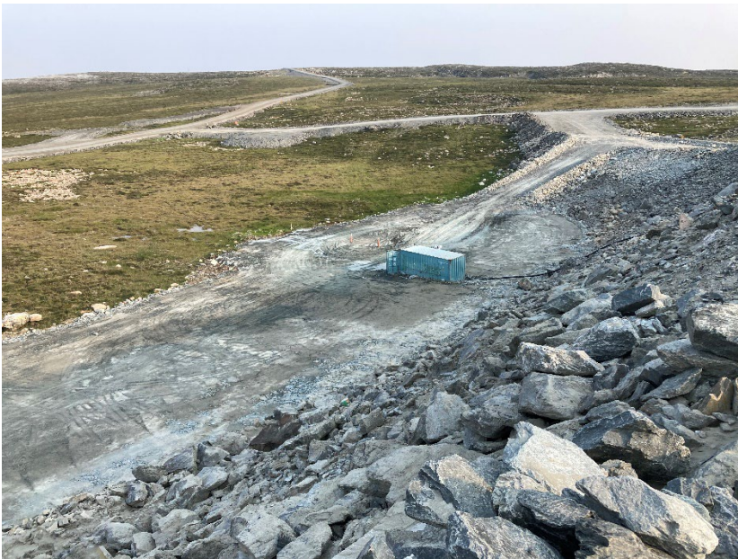
Photograph B2-10 Saddle Dam 1
