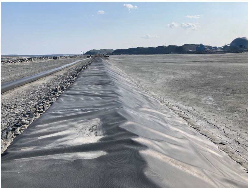
Photograph B7-06 Central Dike and Saddle Dam 5
