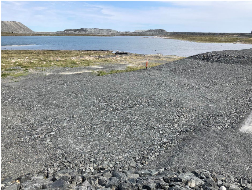
Photograph A6-3 IVR Dike D-1
