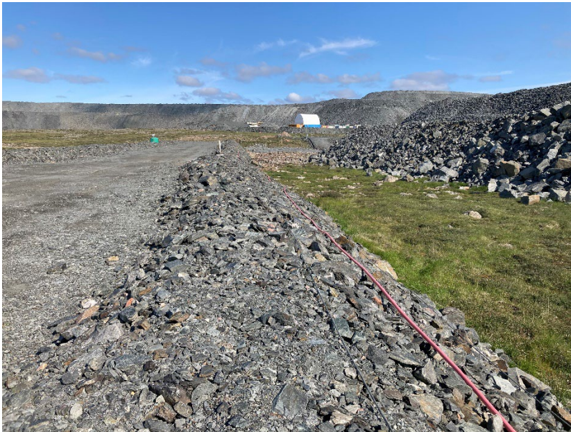
Photograph A8-2 Mammoth Dike
