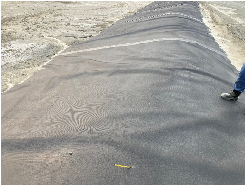
Photograph B3-03 Saddle Dam 2
