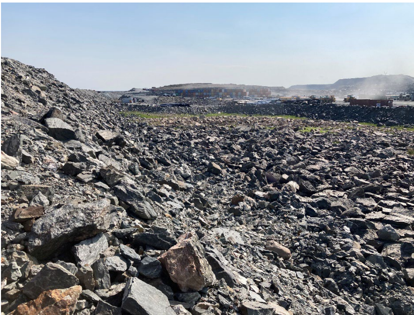
Photograph A1-10 East Dike
