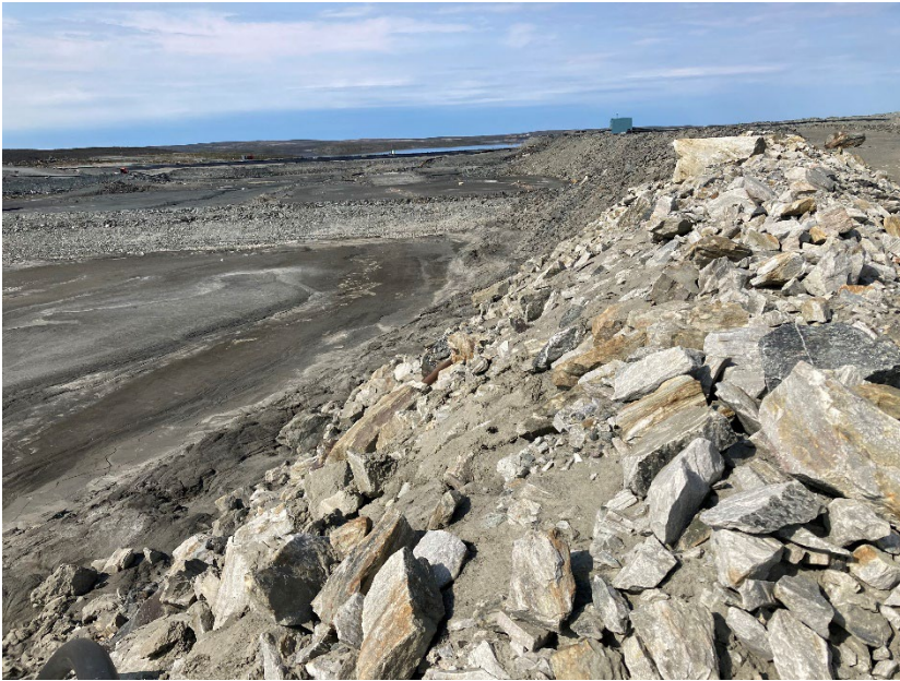
Photograph B4-13 Stormwater Dike
