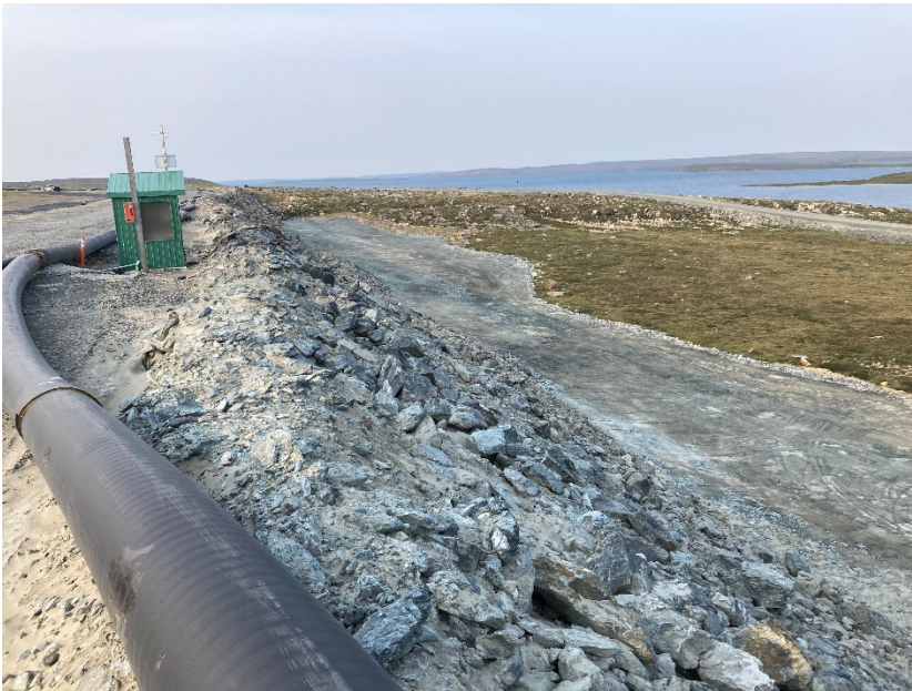
Photograph B2-08 Saddle Dam 1
