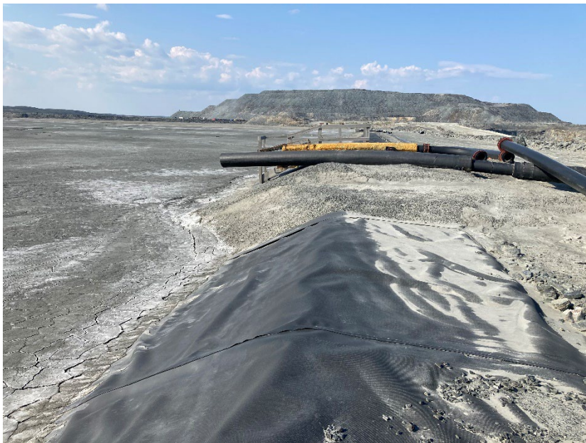
Photograph B7-04 Central Dike and Saddle Dam 5
