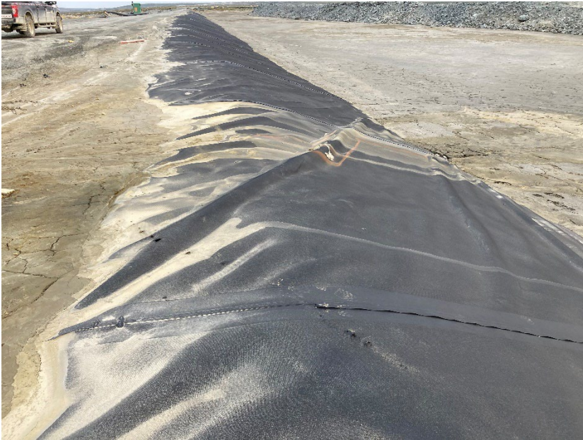
Photograph B3-01 Saddle Dam 2
