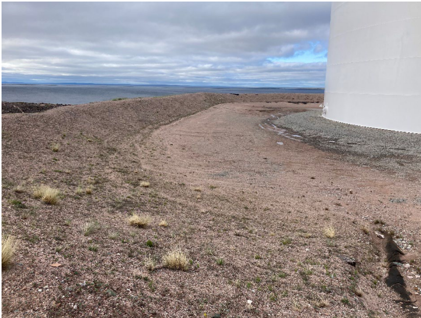
Photograph G1-10 Baker Lake Tank Farm
