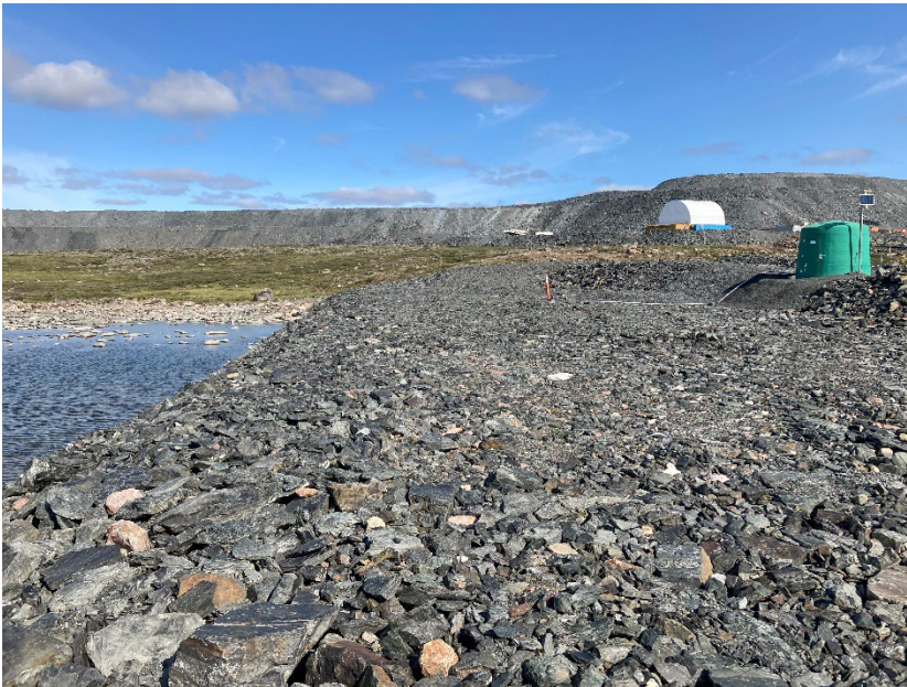
Photograph A8-6 Mammoth Dike
