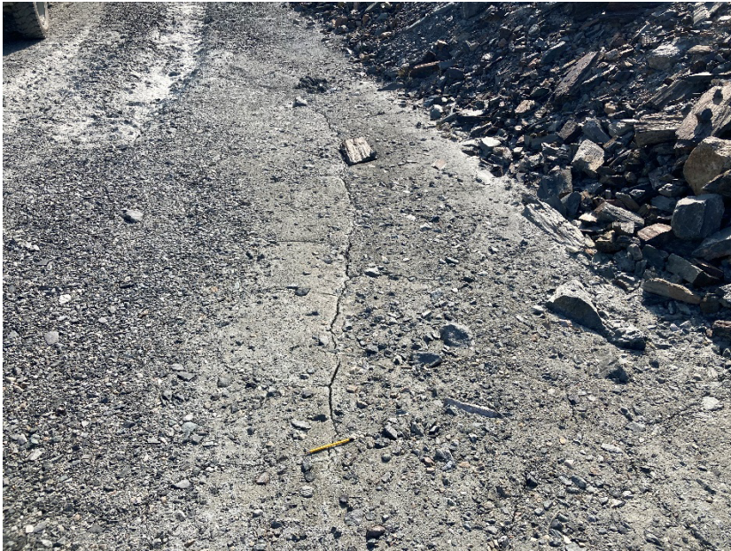
Photograph A1-15 East Dike
