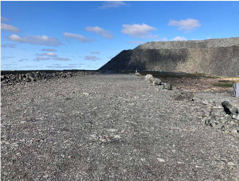
Photograph A7-6 WRSF Dike
