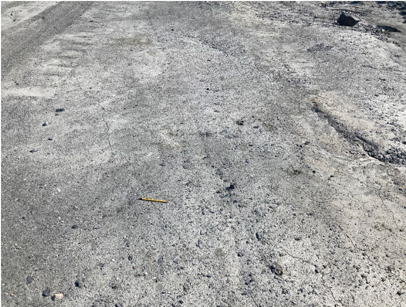
Photograph B4-14 Stormwater Dike
