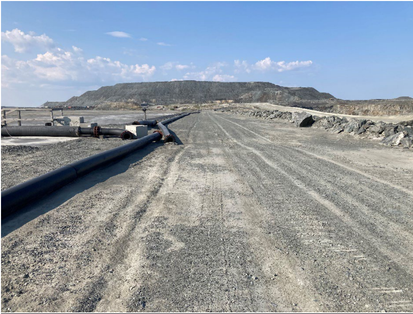
Photograph B7-09 Central Dike and Saddle Dam 5
