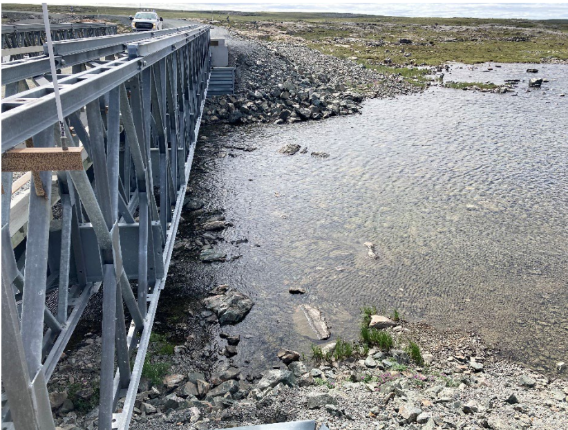
Photograph D3-6 Bridges 3 – R06 km 23+100
