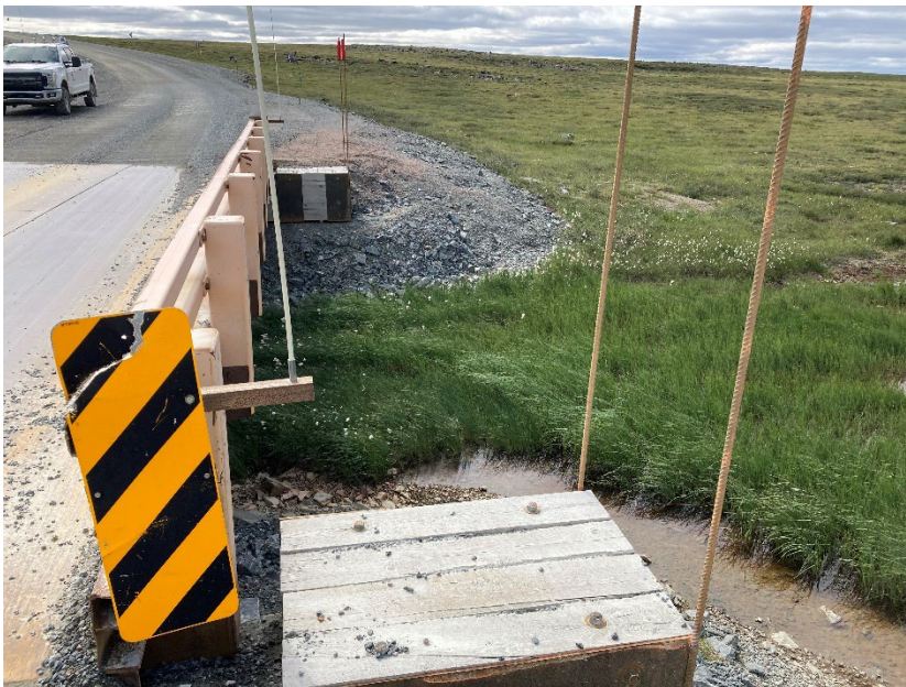
Photograph D3-10 Bridges 5 – R13 km 62+060
