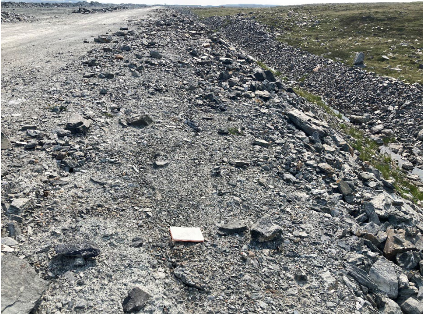
Photograph H2-19 Diversion Ditch and its Sediment and Erosion Protection Structure
