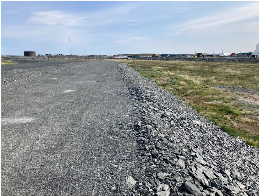
Photograph A6-10 IVR Dike D-1
