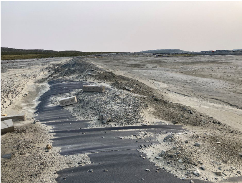
Photograph B2-04 Saddle Dam 1
