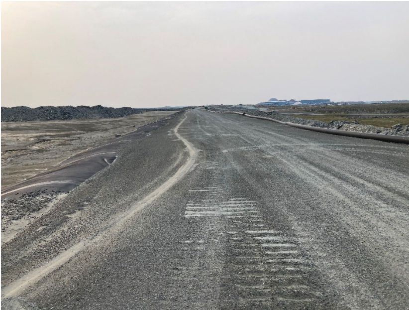
Photograph B3-07 Saddle Dam 2
