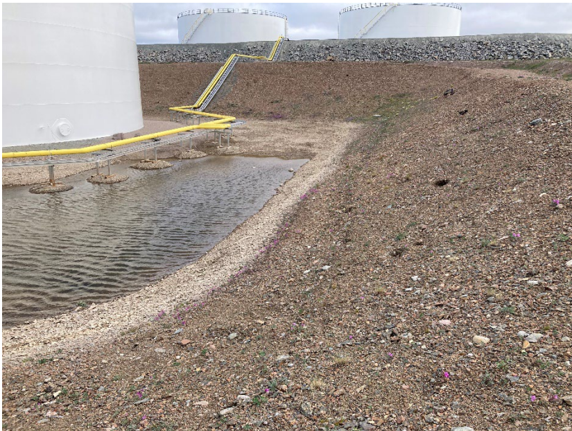
Photograph G1-24 Baker Lake Tank Farm
