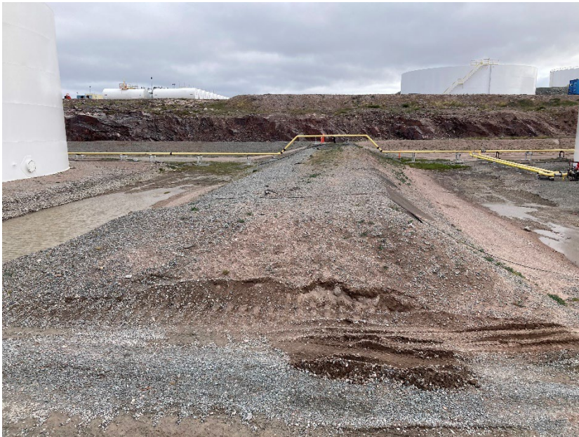
Photograph G1-06 Baker Lake Tank Farm
