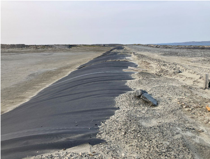
Photograph B2-03 Saddle Dam 1
