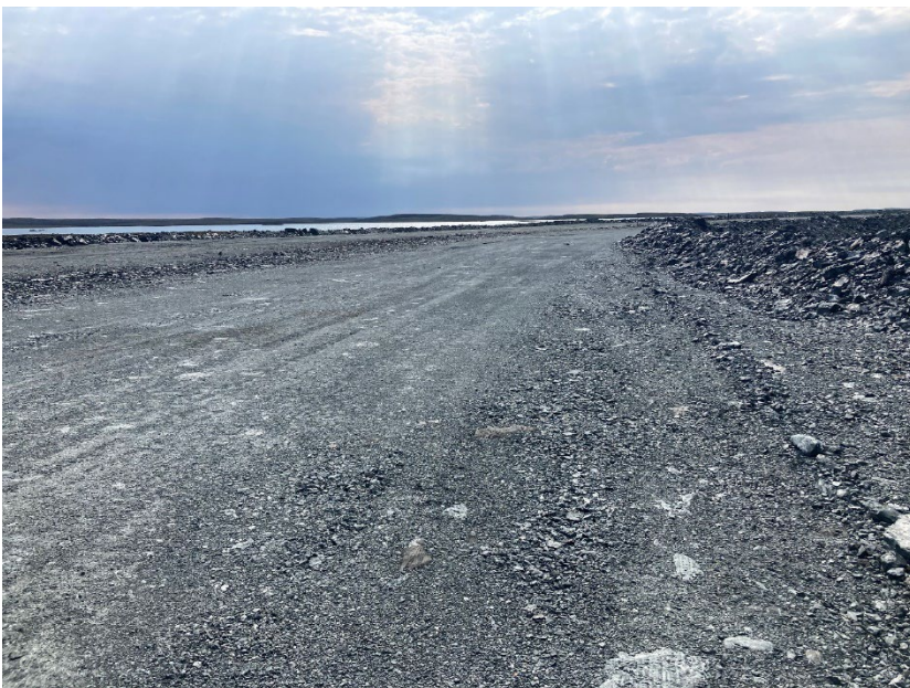
Photograph A3-20 Bay Goose Dike
