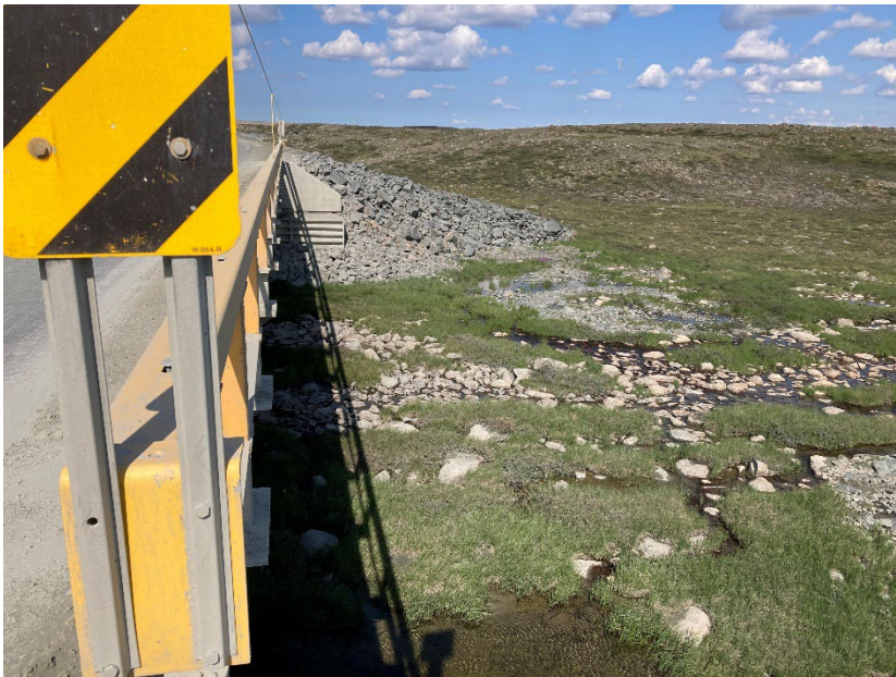
Photograph E2-19 Bridges 9 – km 160+800
