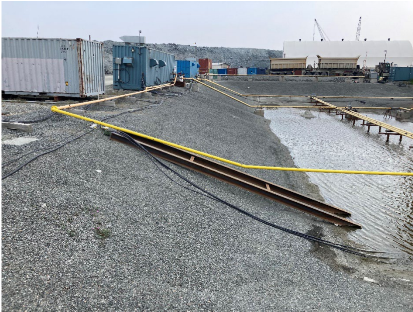
Photograph G2-01 Meadowbank Tank Farm
