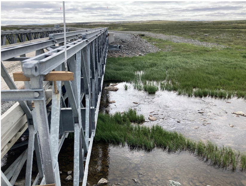
Photograph D3-4 Bridges 2 – R05 km 17+600
