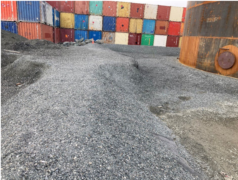
Photograph G2-05 Meadowbank Tank Farm
