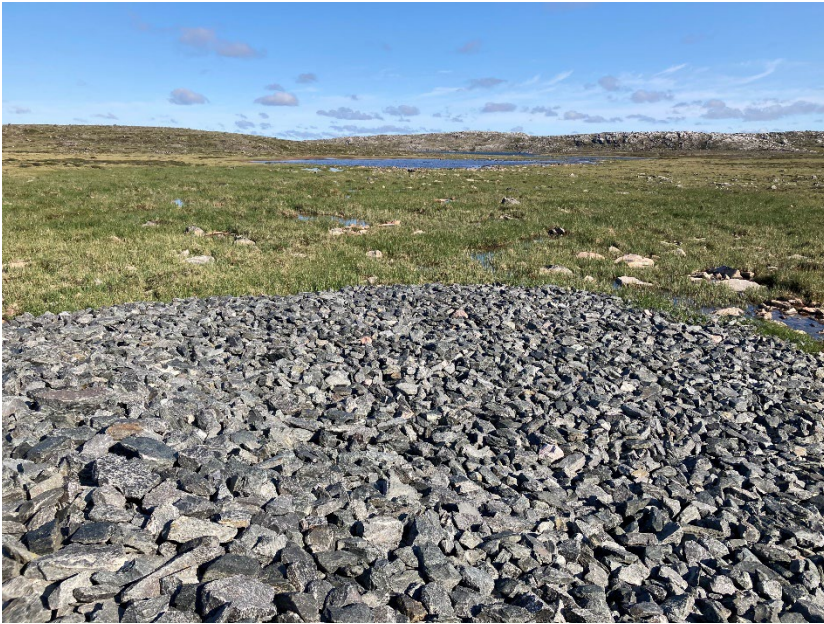
Photograph H13-5 IVR Diversion Channel
