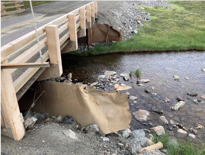
Photograph D3-17 Bridges 9 – R19 km 83+150
