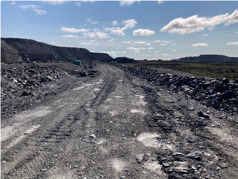
Photograph A7-9 WRSF Dike
