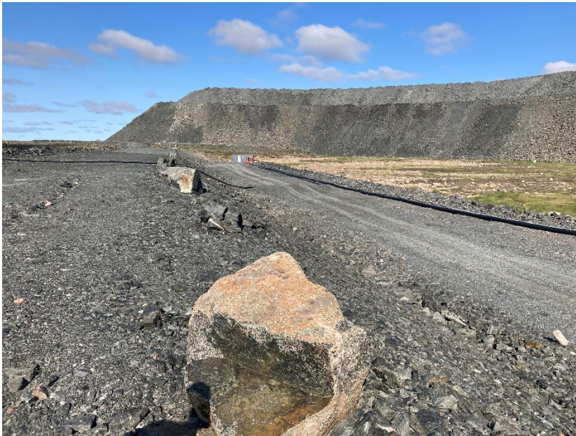
Photograph A7-4 WRSF Dike
