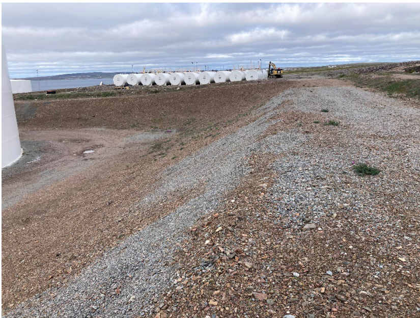
Photograph G1-20 Baker Lake Tank Farm
