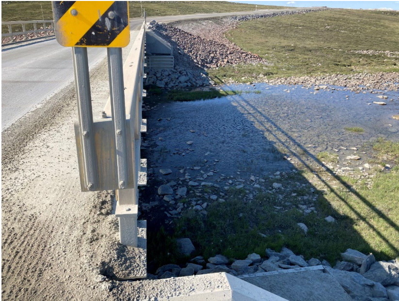
Photograph E2-6 Bridges 3 – km 132+000
