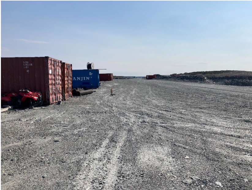
Photograph A1-05 East Dike
