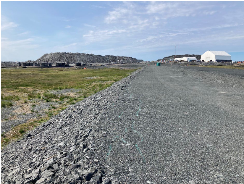
Photograph A6-18 IVR Dike D-1
