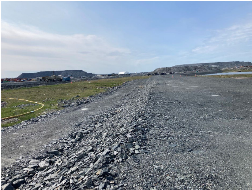
Photograph A6-12 IVR Dike D-1
