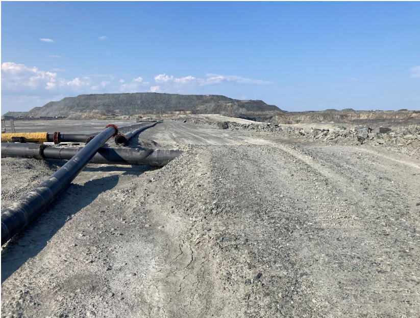
Photograph B7-05 Central Dike and Saddle Dam 5
