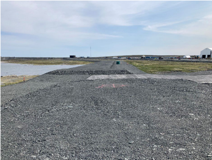
Photograph A6-1 IVR Dike D-1
