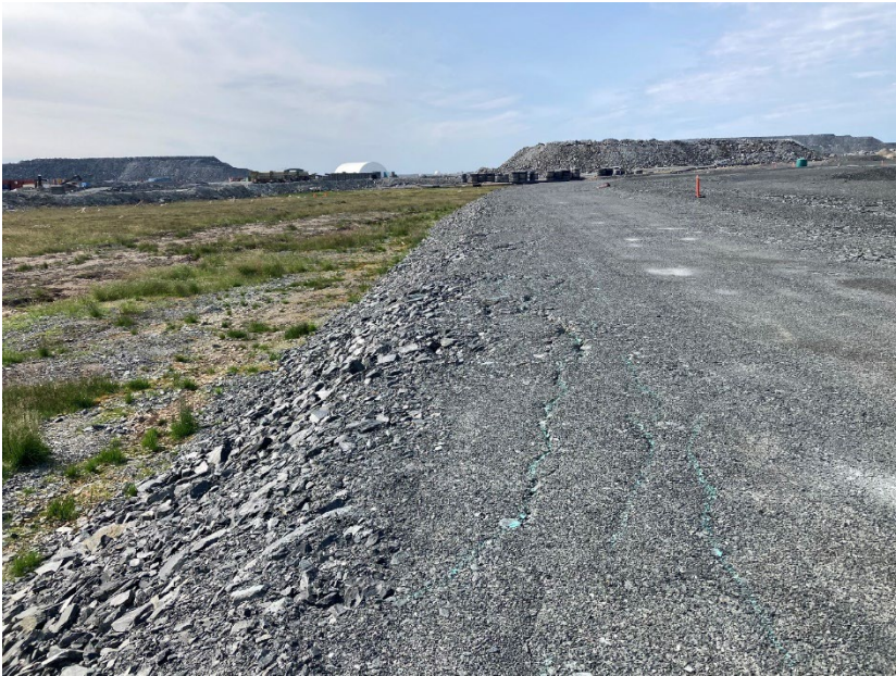
Photograph A6-13 IVR Dike D-1
