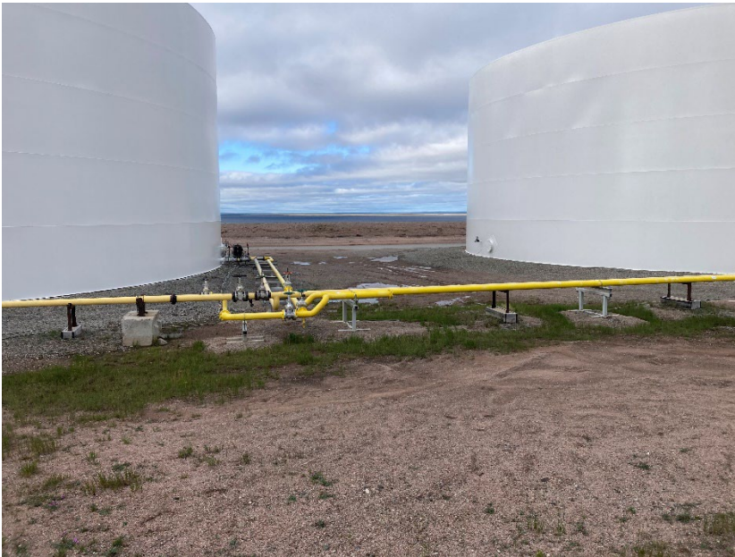
Photograph G1-12 Baker Lake Tank Farm
