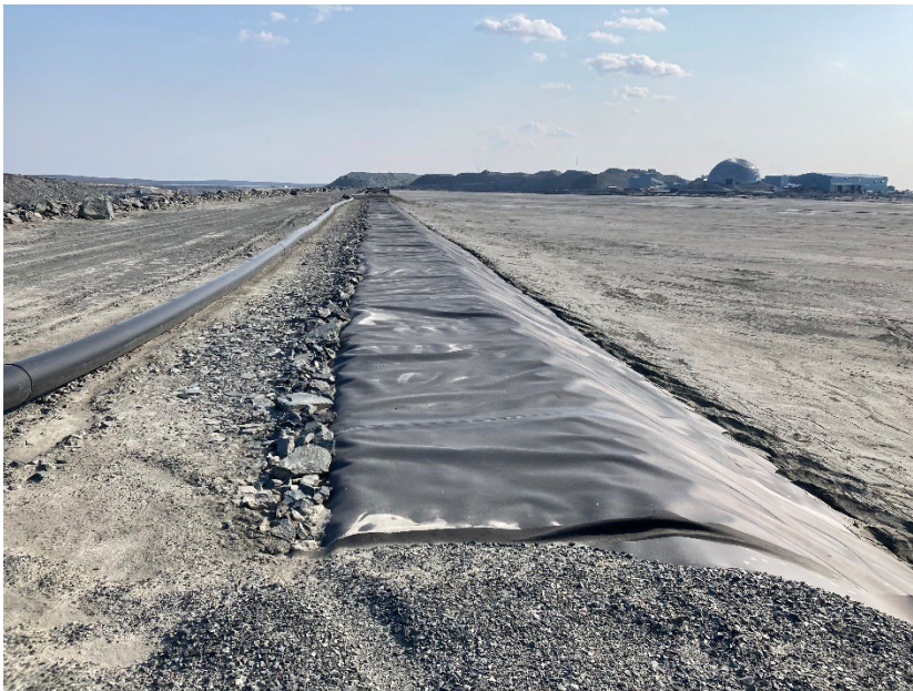
Photograph B7-10 Central Dike and Saddle Dam 5
