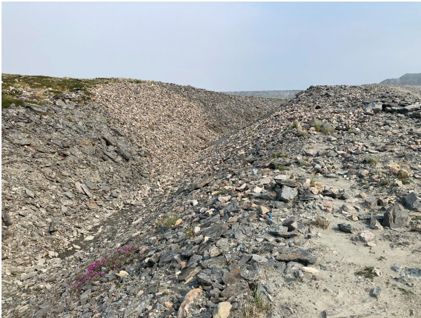
Photograph H2-22 Diversion Ditch and its Sediment and Erosion Protection Structure
