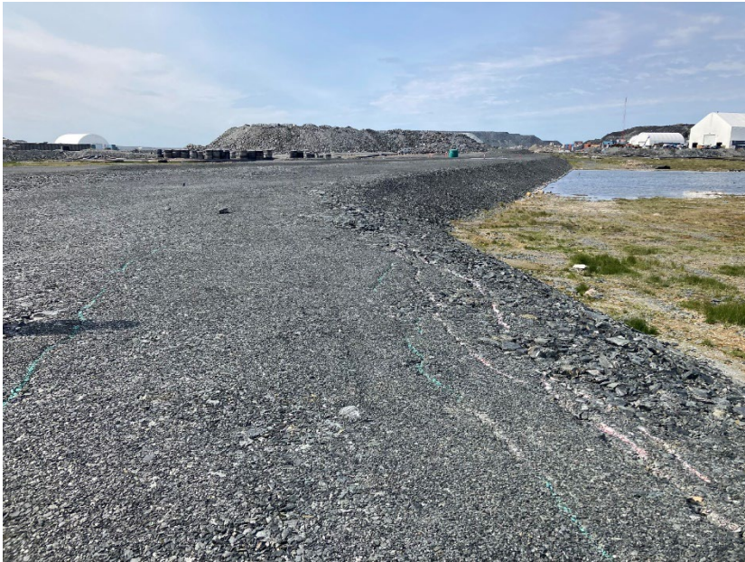
Photograph A6-9 IVR Dike D-1
