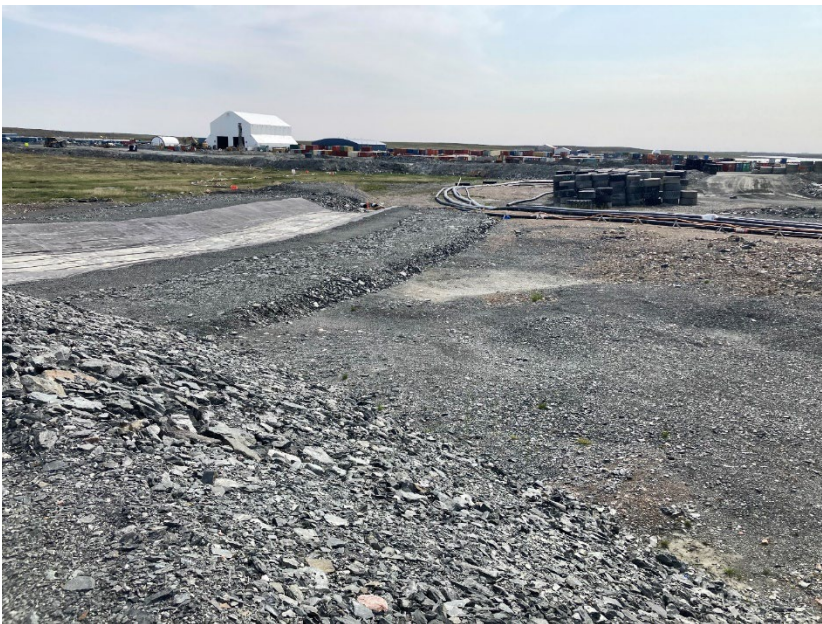
Photograph A6-2 IVR Dike D-1
