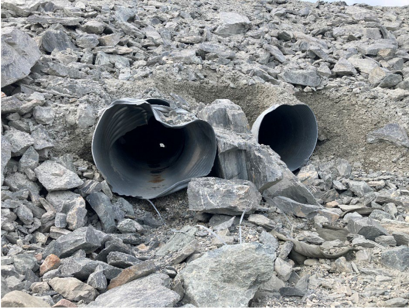
Photograph H2-01 Diversion Ditch and its Sediment and Erosion Protection Structure
