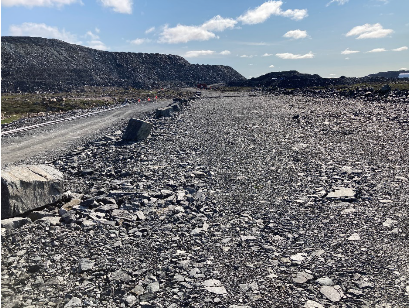
Photograph A7-5 WRSF Dike
