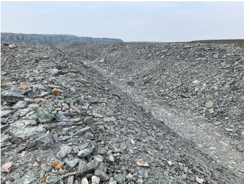
Photograph H2-02 Diversion Ditch and its Sediment and Erosion Protection Structure
