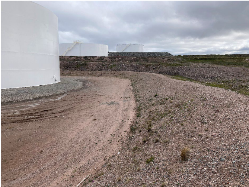
Photograph G1-09 Baker Lake Tank Farm
