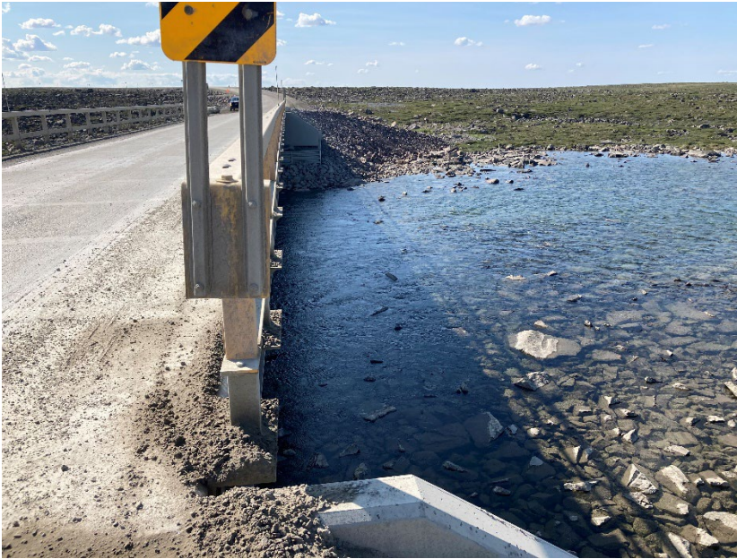
Photograph E2-10 Bridges 5 – km 139+900
