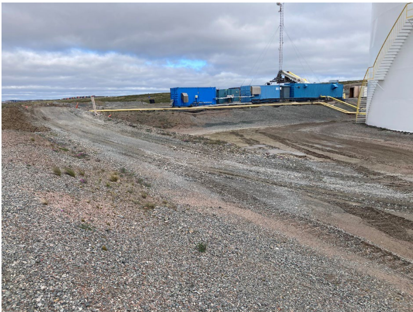
Photograph G1-02 Baker Lake Tank Farm
