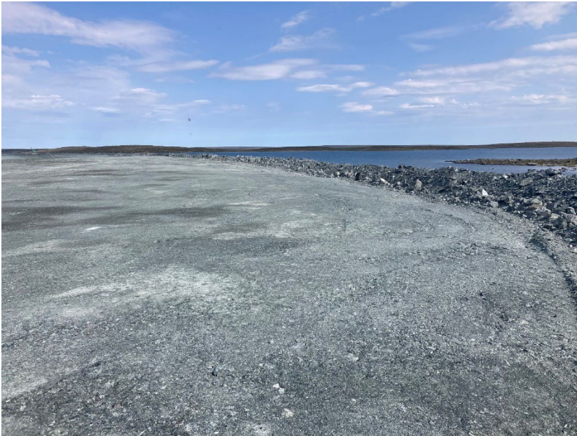
Photograph A3-19 Bay Goose Dike
