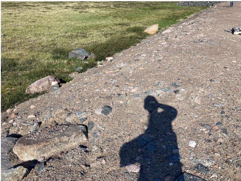
Photograph H13-8 IVR Diversion Channel
