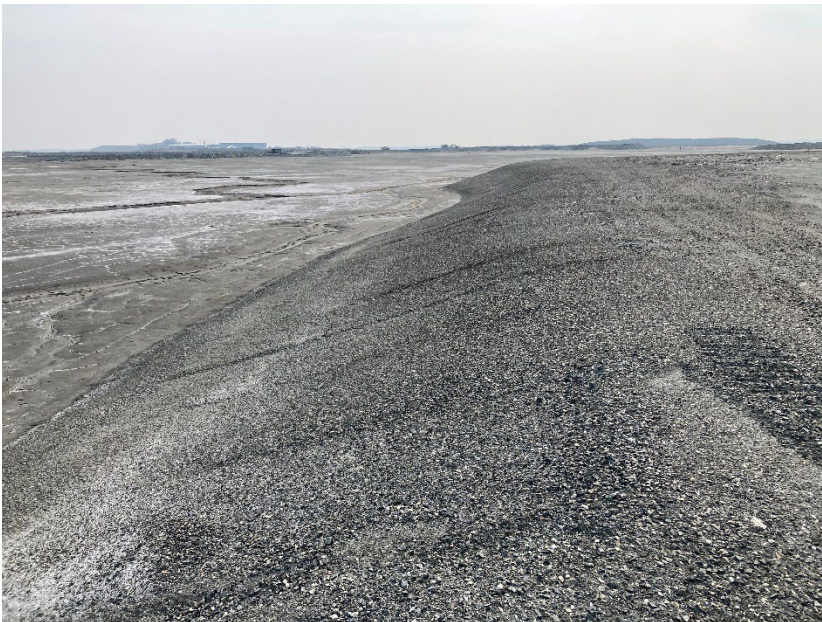
Photograph B1-04 Tailings Storage Facility
