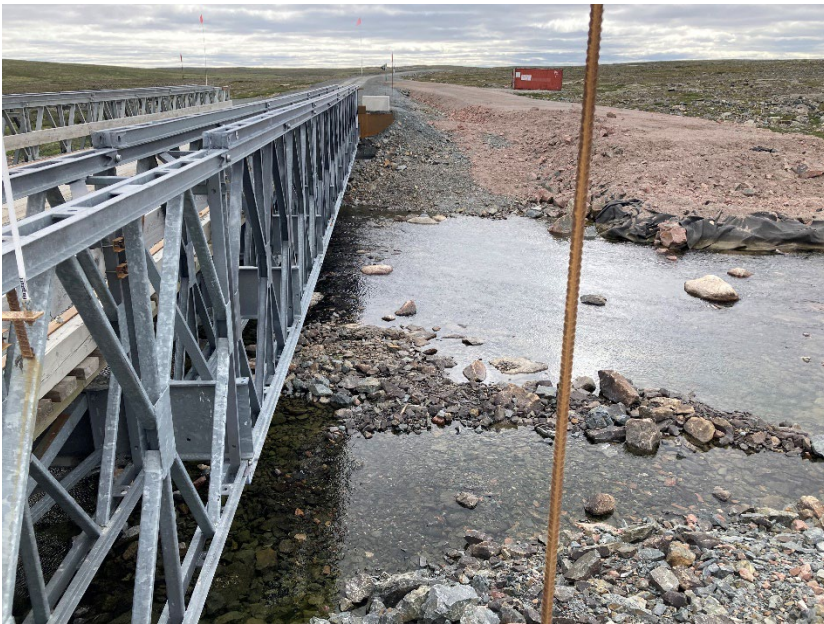
Photograph D3-12 Bridges 6 – R15 km 69+200
