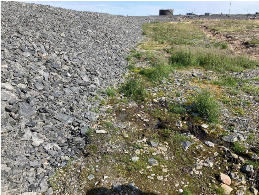
Photograph A6-16 IVR Dike D-1
