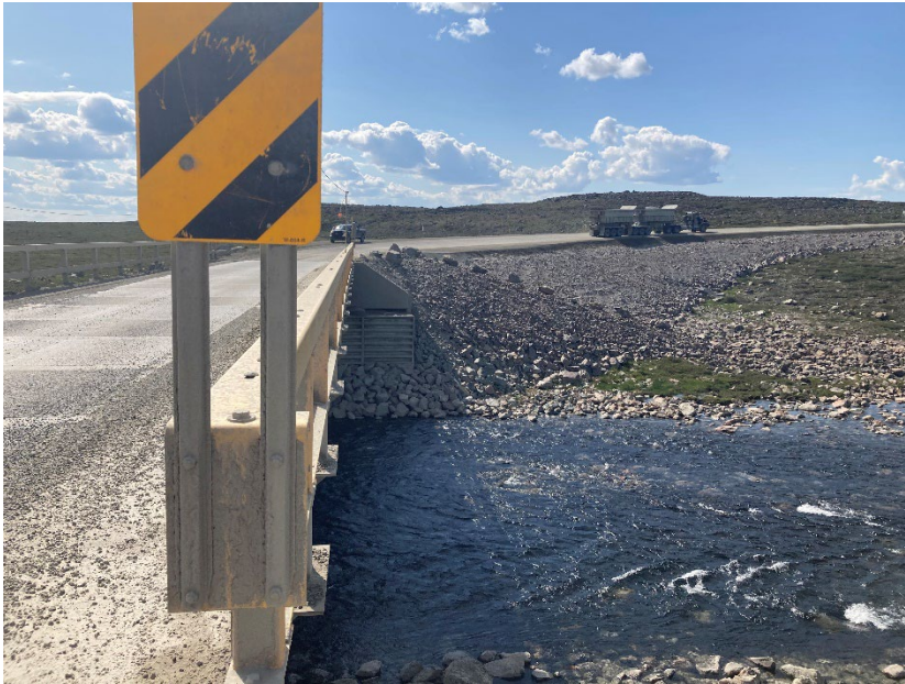
Photograph E2-14 Bridges 7 – km 148+300
