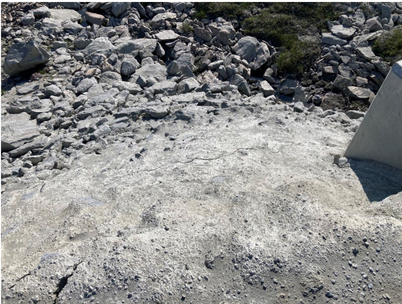
Photograph E2-3 Bridges 1 – km 119+400
