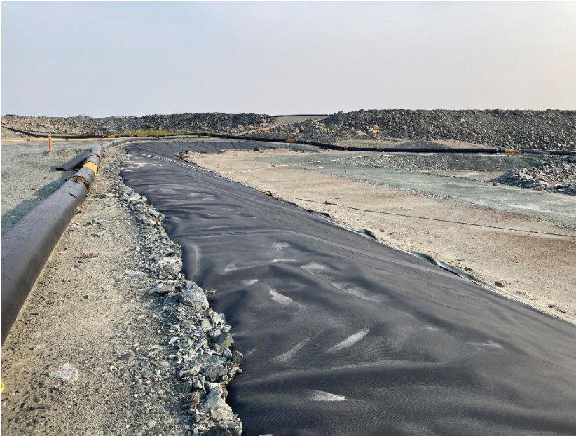
Photograph B5-03 Saddle Dam 3
