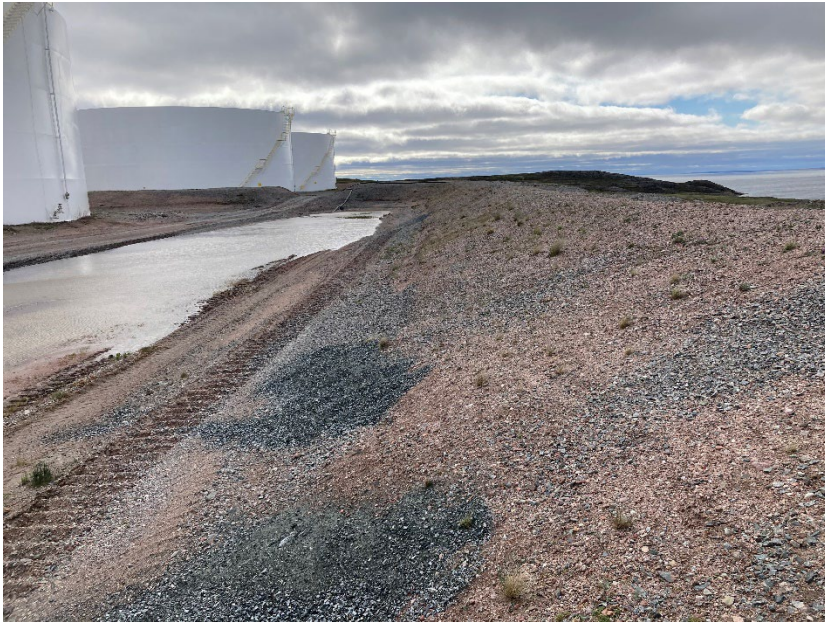
Photograph G1-01 Baker Lake Tank Farm
