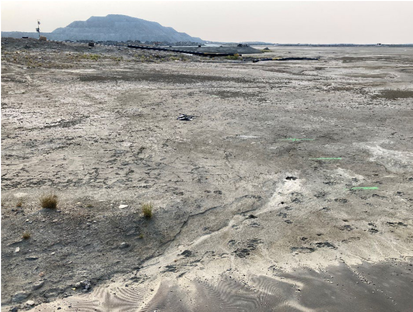
Photograph B2-07 Saddle Dam 1
