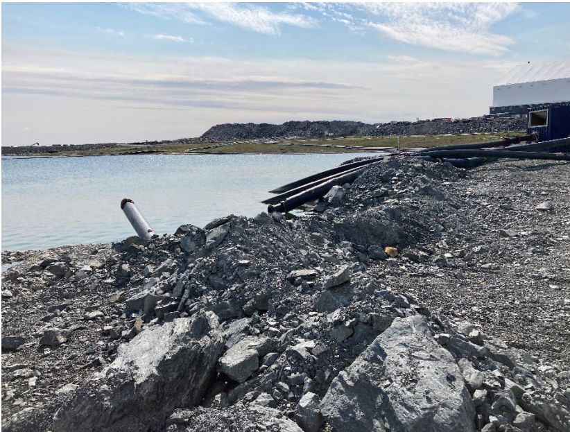
Photograph H8-02 IVR Attenuation Pond Jetty
