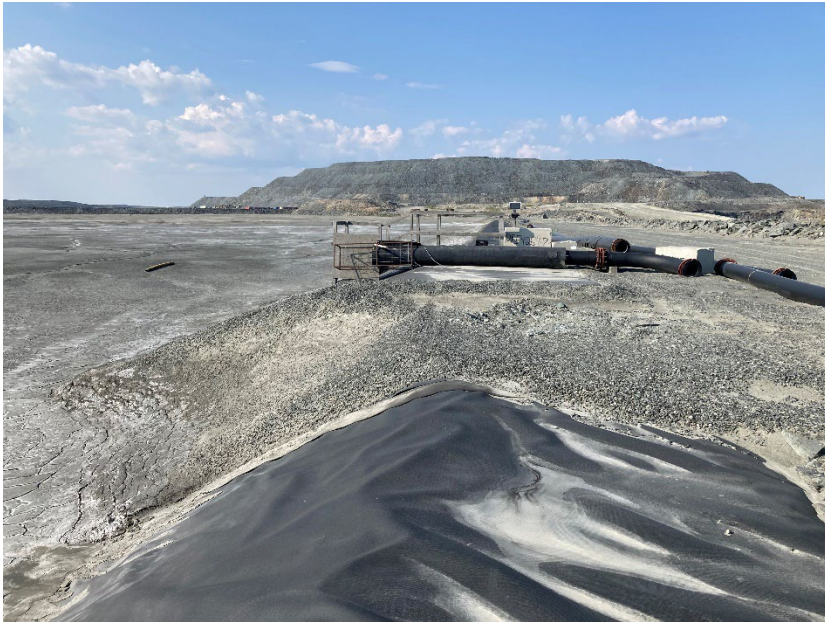
Photograph B7-07 Central Dike and Saddle Dam 5
