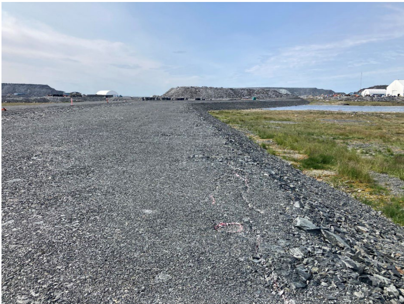
Photograph A6-10 IVR Dike D-1
