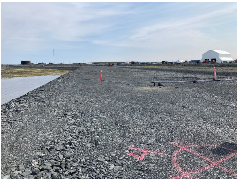
Photograph A6-6 IVR Dike D-1
