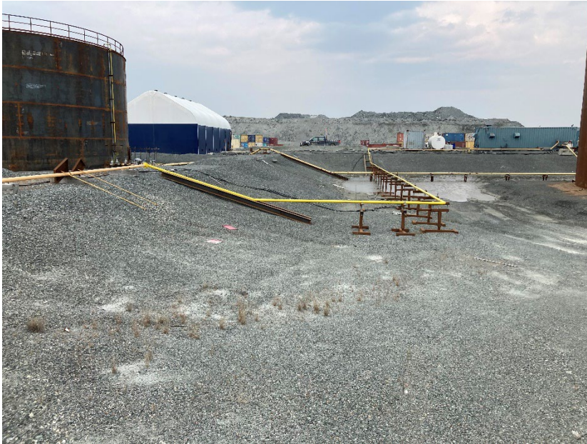
Photograph G2-07 Meadowbank Tank Farm
