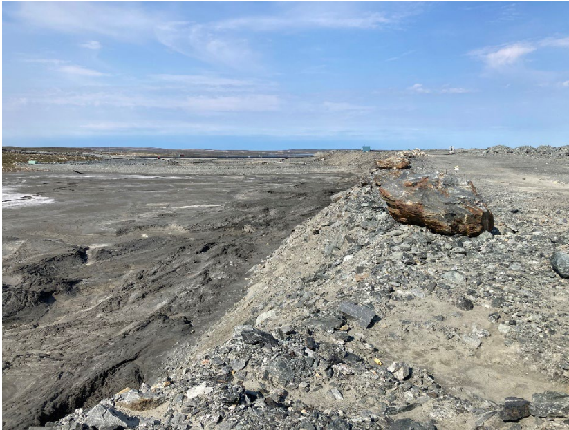
Photograph B4-07 Stormwater Dike
