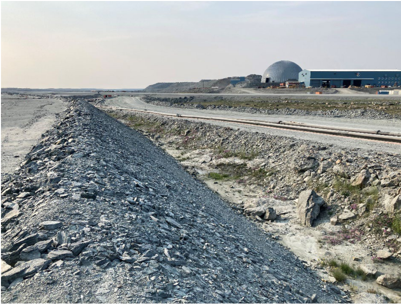
Photograph B6-03 Saddle Dam 4
