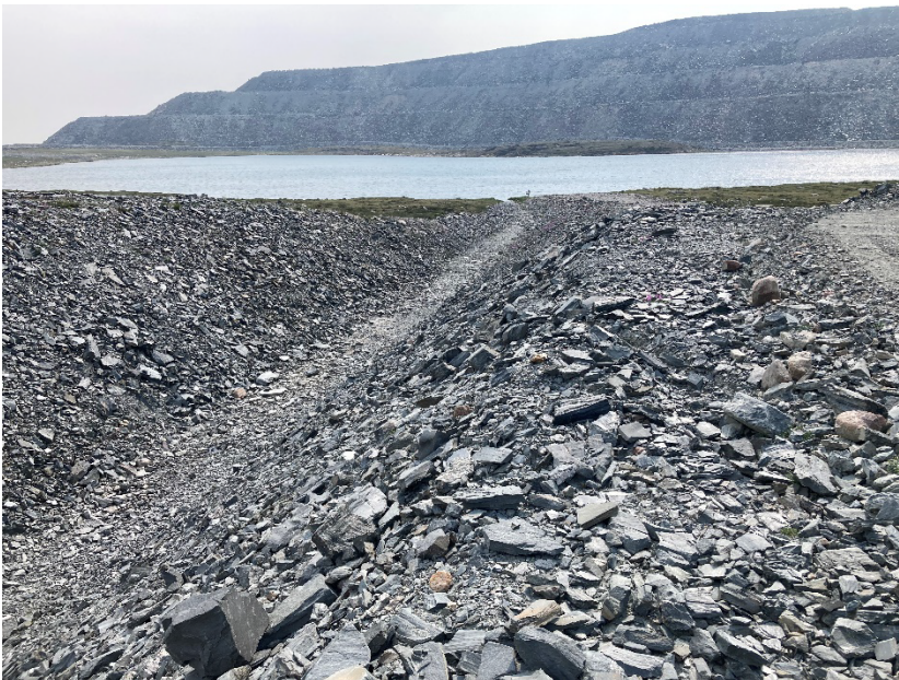
Photograph H2-04 Diversion Ditch and its Sediment and Erosion Protection Structure
