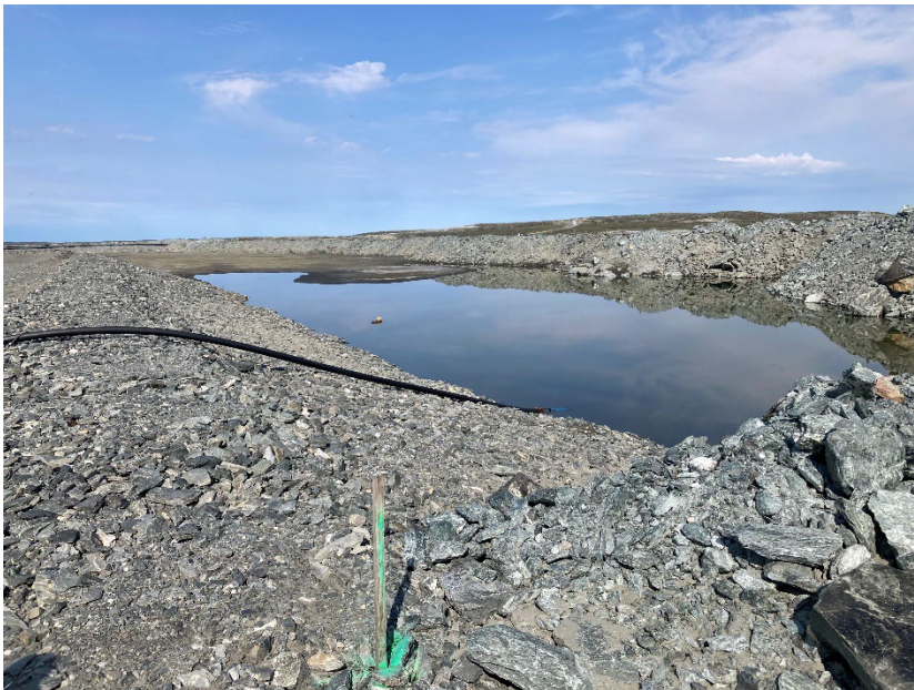
Photograph B4-08 Stormwater Dike
