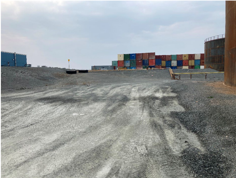
Photograph G2-09 Meadowbank Tank Farm
