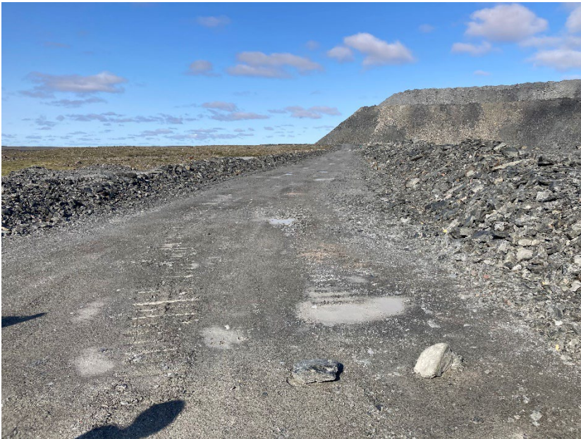
Photograph A7-2 WRSF Dike
