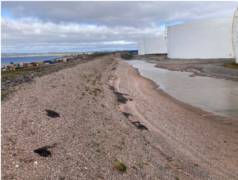
Photograph G1-08 Baker Lake Tank Farm
