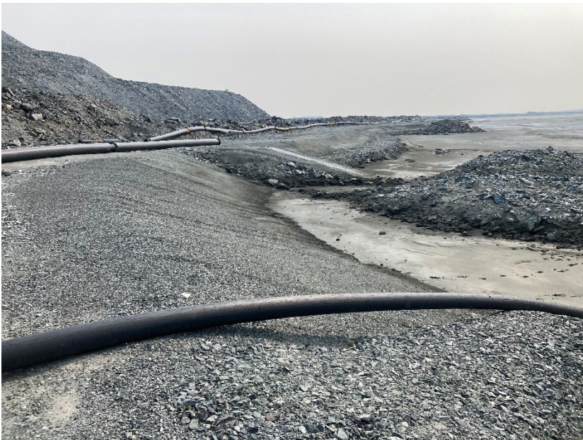
Photograph B1-12 Tailings Storage Facility
