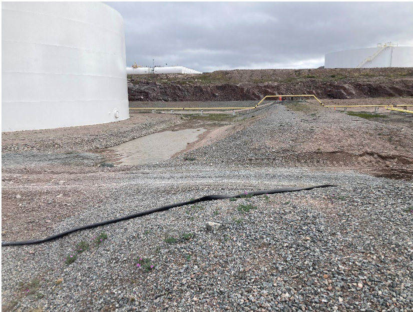
Photograph G1-04 Baker Lake Tank Farm
