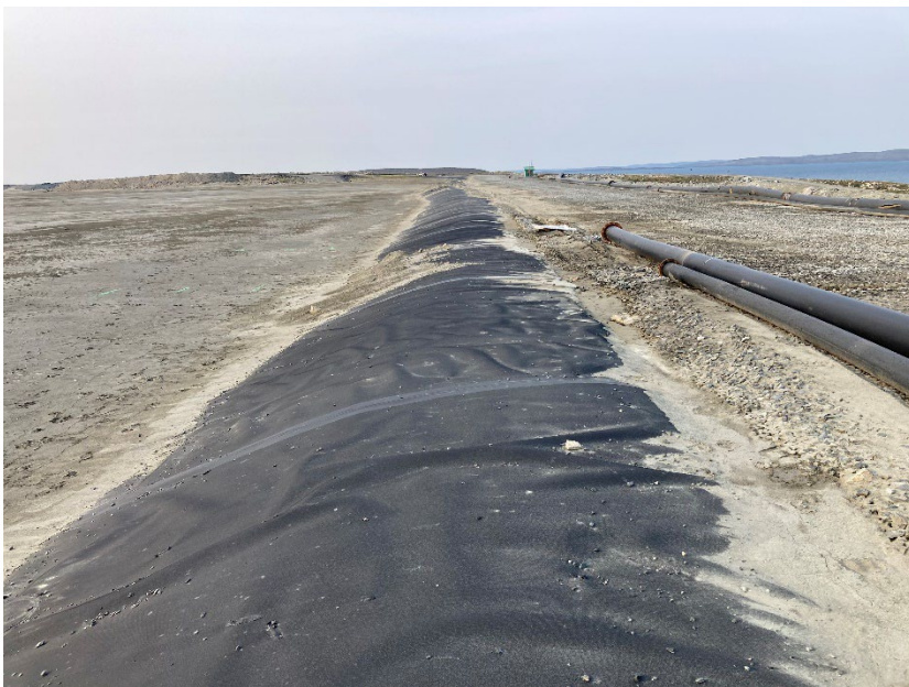
Photograph B2-06 Saddle Dam 1
