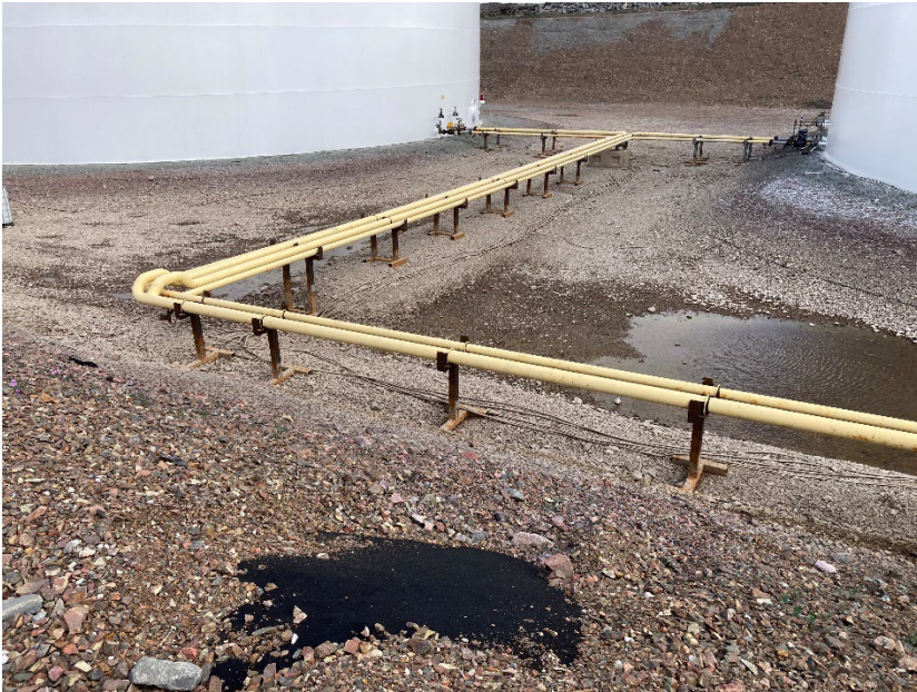
Photograph G1-25 Baker Lake Tank Farm
