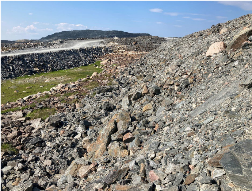
Photograph A1-09 East Dike
