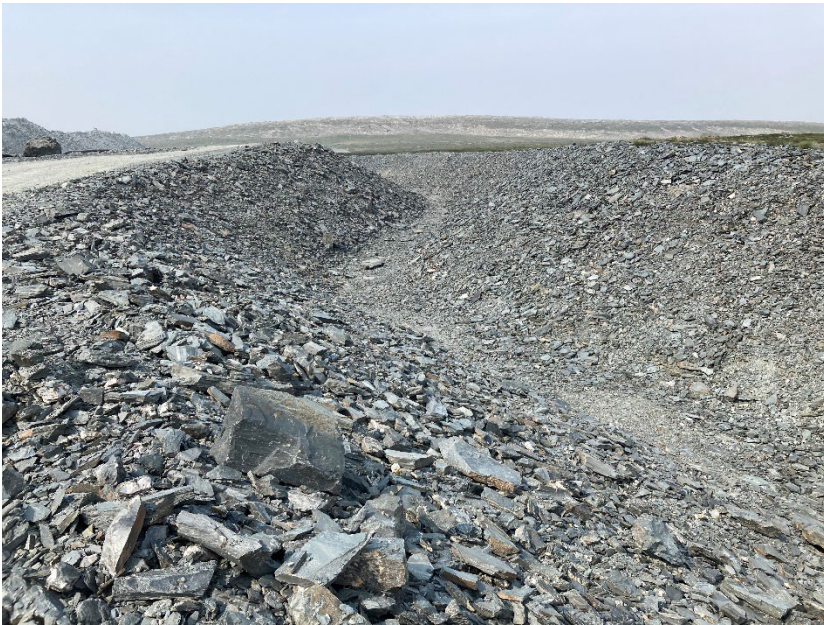
Photograph H2-06 Diversion Ditch and its Sediment and Erosion Protection Structure
