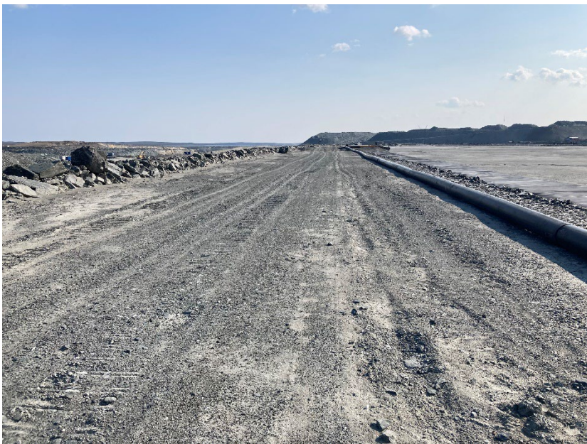
Photograph B7-08 Central Dike and Saddle Dam 5
