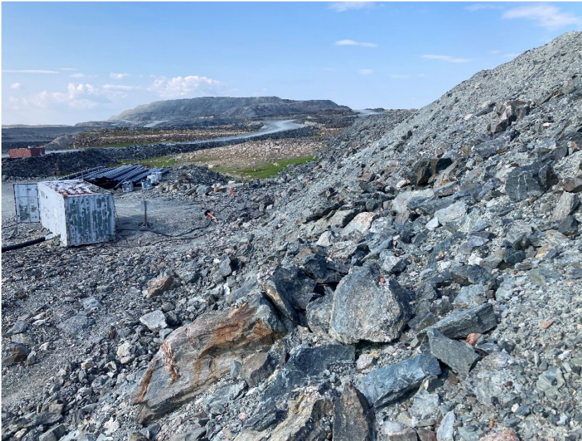
Photograph A1-11 East Dike
