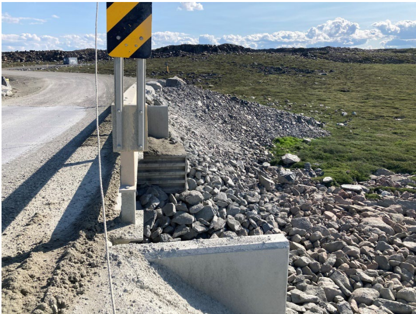
Photograph E2-5 Bridges 2 – km 126+700
