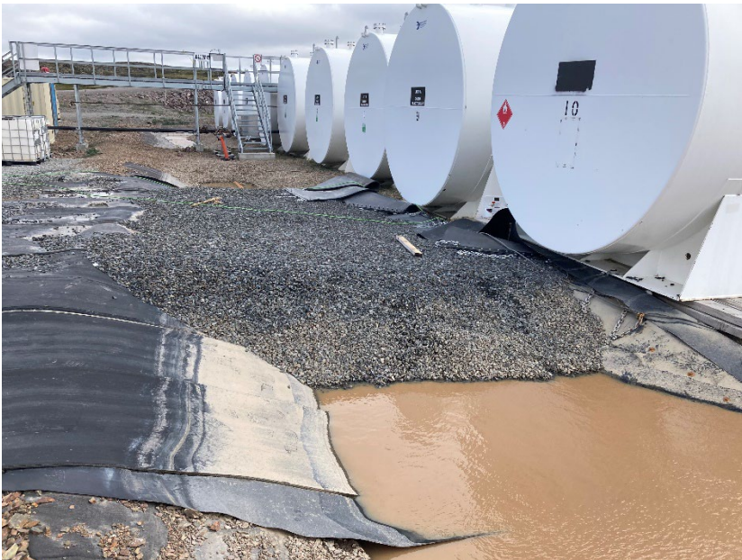
Photograph G1-16 Baker Lake Tank Farm
