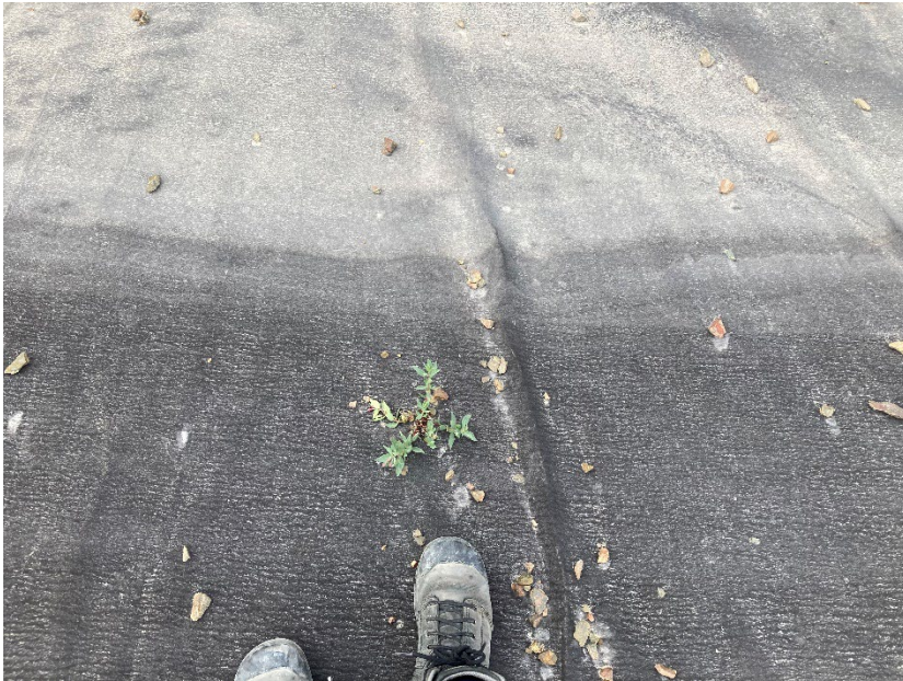
Photograph G1-19 Baker Lake Tank Farm
