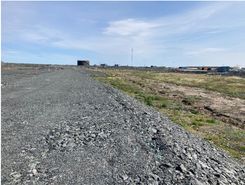
Photograph A6-17 IVR Dike D-1
