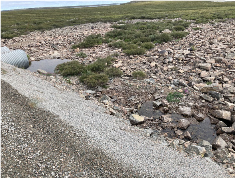
Photograph D2-01: PC-17A km 8+830
