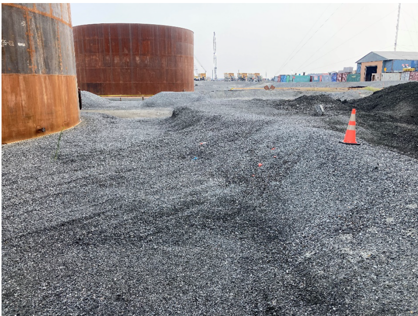
Photograph G2-04 Meadowbank Tank Farm
