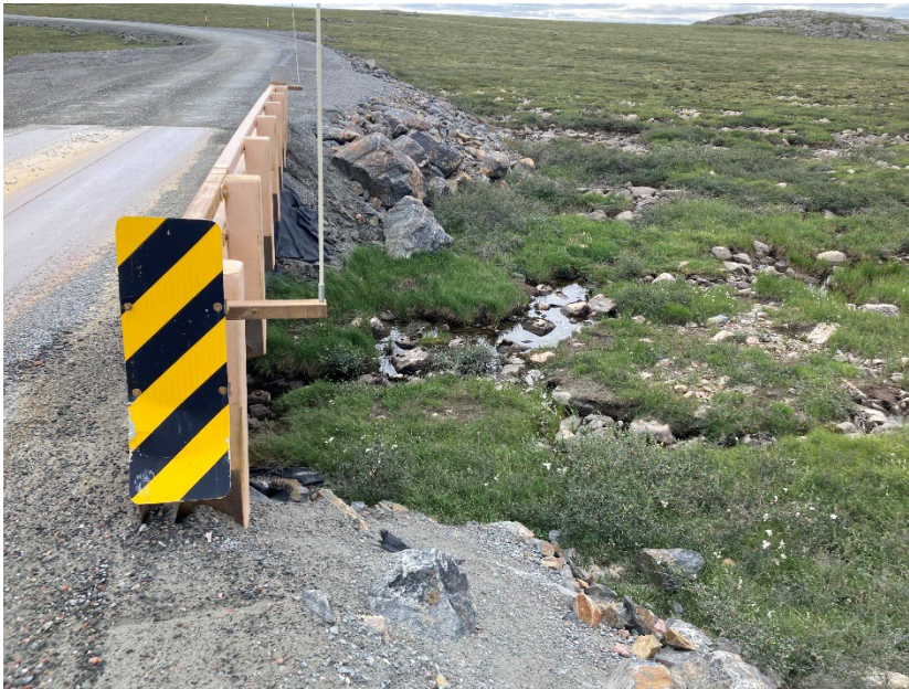
Photograph D3-14 Bridges 7 – R16 km 73+800
