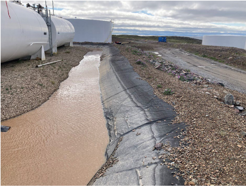
Photograph G1-15 Baker Lake Tank Farm
