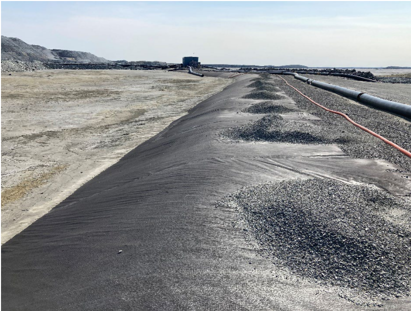
Photograph B4-11 Stormwater Dike
