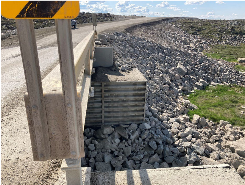
Photograph E2-13 Bridges 6 – km 142+100
