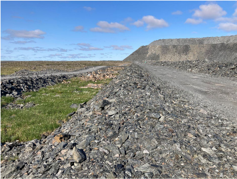
Photograph A7-1 WRSF Dike
