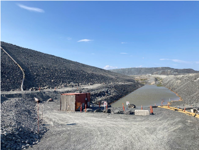
Photograph B7-01 Central Dike and Saddle Dam 5
