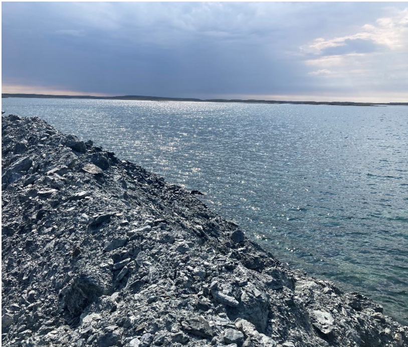
Photograph A3-12 Bay Goose Dike
