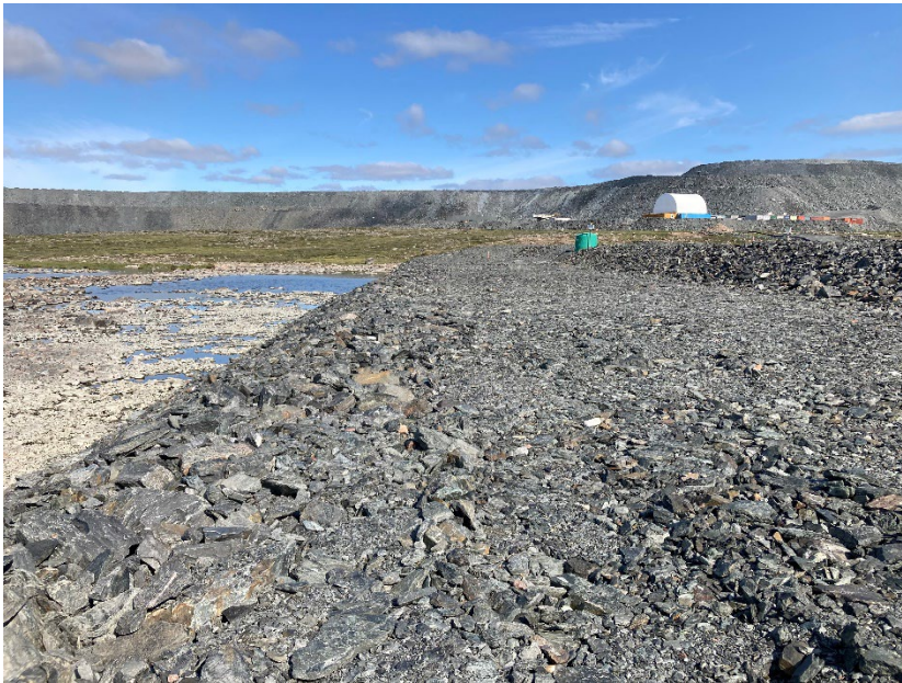
Photograph A8-8 Mammoth Dike
