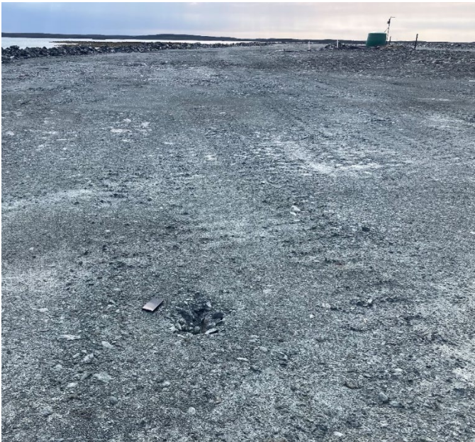
Photograph A3-26 Bay Goose Dike
