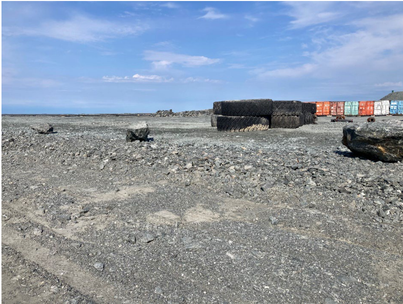
Photograph B4-01 Stormwater Dike
