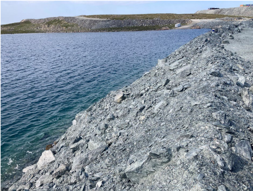
Photograph A3-07 Bay Goose Dike
