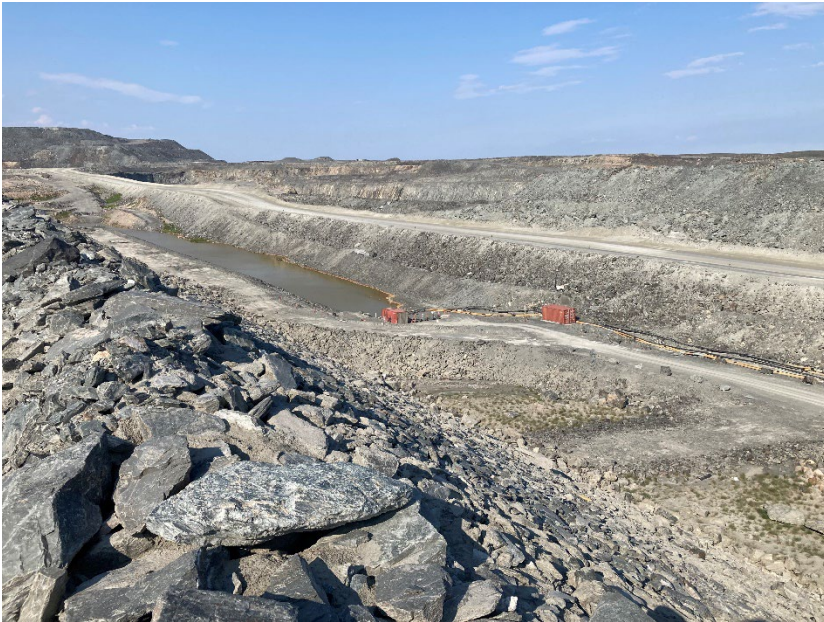
Photograph B7-03 Central Dike and Saddle Dam 5
