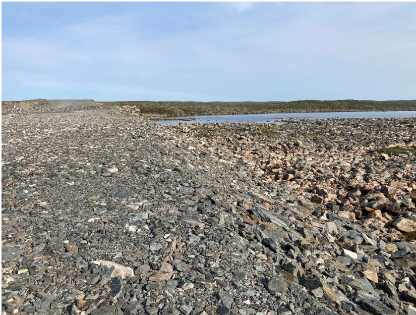
Photograph A4-1 Vault Dike
