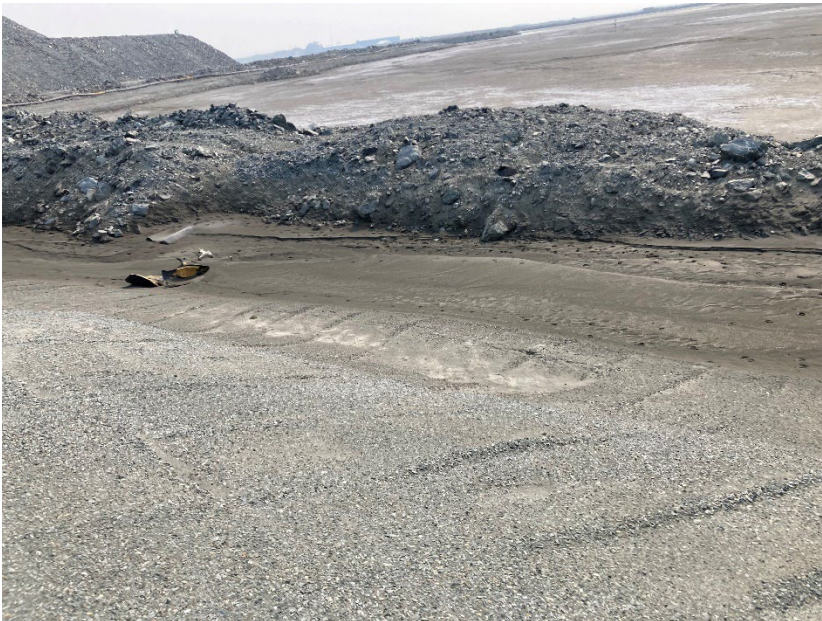
Photograph B1-10 Tailings Storage Facility
