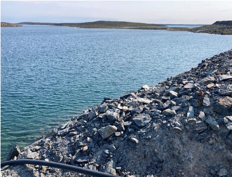
Photograph A1-01 East Dike
