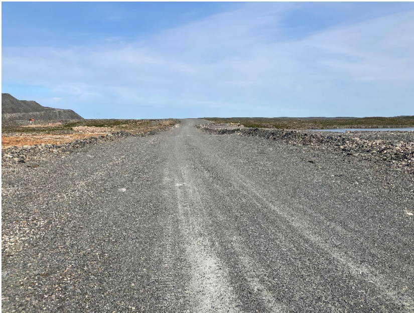
Photograph A4-7 Vault Dike
