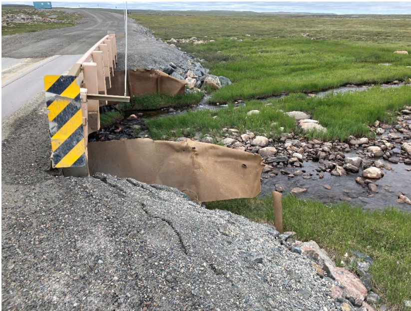
Photograph D3-18 Bridges 9 – R19 km 83+150
