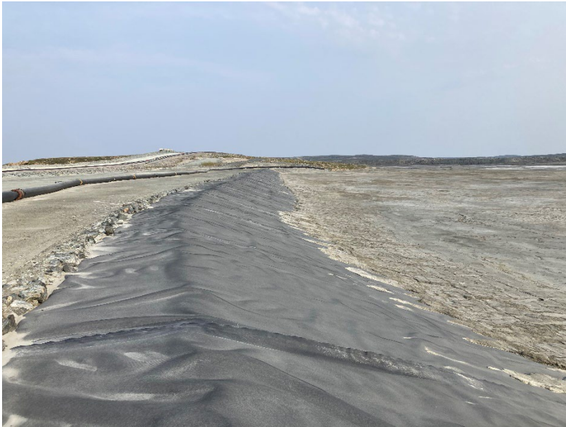
Photograph B6-05 Saddle Dam 4
