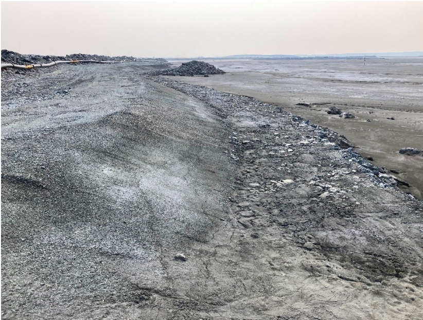
Photograph B1-7 Tailings Storage Facility
