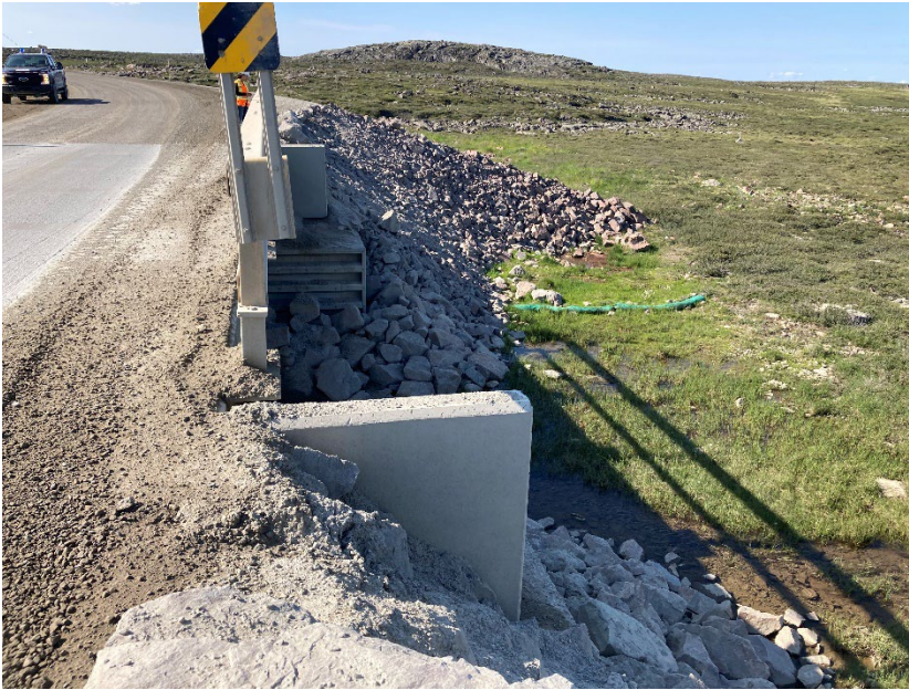
Photograph E2-9 Bridges 4 – km 136+000
