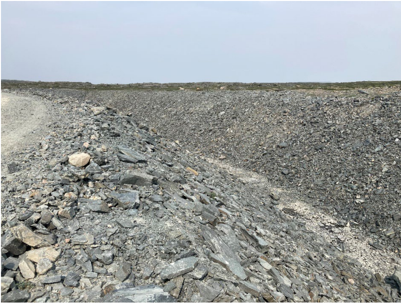
Photograph H2-05 Diversion Ditch and its Sediment and Erosion Protection Structure
