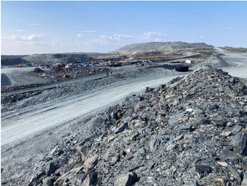
Photograph A1-13 East Dike
