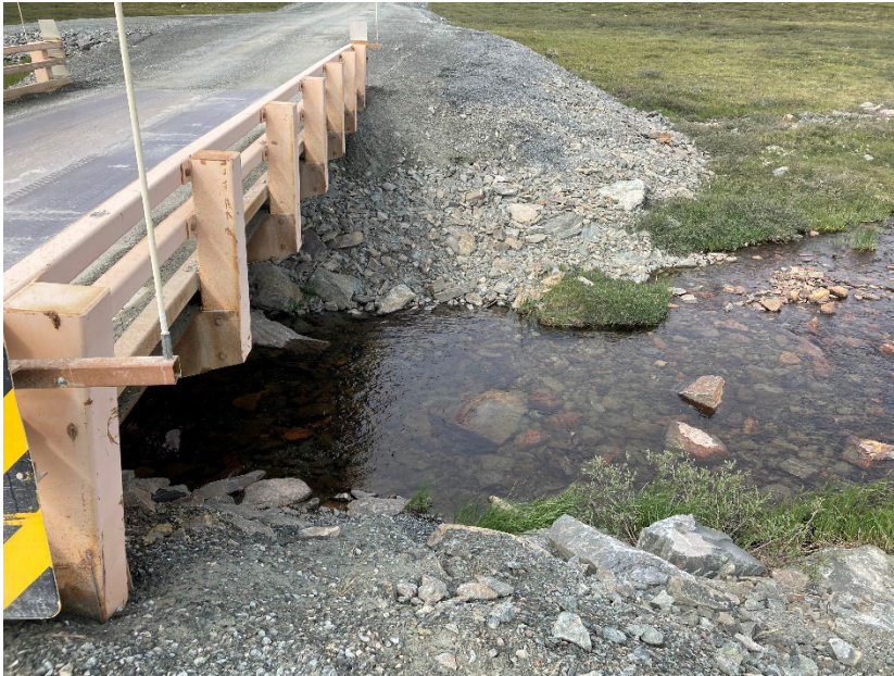
Photograph D3-7 Bridges 4 – R09 km 48+500
