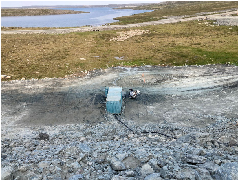
Photograph B2-09 Saddle Dam 1
