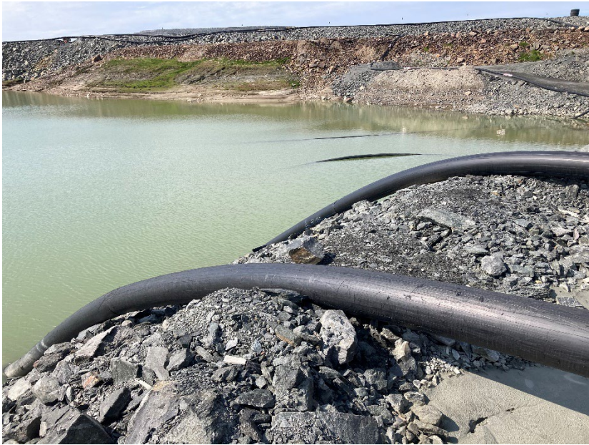
Photograph H7-03 Whale Tail Mine Site Attenuation Pond Jetty
