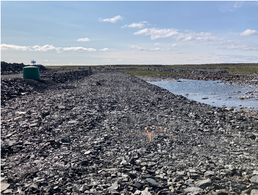
Photograph A8-5 Mammoth Dike
