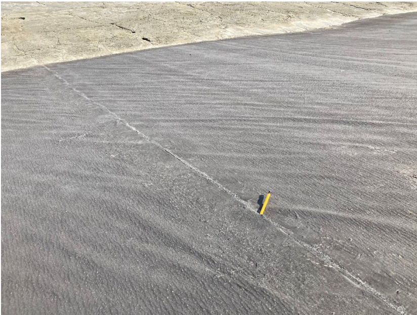
Photograph B4-10 Stormwater Dike
