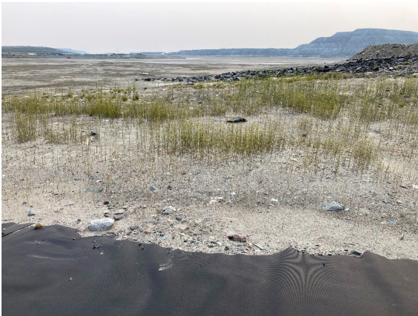
Photograph B2-01 Saddle Dam 1
