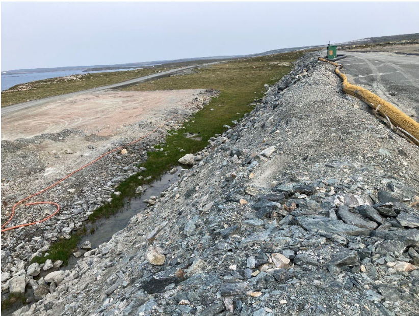
Photograph B3-10 Saddle Dam 2
