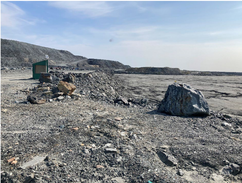
Photograph B4-06 Stormwater Dike
