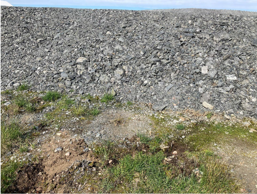
Photograph A6-15 IVR Dike D-1
