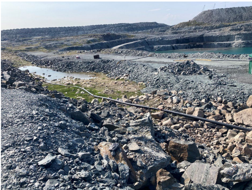
Photograph A3-34 Bay Goose Dike
