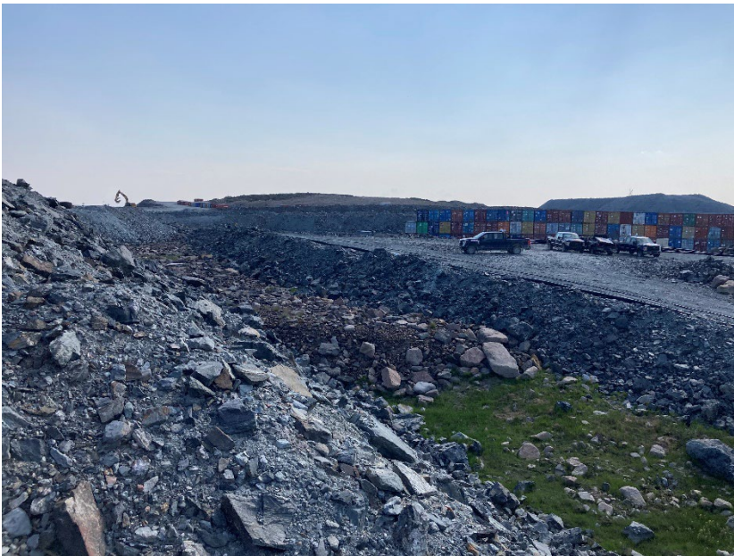
Photograph A1-12 East Dike
