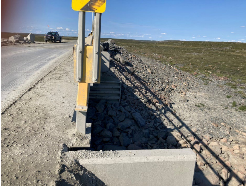
Photograph E2-4 Bridges 2 – km 126+700
