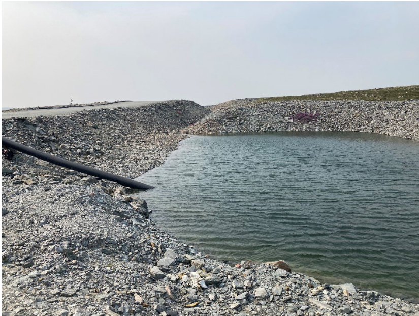
Photograph H2-21 Diversion Ditch and its Sediment and Erosion Protection Structure
