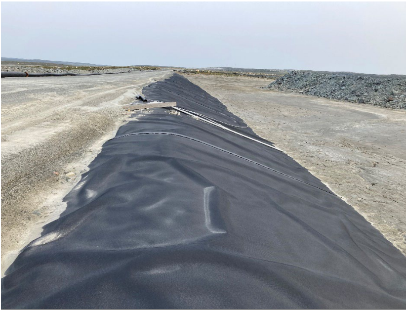
Photograph B3-04 Saddle Dam 2
