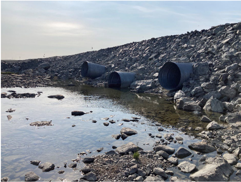
Photograph H1-01 Vault Road Culverts
