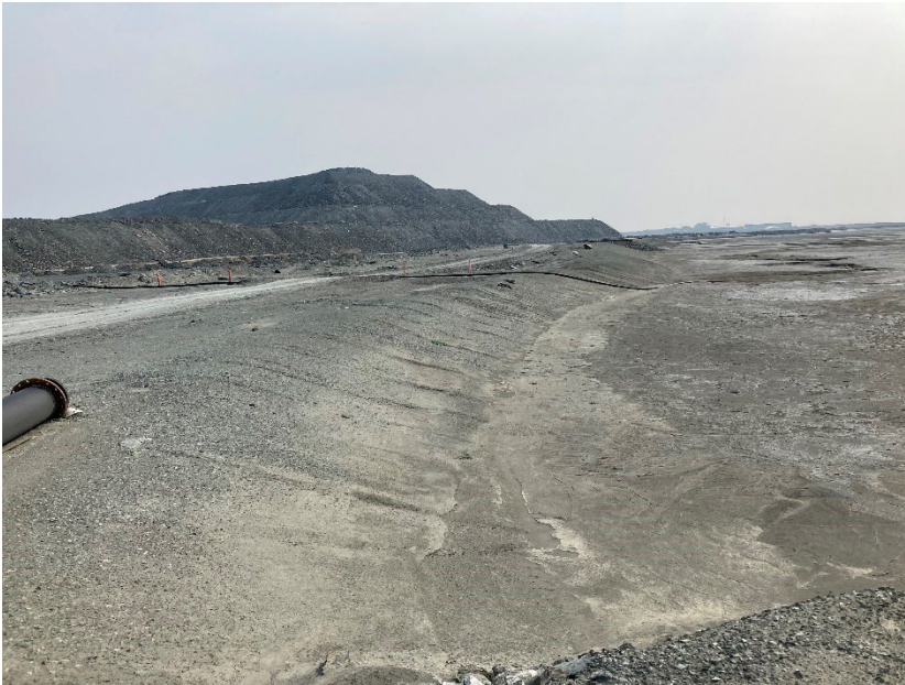
Photograph B1-09 Tailings Storage Facility
