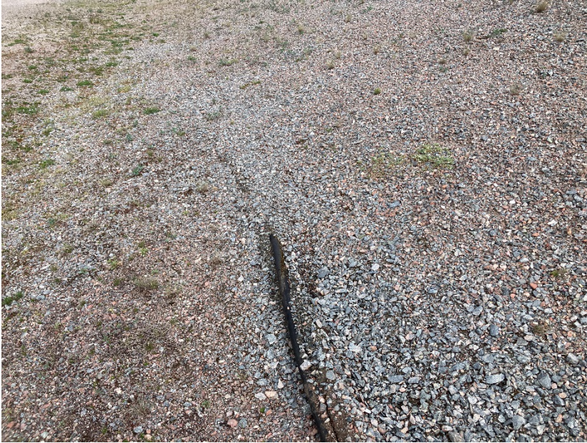
Photograph G1-13 Baker Lake Tank Farm
