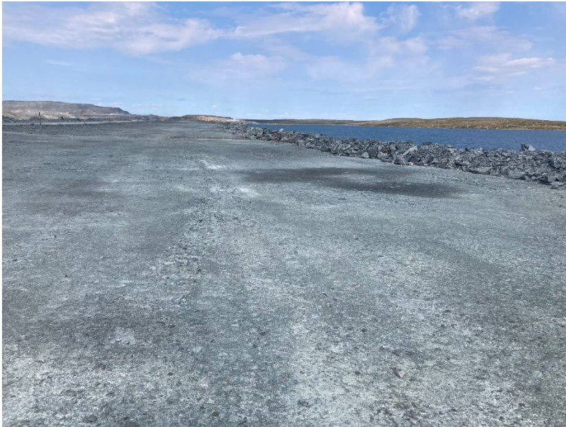
Photograph A3-27 Bay Goose Dike
