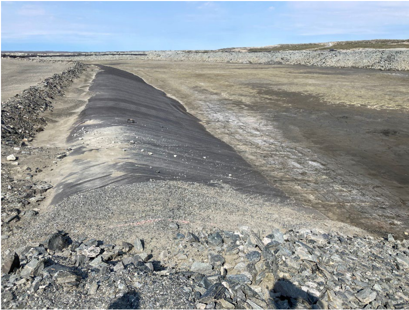
Photograph B4-09 Stormwater Dike
