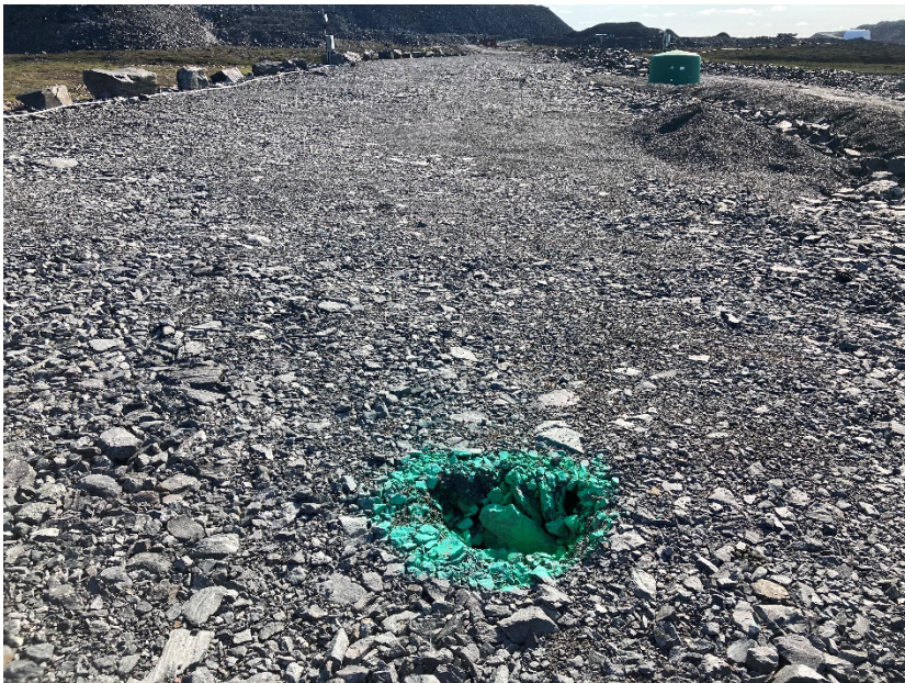
Photograph A7-8 WRSF Dike
