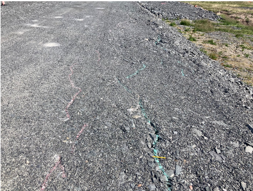
Photograph A6-14 IVR Dike D-1
