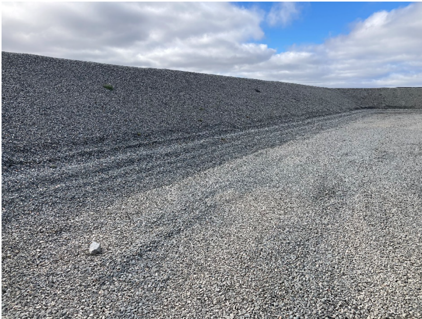
Photograph G1-28 Baker Lake Tank Farm
