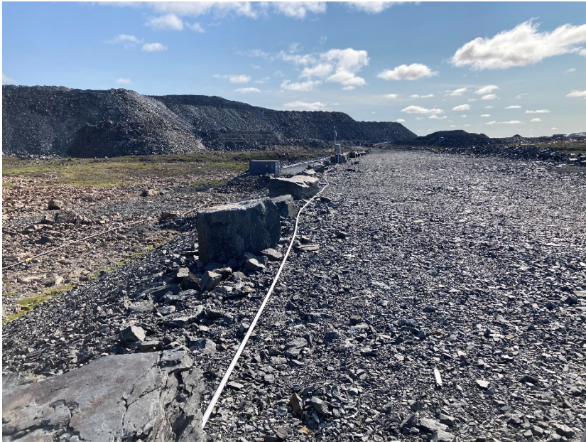
Photograph A7-7 WRSF Dike
