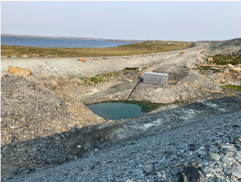
Photograph B5-04 Saddle Dam 3
