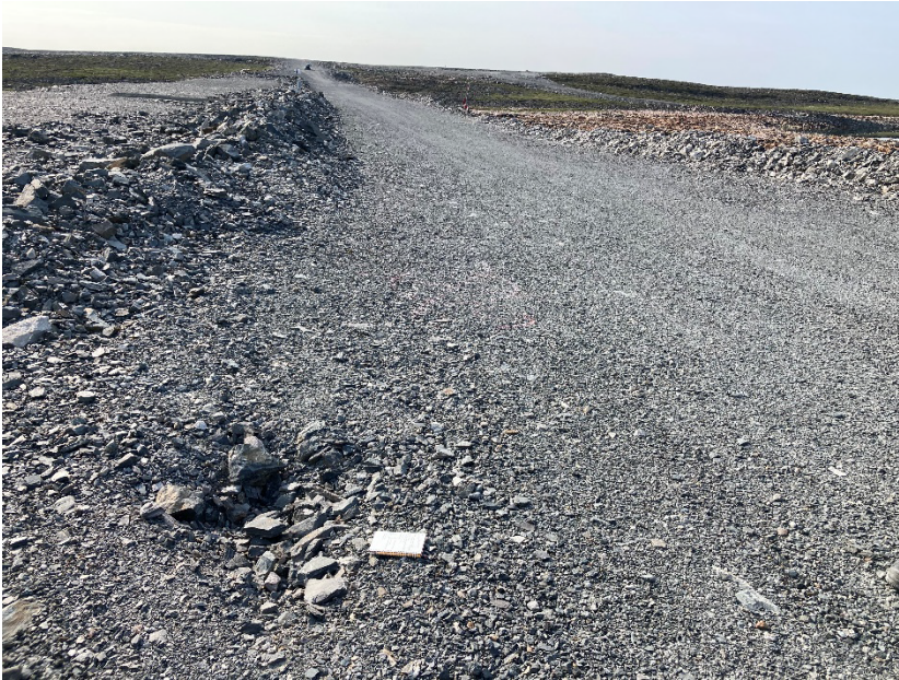
Photograph A4-3 Vault Dike
