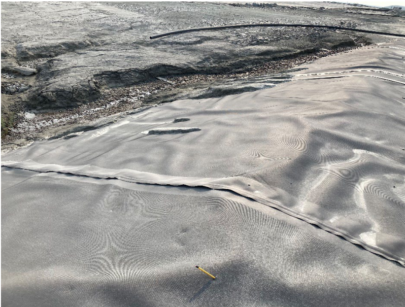
Photograph B6-08 Saddle Dam 4
