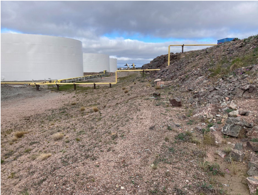
Photograph G1-11 Baker Lake Tank Farm
