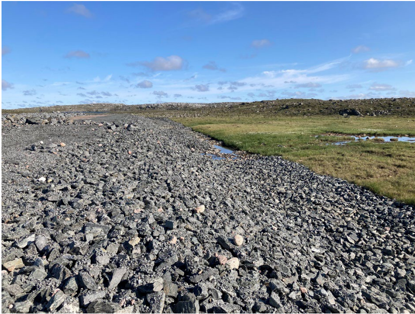
Photograph H13-1 IVR Diversion Channel
