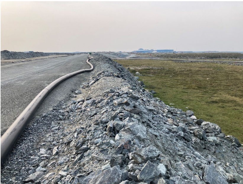
Photograph B3-08 Saddle Dam 2
