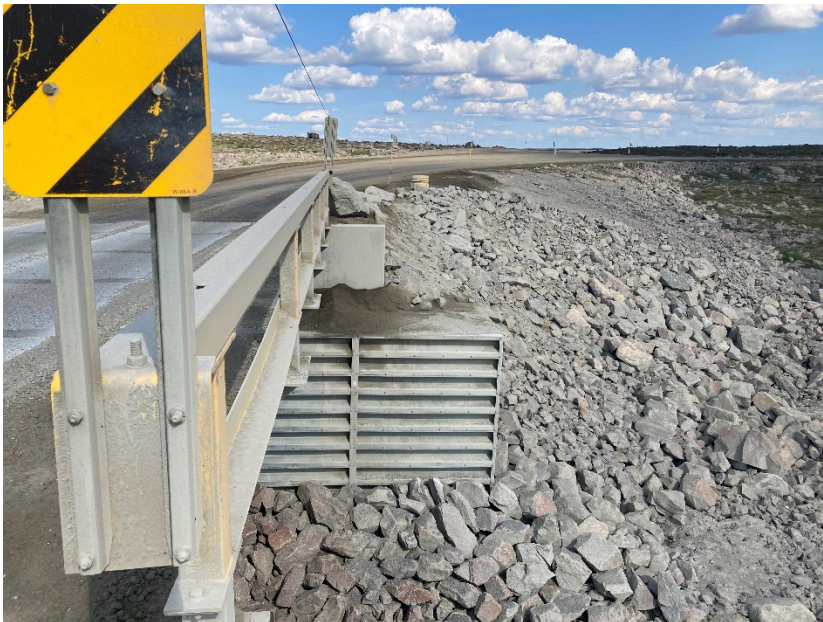
Photograph E2-12 Bridges 6 – km 142+100
