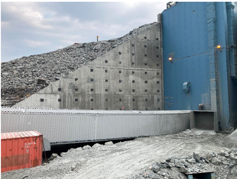
Photograph H6-02 Meadowbank Crusher Retaining Wall
