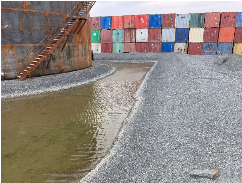
Photograph G2-02 Meadowbank Tank Farm
