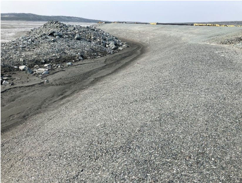
Photograph B1-11 Tailings Storage Facility
