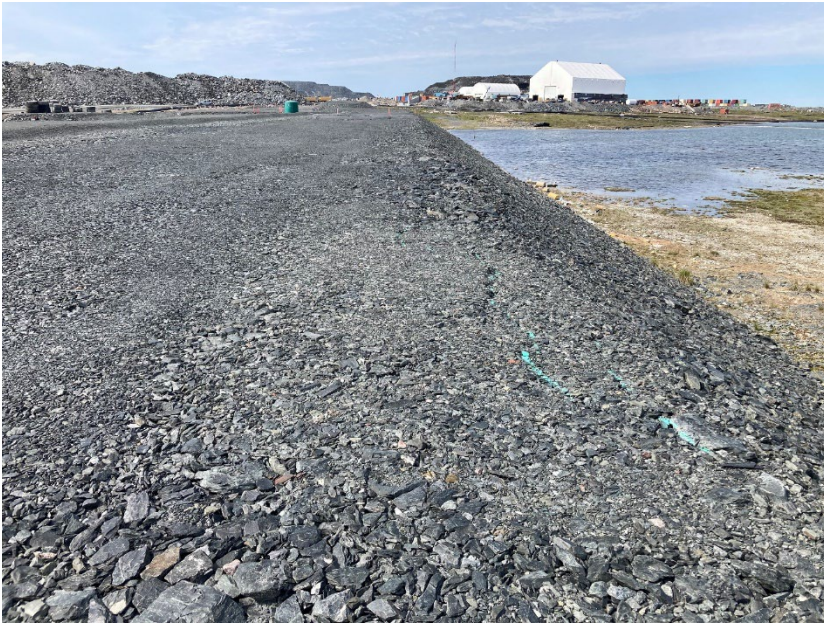
Photograph A6-7 IVR Dike D-1
