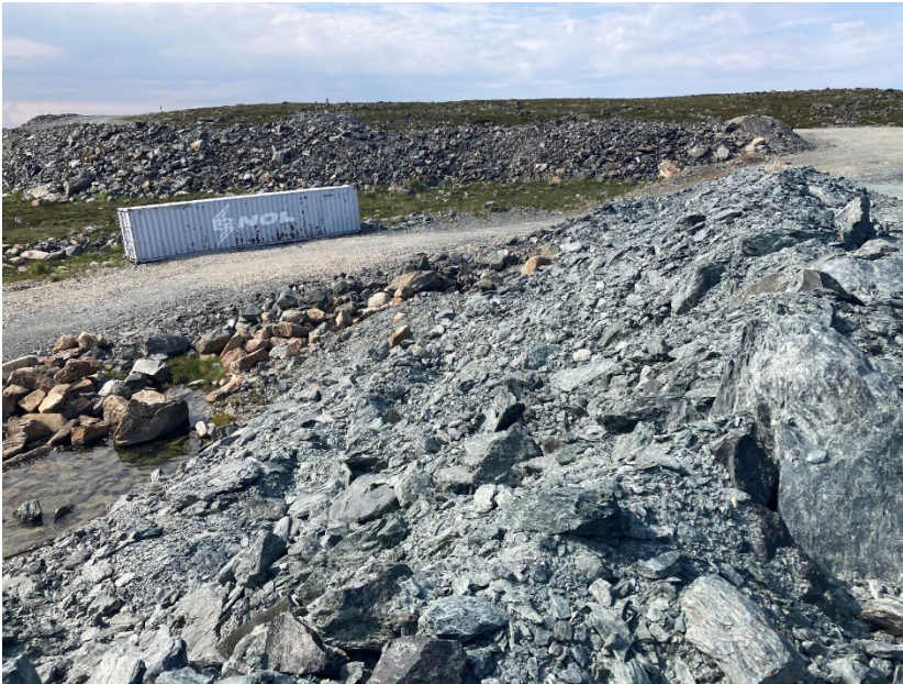
Photograph A3-01 Bay Goose Dike
