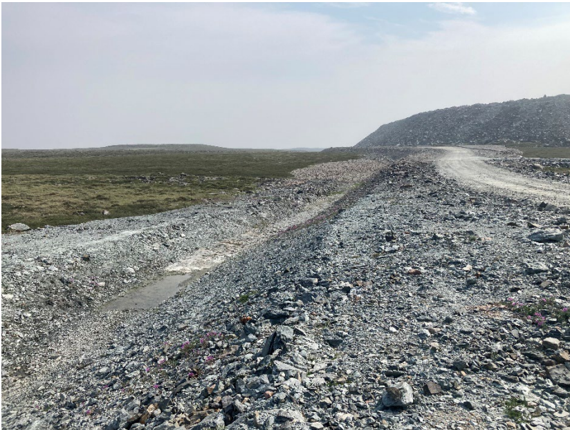
Photograph H2-08 Diversion Ditch and its Sediment and Erosion Protection Structure
