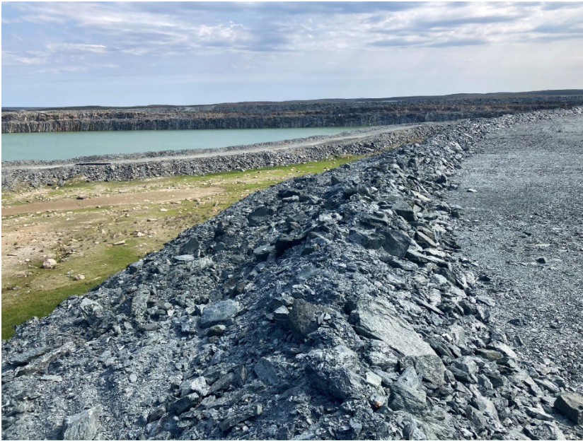
Photograph A3-03 Bay Goose Dike
