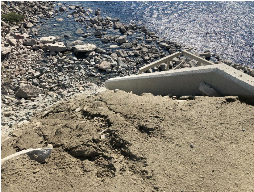
Photograph E2-16 Bridges 7 – km 148+300
