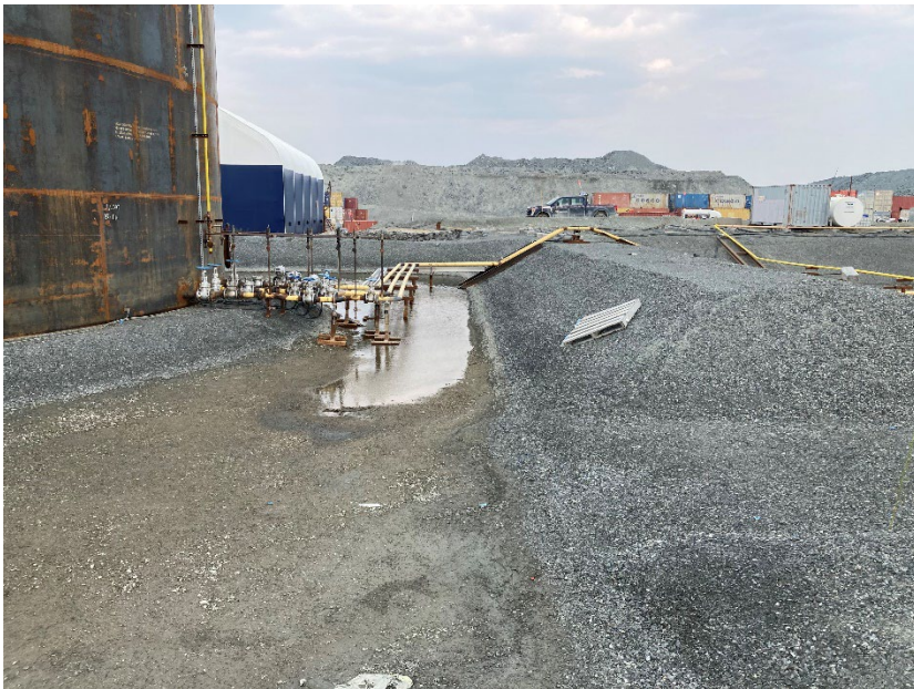
Photograph G2-06 Meadowbank Tank Farm
