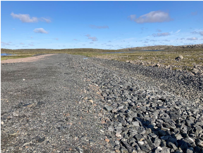
Photograph H13-4 IVR Diversion Channel
