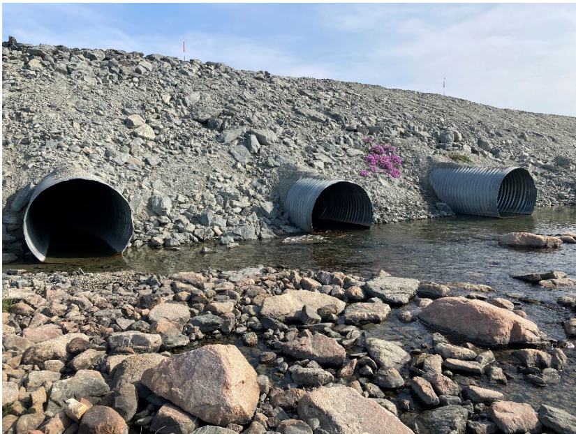
Photograph H1-02 Vault Road Culverts
