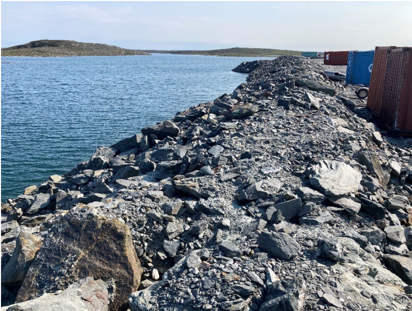
Photograph A1-03 East Dike
