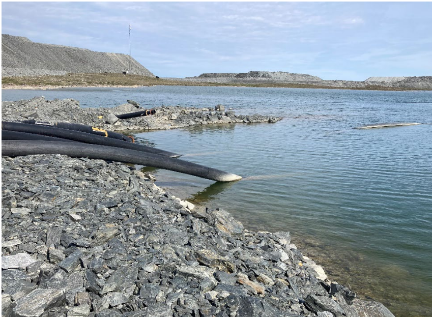
Photograph H8-04 IVR Attenuation Pond Jetty
