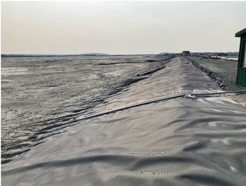
Photograph B6-06 Saddle Dam 4
