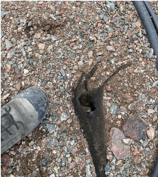
Photograph G1-14 Baker Lake Tank Farm
