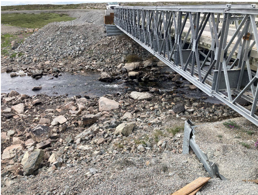
Photograph D3-2 Bridges 1 – R02 km 8+750
