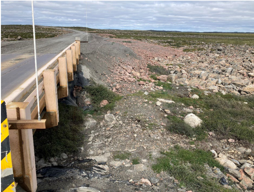
Photograph D3-15 Bridges 8 – R18 km 79+500
