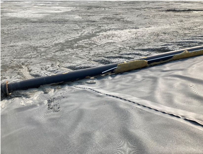
Photograph B6-07 Saddle Dam 4
