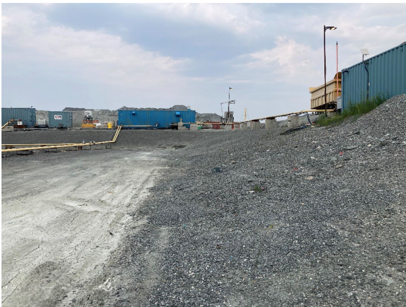
Photograph G2-10 Meadowbank Tank Farm
