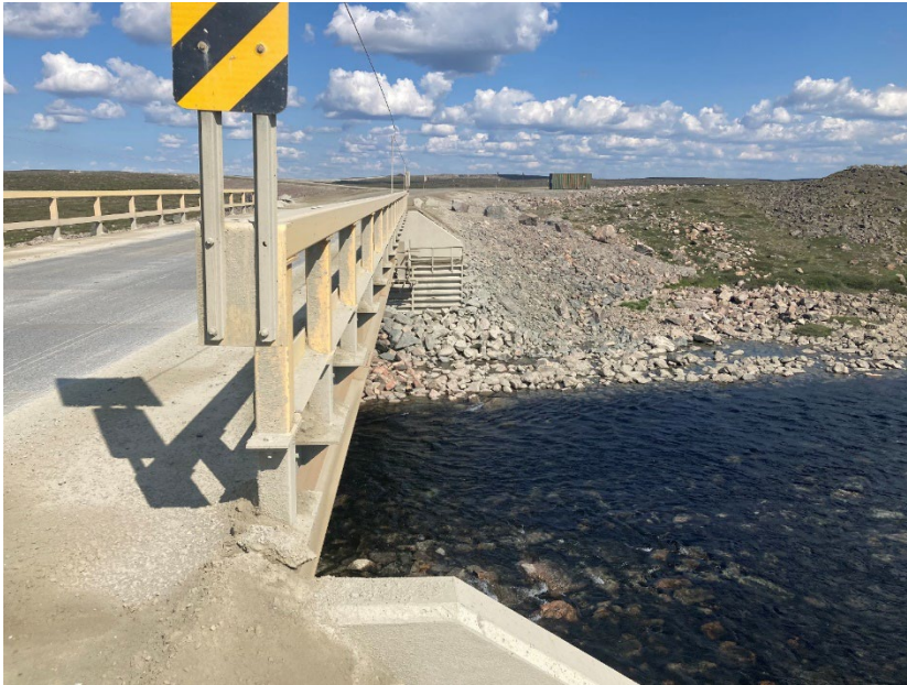
Photograph E2-15 Bridges 7 – km 148+300
