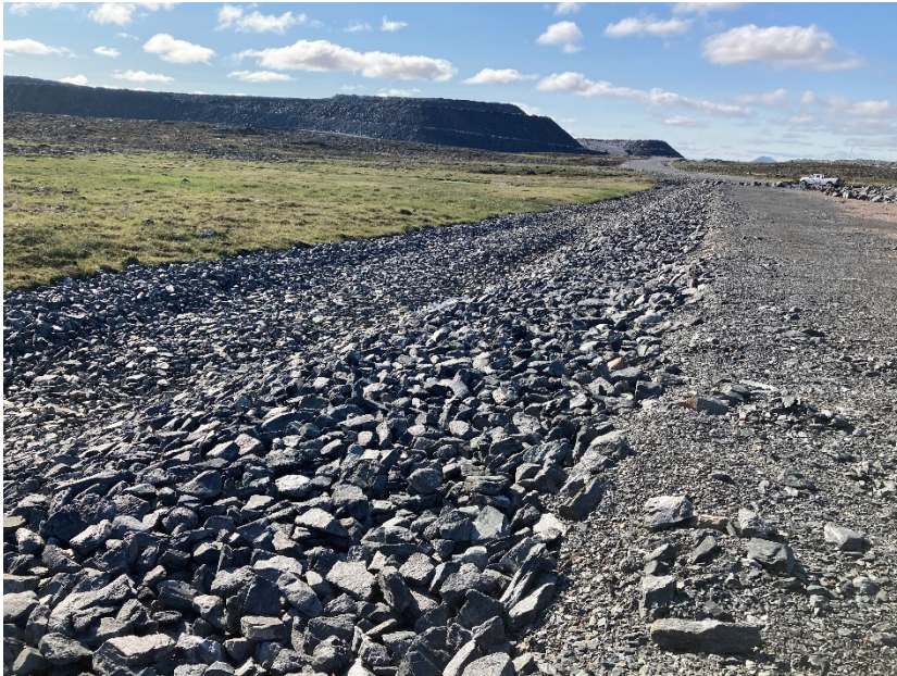
Photograph H13-3 IVR Diversion Channel
