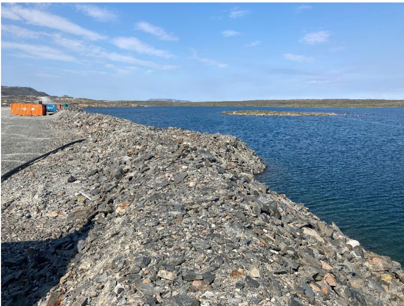
Photograph A1-02 East Dike
