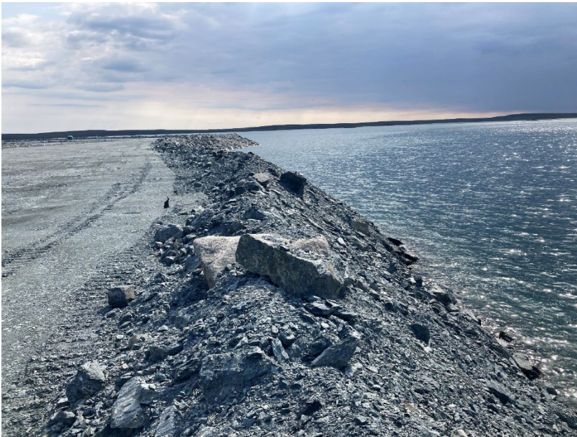
Photograph A3-08 Bay Goose Dike
