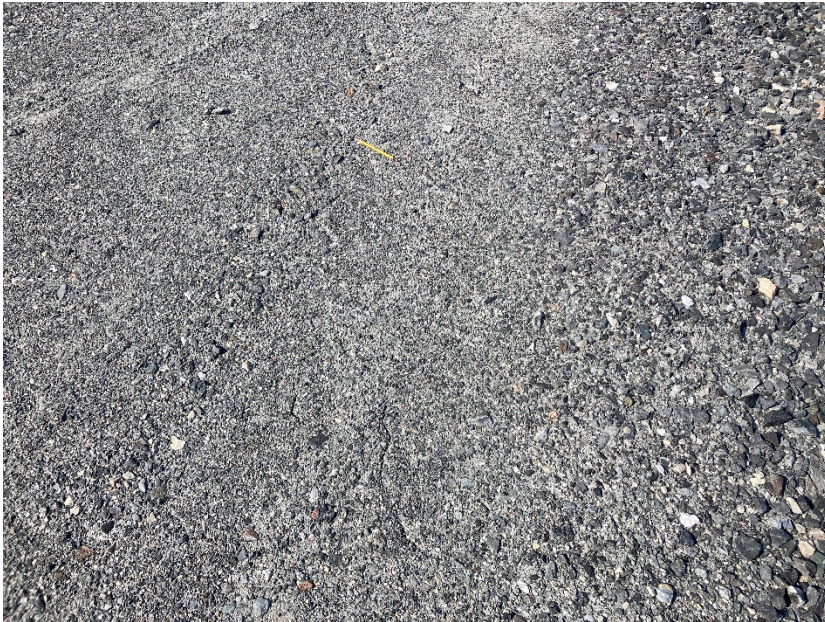
Photograph A1-07 East Dike
