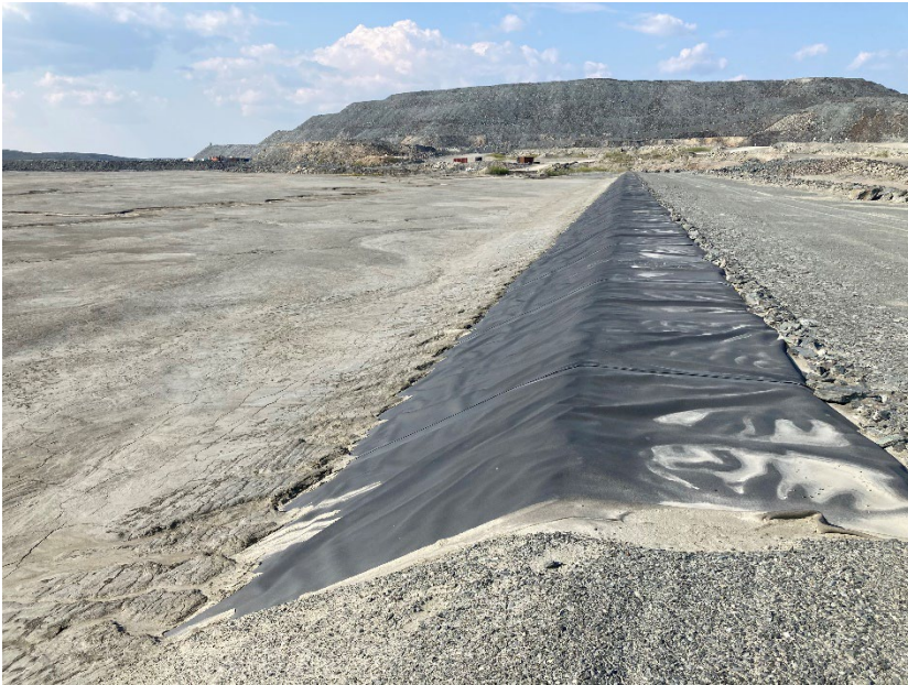
Photograph B7-11 Central Dike and Saddle Dam 5
