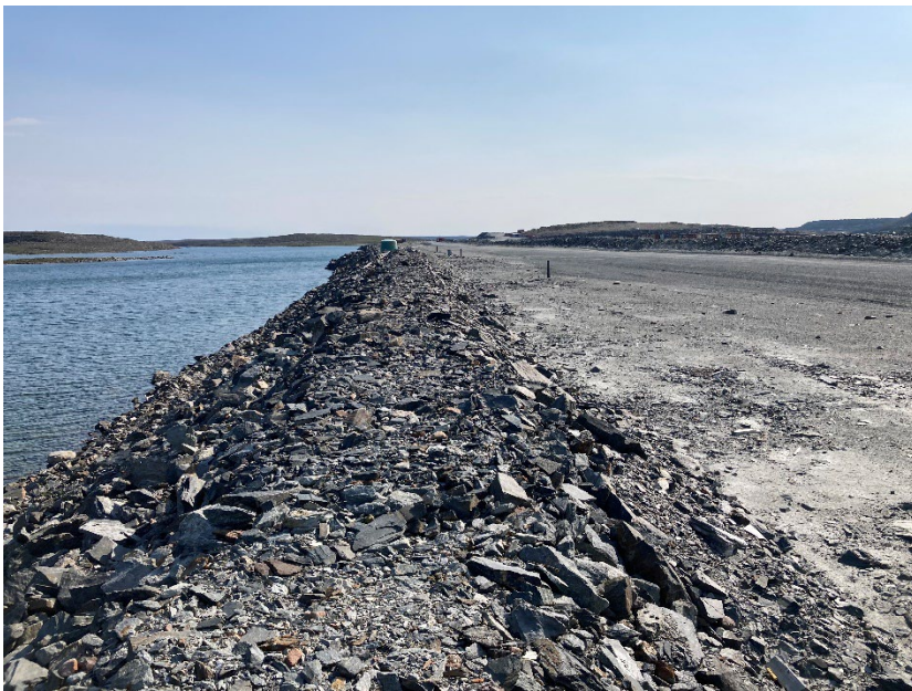
Photograph A1-08 East Dike
