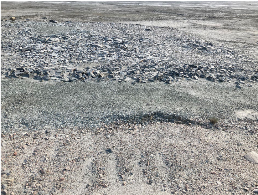
Photograph B6-04 Saddle Dam 4
