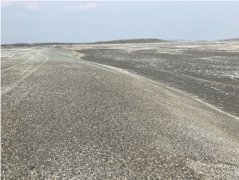
Photograph B1-05 Tailings Storage Facility
