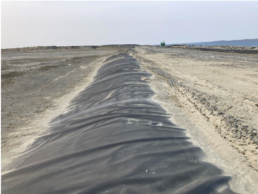
Photograph B2-05 Saddle Dam 1
