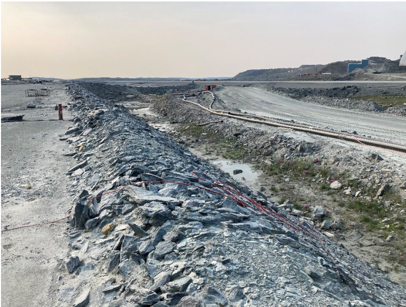
Photograph B6-02 Saddle Dam 4
