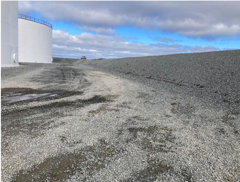
Photograph G1-29 Baker Lake Tank Farm
