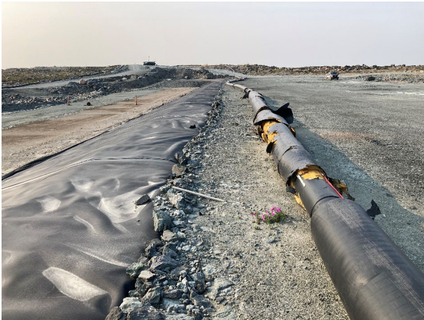
Photograph B5-02 Saddle Dam 3
