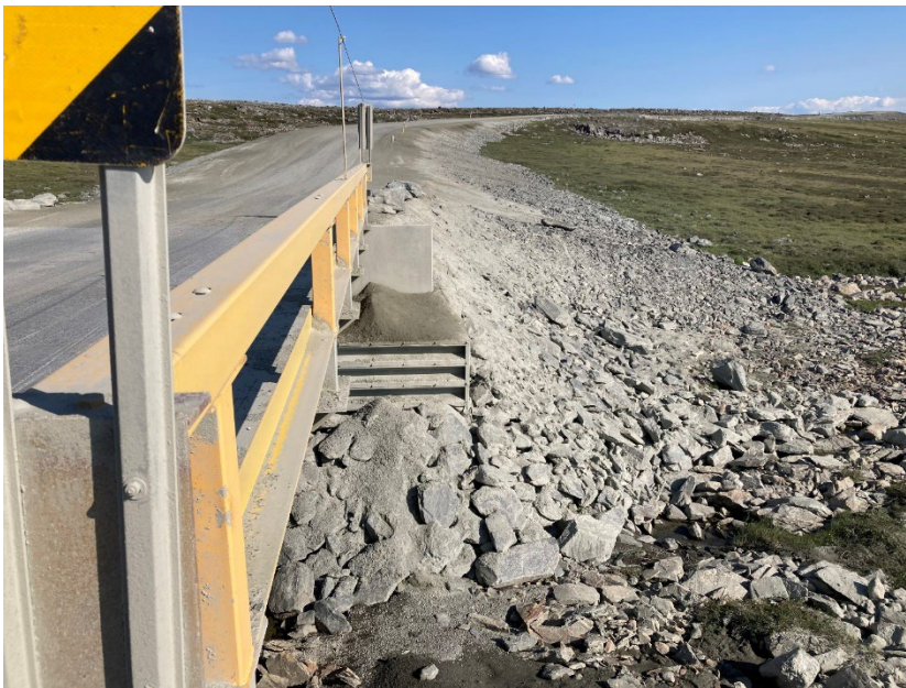
Photograph E2-2 Bridges 1 – km 119+400
