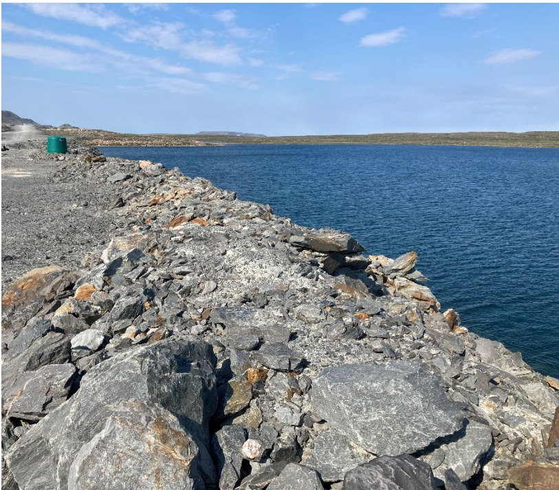
Photograph A1-04 East Dike
