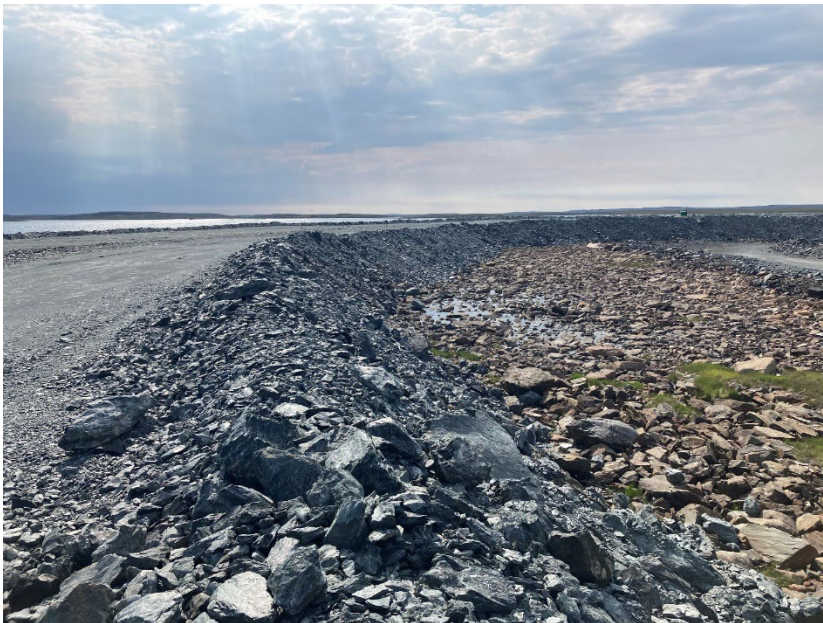
Photograph A3-22 Bay Goose Dike
