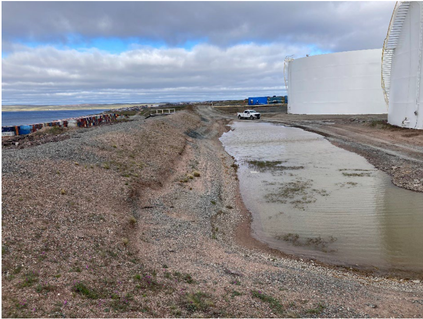
341244 Photograph G1-03 Baker Lake Tank Farm
