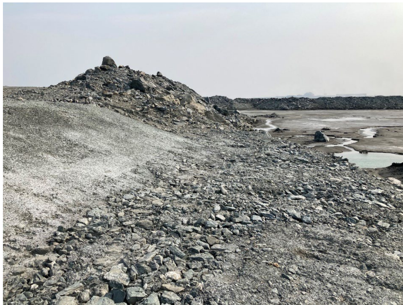
Photograph B1-14 Tailings Storage Facility
