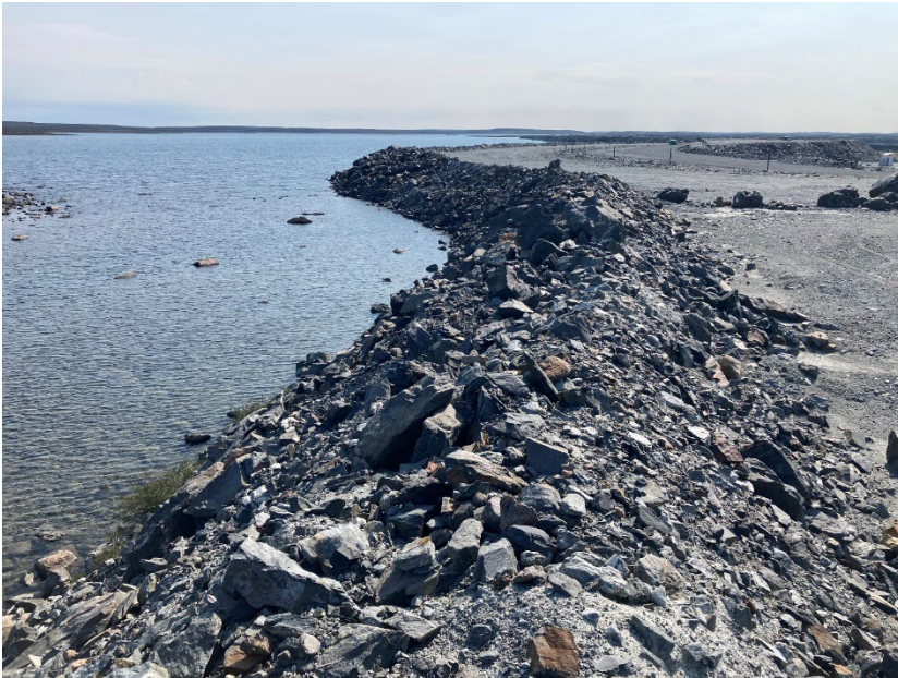
Photograph A3-35 Bay Goose Dike
