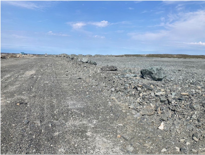
Photograph B4-05 Stormwater Dike
