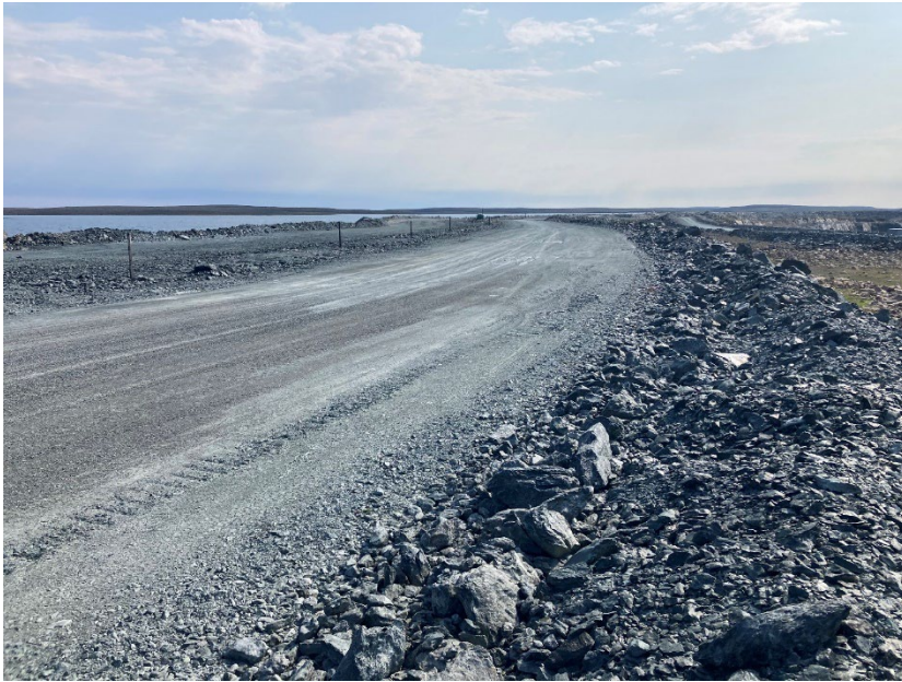
Photograph A3-31 Bay Goose Dike
