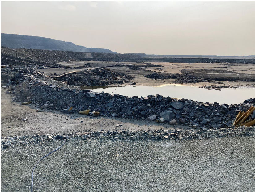
Photograph B5-05 Saddle Dam 3
