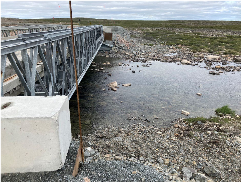
Photograph D3-11 Bridges 6 – R15 km 69+200
