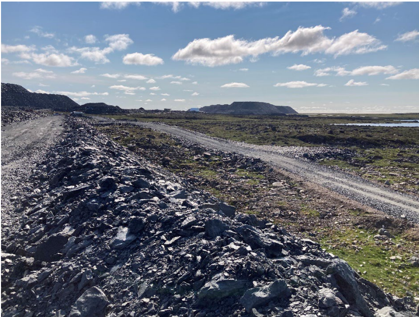
Photograph A7-10 WRSF Dike
