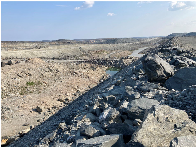
Photograph B7-13 Central Dike and Saddle Dam 5
