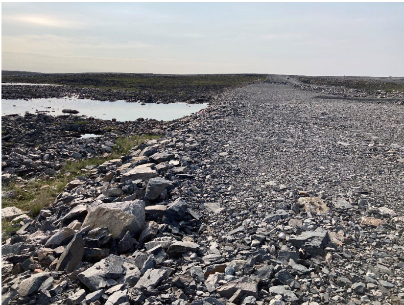
Photograph A4-2 Vault Dike
