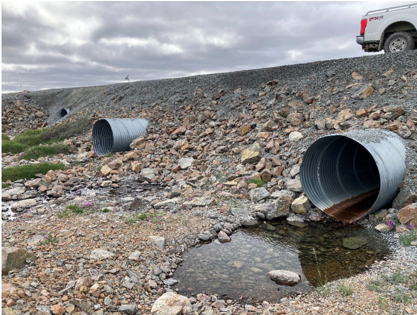
Photograph D2-03: R-14 km 67+840
