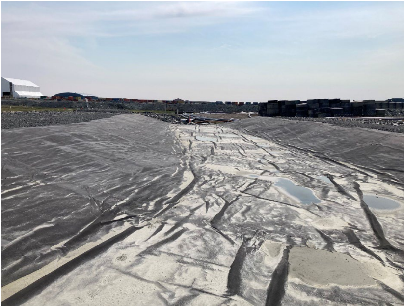
Photograph A6-5 IVR Dike D-1
