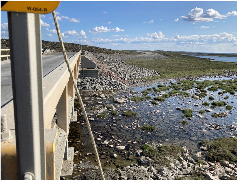
Photograph E2-7 Bridges 3 – km 132+000
