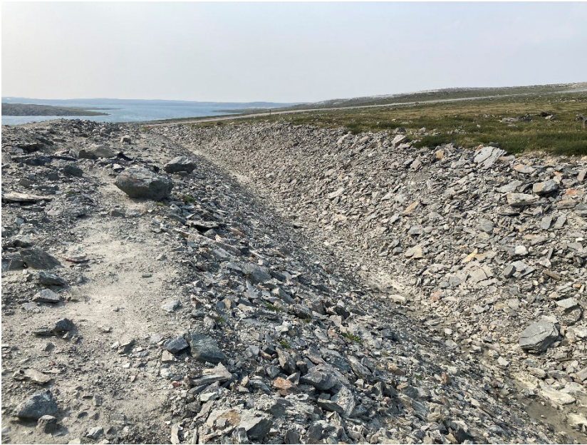
Photograph H2-23 Diversion Ditch and its Sediment and Erosion Protection Structure
