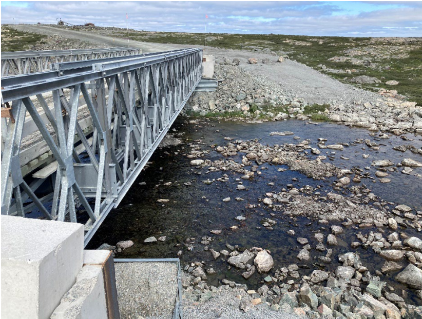
Photograph D3-5 Bridges 3 – R06 km 23+100
