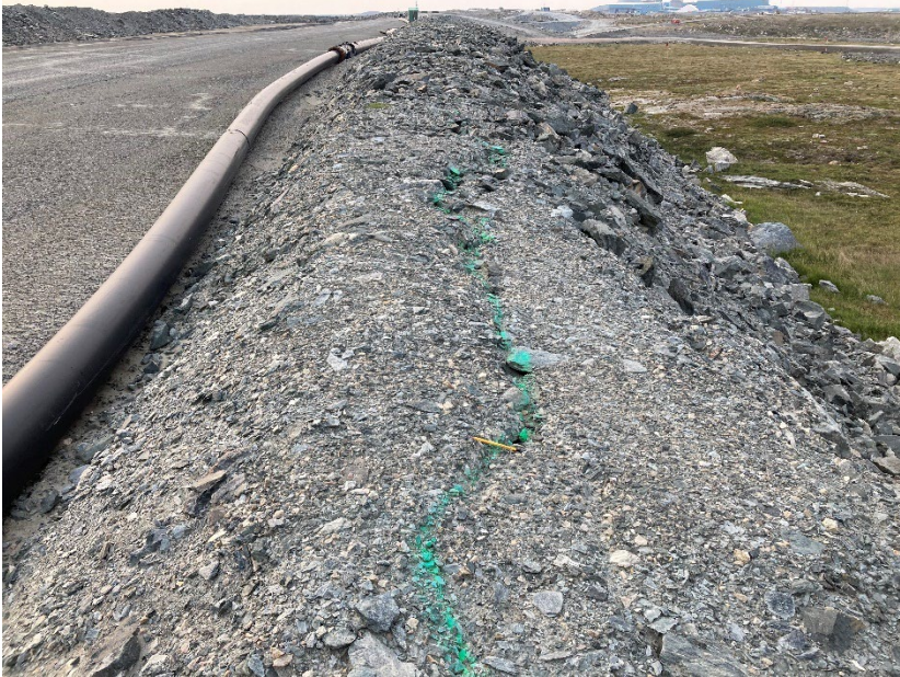
Photograph B3-09 Saddle Dam 2
