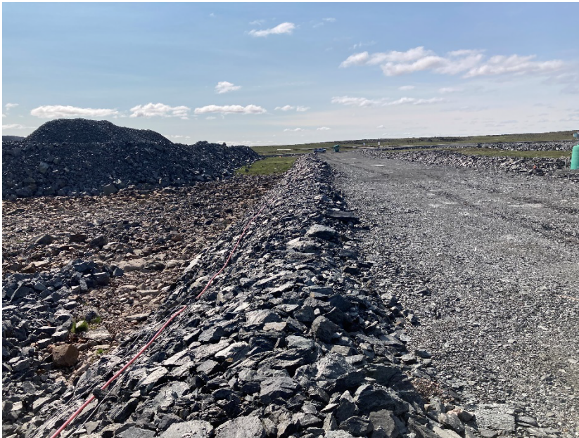
Photograph A8-4 Mammoth Dike
