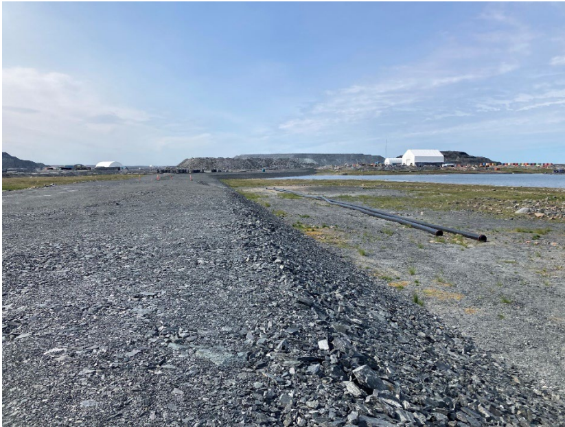
Photograph A6-11 IVR Dike D-1
