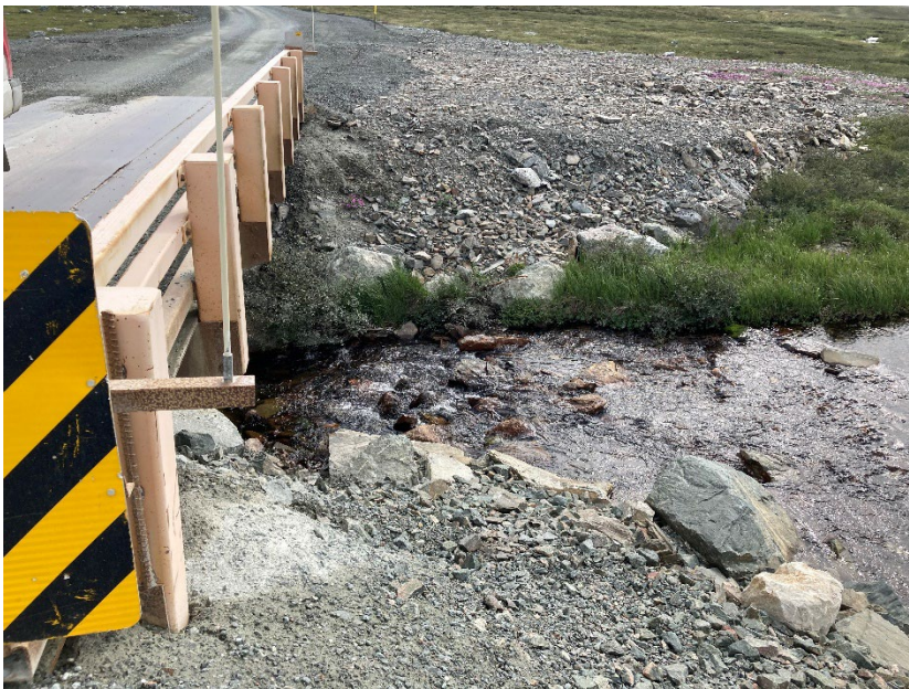
Photograph D3-8 Bridges 4 – R09 km 48+500
