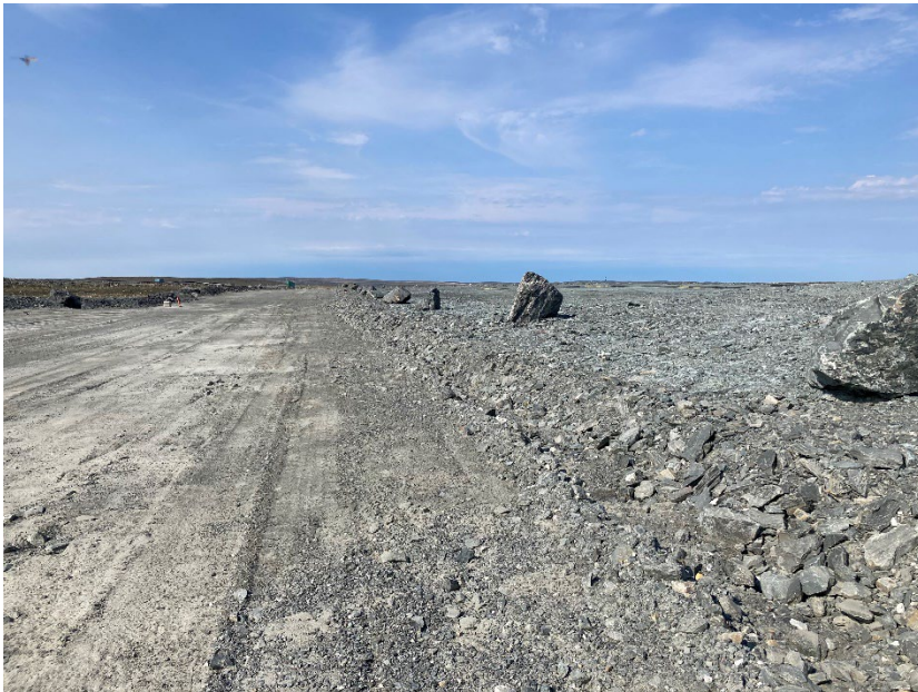
Photograph B4-02 Stormwater Dike
