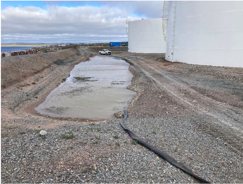
Photograph G1-07 Baker Lake Tank Farm
