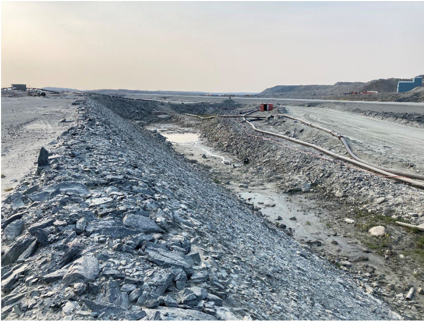
Photograph B6-01 Saddle Dam 4
