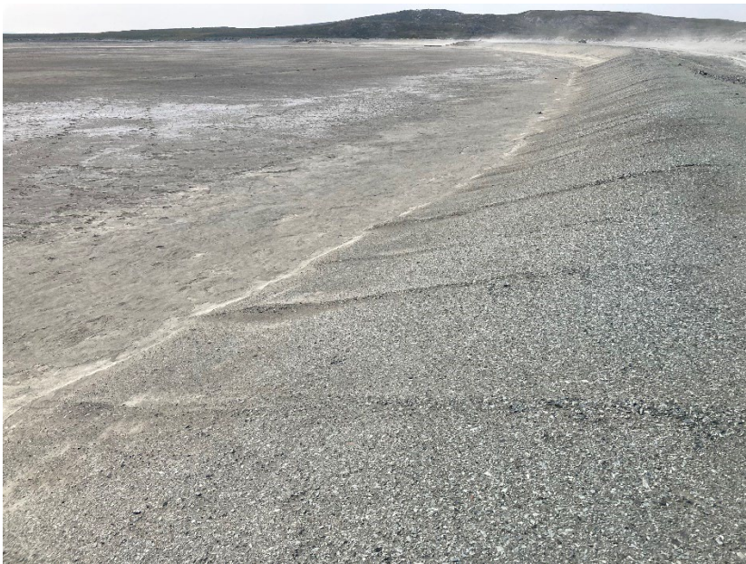
Photograph B1-08 Tailings Storage Facility
