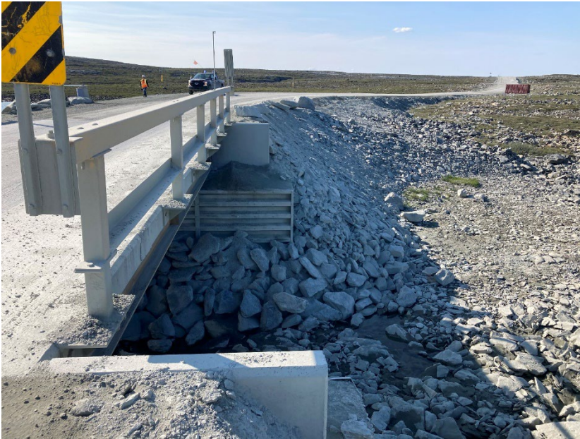
Photograph E2-1 Bridges 1 – km 119+400
