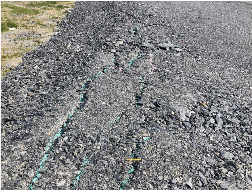
Photograph A6-8 IVR Dike D-1
