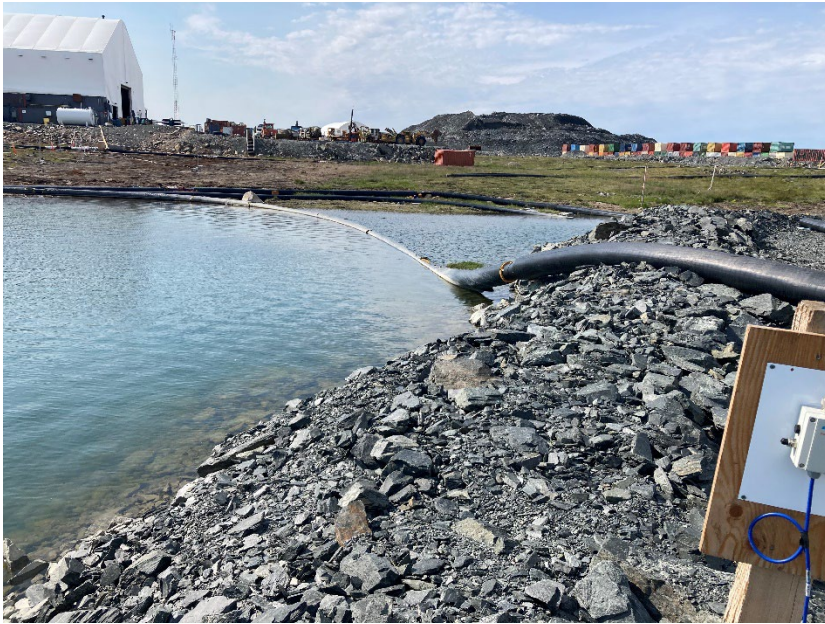
Photograph H8-03 IVR Attenuation Pond Jetty
