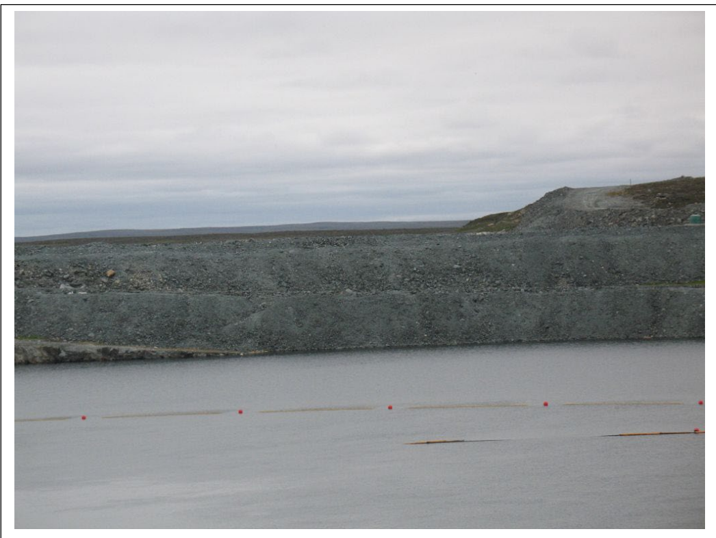
Photo #6 Bay-Goose pit, channels 1 and 2 of Bay-Goose dike.
