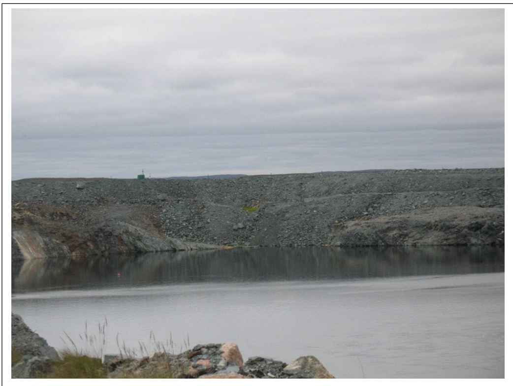
Photo #7 Bay-Goose pit, channel 3 of Bay-Goose dike
