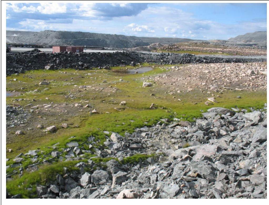
Photo #1 East Dike toe area at 60+550
