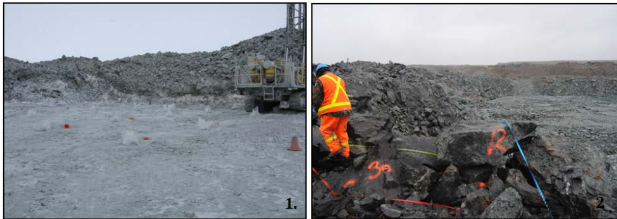
Photo 1: Preparation of the samples from drill cuttings Photo 2: Differentiation of PAG/NAG rock and ore after a blast based on laboratory results and blast pattern
