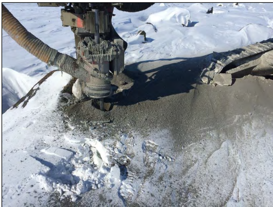
Figure 21: Poor bedrock drilling in SWTC-19-06
