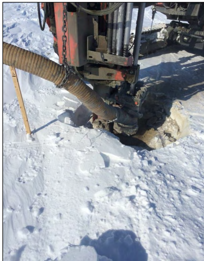
Figure 11: Overburden drilling in SWTC-19-01
