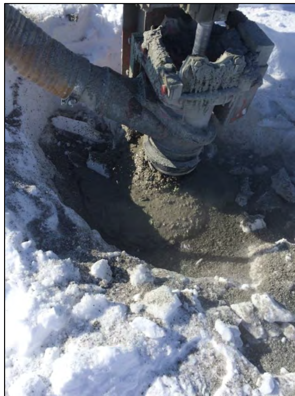
Figure 19: Presence of water in SWTC-19-05
