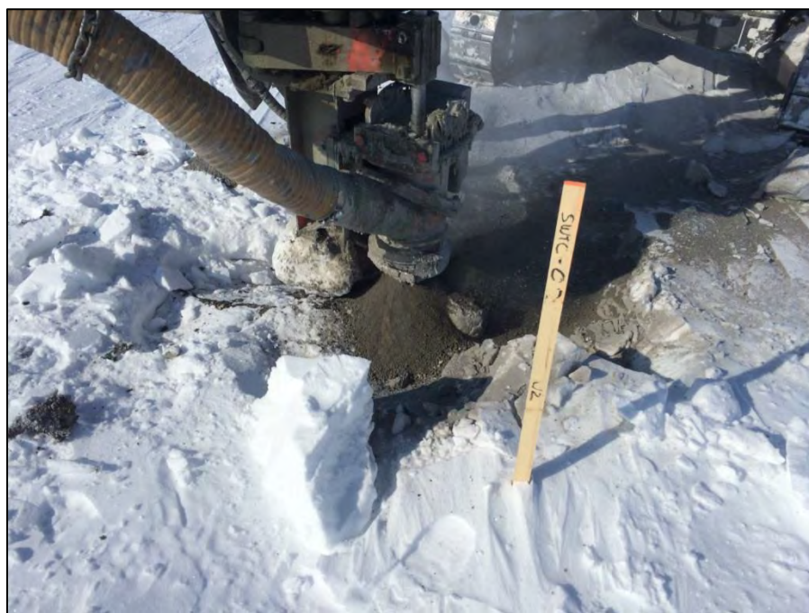
Figure 13: Overburden drilling in SWTC-19-02
