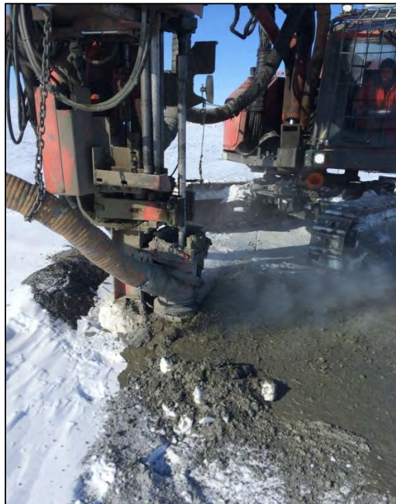
Figure 17: Presence of water in SWTC-19-04
