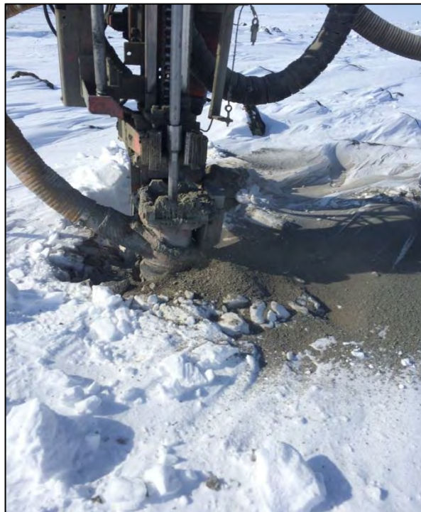
Figure 15: Bedrock drilling in SWTC-19-03
