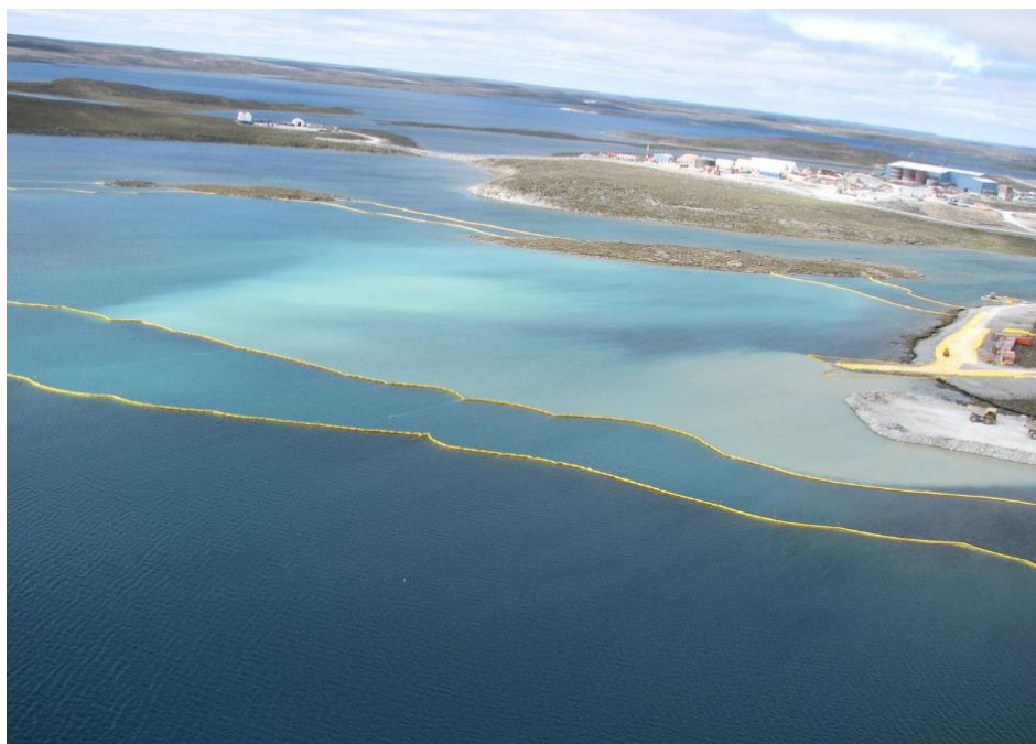
Figure 2 : Typical Sediment Barrier for Turbidity / Sediment containment 1
