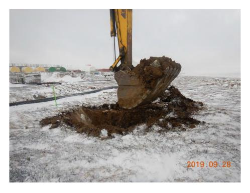
Figure 1: Test pit excavation (IVR-TP2, 2019-09-28).
