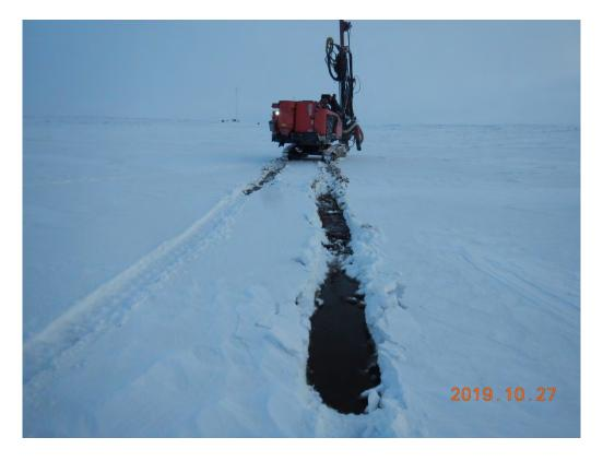
Figure 6: Water in the tracks of the drill between boreholes #14 and 8 (2019-10-27).
